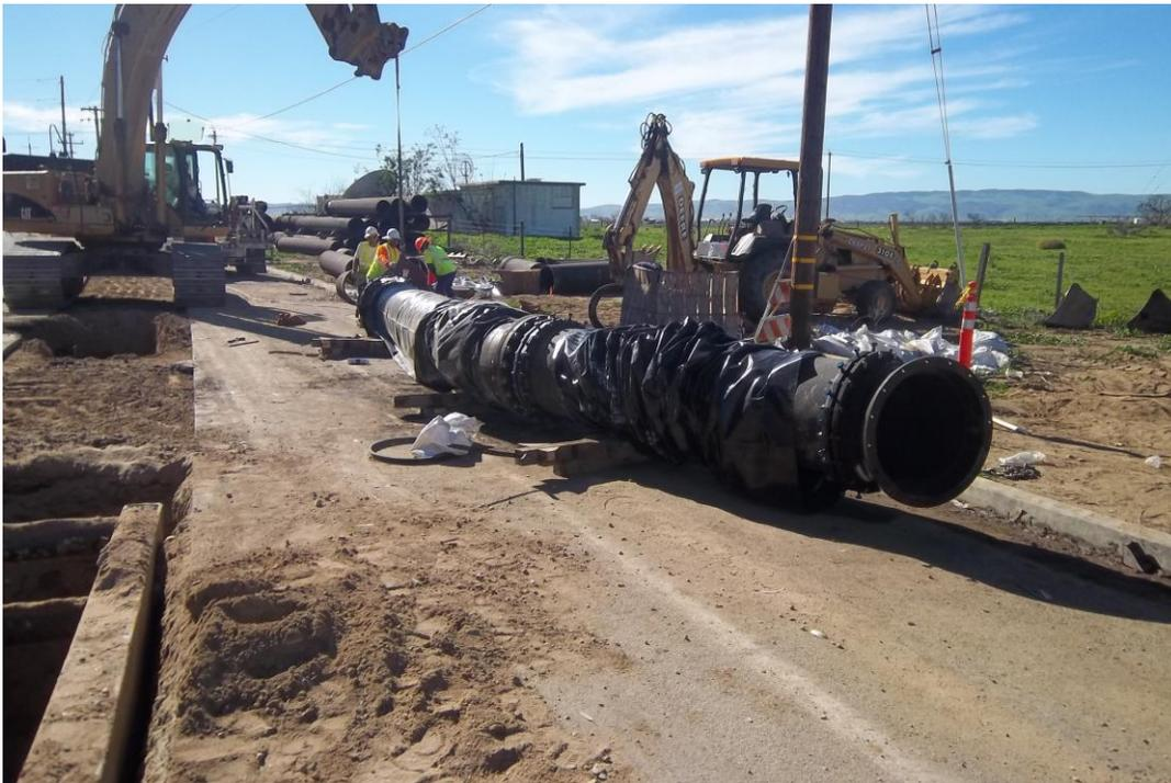
D-KAL bolting up pipe and fittings for 12-inch storm drain crossing.
