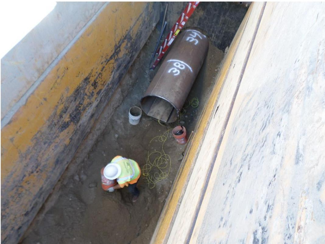
D-KAL removing spoils from inside casing end as it is pushed by the excavator under the 72-inch storm drain crossing.
