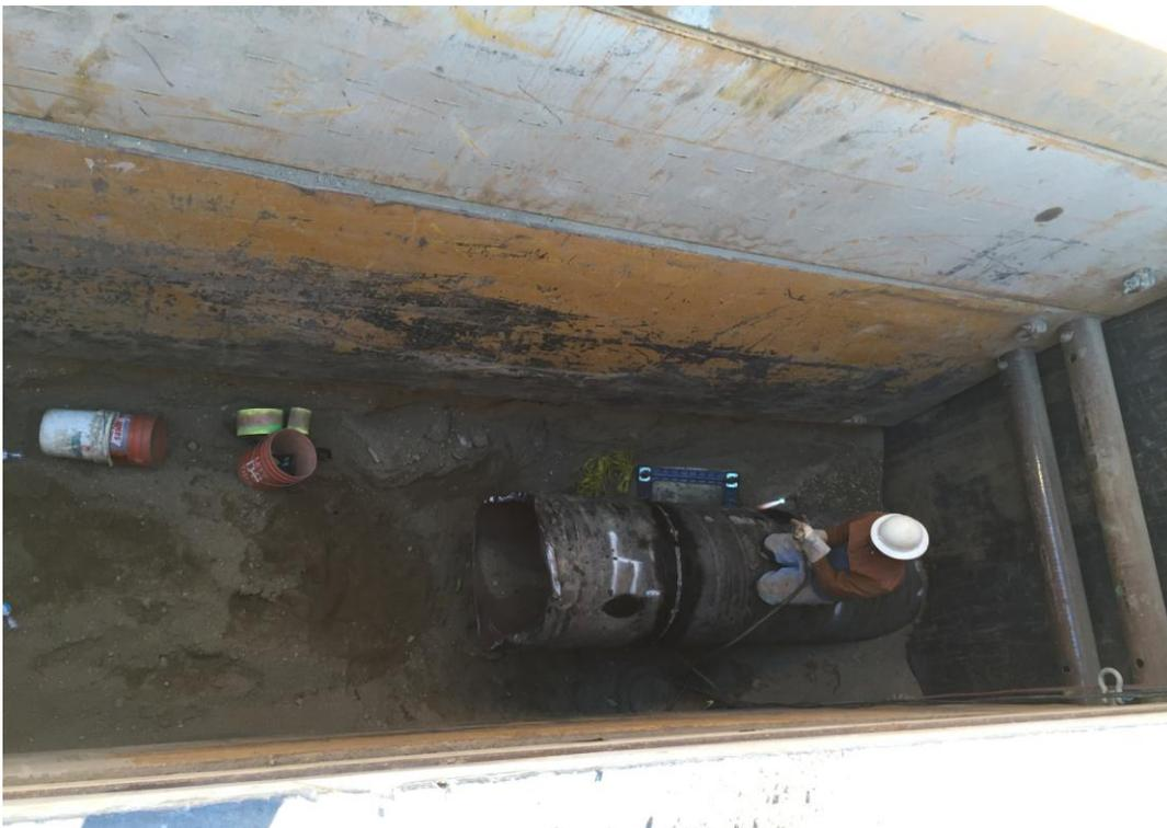
D-KAL cutting off the end of the 36-inch steel casing where it was damaged by the excavator during pushing underneath the 72-inch storm drain crossing.
