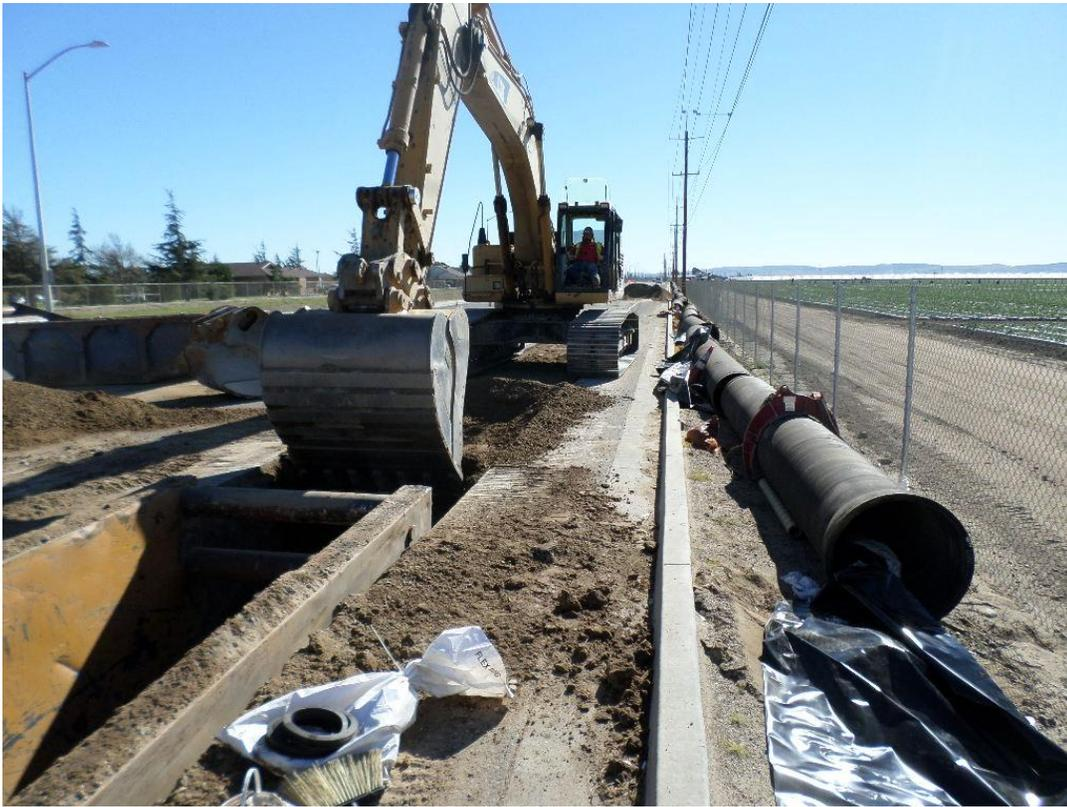
D-KAL continuing installation of the 24-inch DIP in Blosser Road south of the Flow Metering Station to Taylor Street.
