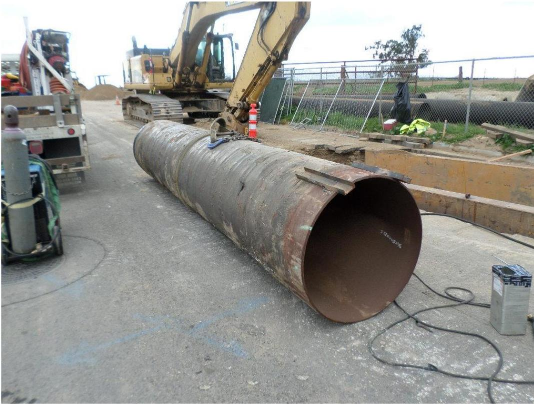
D-KAL preparing to lower next section of 36-inch steel casing into the trench for pushing under the 72-inch storm drain crossing.
