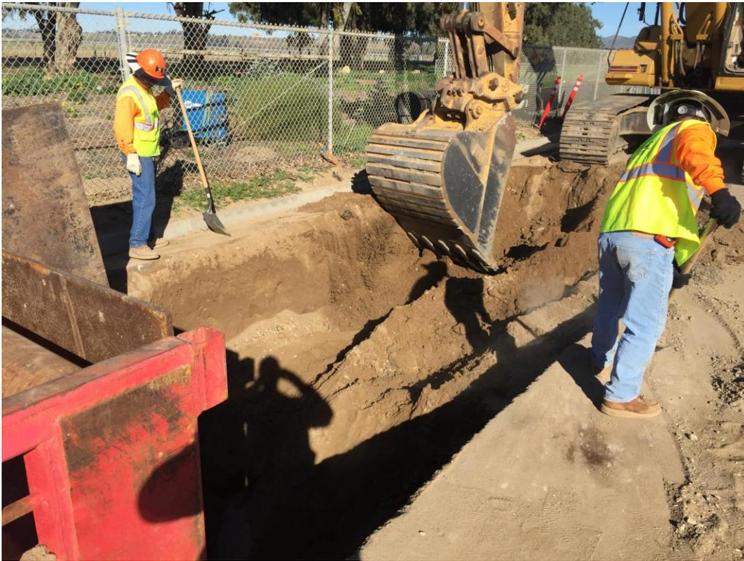
D-KAL excavating up station of the 48-inch storm drain crossing to prepare for pushing the 36-inch steel casing down station to connect to the casing already installed under the 72-inch storm drain.
