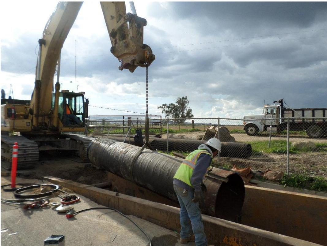
D-KAL lowering next section of 36-inch steel casing into the trench.
