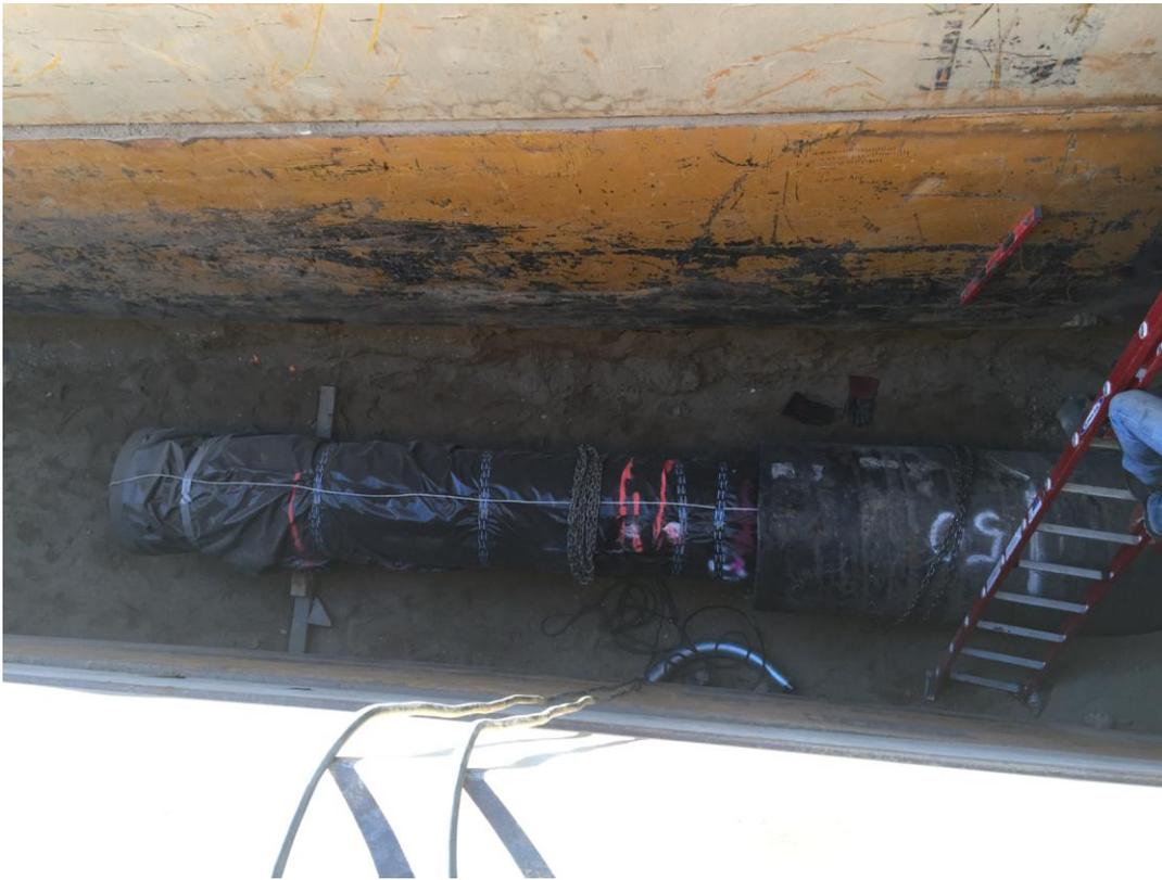
24-inch DIP pushed through 36-inch steel casing.
