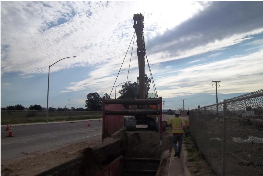
D-KAL removing shields as the space between the storm drain crossings is backfilled.
