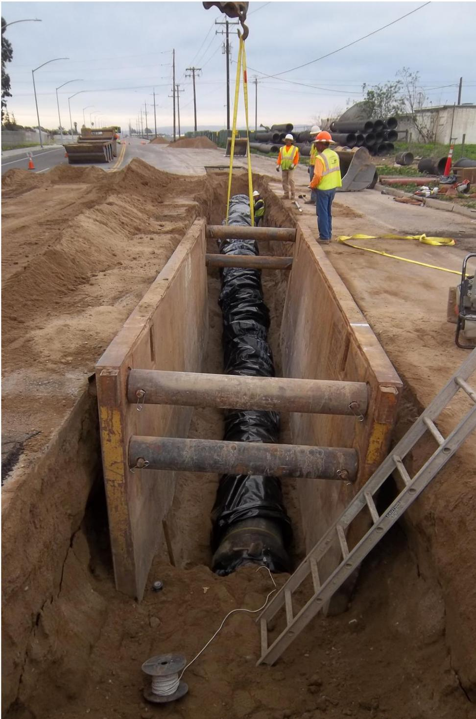
24-inch DIP in place over 12-inch storm drain crossing.
