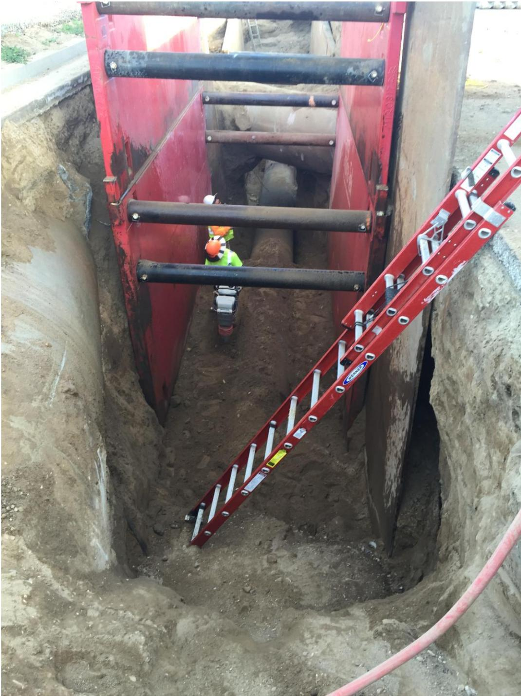
D-KAL compacting around the 36-inch steel casing between the storm drain crossings.
