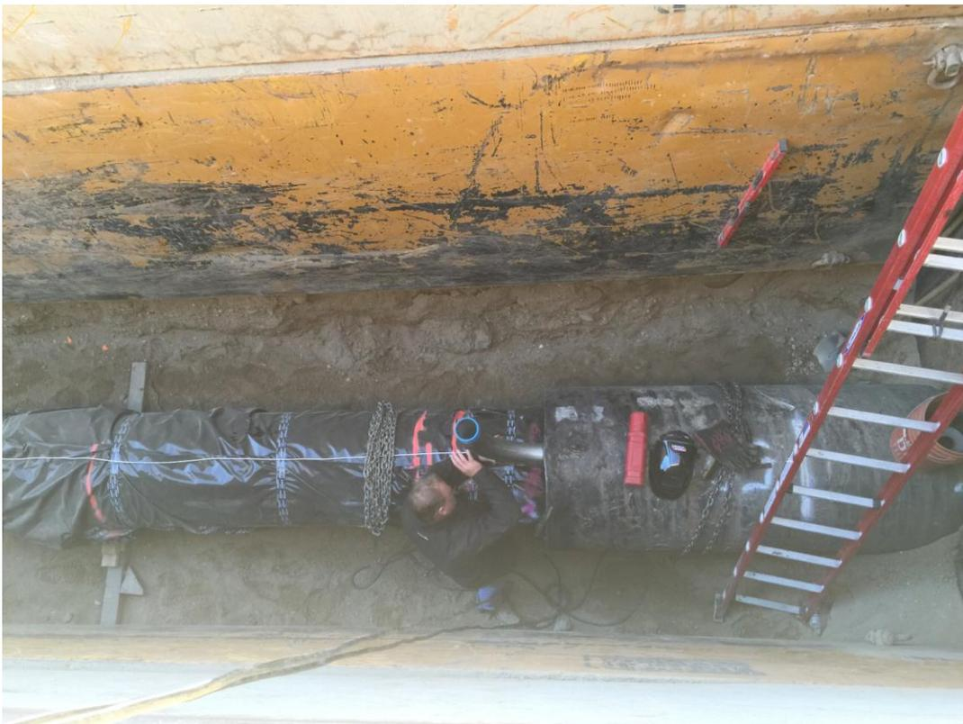
Installing 90 degree steel elbow on pipe used for blowing sand into the casing to fill the annular space around the 24-inch DIP.
