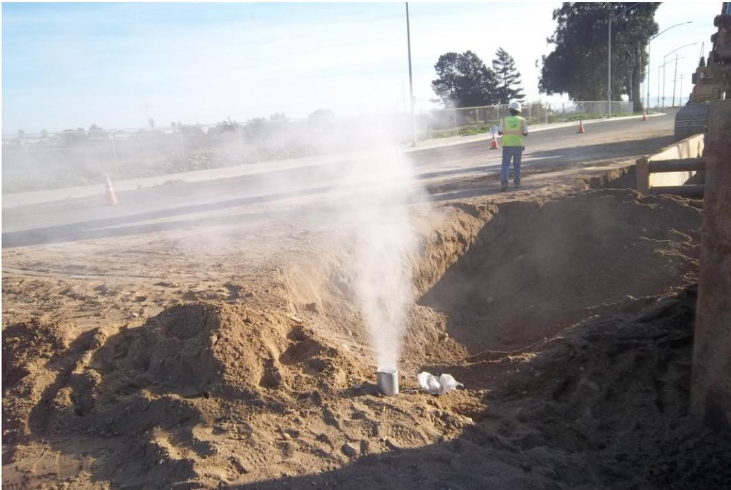
Filling casing annular space with sand. The sand coming out here indicates the casing is full.
