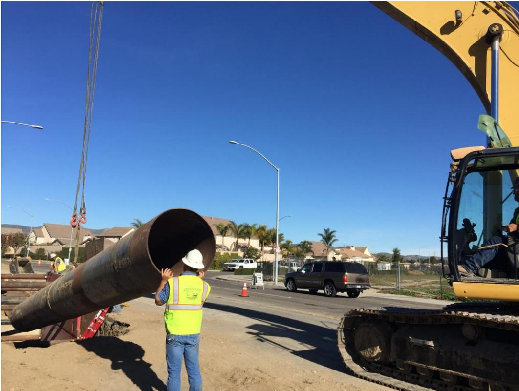
D-KAL installing a 35 foot section of 36-inch steel casing pipe.
