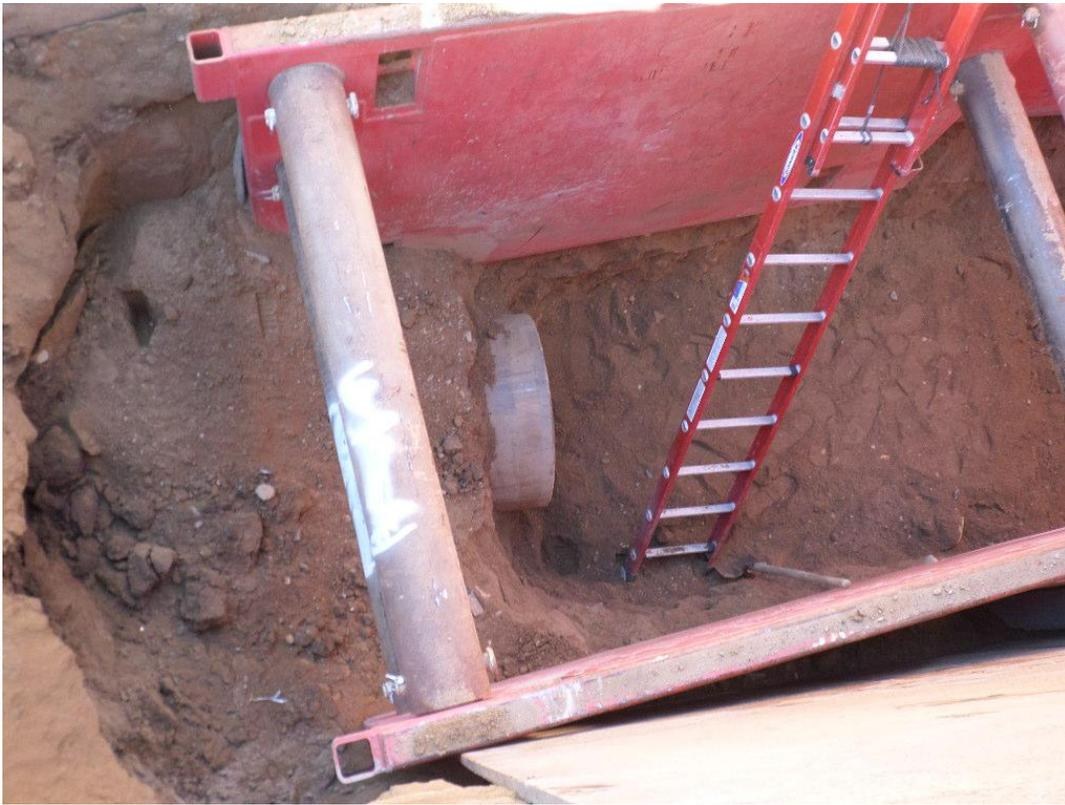
End of 36-inch steel casing after being pushed under the 72-inch storm drain crossing.
