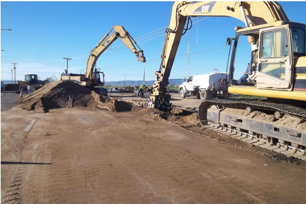
D-KAL compacting trench over 24-inch DIP.
