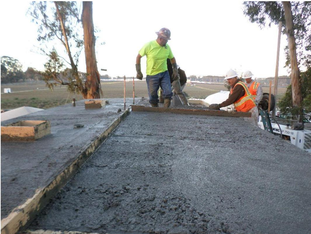
Spieß finishing concrete for the chemical building roof.
