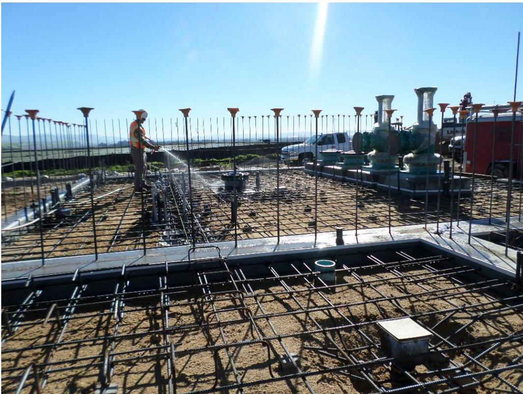
Spieß wetting down the sand and washing off rebar in preparation for the pump station slab pour.
