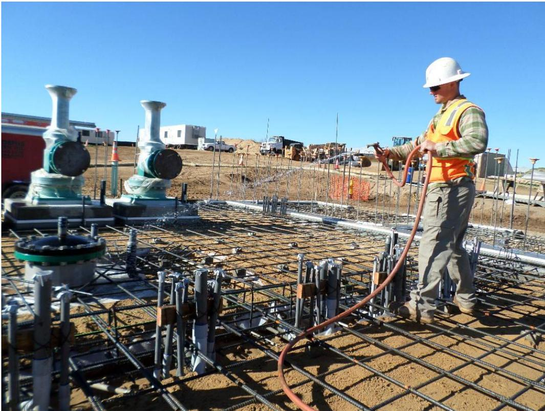
Spieß wetting down sand bedding in preparation for concrete pour of the pump station slab.
