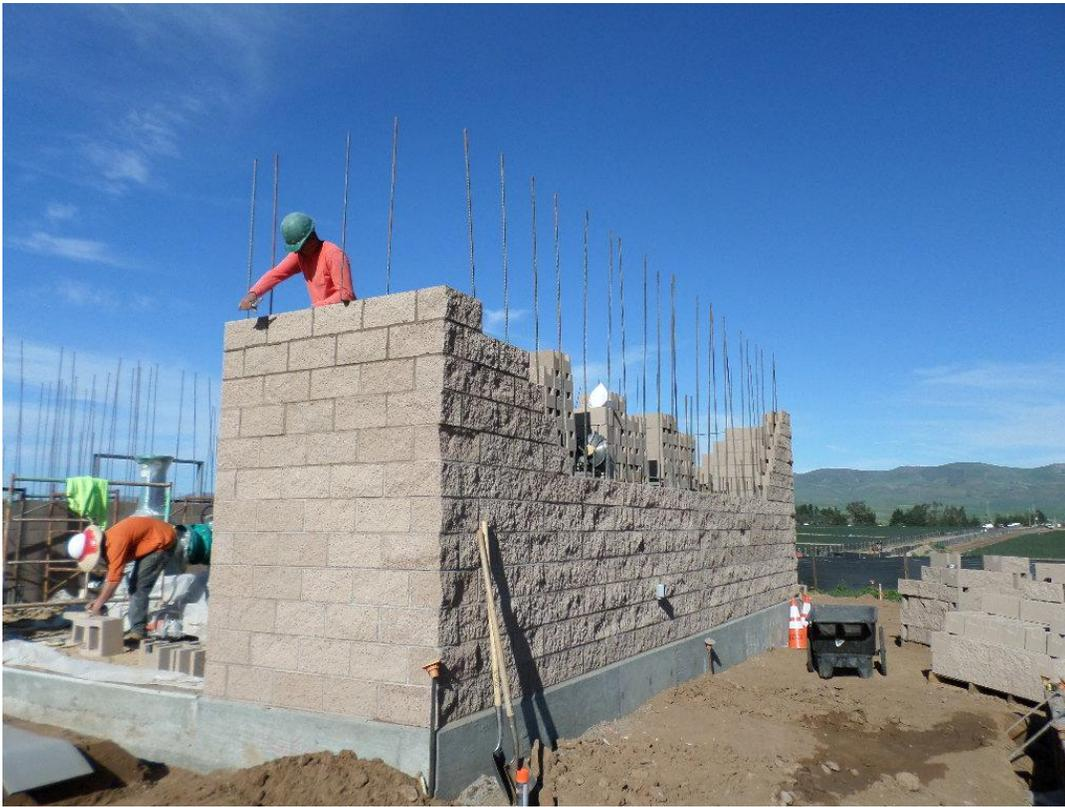
Rocky Boydston Masonry installing second course of block at pump station.
