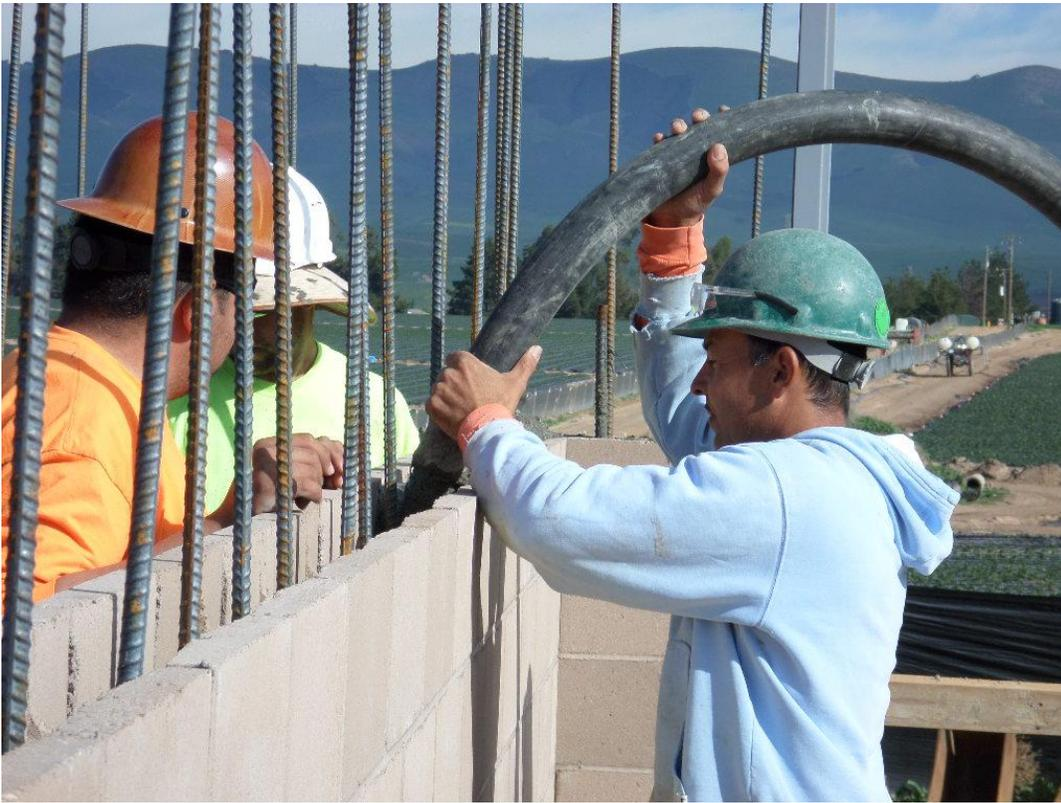
Rocky Boydston Masonry grouting first course of block at the pump station.
