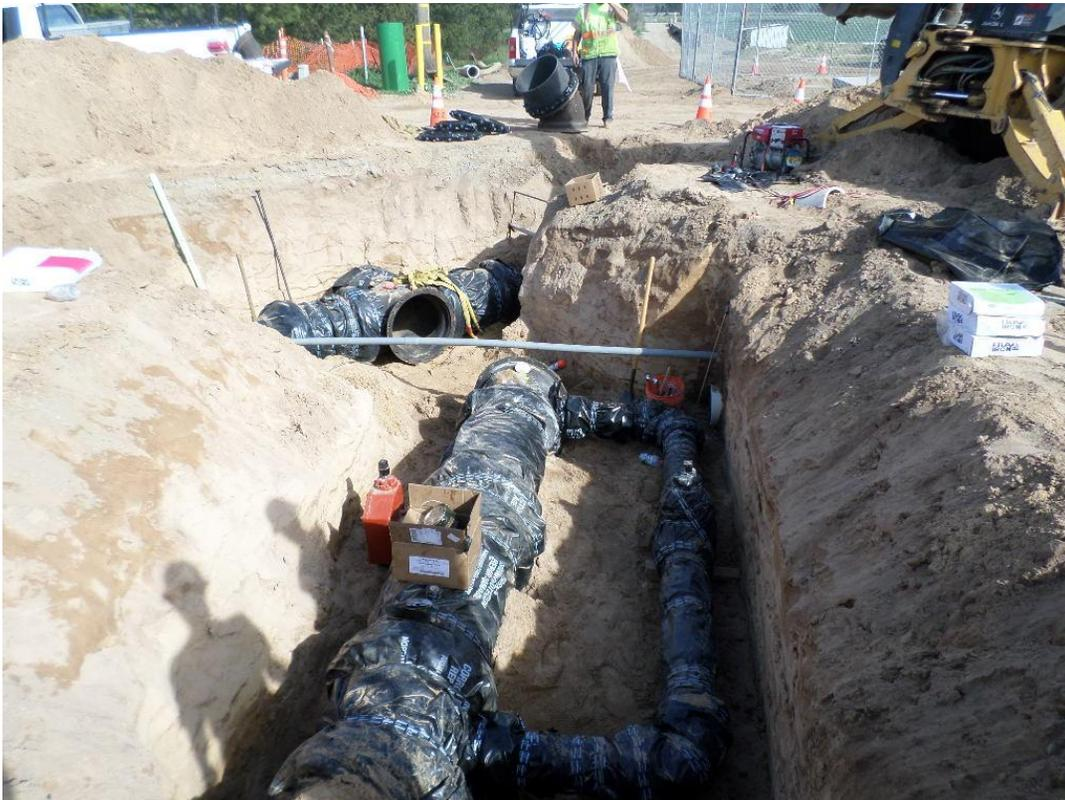
Spieß installing plastic wrap on the 24-inch DIP bypass.
