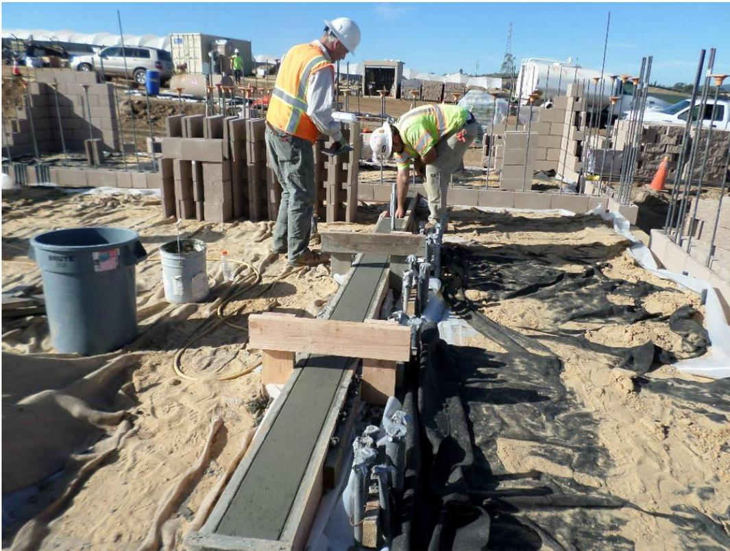
Spieß pouring stem wall for interior metal stud wall at pump station.
