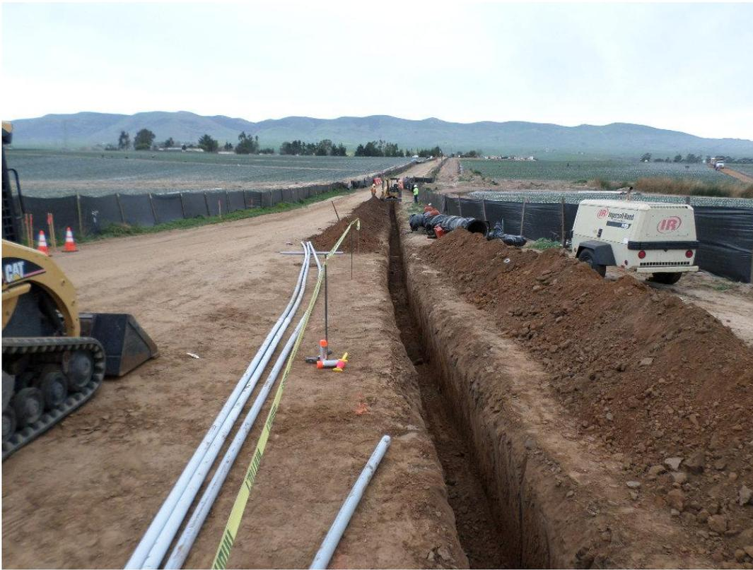
St Dennis Electric installing AT&T conduit in access road.
