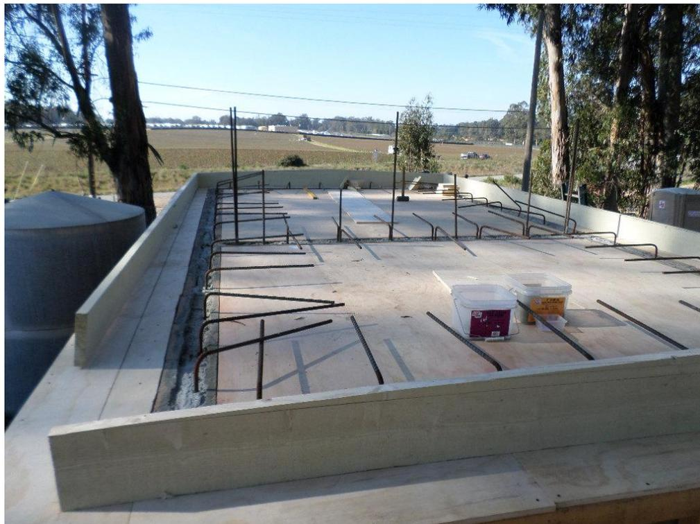
Spiess installing forms for the chemical roof pour.
