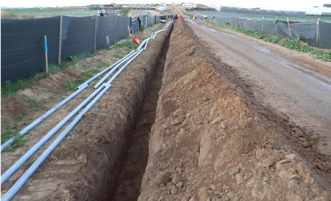
St. Dennis Electric installing AT&T conduit in access road.
