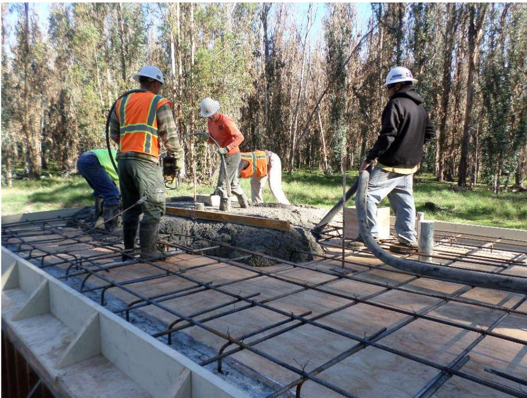
Spieß pouring concrete for the chemical building roof.
