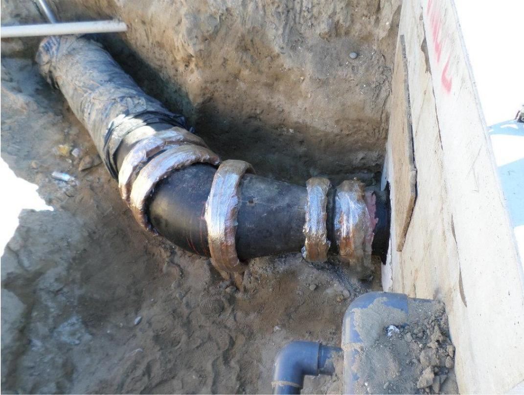
Wax tape applied after new 45 degree elbows were installed.
