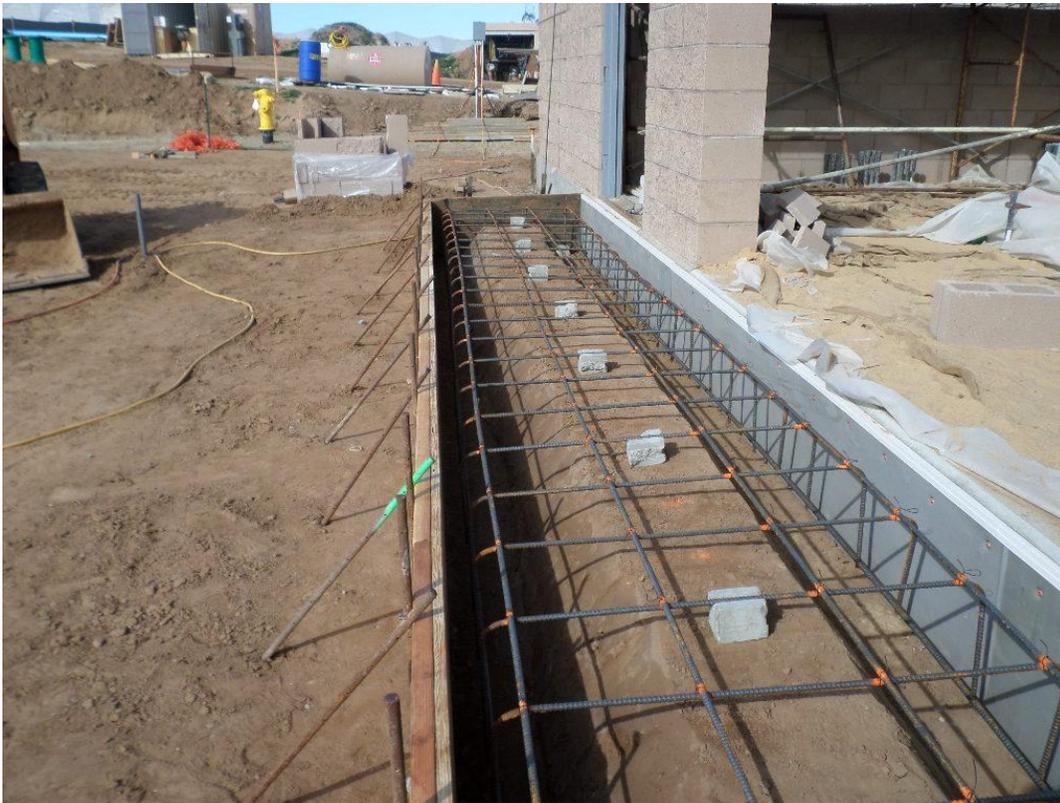
Forms and reinforcing for concrete landing at roll-up door.
