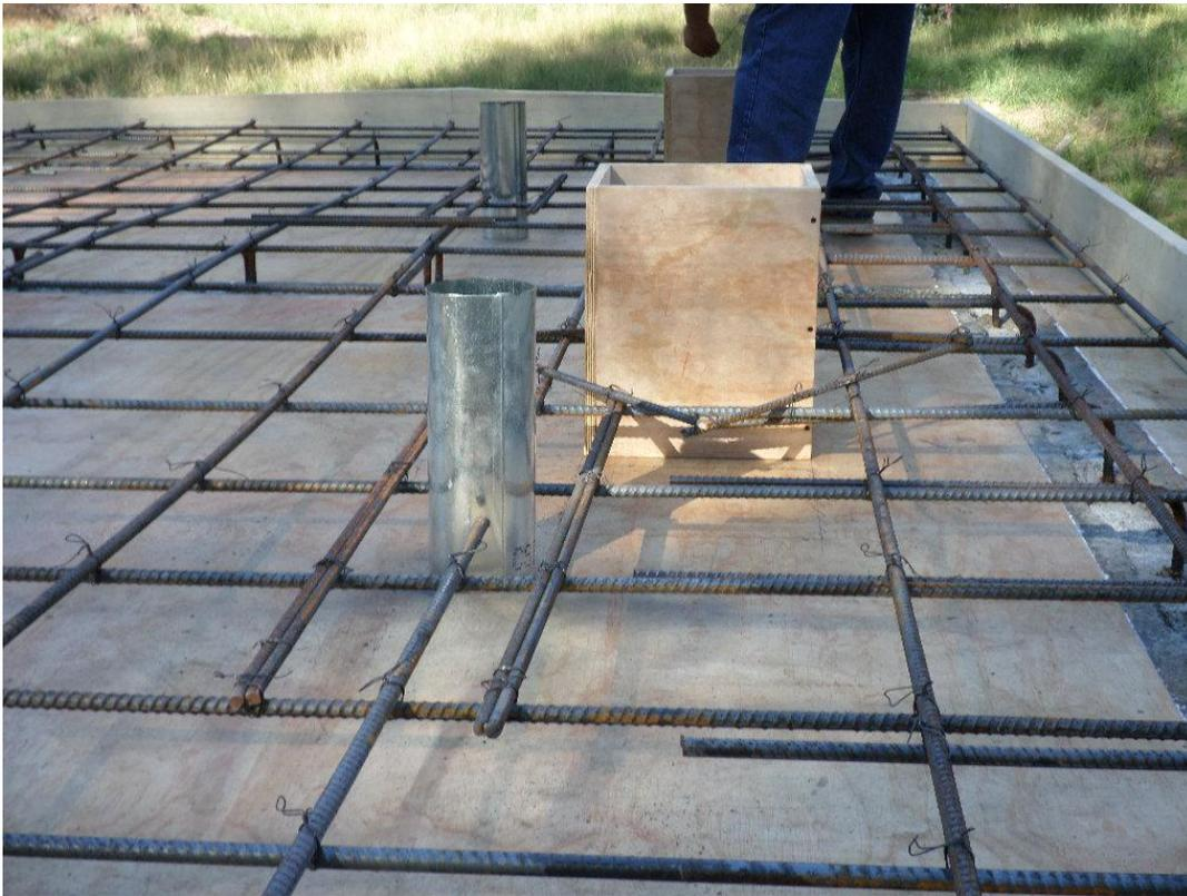
Spieß installing vent piping for the chemical building roof pour.
