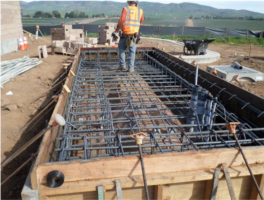
Vista Steel installing reinforcing for the emergency generator pad.
