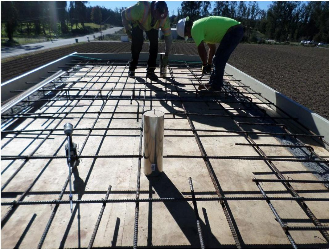
Installing vent sleeves for the chemical building roof pour.
