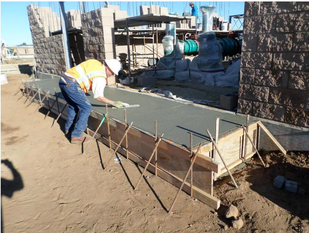
Pouring concrete landings around the pump station building.
