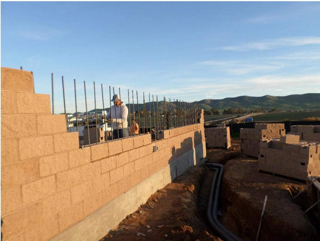
Rocky Boydston Masonry installing the first course of block at the pump station.
