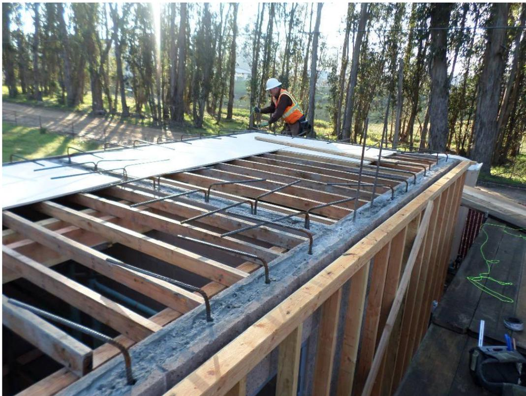
Spiess installing sheeting and false work for chemical building roof pour.
