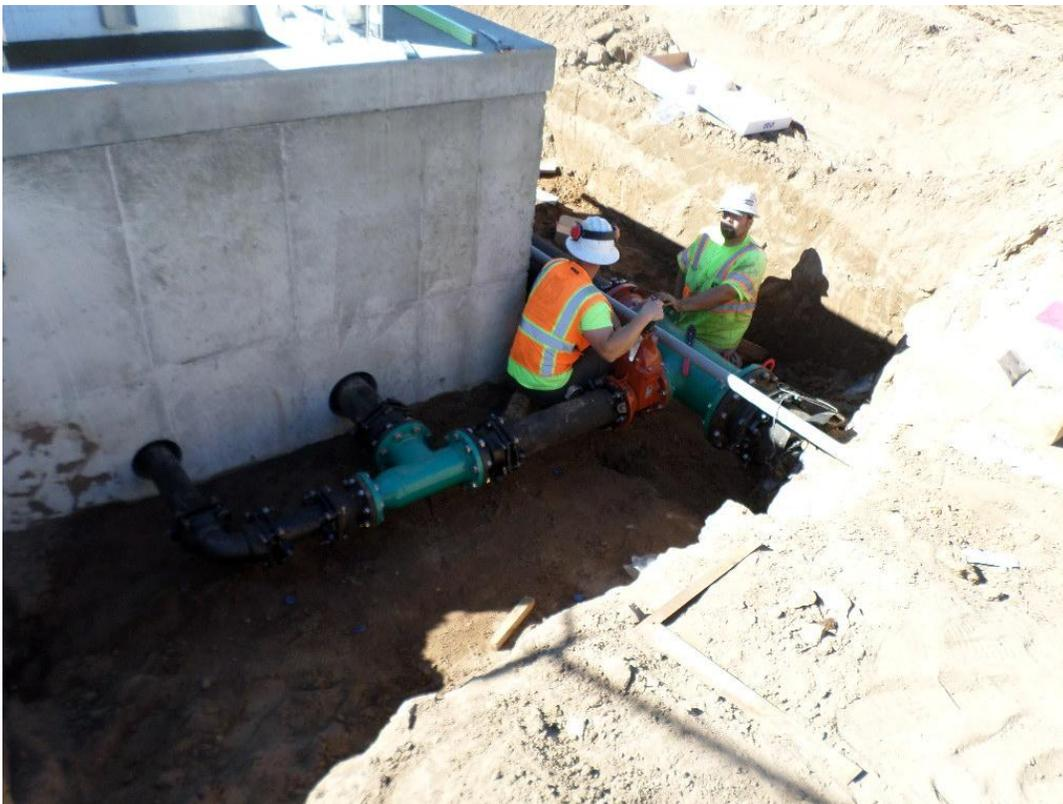
Spiess installing piping at PRV vault.
