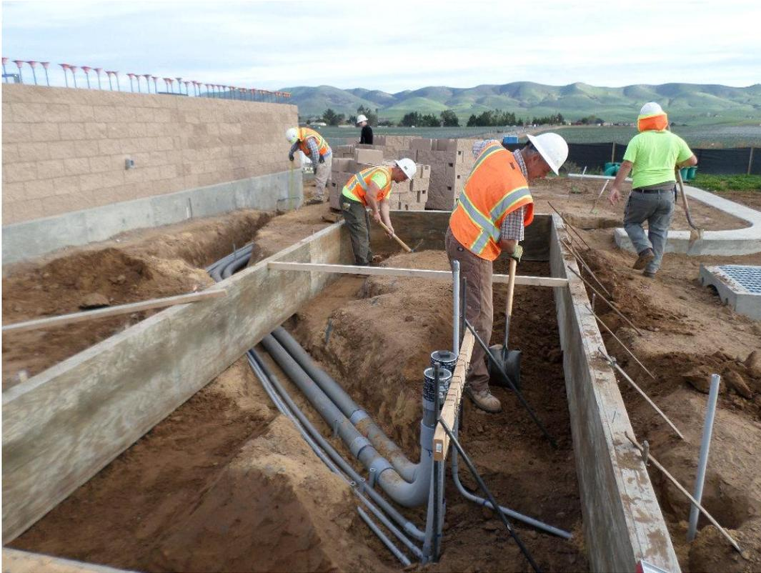
St. Dennis Electric installing conduit for emergency generator and Spiess preparing forms.
