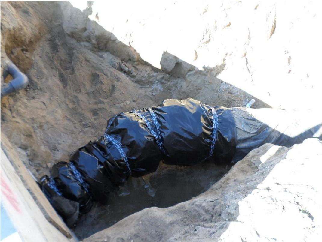
Fittings wrapped with plastic after new 45 degree elbows were installed.
