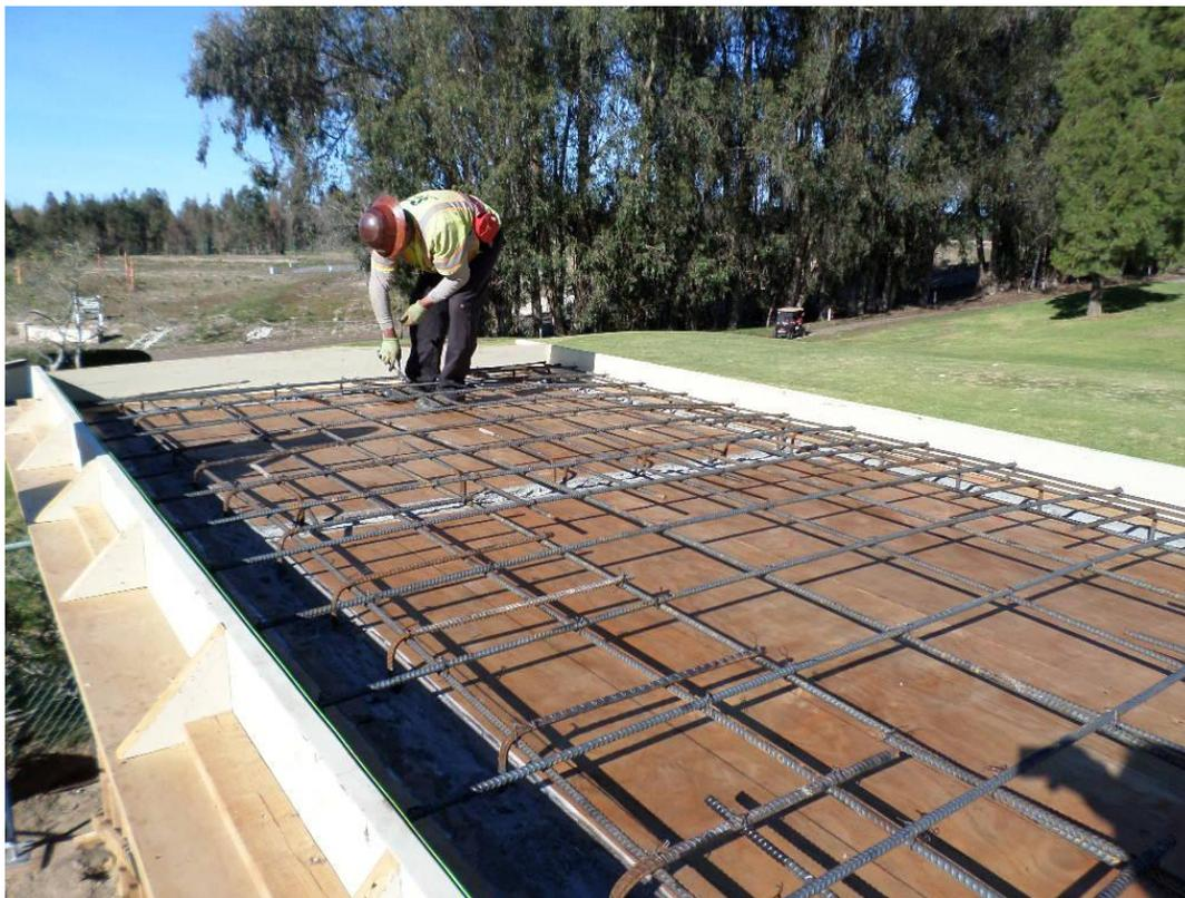
Vista Steel installing reinforcing for the chemical building roof.
