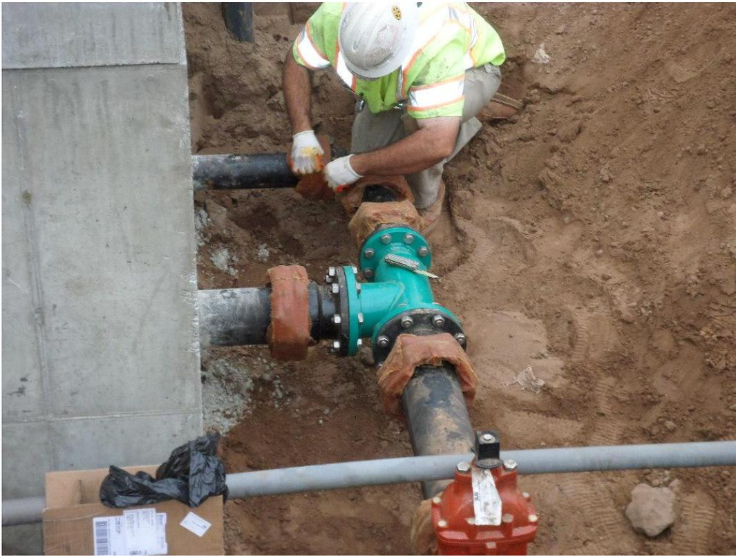
Spiess applying wax tape to piping at PRV vault.
