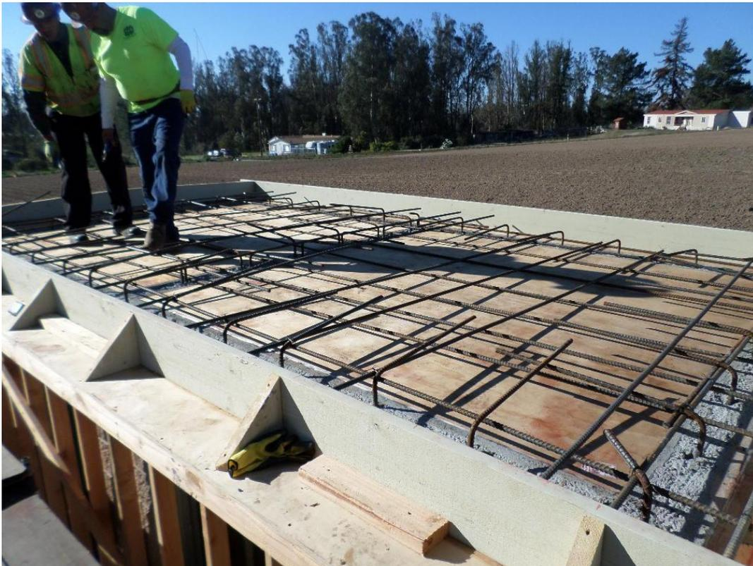
Vista Steel installing reinforcing at the chemical building roof.
