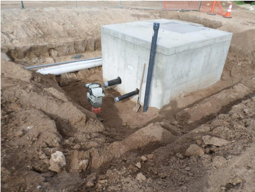
Spiess backfilling around PRV vault.
