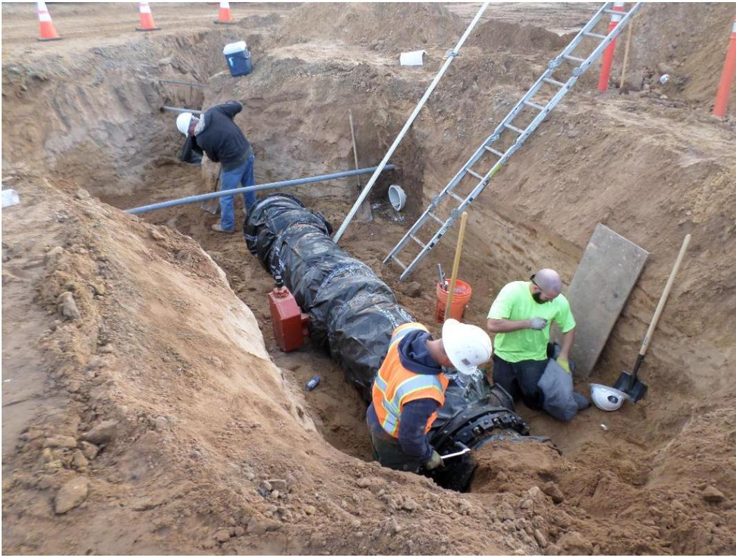
Spieß installing the 24-inch DIP bypass.
