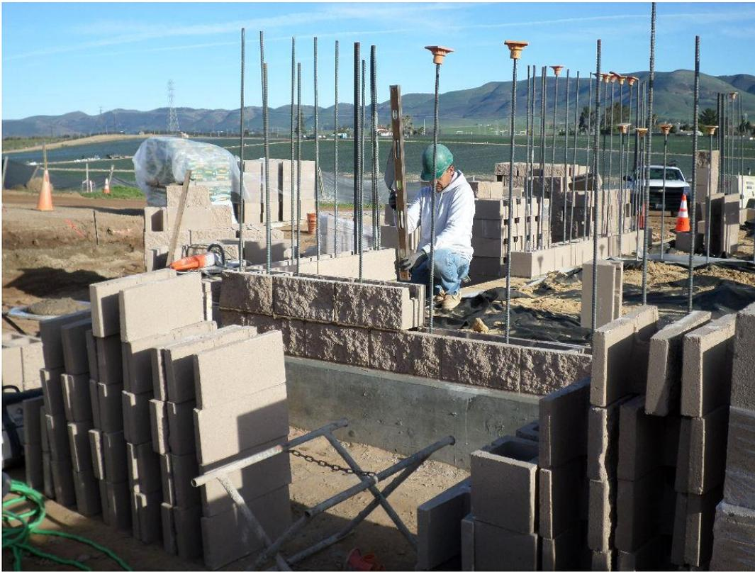
Rocky Boydston Masonry installing first course of block at the pump station.
