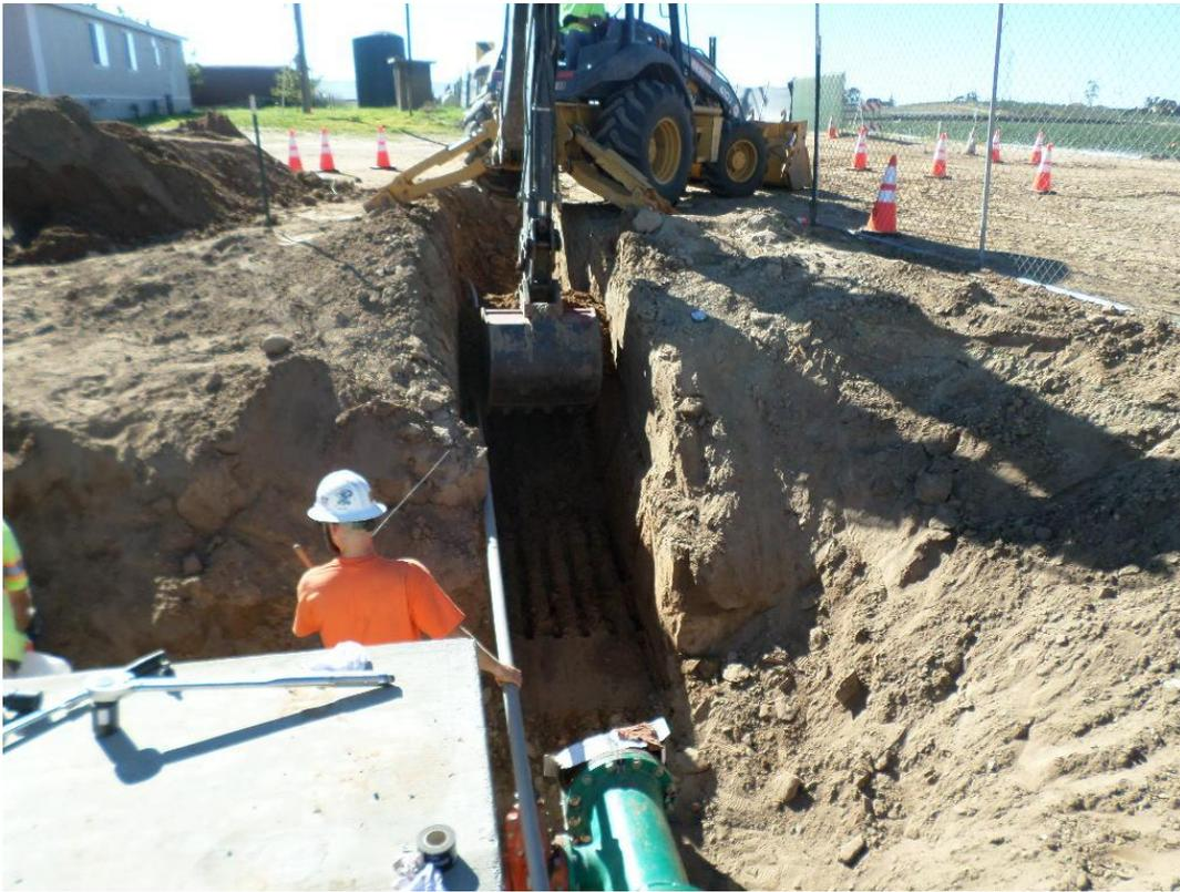
Spiess trenching for installation of the 24-inch DIP near the PRV vault.
