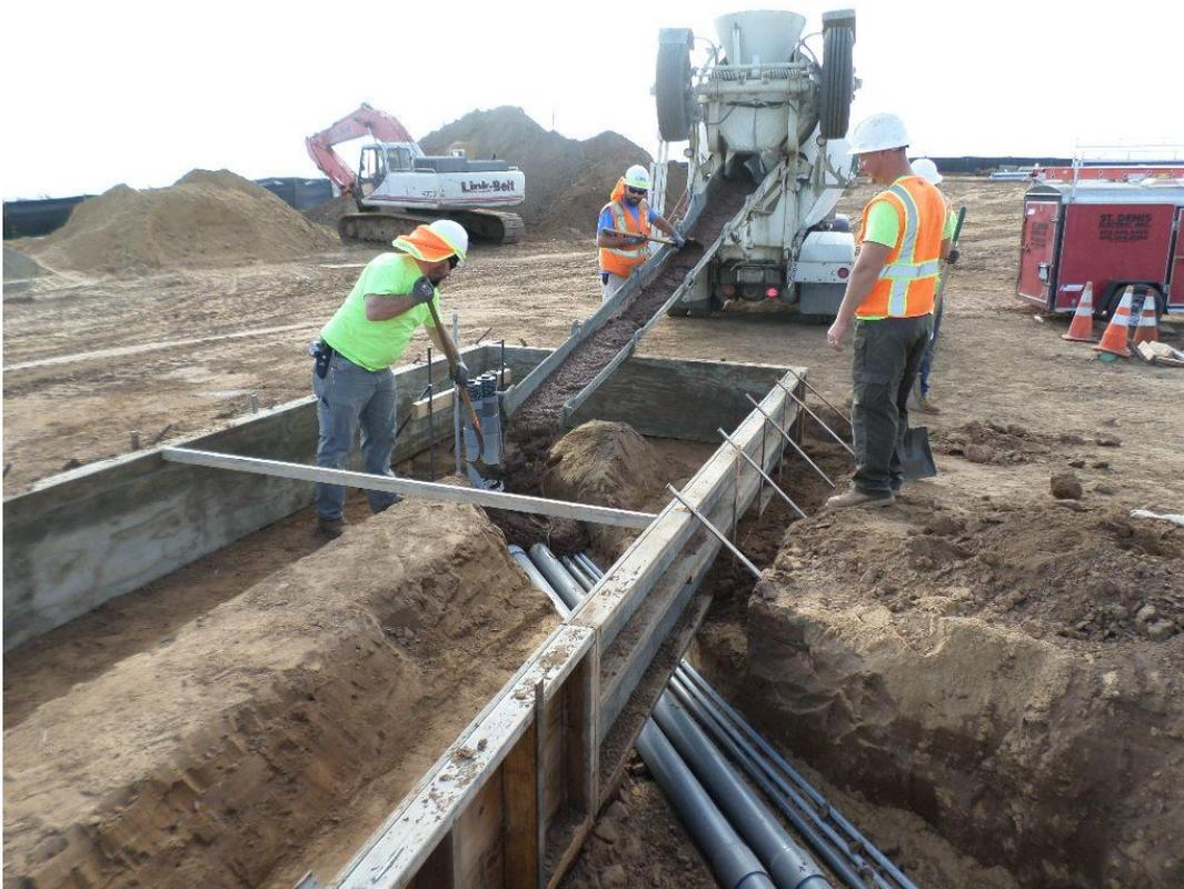
St. Dennis Electric pouring red slurry over emergency generator conduit.
