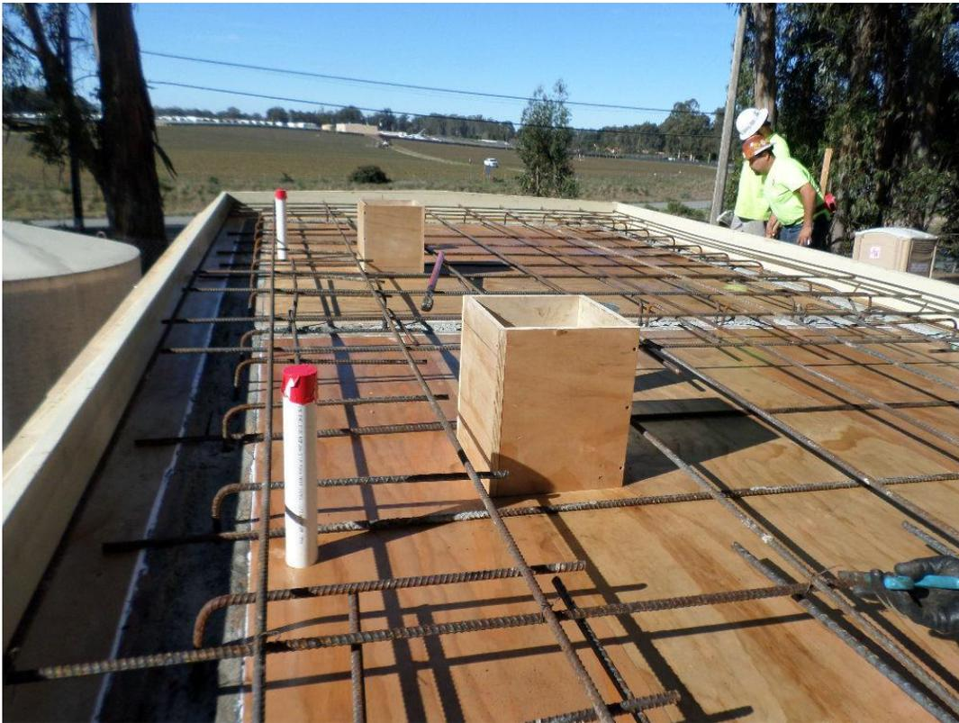
Forms completed and Vista Steel installing reinforcing for the chemical building roof pour.
