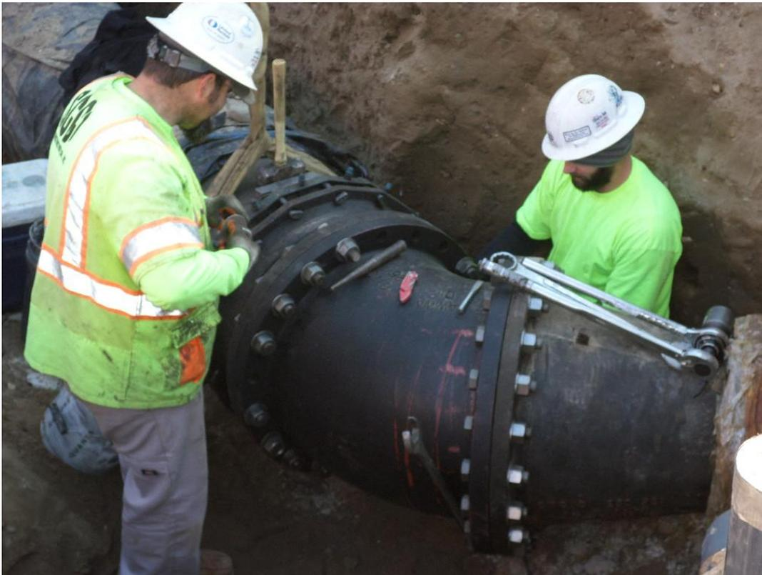
Spiess installing new 45 degree elbows to replace the defective elbows supplied to the District by Ferguson.
