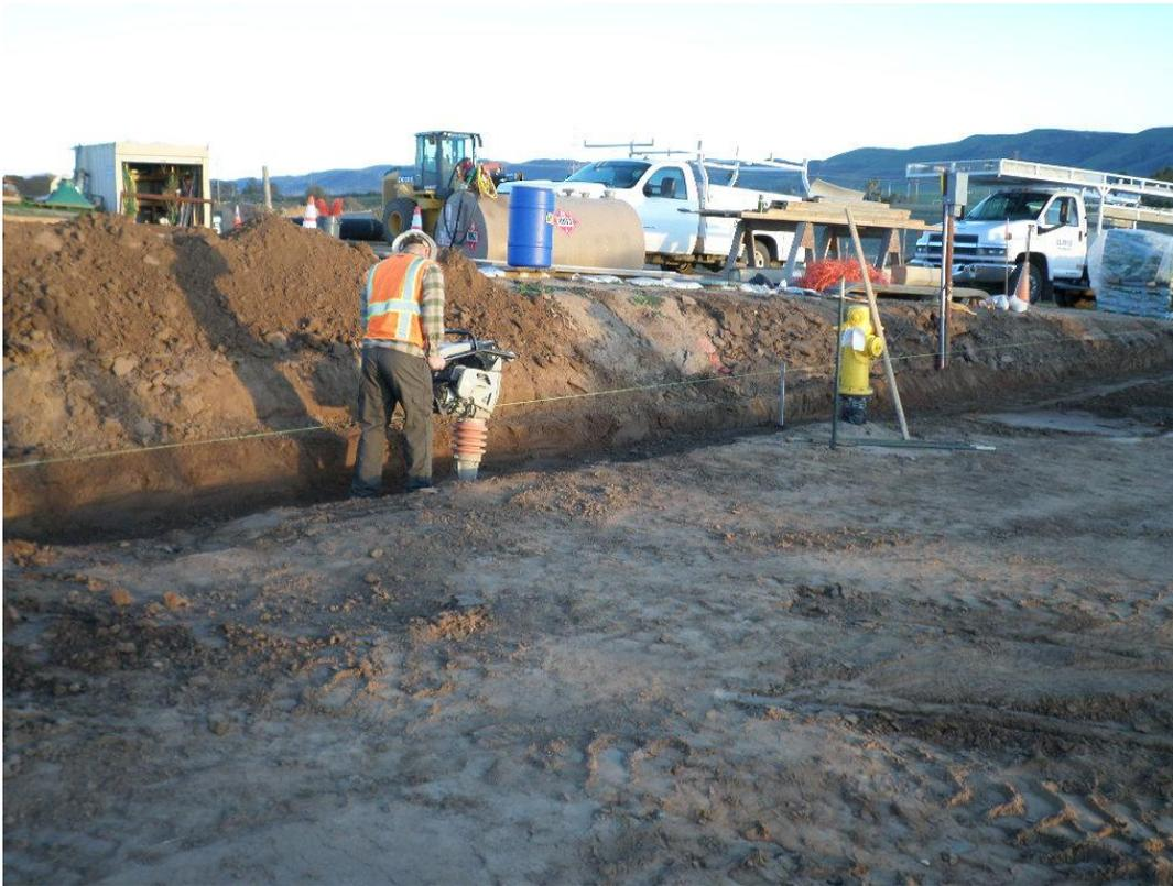
Spiess preparing base for curb and gutter construction.
