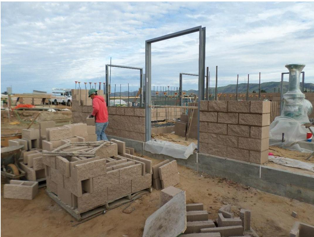
Door frames and block being installed at the pump station.
