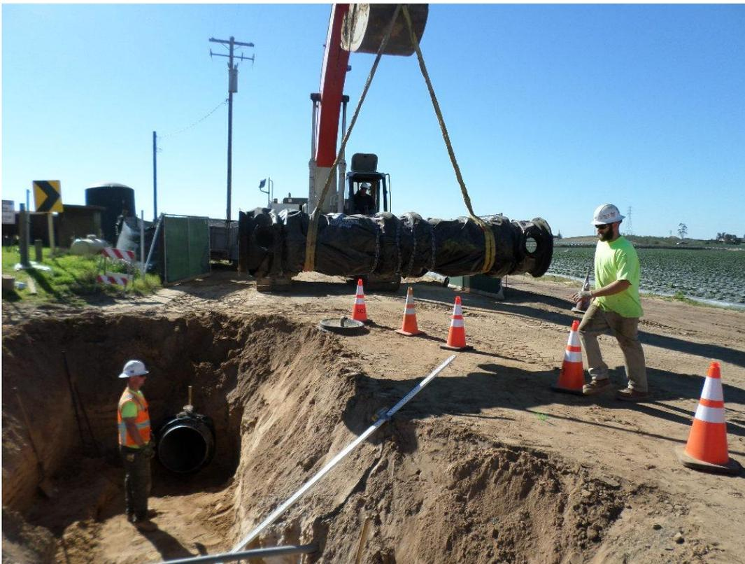
Spiess installing the 24-inch DIP bypass.
