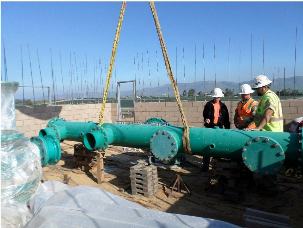
Spiess installing the discharge manifold at the pump station.
