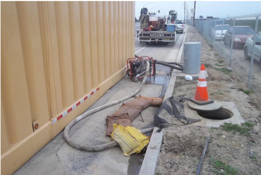
Dechlorinated water from flushing being released into a storm drain which connects to the SBCFC drainage channel.
