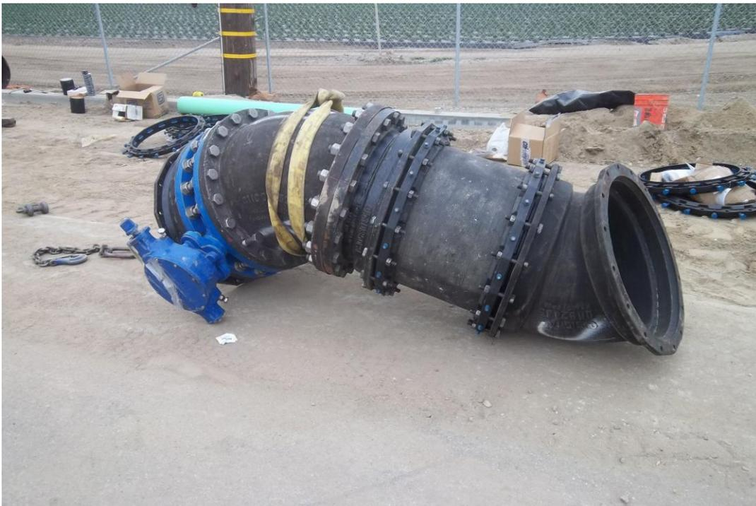
Butterfly valve bolted together with 45's for storm drain crossing approximate Station 12+00.
