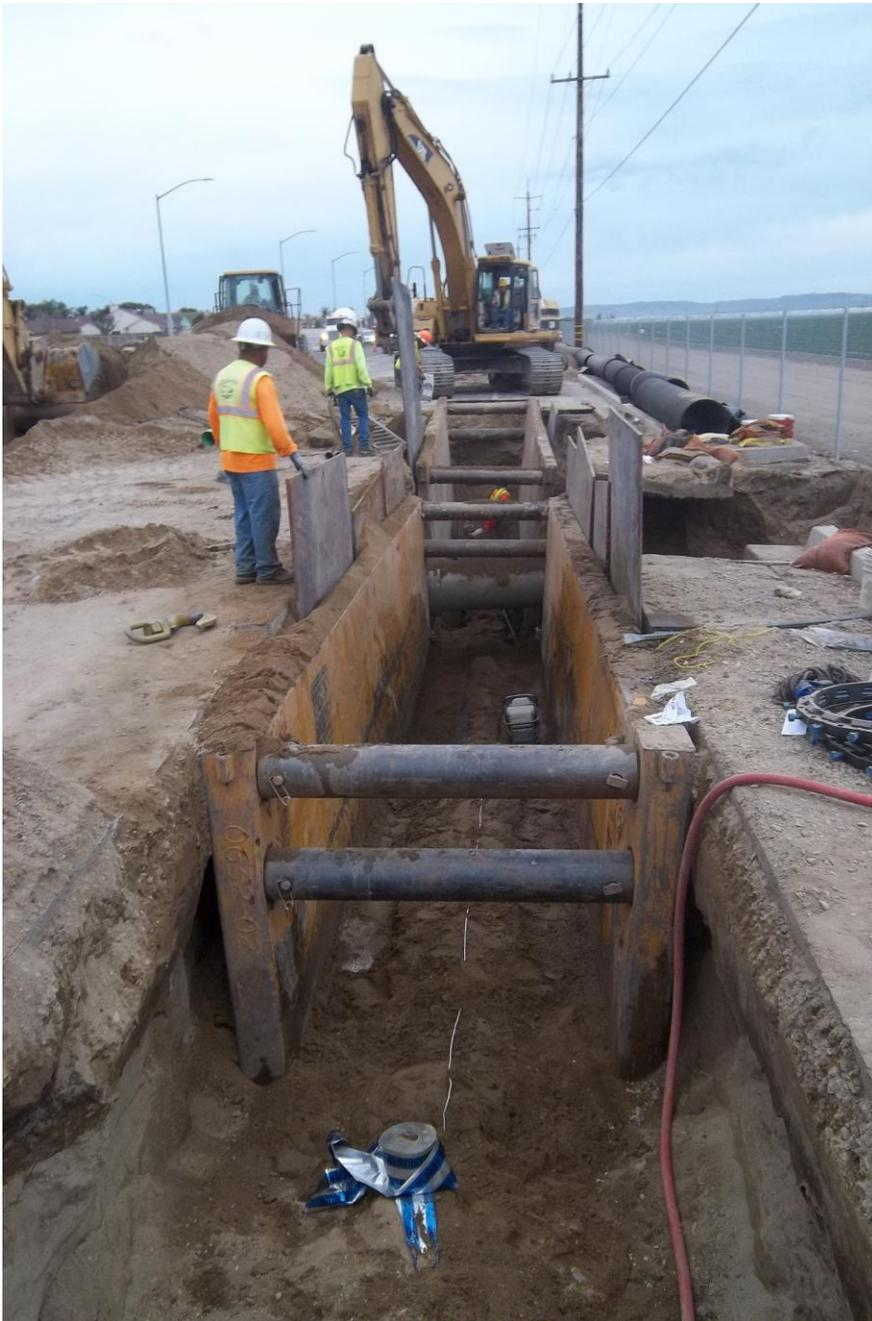
D-KAL placing steel plates to support area around catch basin at 18-inch RCP storm drain when trench shields are removed.
