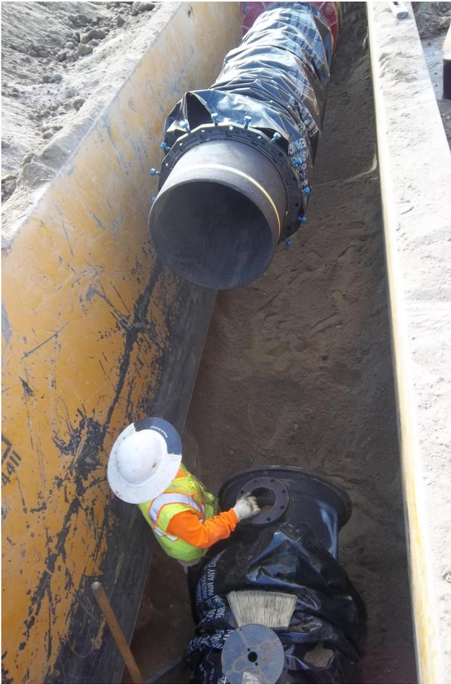
D-KAL installing 24-inch DIP.
