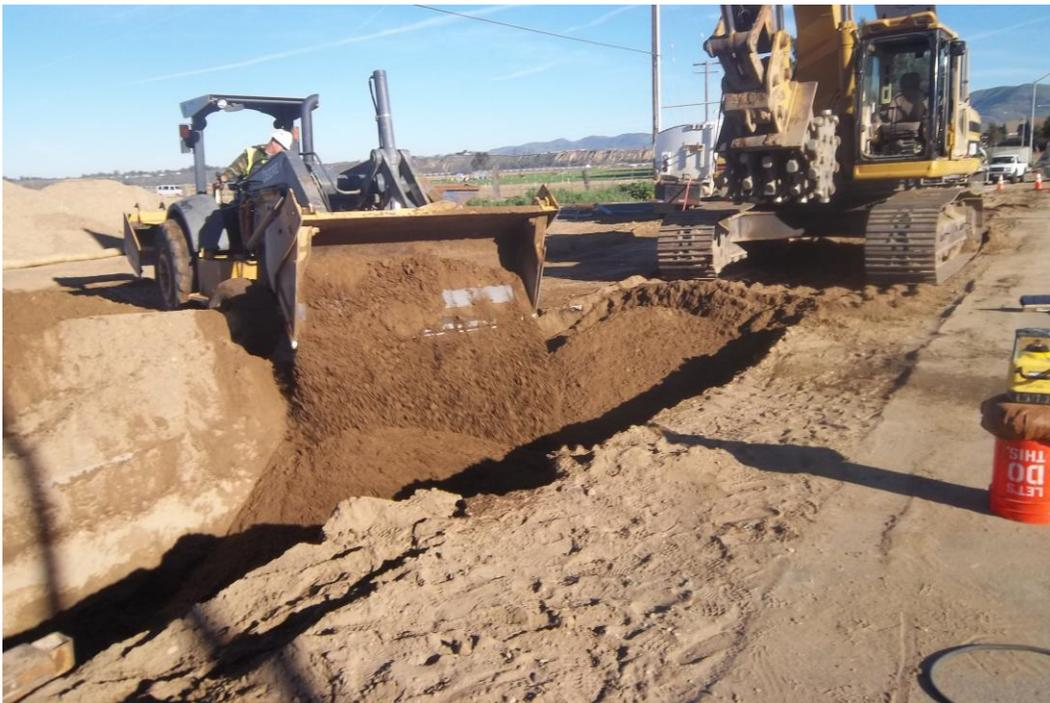
D-KAL backfilling and compacting over storm drain as it is relocated.
