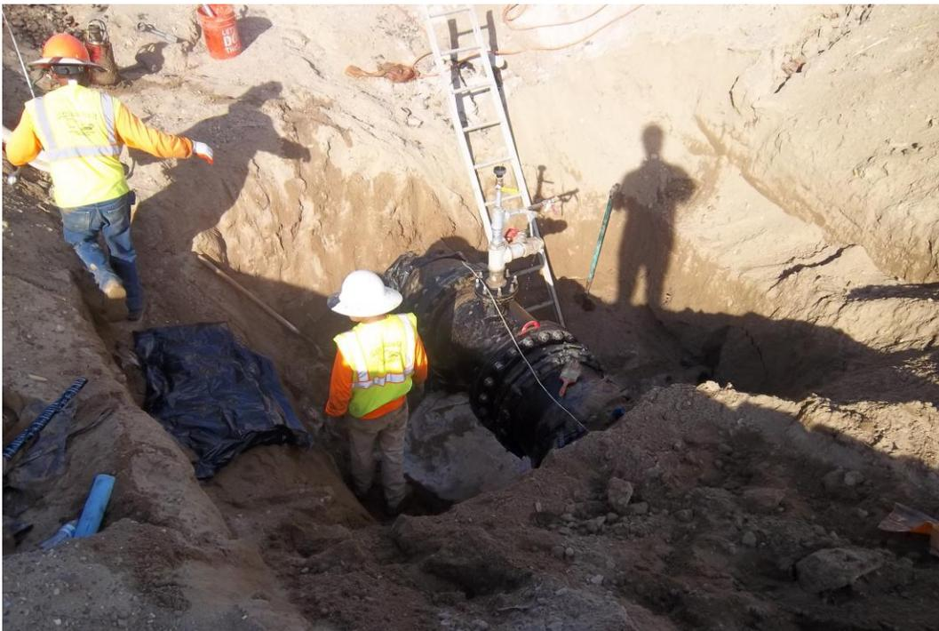
D-KAL preparing to remove the test plate from previously tested section of pipe under the levee and river area.
