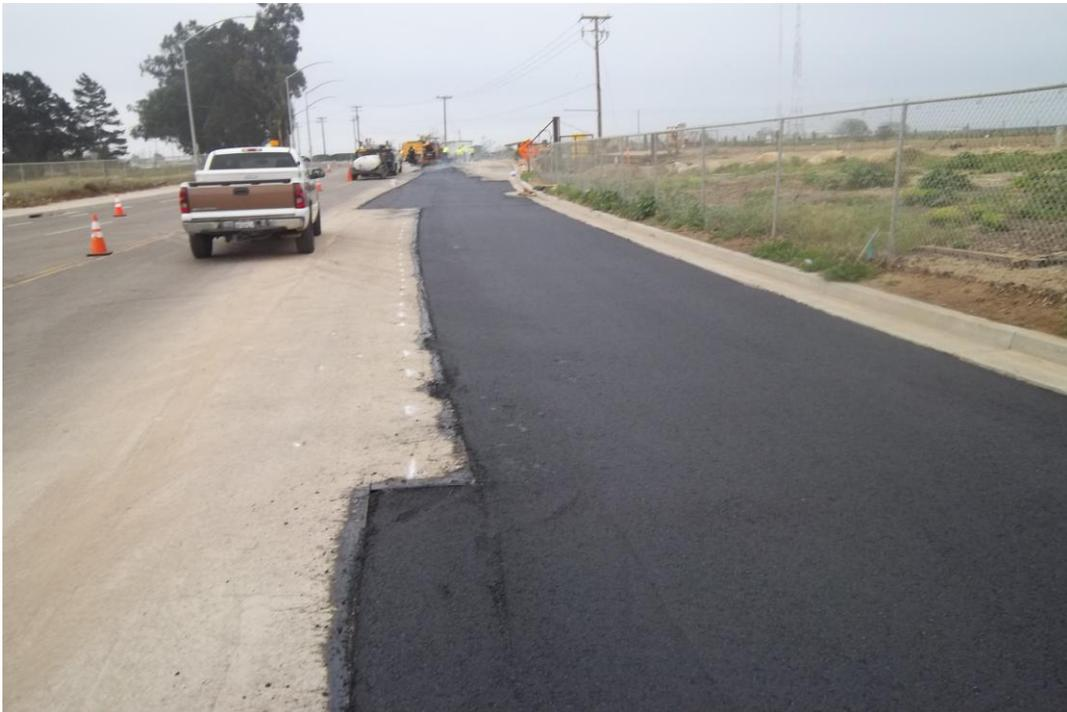
First lift of paving completed.
