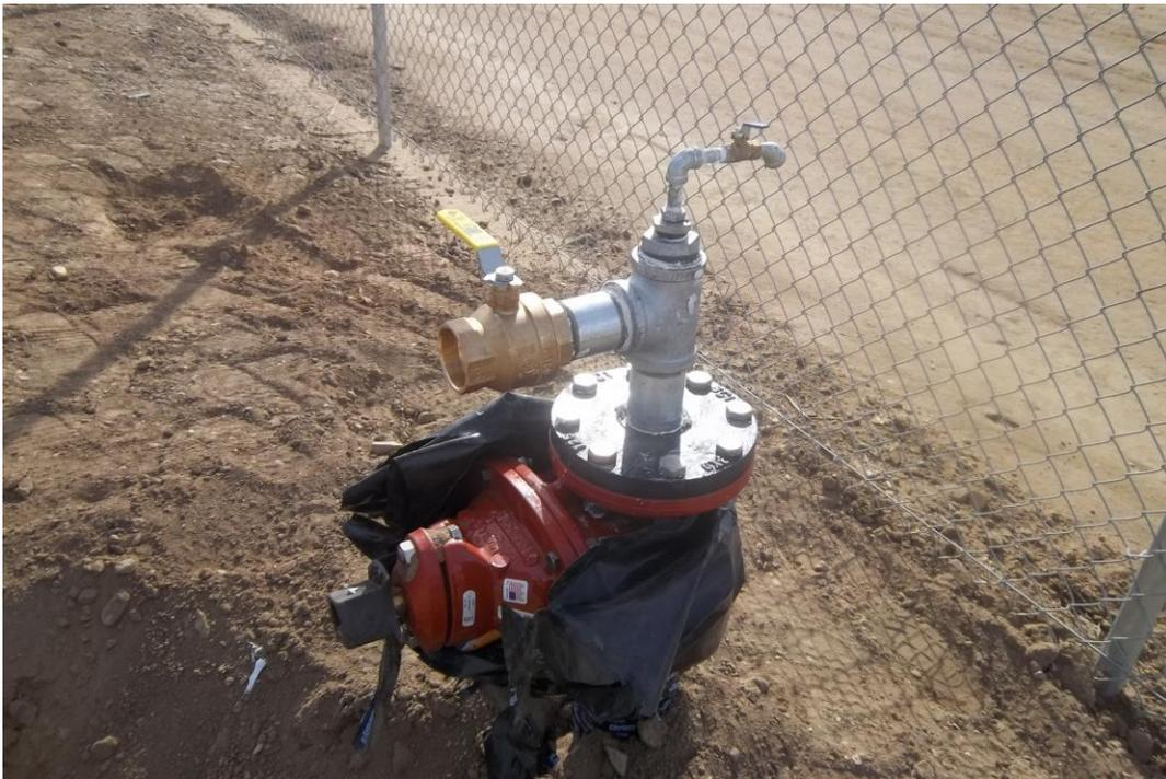
CAV installed at Station 5+33.
