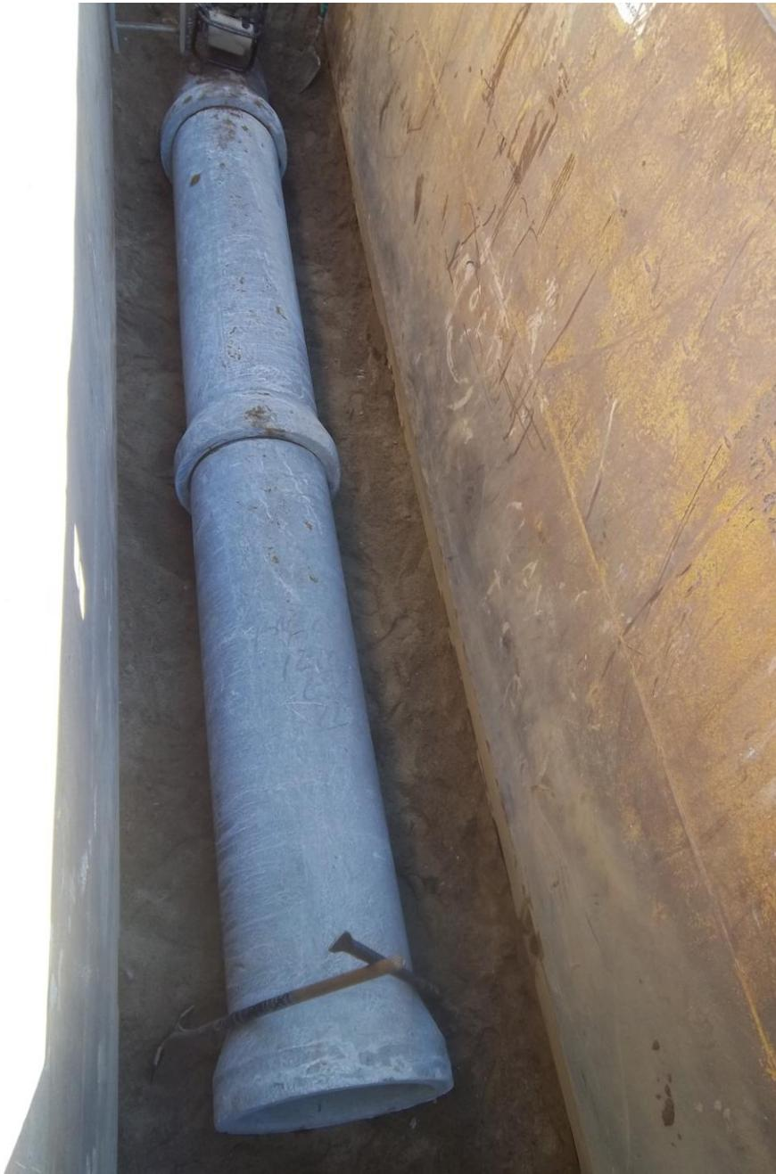
New and relocated 18-inch RCP installed a minimum of 4 feet from the 24-inch DIP waterline.
