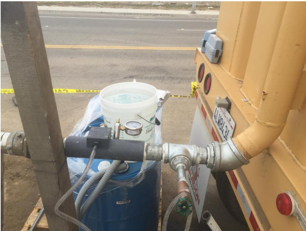
Sodium hypochlorite injection and monitoring for dechlorinating water flushed from 24-inch DIP into Baker tank.
