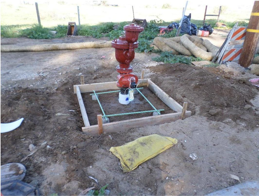
D-KAL installing concrete pads around CAV's.
