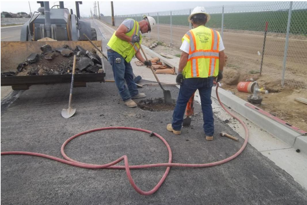
D-KAL jack hammering new pavement to locate valve risers and install valve cans and lids to grade.
