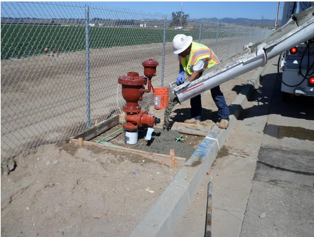
D-KAL pouring the concrete pads at the CAV's.
