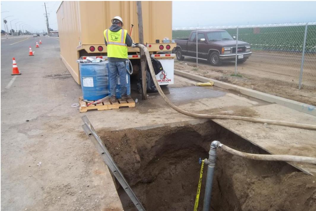
D-KAL flushing water from the end of the pipe line Taylor Street where it is dechlorinated going into a Baker tank before being released into the SBCFC drainage channel.
