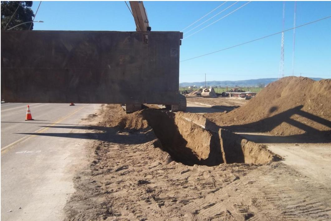
D-KAL installing trench shields for construction of the new 18-inch RCP located a minimum of 4 feet from the new 24-inch DIP waterline in Blosser Road.
