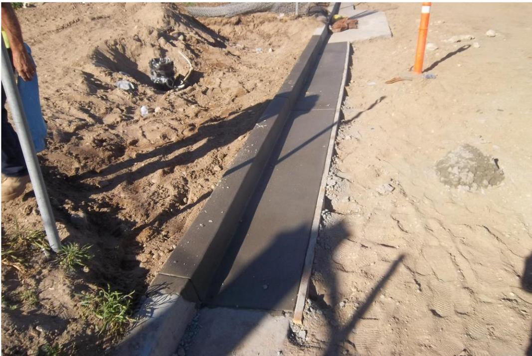
Finished repair of concrete curb and gutter along Blosser Road.
