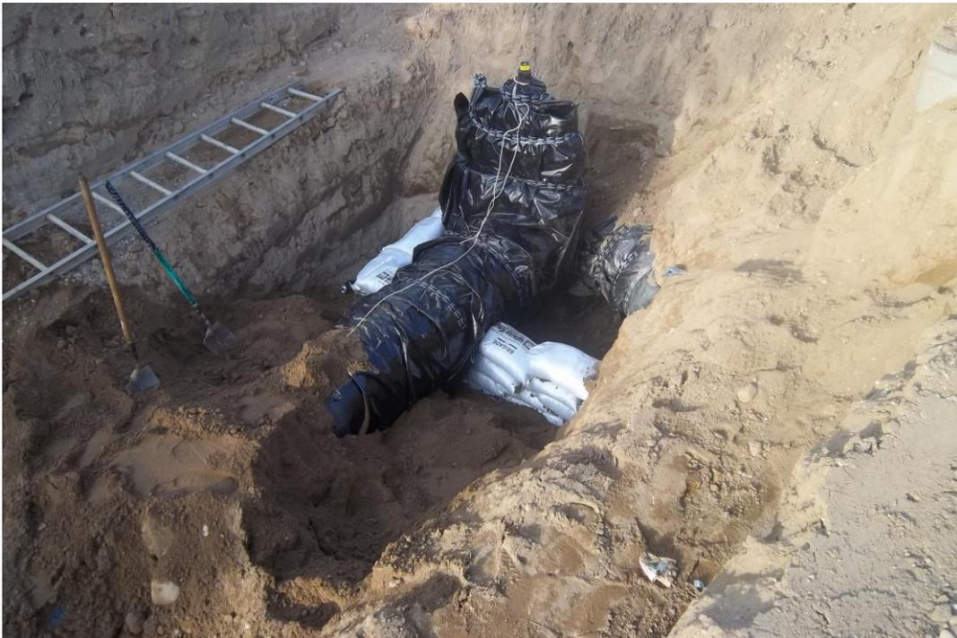
D-KAL preparing to pour concrete to support 24-inch gate valve.
