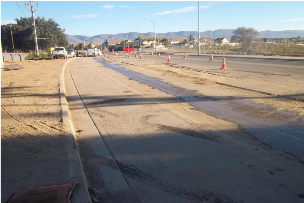
Saw cutting trench for storm drain relocation.
