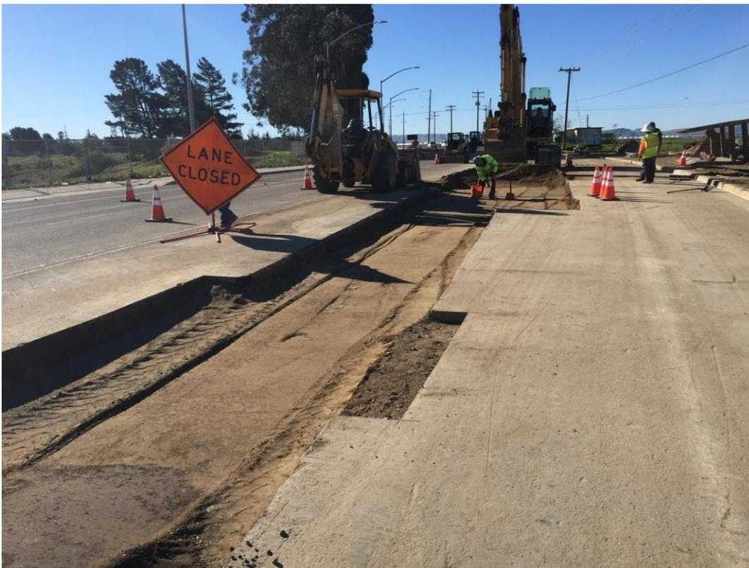
Furgo on site taking compaction tests of the subgrade.
