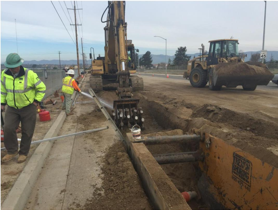
D-KAL continuing compaction over 24-inch DIP.
