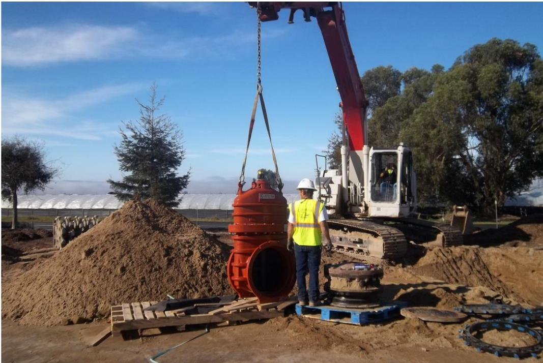
D-KAL lowering 24-inch gate valve into trench at pig launcher.
