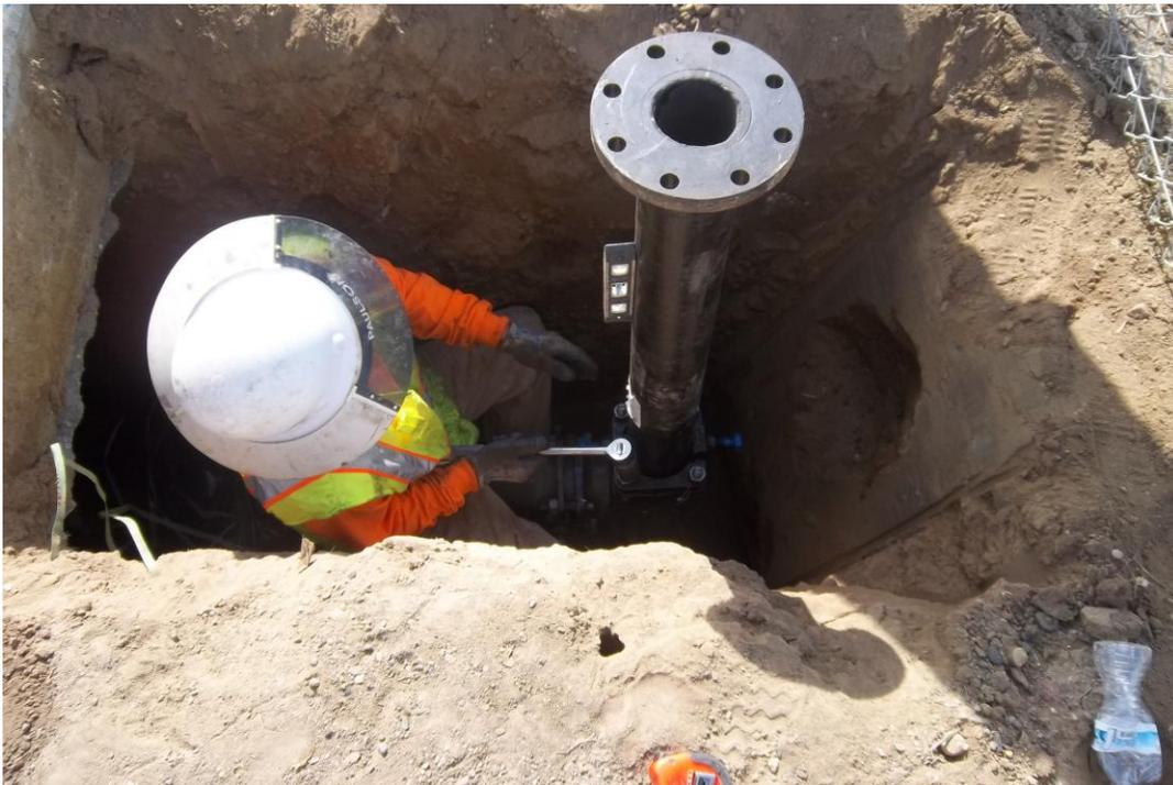
Installing riser for CAV at Station 5+33.
