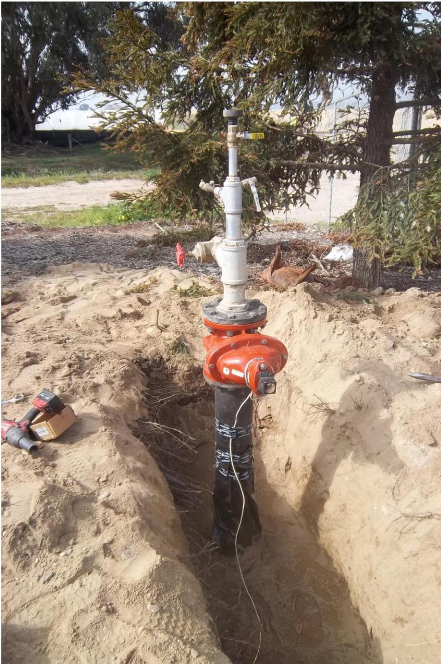
D-KAL set-up for pressure test off gate valve at Station 50+83.
