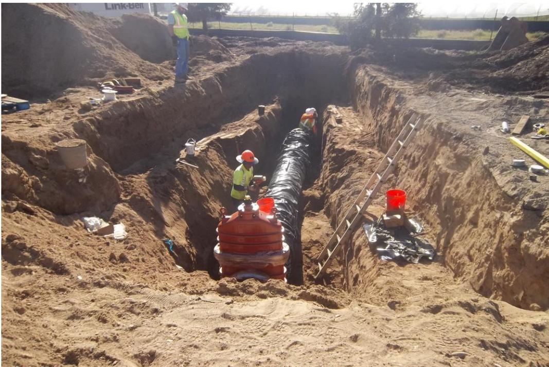
Gate valve installed with pig launcher.
