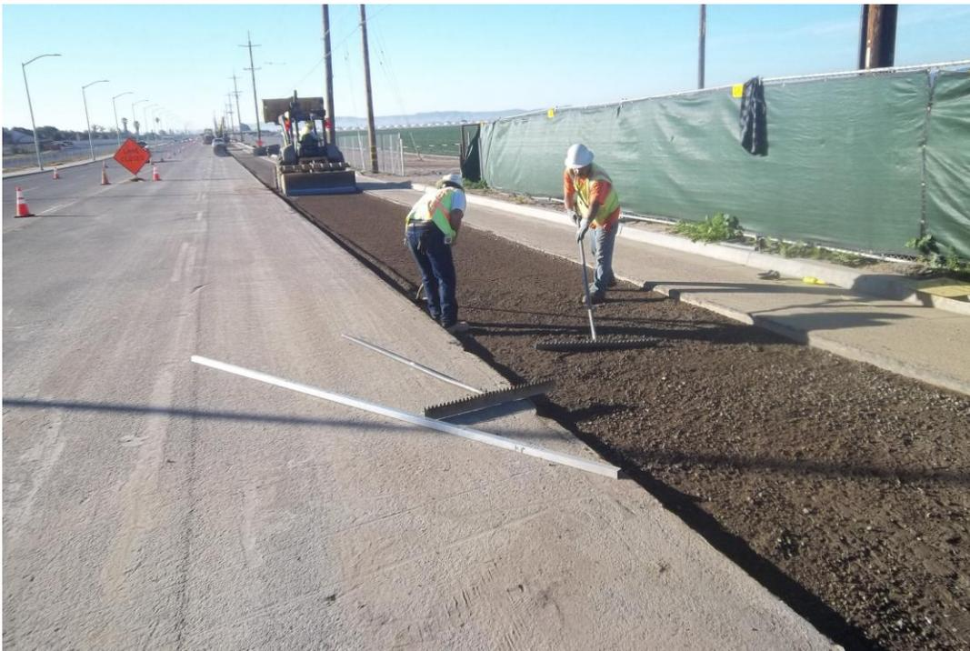
D-KAL spreading and grading the aggregate base over the trench.
