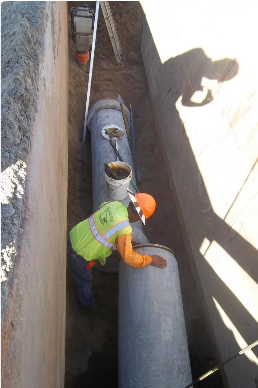
D-KAL installing the relocated 18-inch RCP storm drain.
