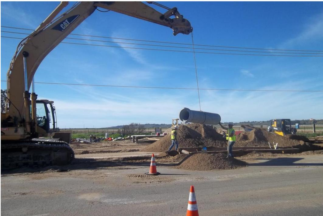
D-KAL installing the relocated 18-inch RCP storm drain in Blosser Road.
