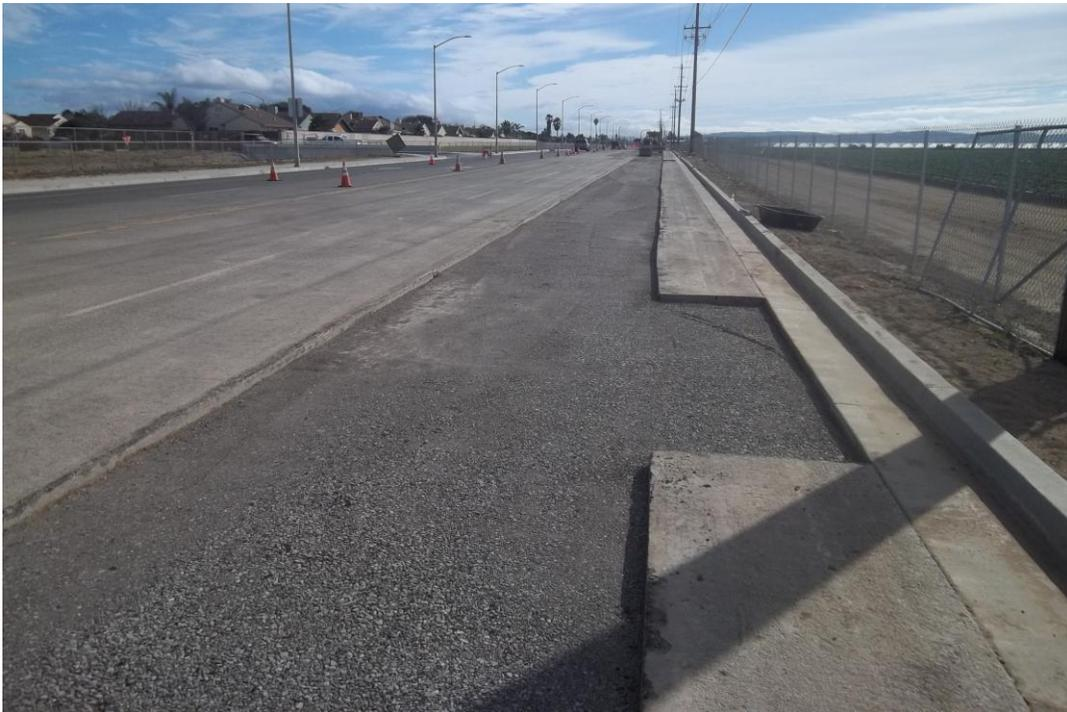
D-KAL compacting the aggregate base over the trench in preparation for paving.
