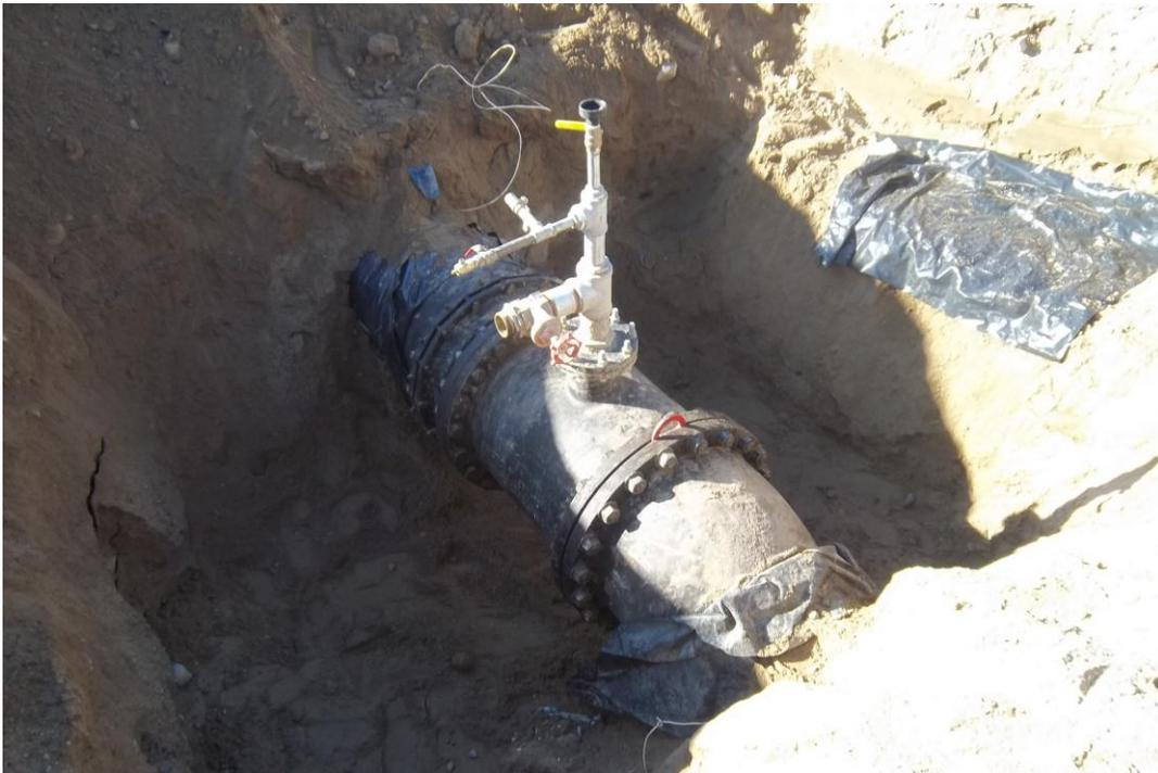
Test plate relocated to the other side of the 24 X 6-inch tee for testing remaining section of pipe from Atlantic to Taylor.
