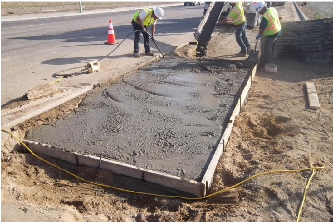
D-KAL pouring two sack slurry over storm drain crossing at approximate Station 12+00.
