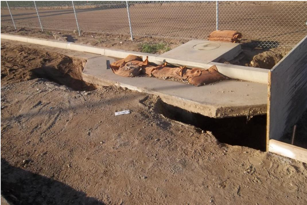
D-KAL preparing the drainage inlet at the storm drain crossing for backfill with two sack slurry.
