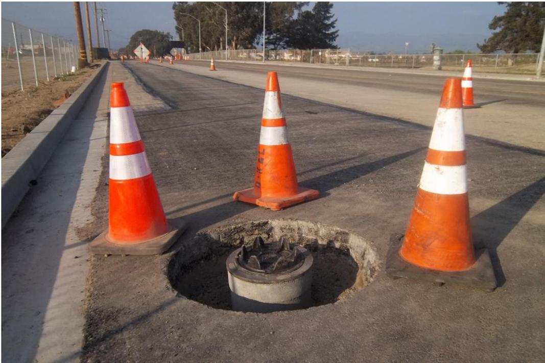
D-KAL installing valve cans and lids to finish grade.
