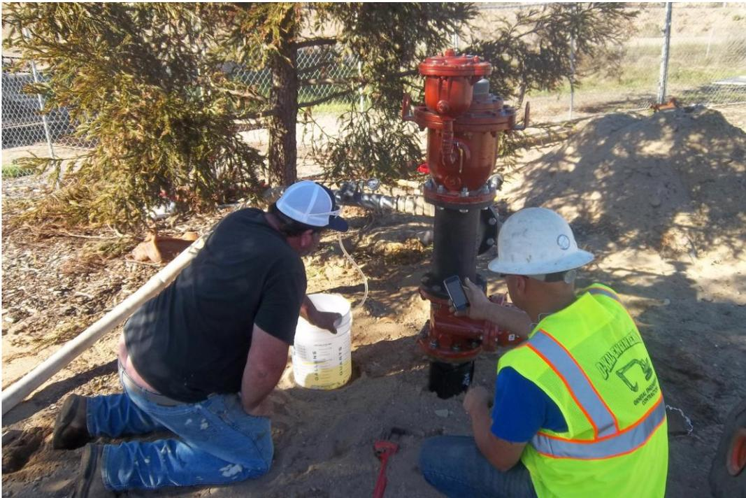
D-KAL injecting chlorine into the 24-inch DIP to disinfect for bacteria test.
