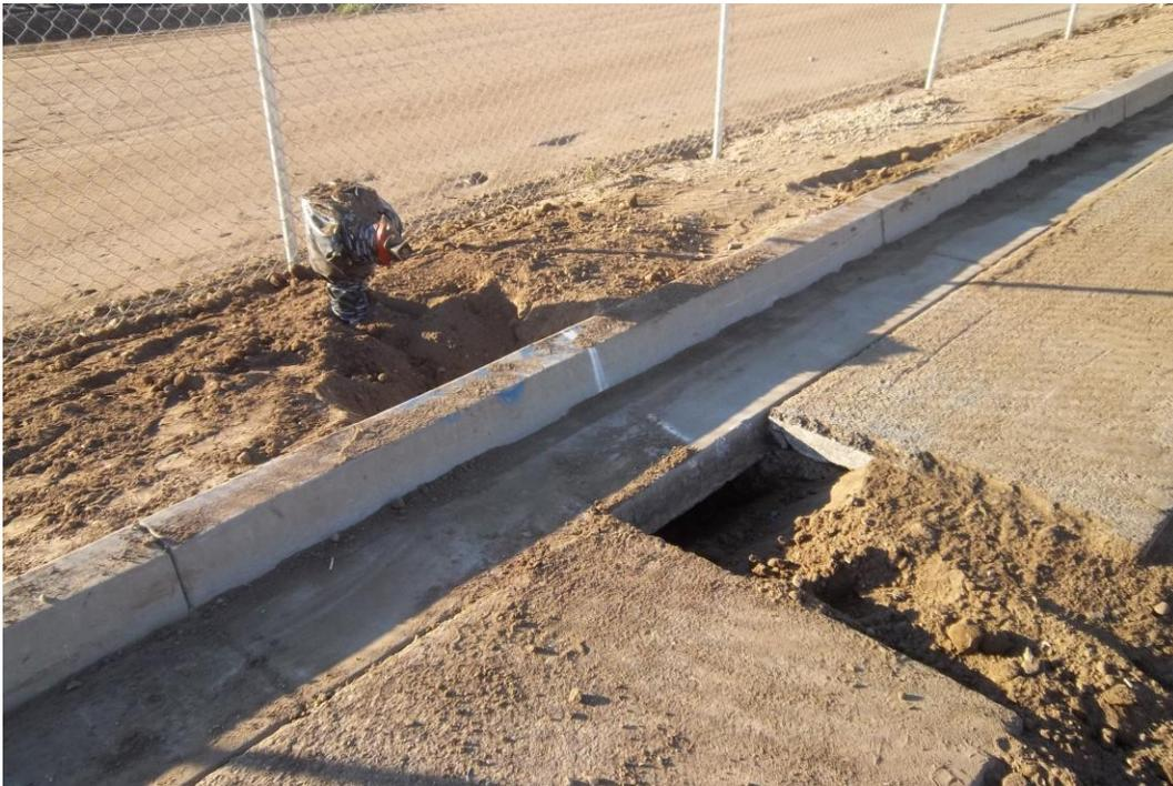
Gate valve and riser installed for CAV.
