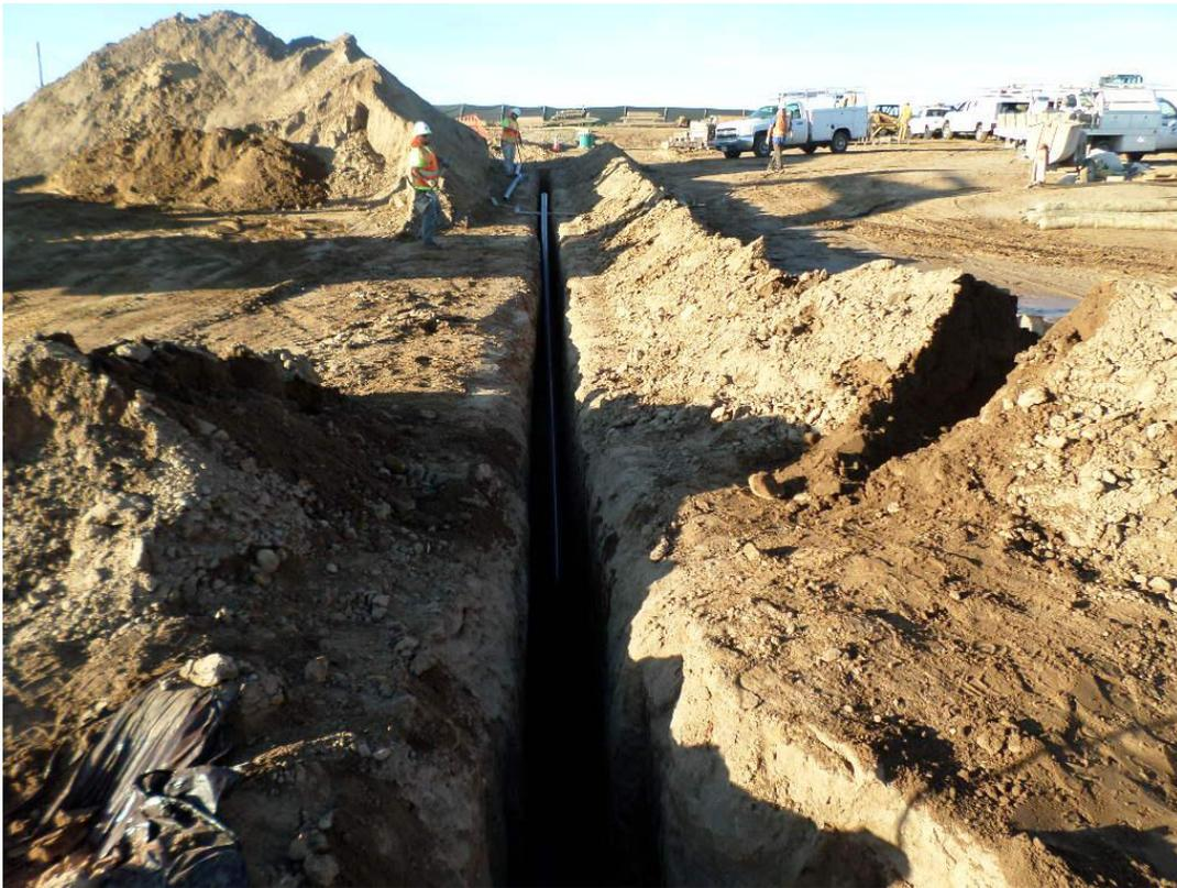
St. Denis Electric installing PG&E conduit across pump station site.
