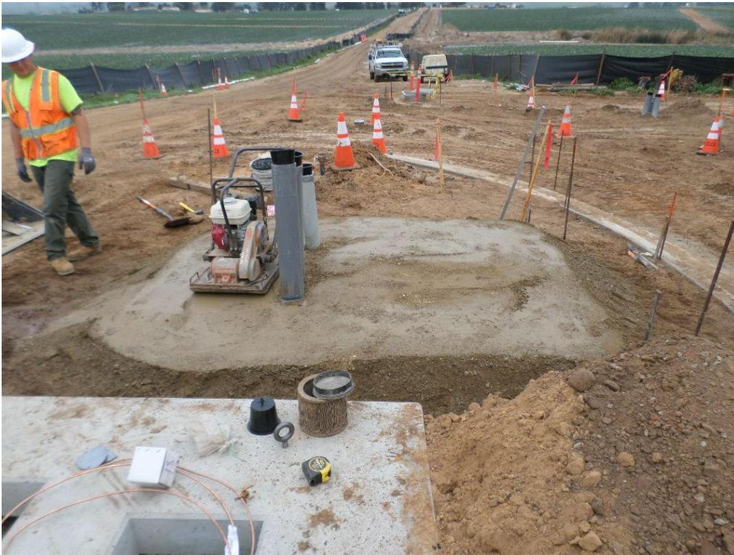
Spiess compacting base for setting transformer pad.
