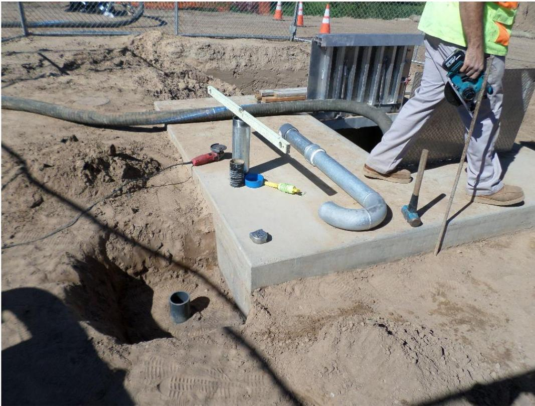
Spiess installing vent piping at the PRV vault.
