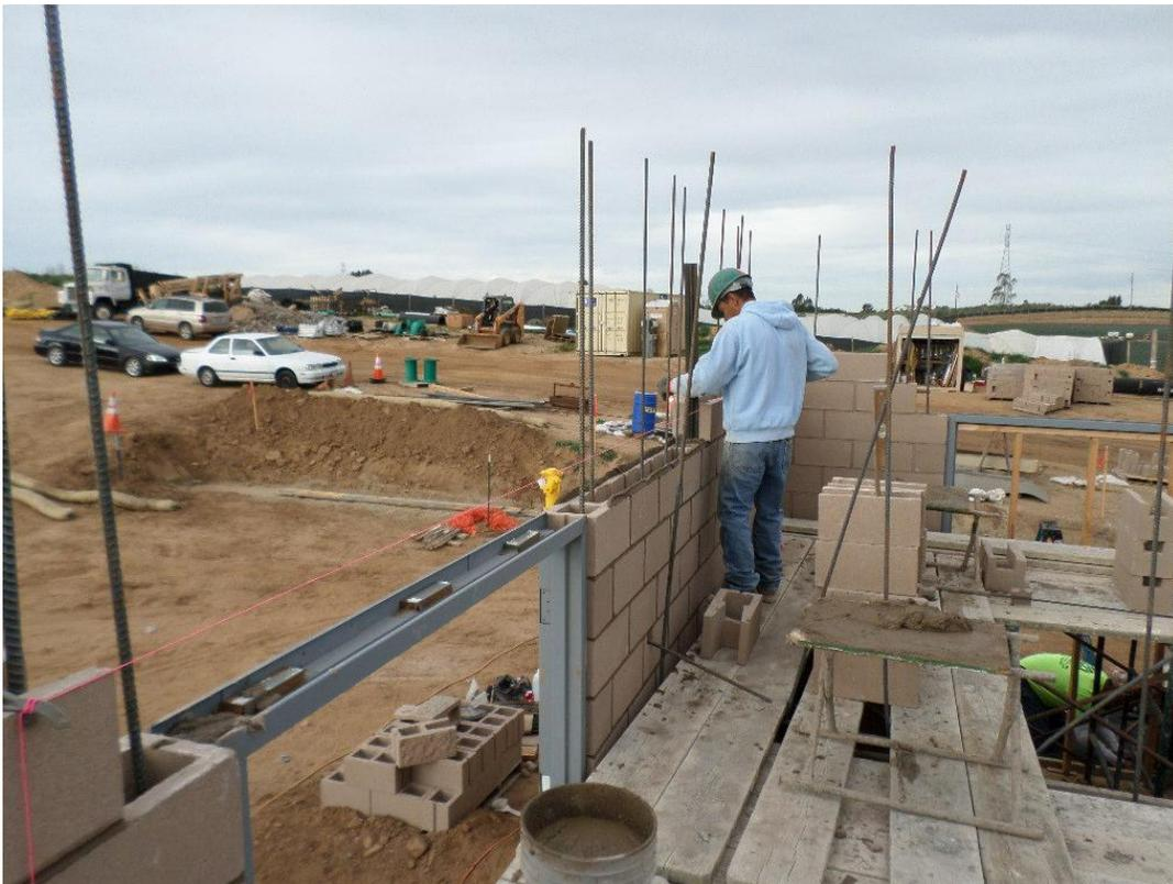
Boydston Masonry installing CMU along the west wall of the pump station building.
