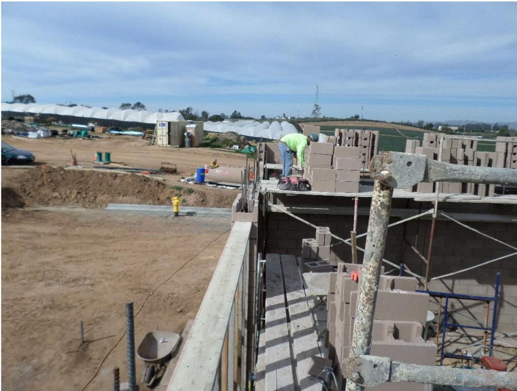
Boydston Masonry laying CMU along the west wall of the pump station building.
