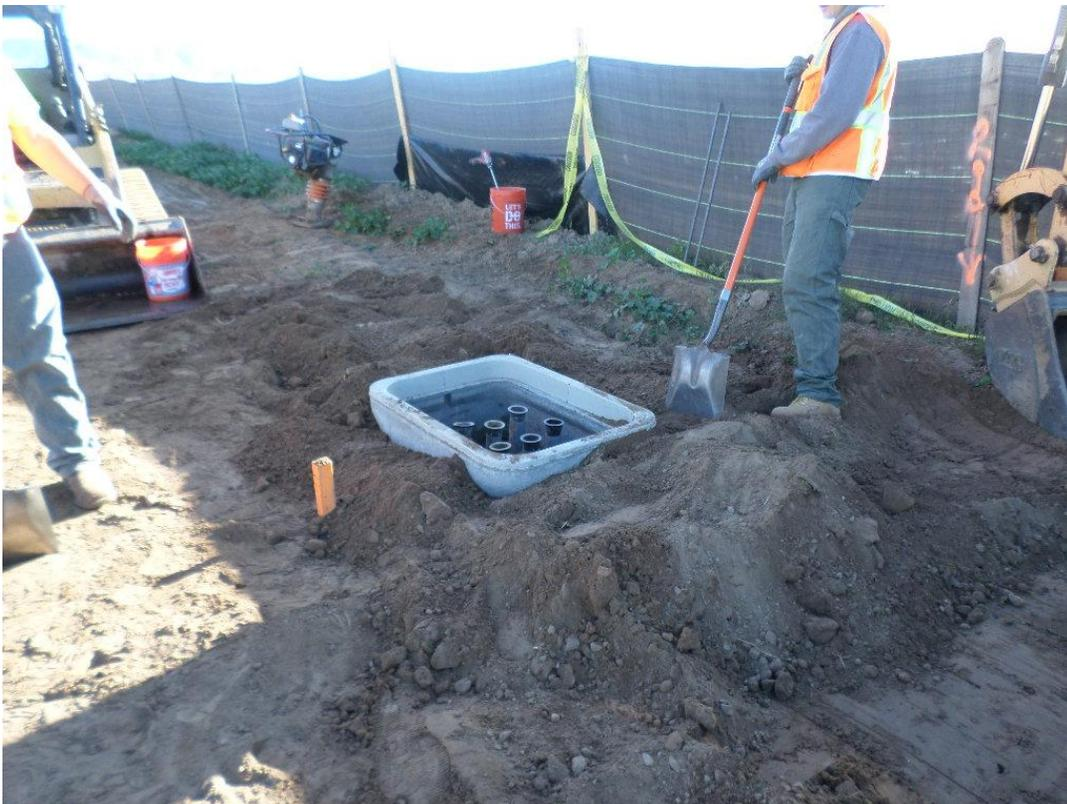
Spiess installing pull boxes along for the AT&T conduit in the access road.
