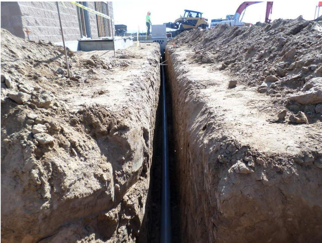
St. Denis Electric installing PG&E duct bank across pump station site.
