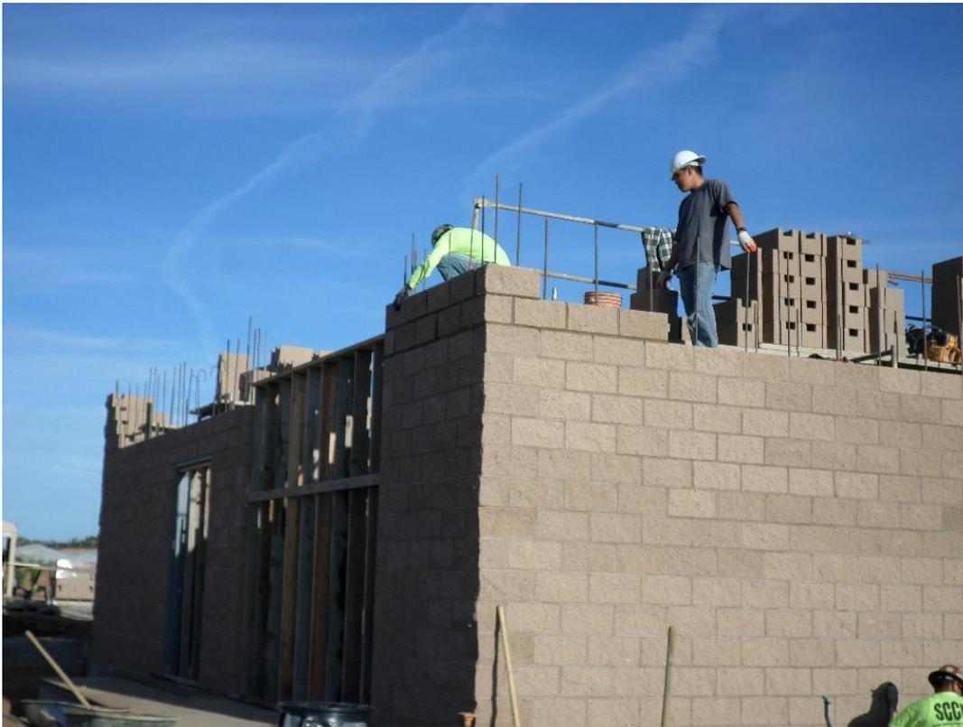
Boydston Masonry laying the corner lead at the pump station building.
