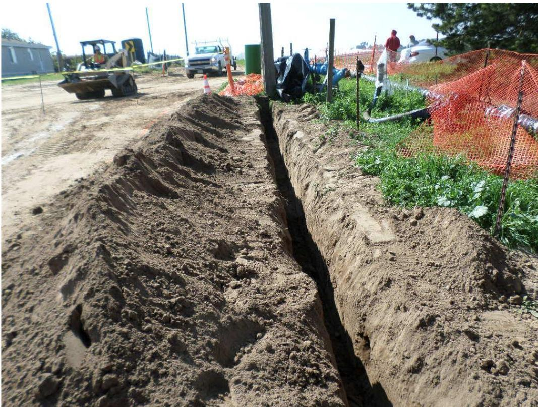
St. Denis Electric excavating for the main power feed conduit to the PRV vault.
