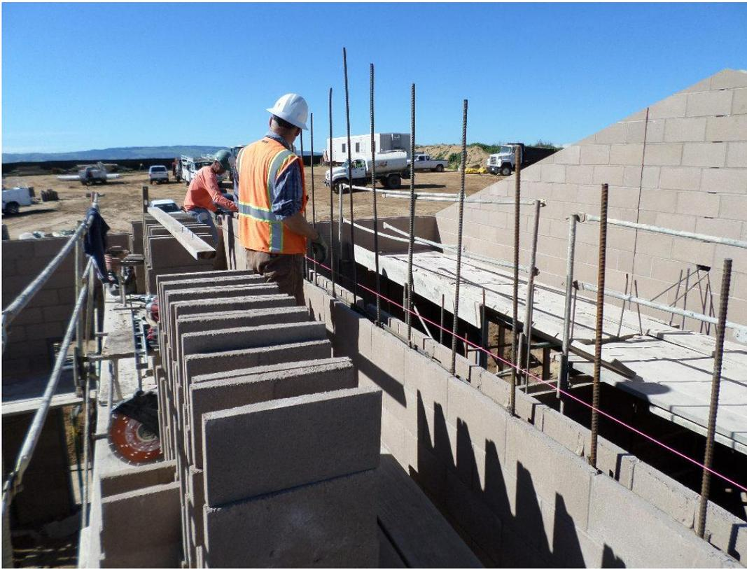
Boydston Masonry constructing the interior wall of the pump station building.
