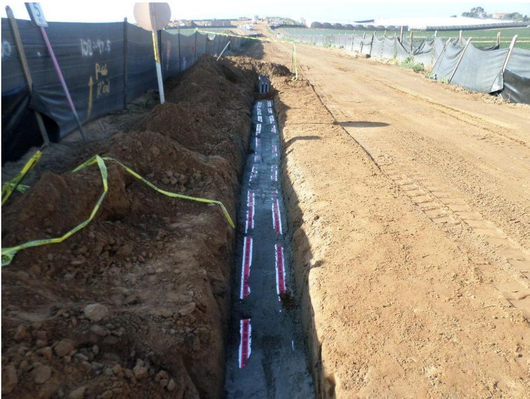
Concrete poured over AT&T conduit at oil line crossing.
