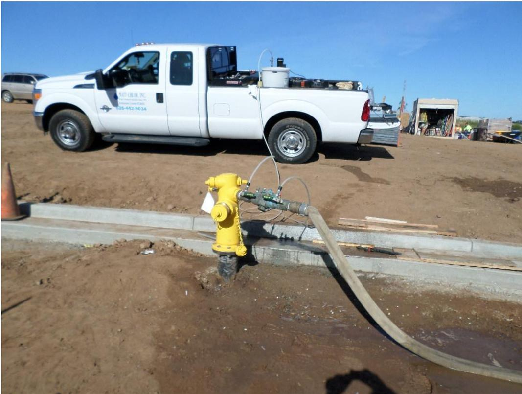
Matt-Chlor dechlorinating water after soaking 24-inch DIP in preparation for bacteria test.
