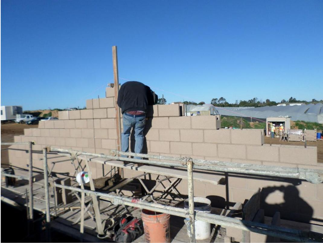
Boydston Masonry installing CMU on north wall of pump station building.
