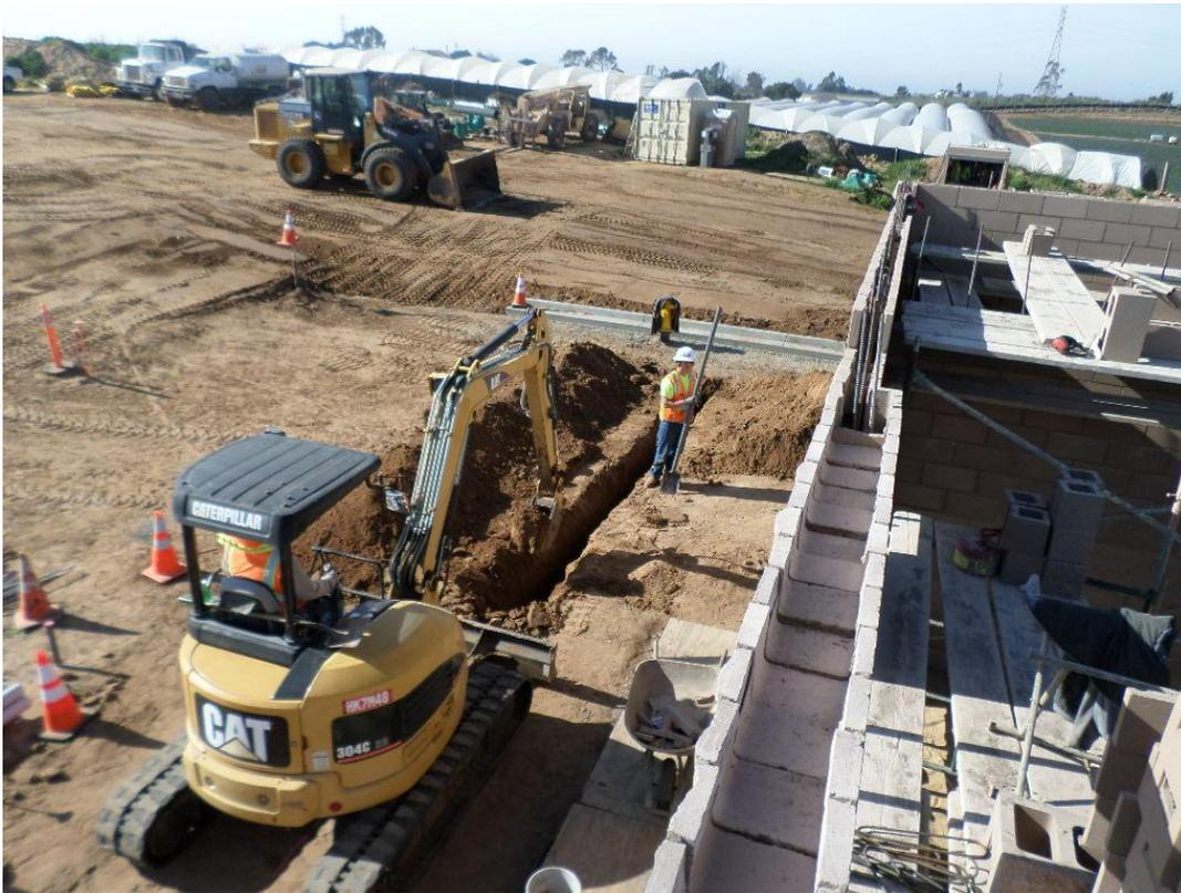
St. Denis Electric starting excavation of trench for PG&E conduit.
