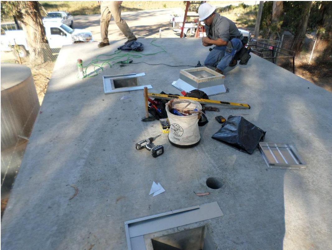
Dahl Air Conditioning installing exhaust fan curb on roof.
