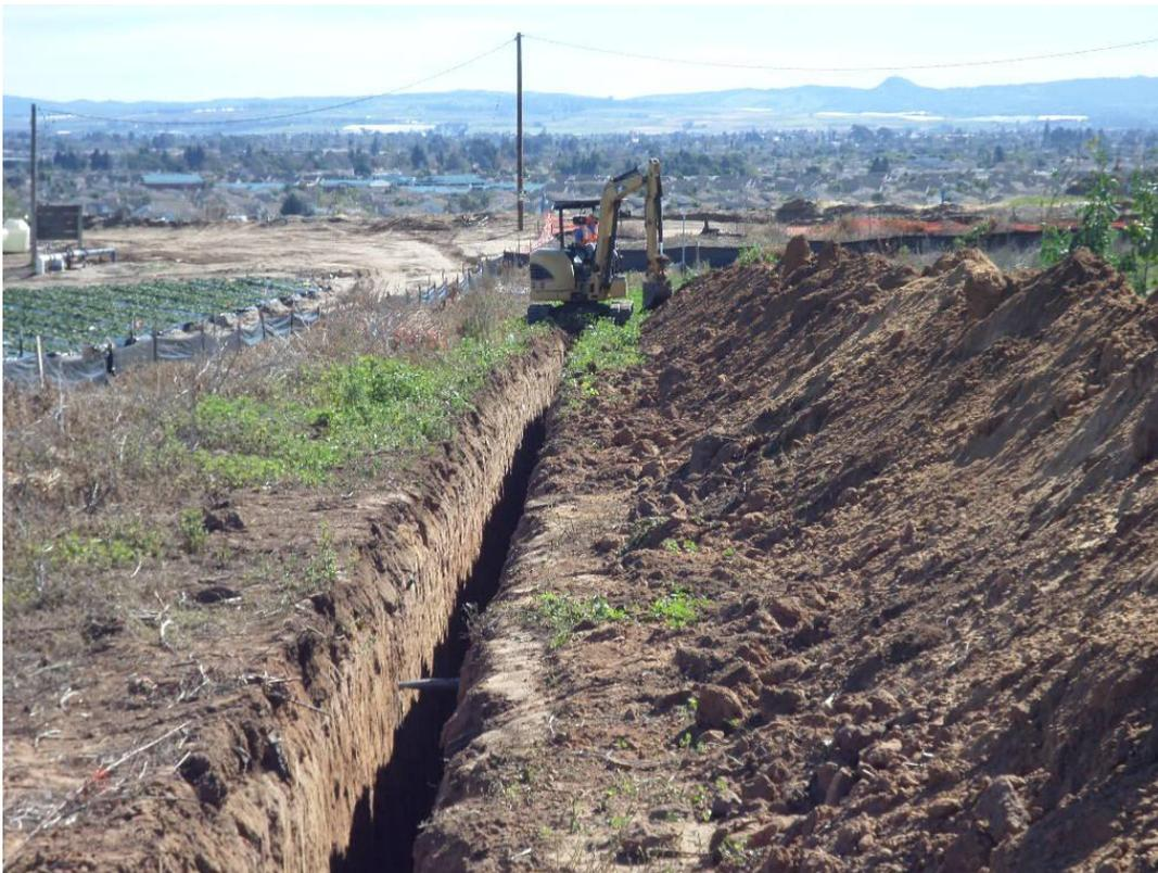
St. Denis Electric installing the PG&E conduit across the easement to the new pole location.
