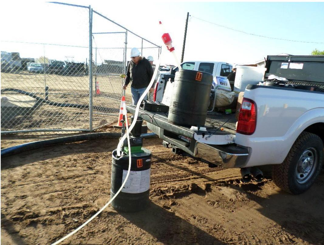
Matt-Chlor injecting chlorine into 24-inch DIP to disinfect pipe in preparation for bacteria test.
