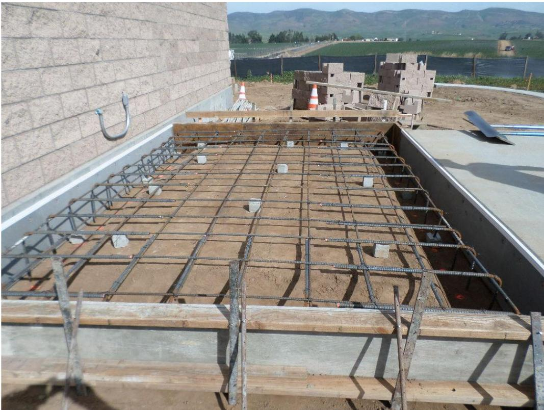
HVAC pad formed and reinforcing installed.
