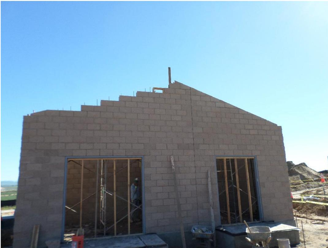
Boydston Masonry installing CMU on the north facing wall of the pump station building.
