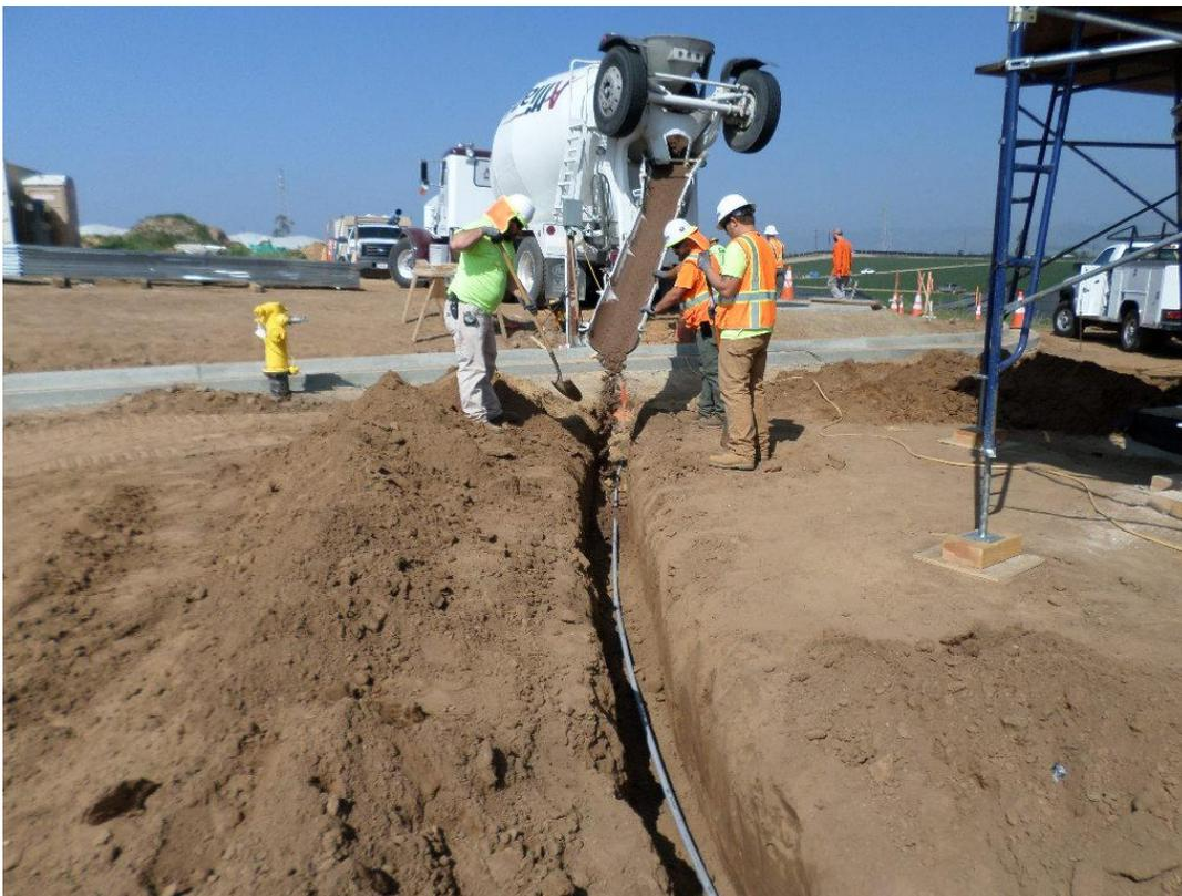
St. Denis Electric pouring red slurry over electrical conduit on site.
