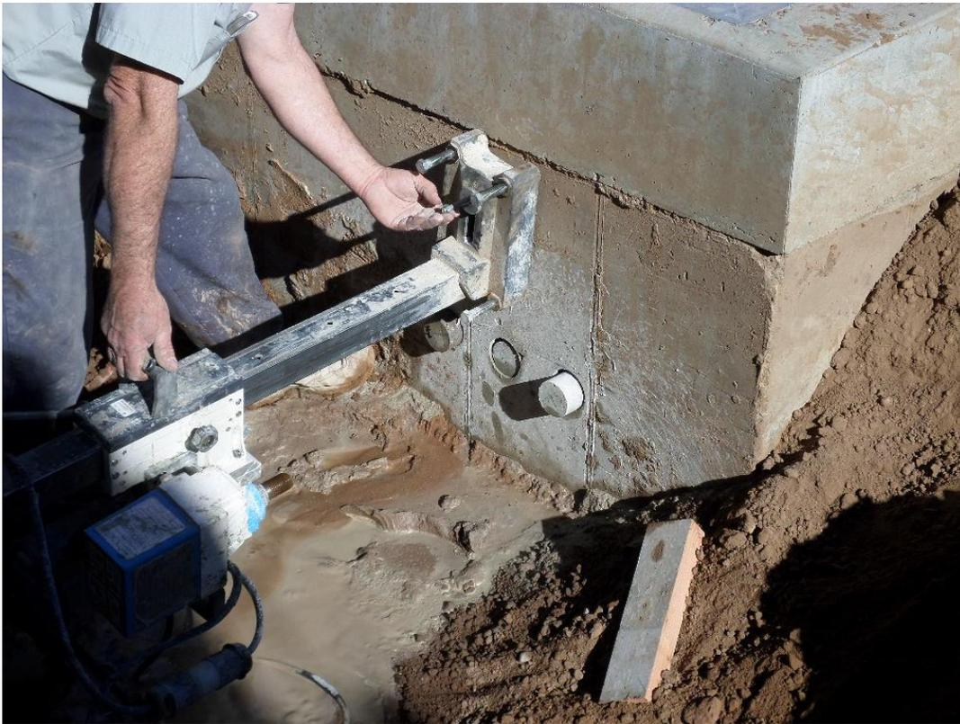
Kahn Concrete Cutting coring electrical conduit penetrations at metering vaults.
