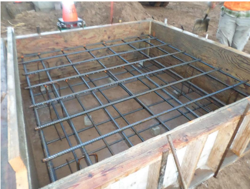
Surge tank pad formed and reinforcing installed.
