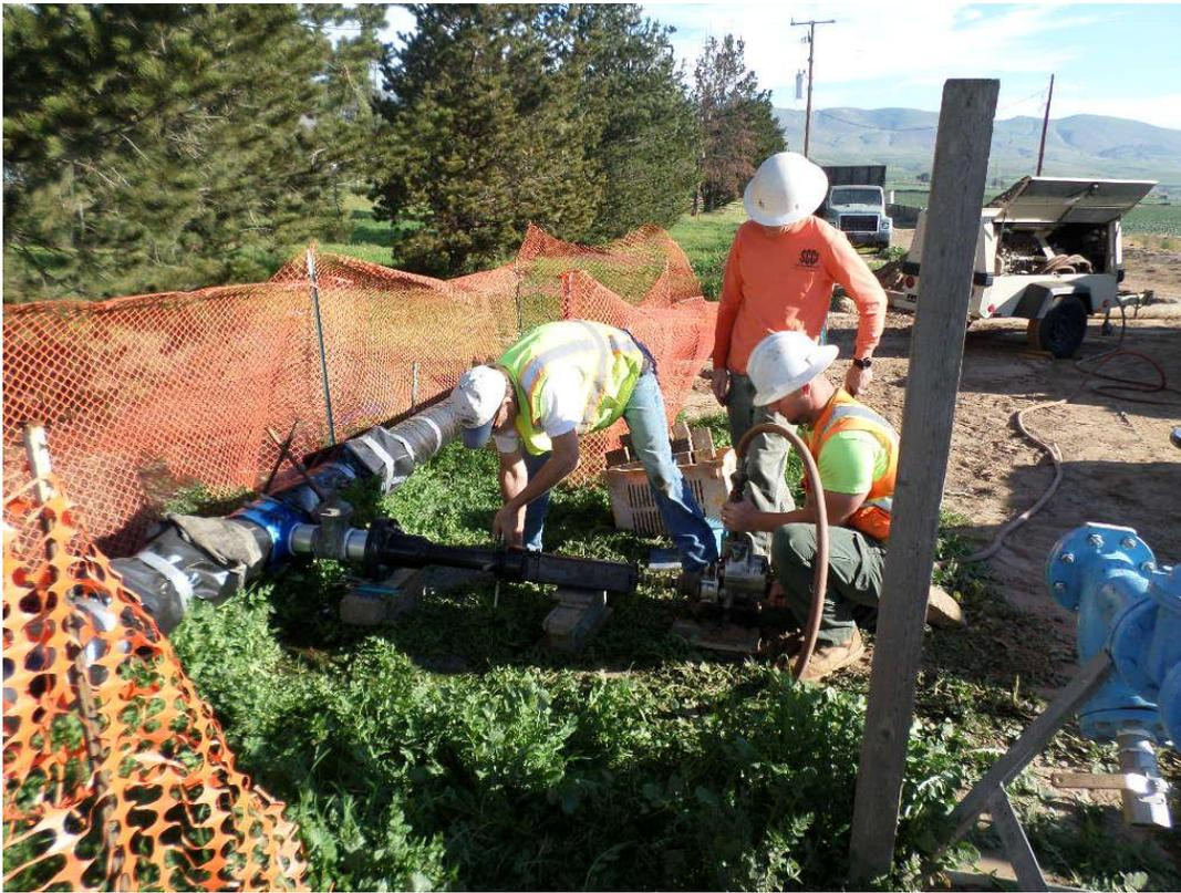
Performing the hot tap on the 8-inch bypass line.
