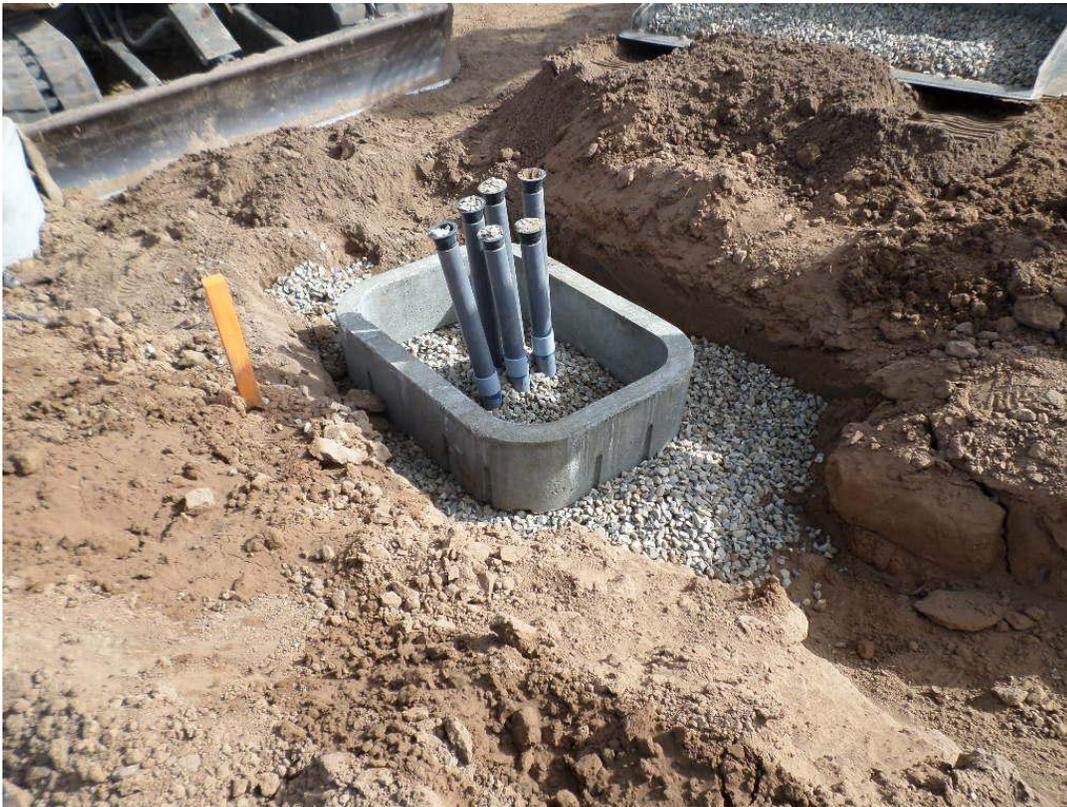
Pull box installed for the AT&T conduit on the access road.
