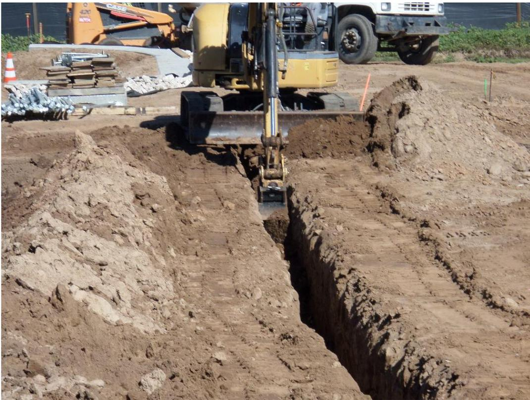
St. Denis Electric backfilling and compacting over PG&E conduit.
