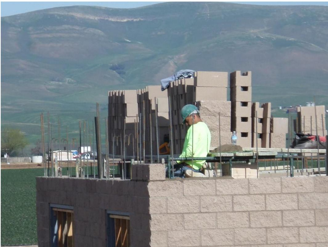
Boydston Masonry installing the corner lead at the pump station building.
