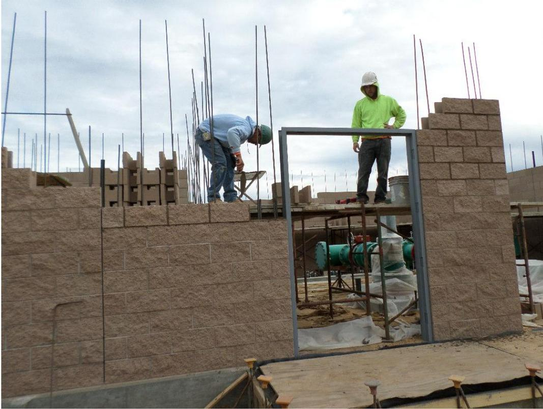
Boydston Masonry installing CUM along the west wall of the pump station building.
