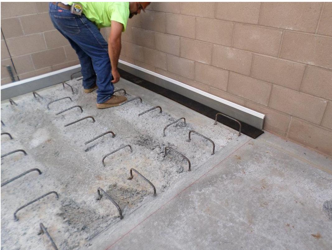
Spiess installing felt expansion joint at the chemical tank pad in the pump station building.
