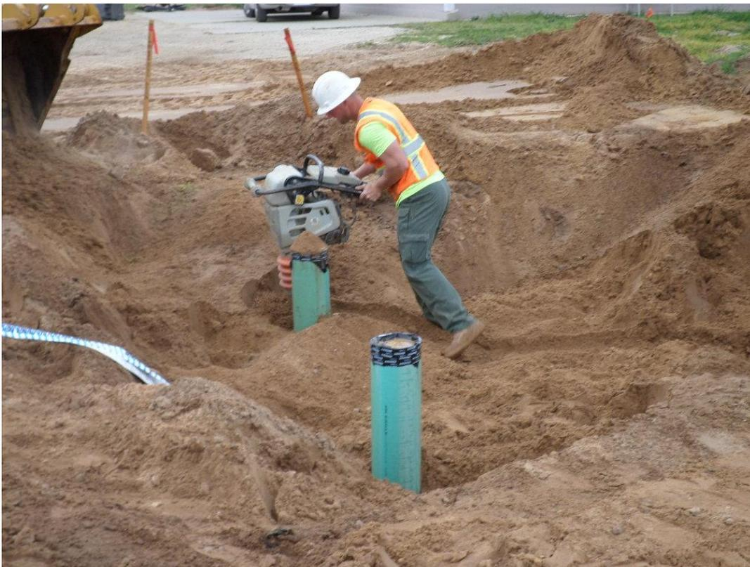
Spiess backfilling native material at entry gate over 24-inch DIP connection.
