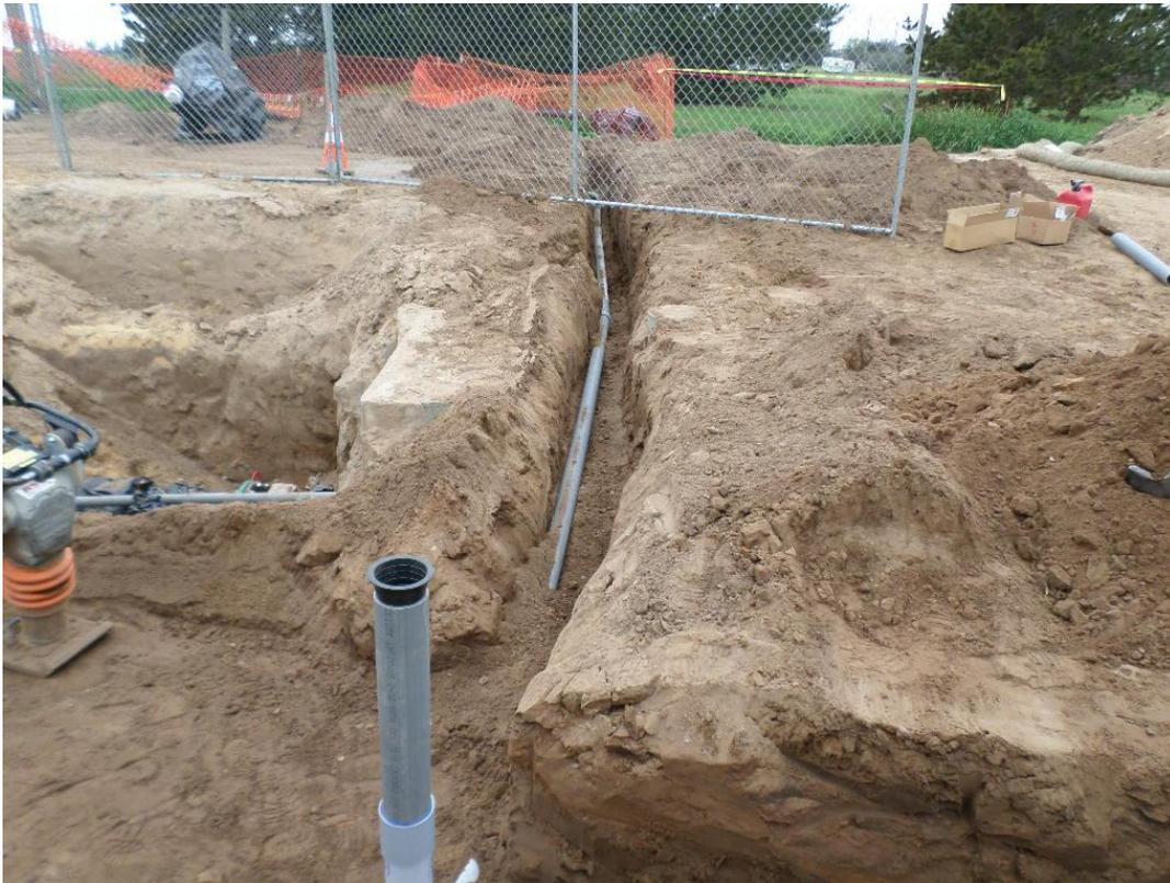
St. Denis Electric installing the main power feed to the PRV vault.
