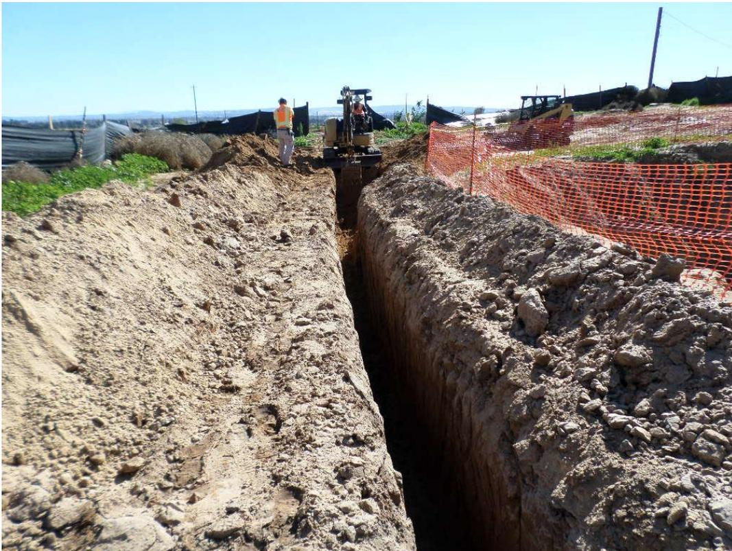
Spieß installing PG&E electrical conduit off site in easement to new pole location.
