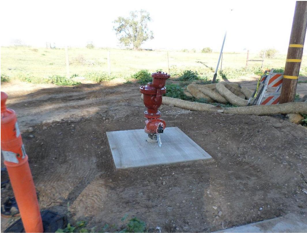
Combination air release valve installed and pad poured prior to cover being installed.
