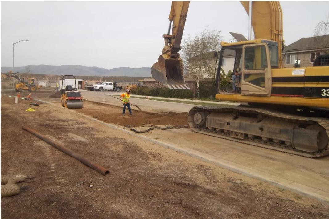
D-KAL removing sawcut pavement along trench edges in preparation for final paving at Blosser and Atlantic.
