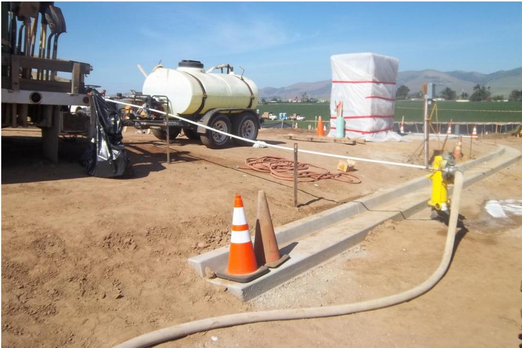
D-KAL using a “water buffalo” to inject chlorine into the pipeline at BP #4 and flush to the end at Taylor and Blosser to achieve 6 ppm throughout the line.
