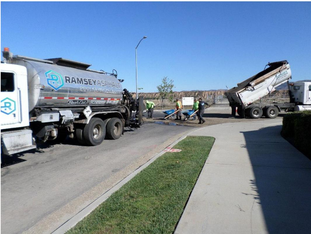
Ramsey Asphalt placing slurry seal at Blosser and Atlantic per the request of the City of Santa Maria.
