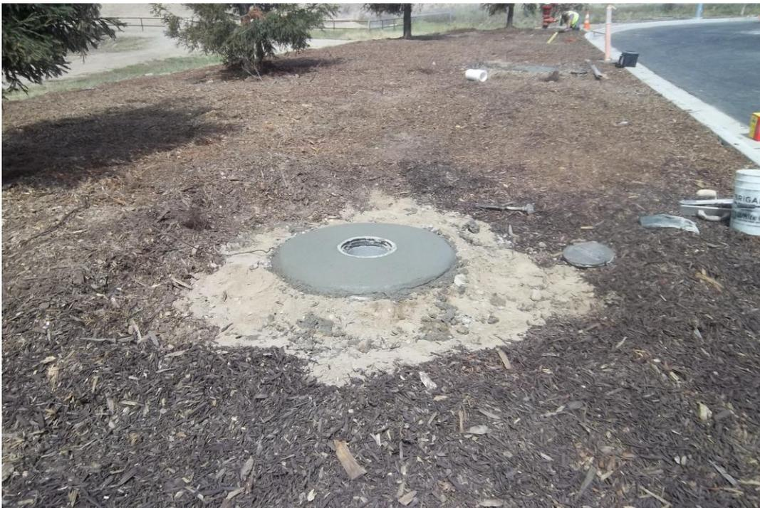
D-KAL finishing concrete collar at pig launcher.
