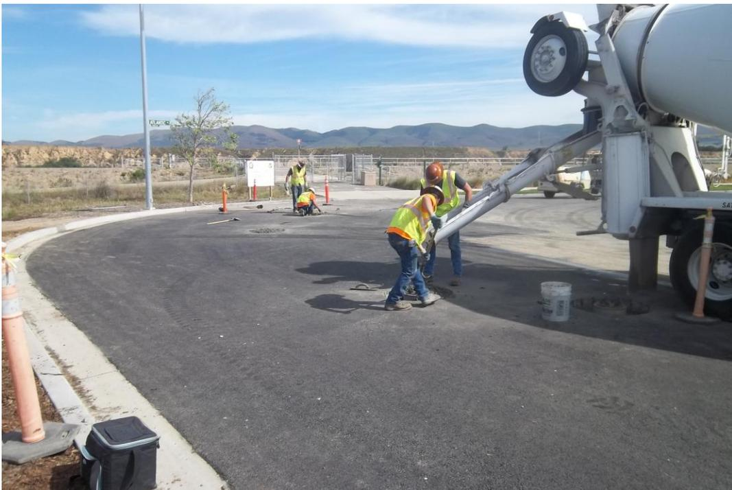
D-KAL pouring concrete collars around valve cans.
