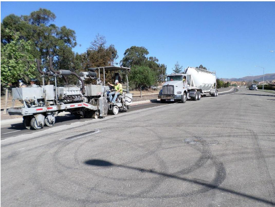
Grinding of the trench being performed under Ramsey Asphalt per the request of the City of Santa Maria.
