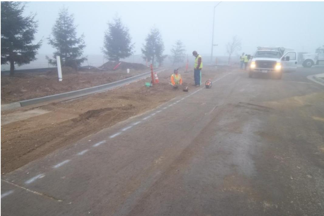
D-KAL preparing to sawcut trench for final paving section at Blosser and Atlantic.
