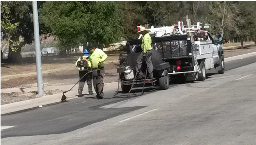
Ramsey Asphalt re-oiling trench edges of previously paved areas and oiling rock pockets in pavement.
