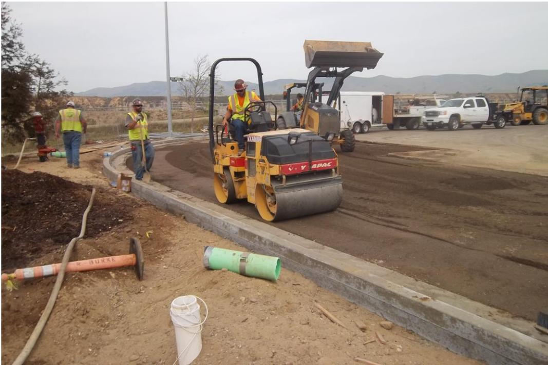
D-KAL compacting aggregate base at Blosser and Atlantic in preparation for final paving.
