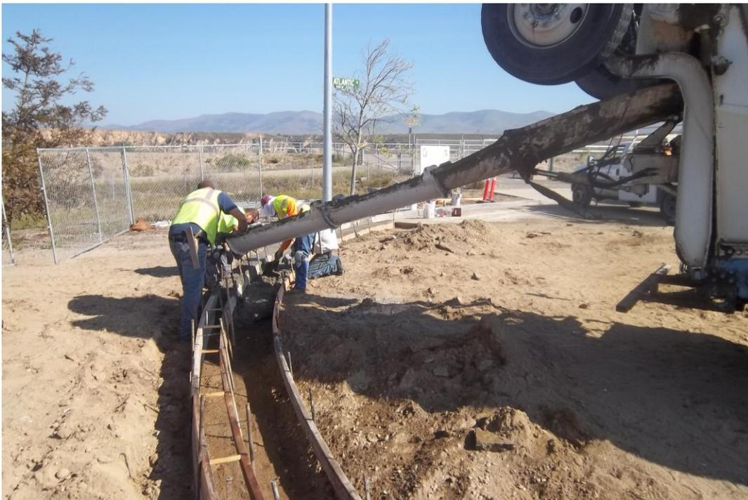
D-KAL pouring curb and gutter.
