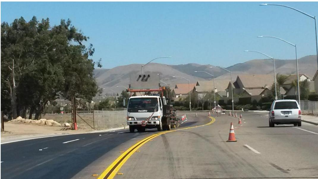
Toste restriping Blosser Road and replacing delineators.
