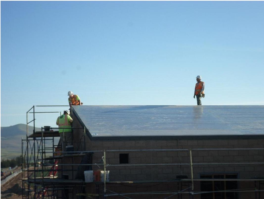
Steel roof deck installed.
