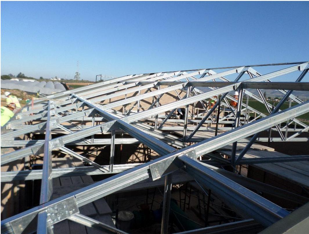
Spiess installing truss framing.
