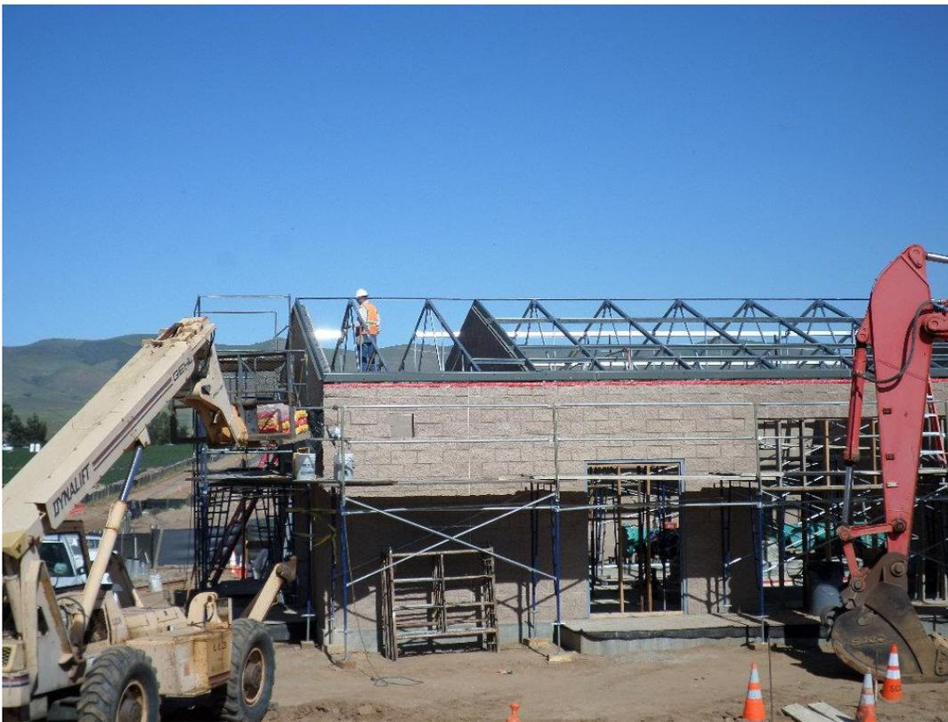
Spiess installing truss framing.
