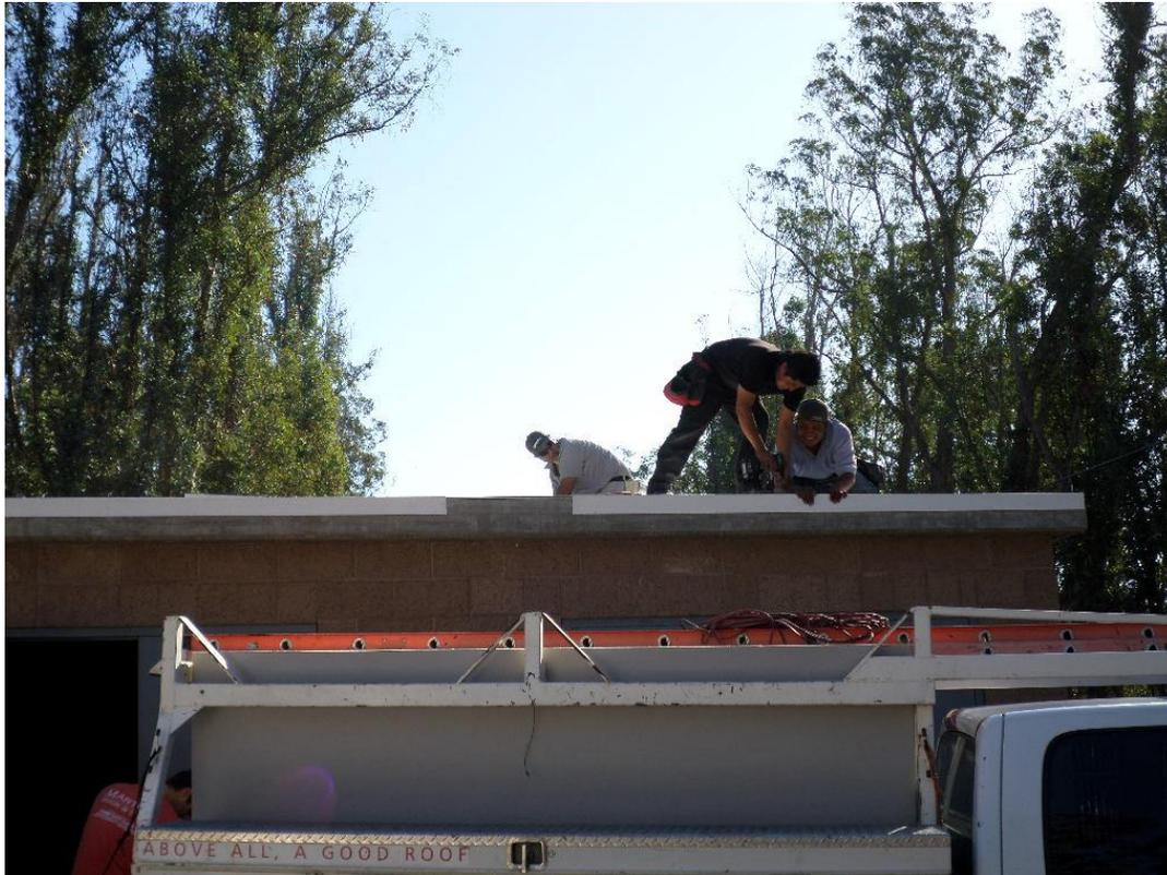
Quaglino Roofing installing the roof membrane.
