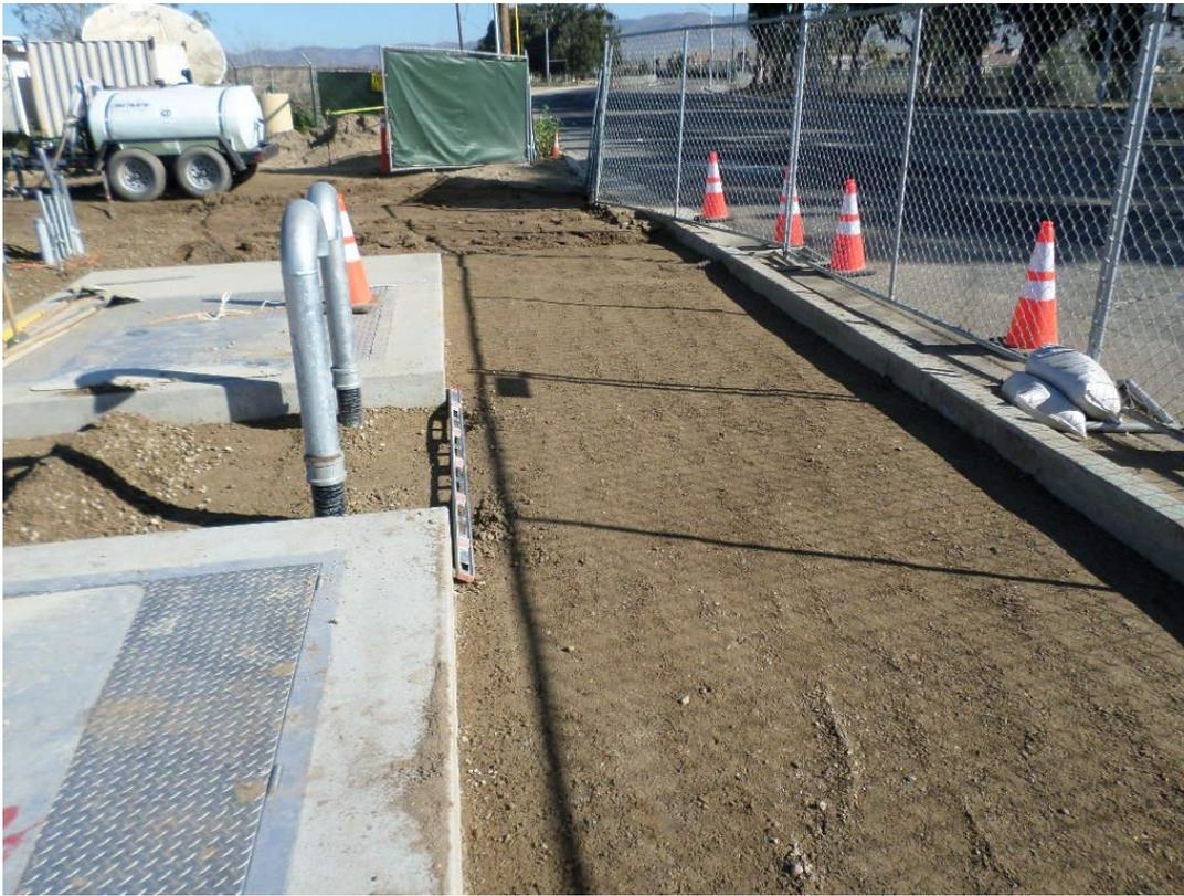
Placing base material around metering vaults.
