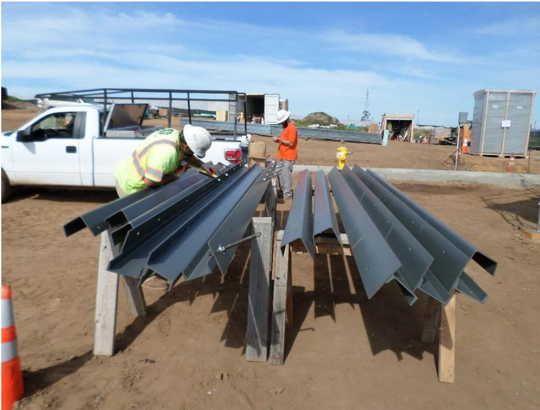
Spiess attaching bolts to roof steel plates.
