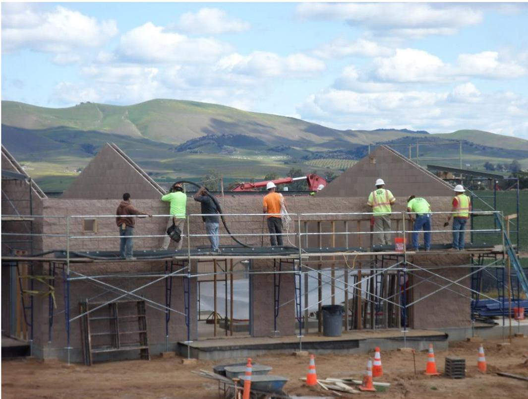
Boydston Masonry pouring final grout while Spieß set steel plates for roof.
