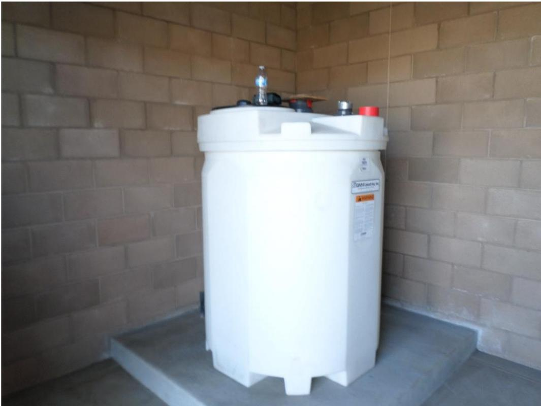
Chemical tank installed at pump station.
