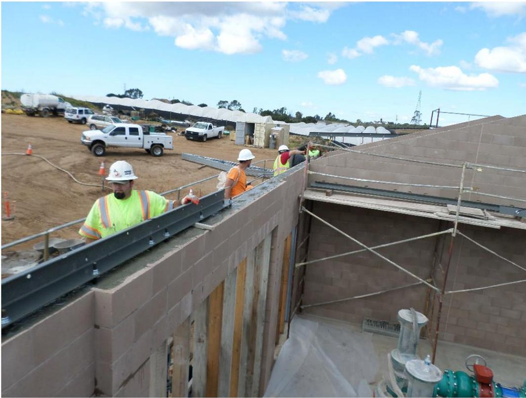
Spieß setting steel roof plates in grout.
