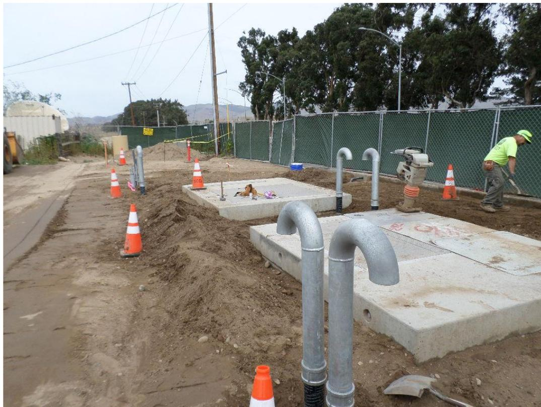
Spiess installing vent piping at metering vaults.
