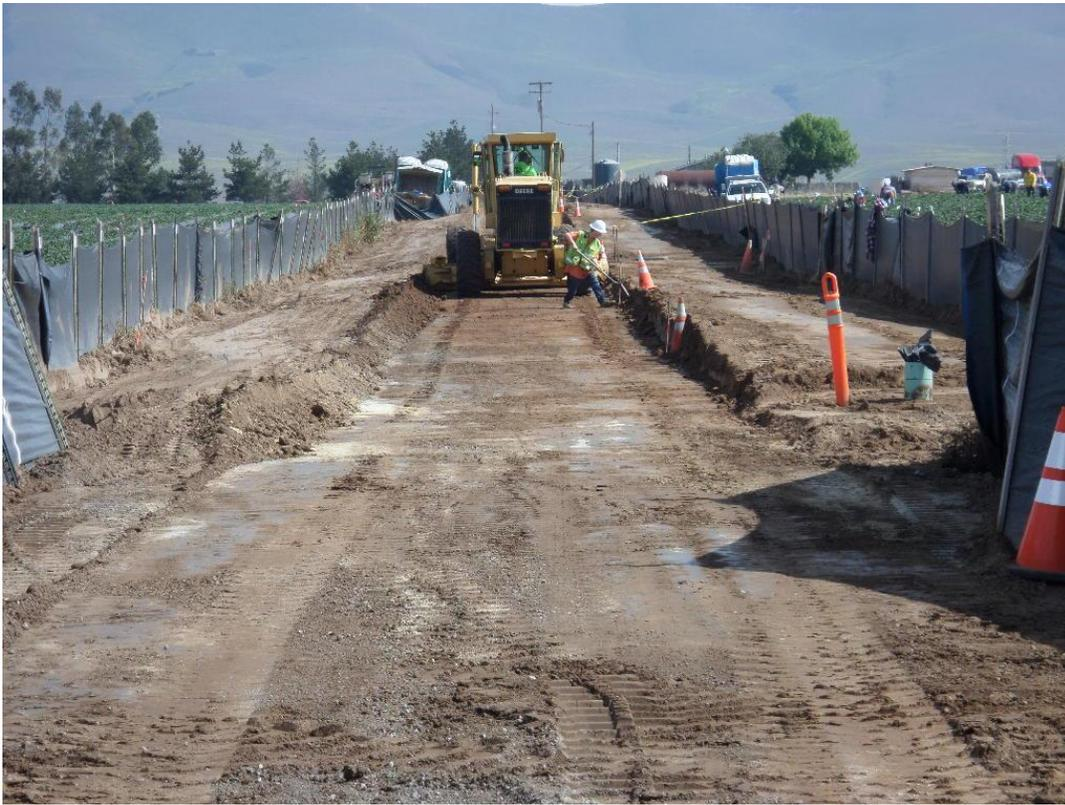
Spieß cutting the access road to subgrade to build permanent access road.
