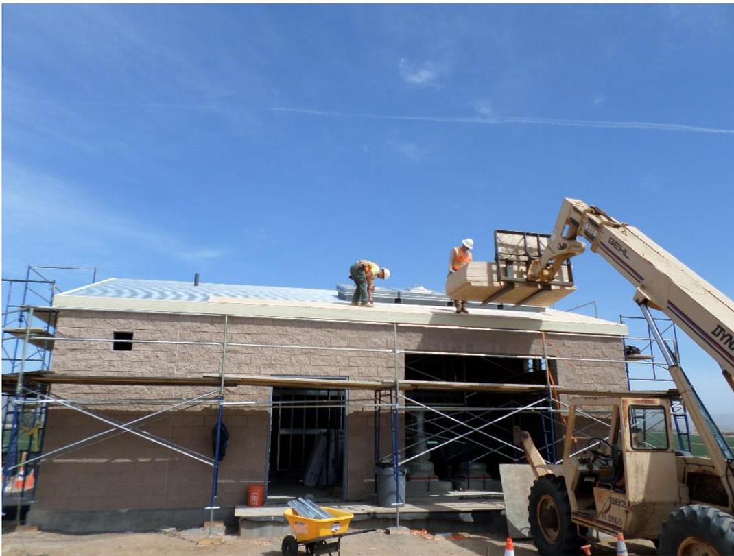
Spieß installing plywood sheeting on pump station roof.
