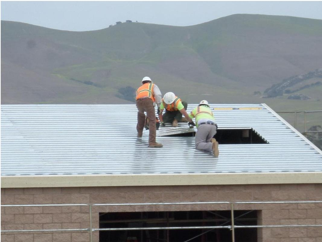
Spies cutting openings for roof hatches.
