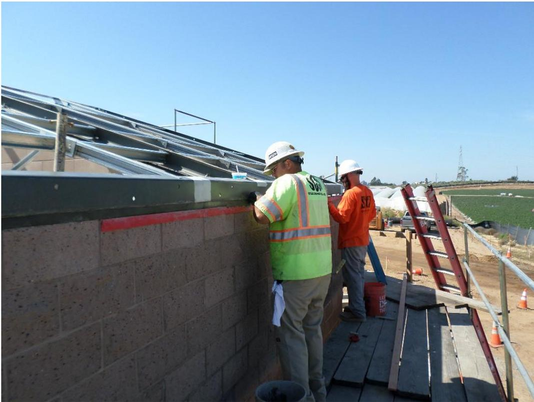
Spieß dry packing grout under steel roof frame plate.
