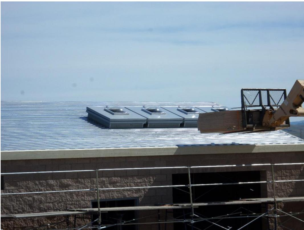
Roof hatches installed.
