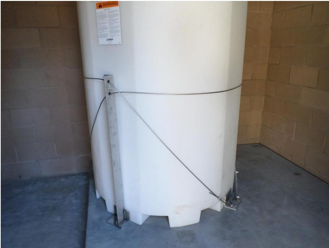
Chemical tank installed with tie-downs.
