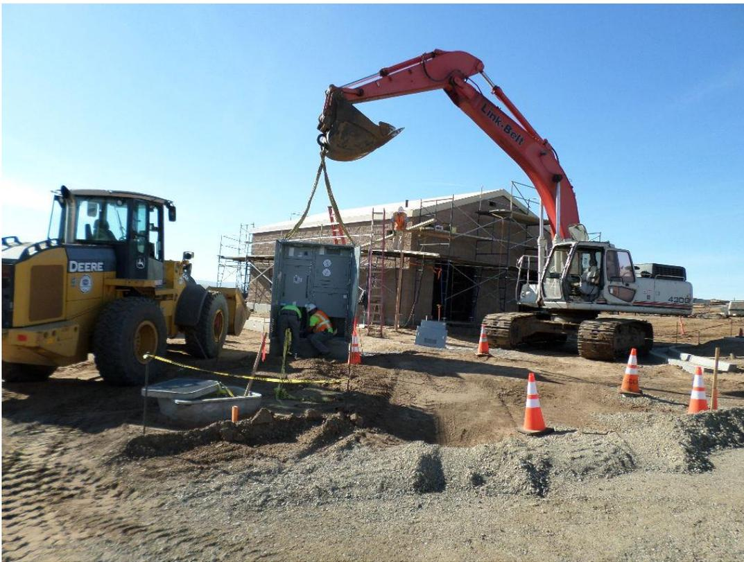
St. Denis Electric installing PG&E metering station.
