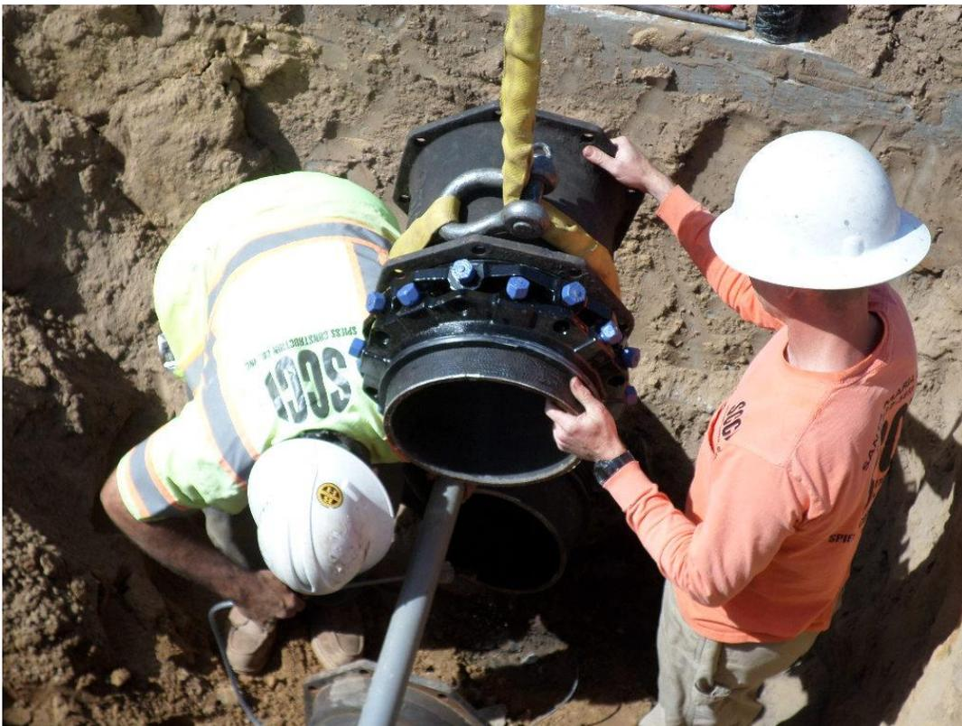
Spies making the final tie-in to the 12-inch water line at the PRV vault.
