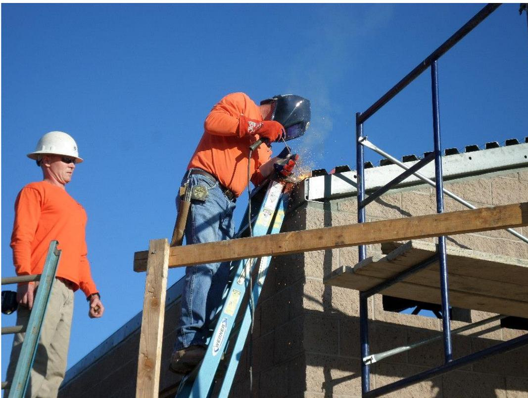
Puddle welding at steel roof plates.
