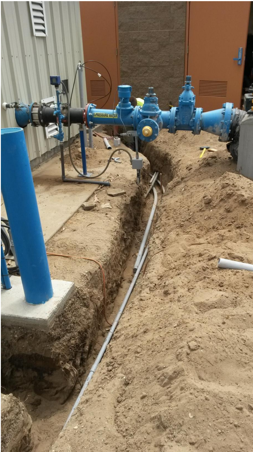
St. Denis Electric installing underground conduit.
