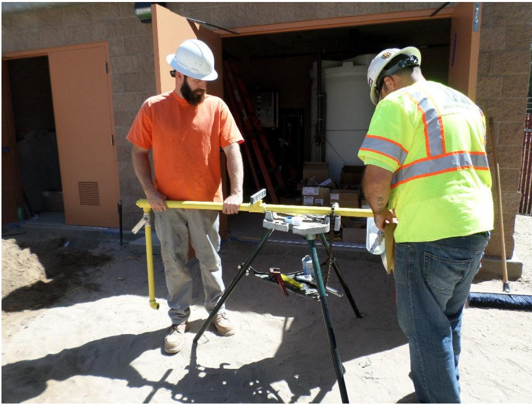
Spiess assembling eyewash station.
