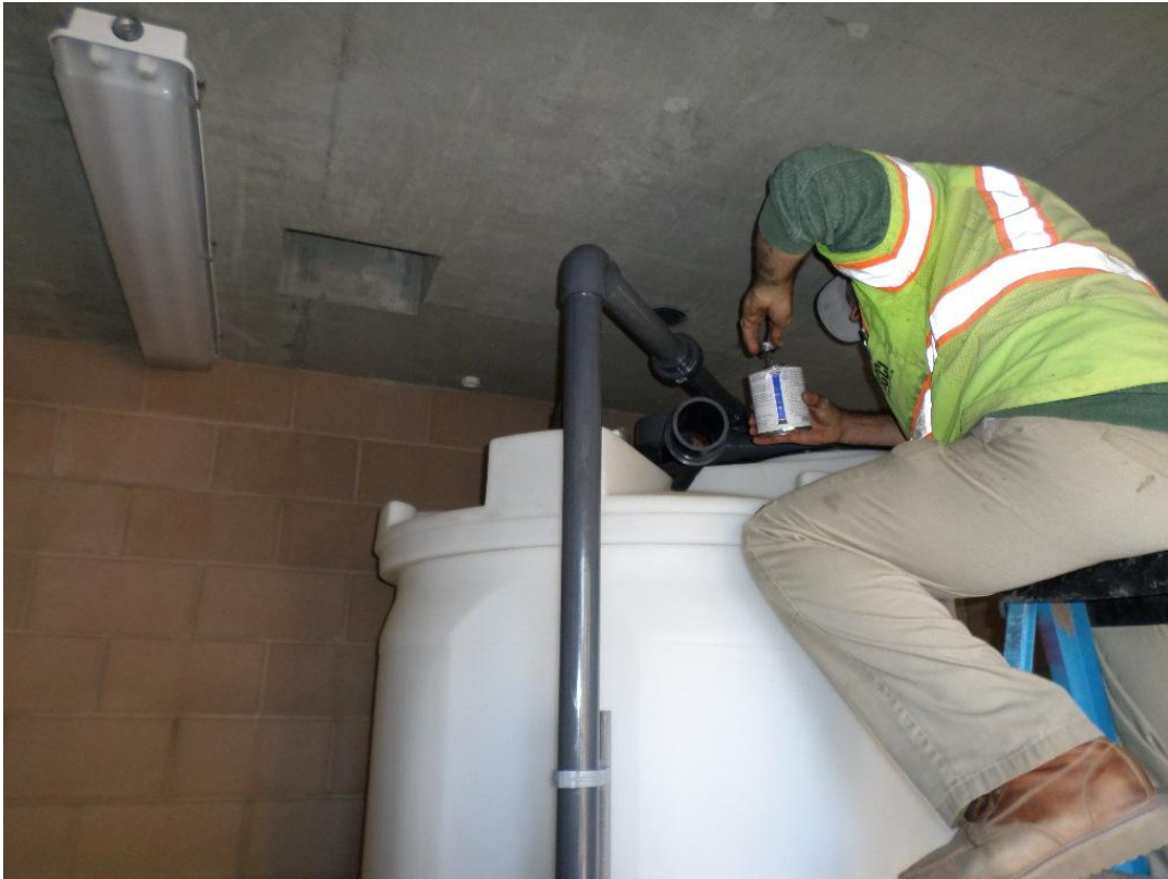
Spiess installing overflow piping on the chemical tanks.
