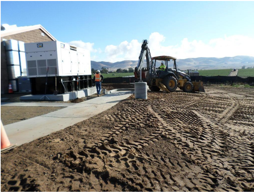
Grading bank between facilities and future fence.
