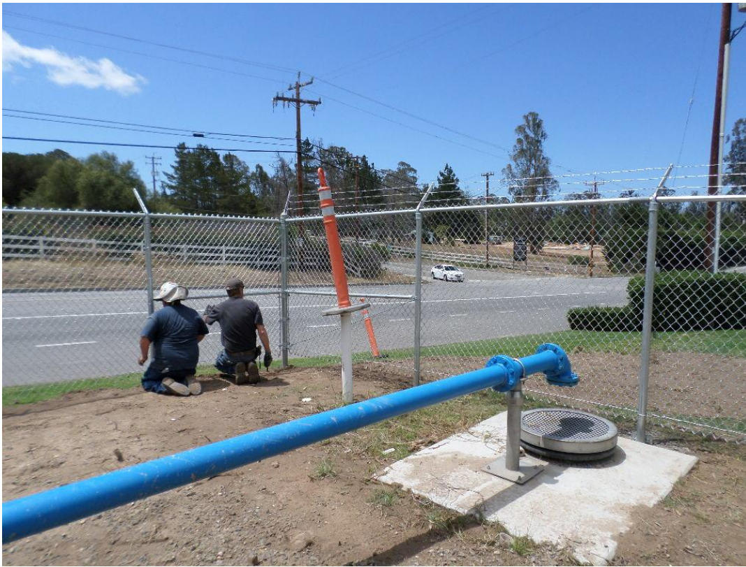
Central Coast Fence installing new fence.
