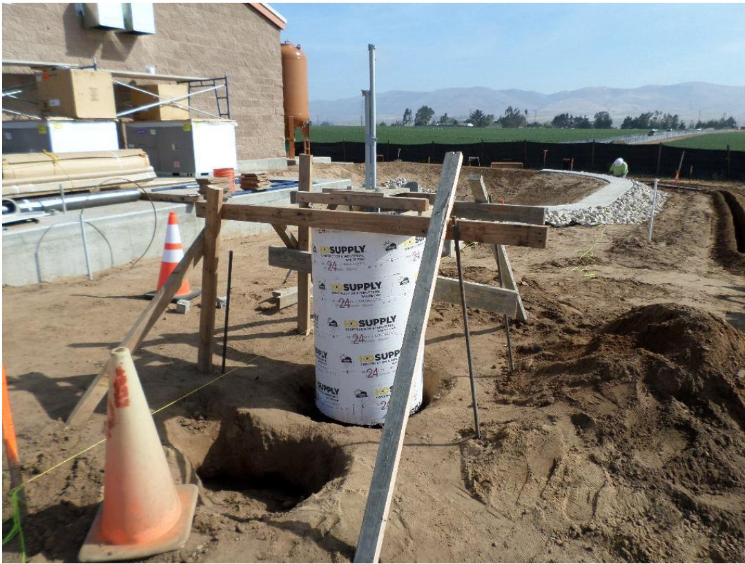
Light pole base formed and reinforcing and conduit installed.
