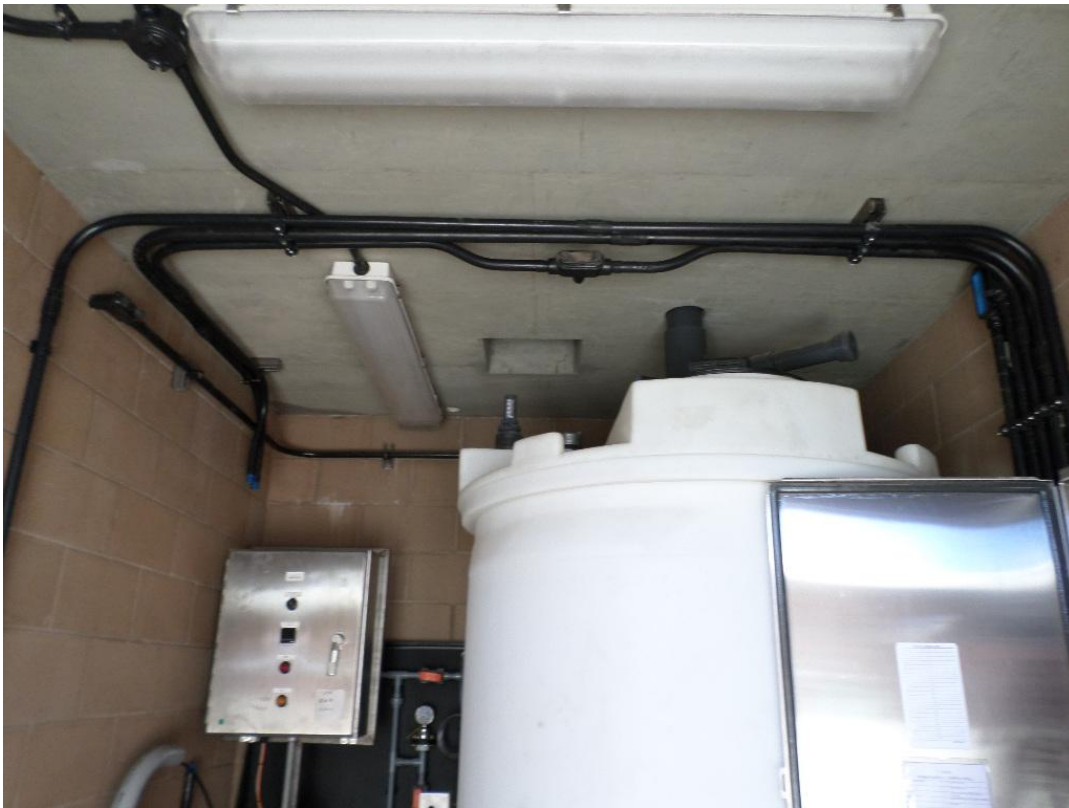
Conduit being installed by St. Denis Electric.
