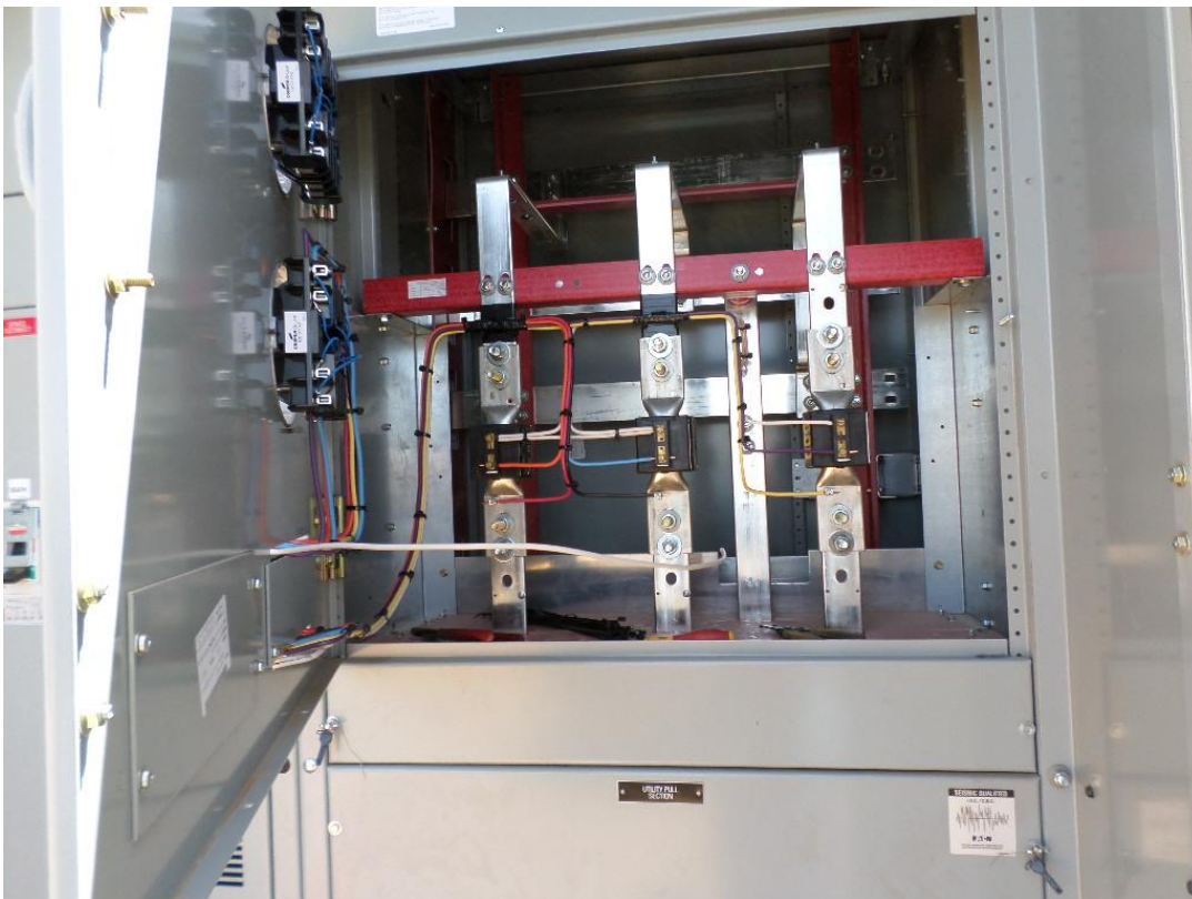
PG&E terminating wires in the electrical service panel.
