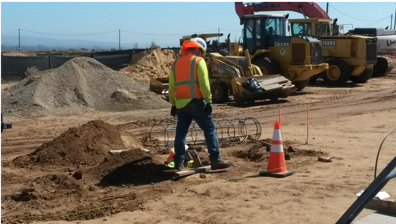
St. Denis Electrical auguring for light pole base.
