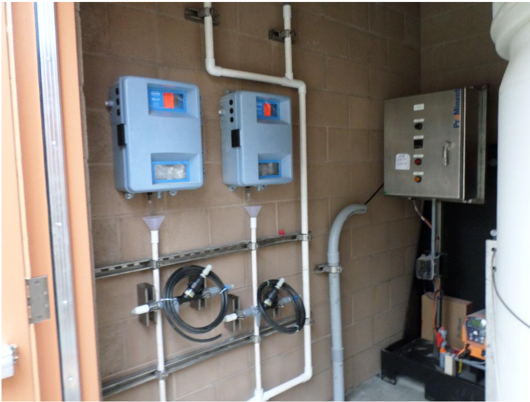
Chemical analyzer piping installed.
