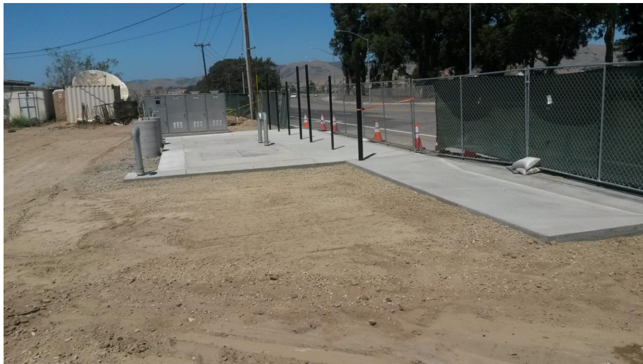
Driveway with forms removed and site graded.
