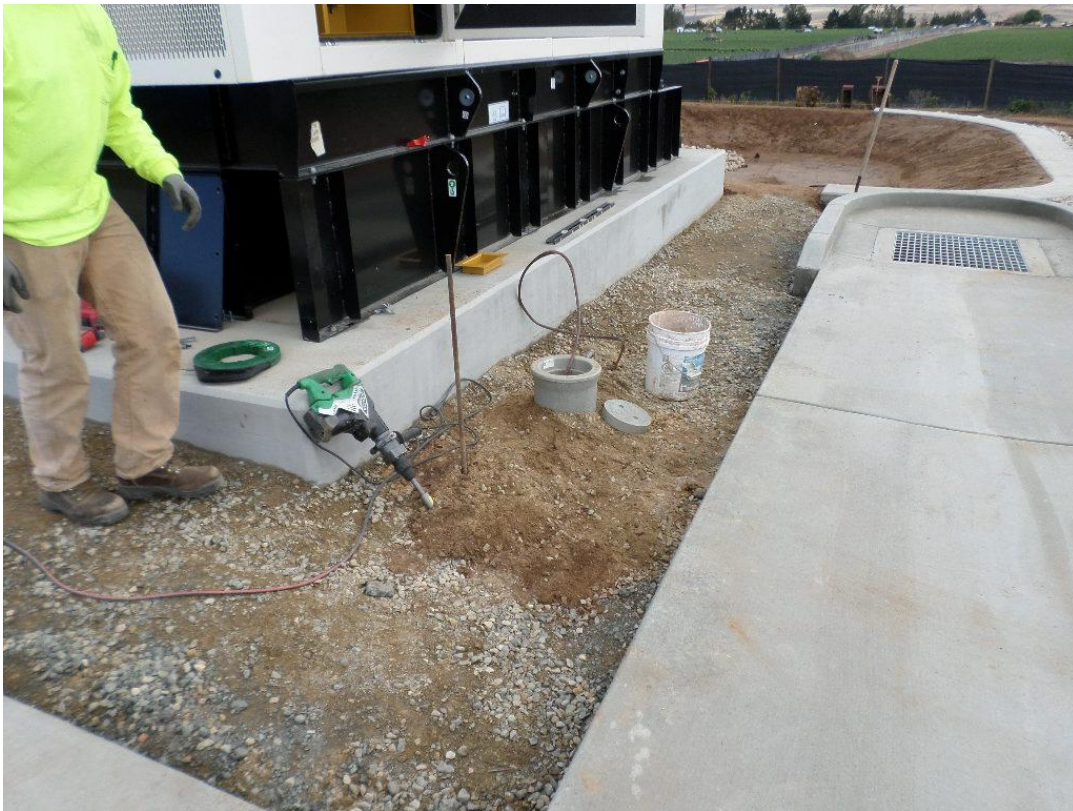
Installing grounding rod for emergency generator.
