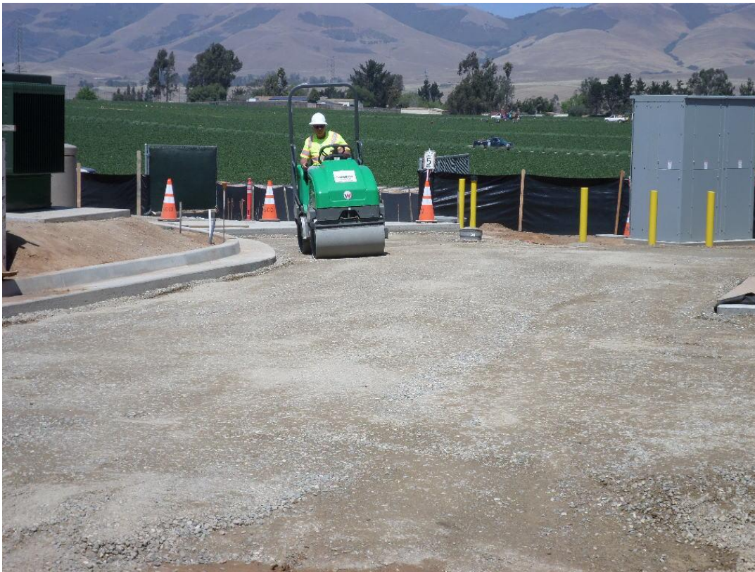
Spiess compacting aggregate base for driveway around building.
