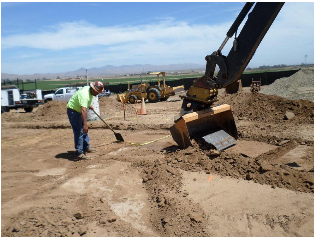
Spiess starting excavation for V-ditch.
