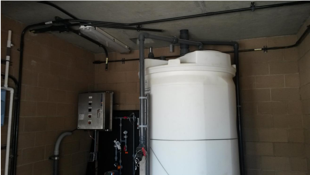
Lighting being installed by St. Denis Electric.
