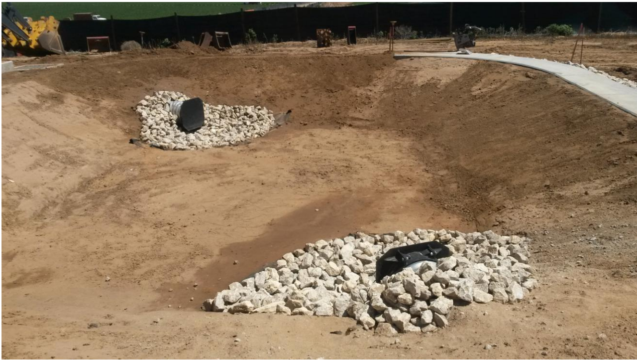
Retention basin with fabric and drain rock installed at storm drain inlets.
