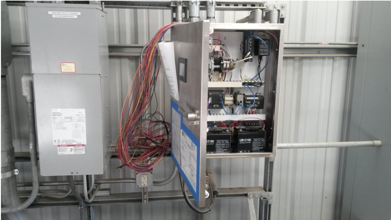
St. Denis Electric pulling wire.
