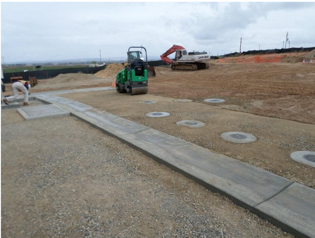
Compacting aggregate base.
