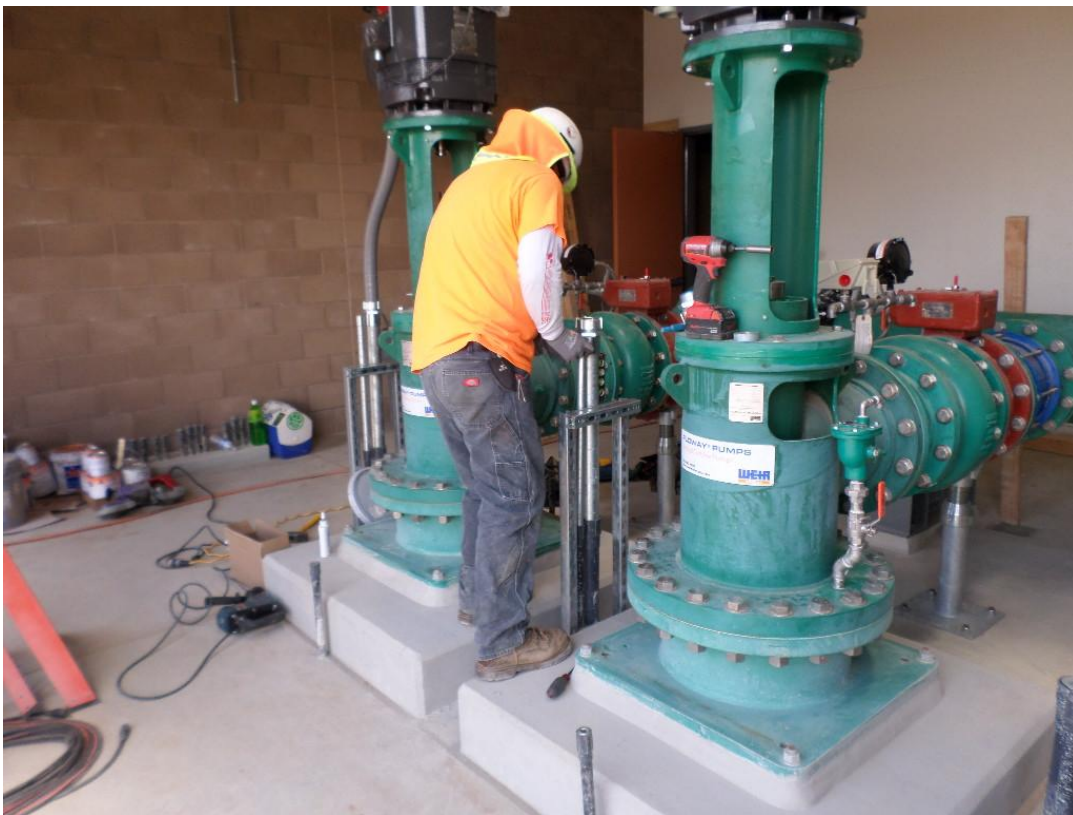
Spieß installing rack and conduit at pumps.
