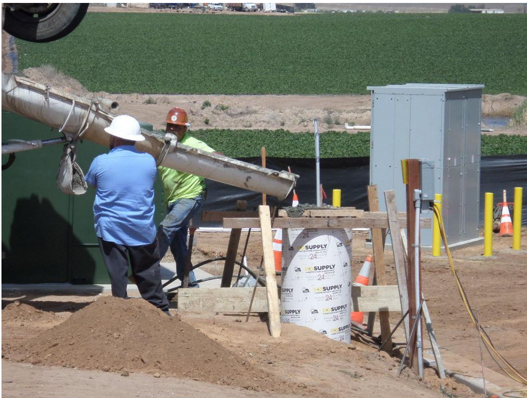
Pouring the light pole base.
