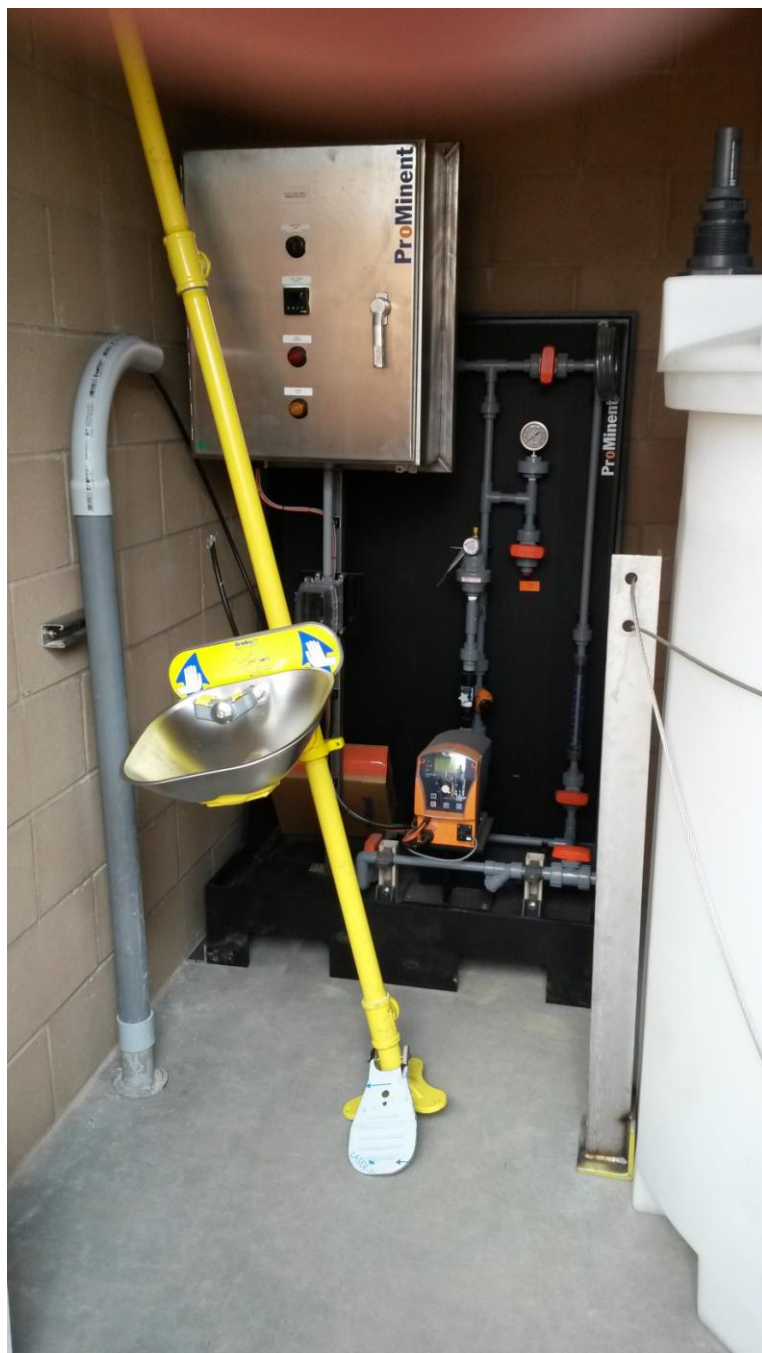
Ammonium sulfate chemical skid installed (eye wash station assembled).
