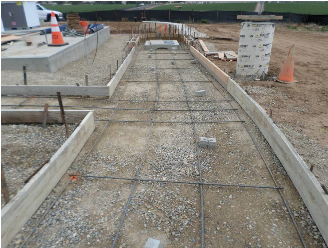
Reinforcing installed in six foot V-ditch.
