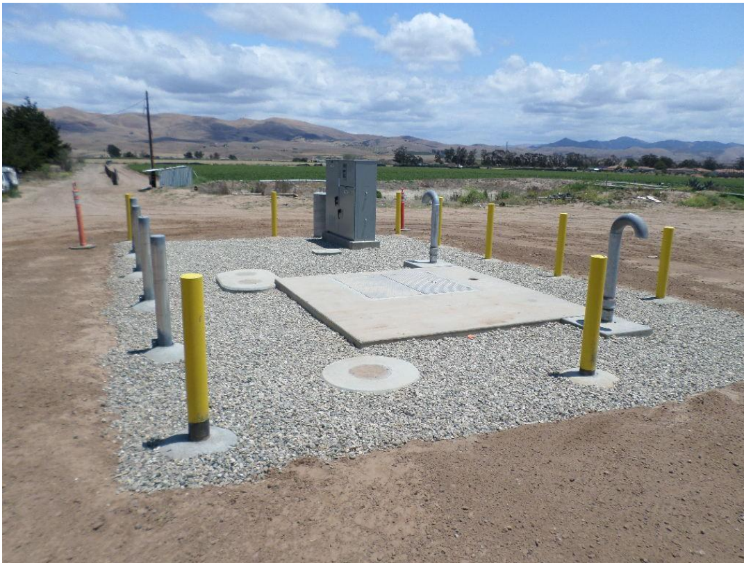
Rock placed around PRV vault site.
