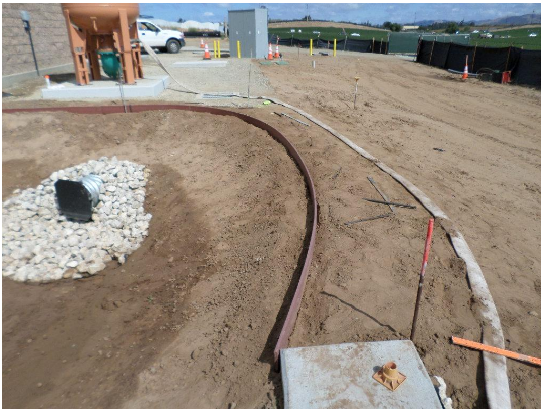
Bender board installed around perimeter of retention basin.
