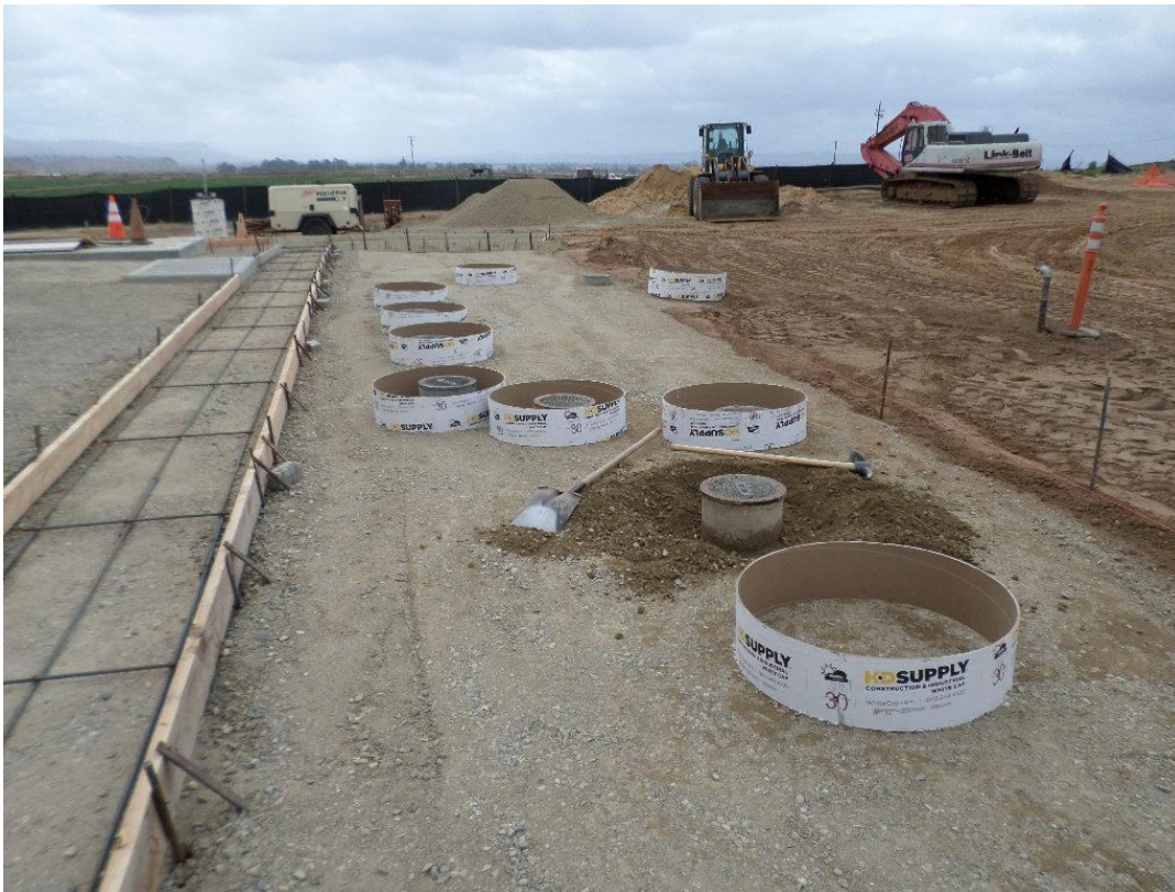
Forms for pouring valve can collars.
