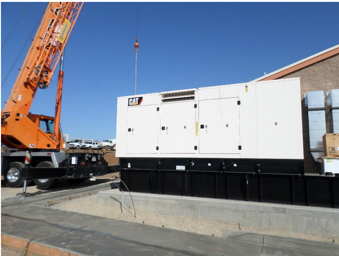
Spiess setting emergency generator onto pad.
