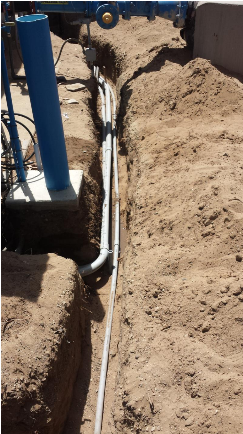
Underground conduit being installed by St. Denis Electric.
