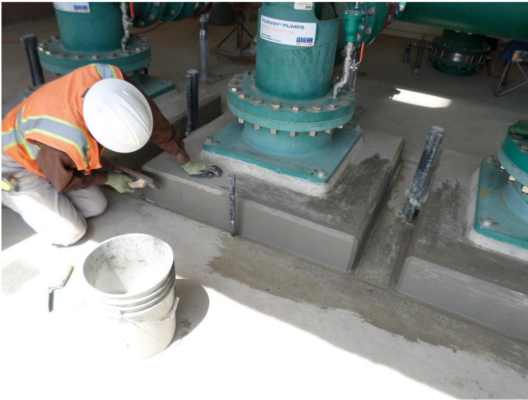
Spieß patching surface defects in concrete pump pads.
