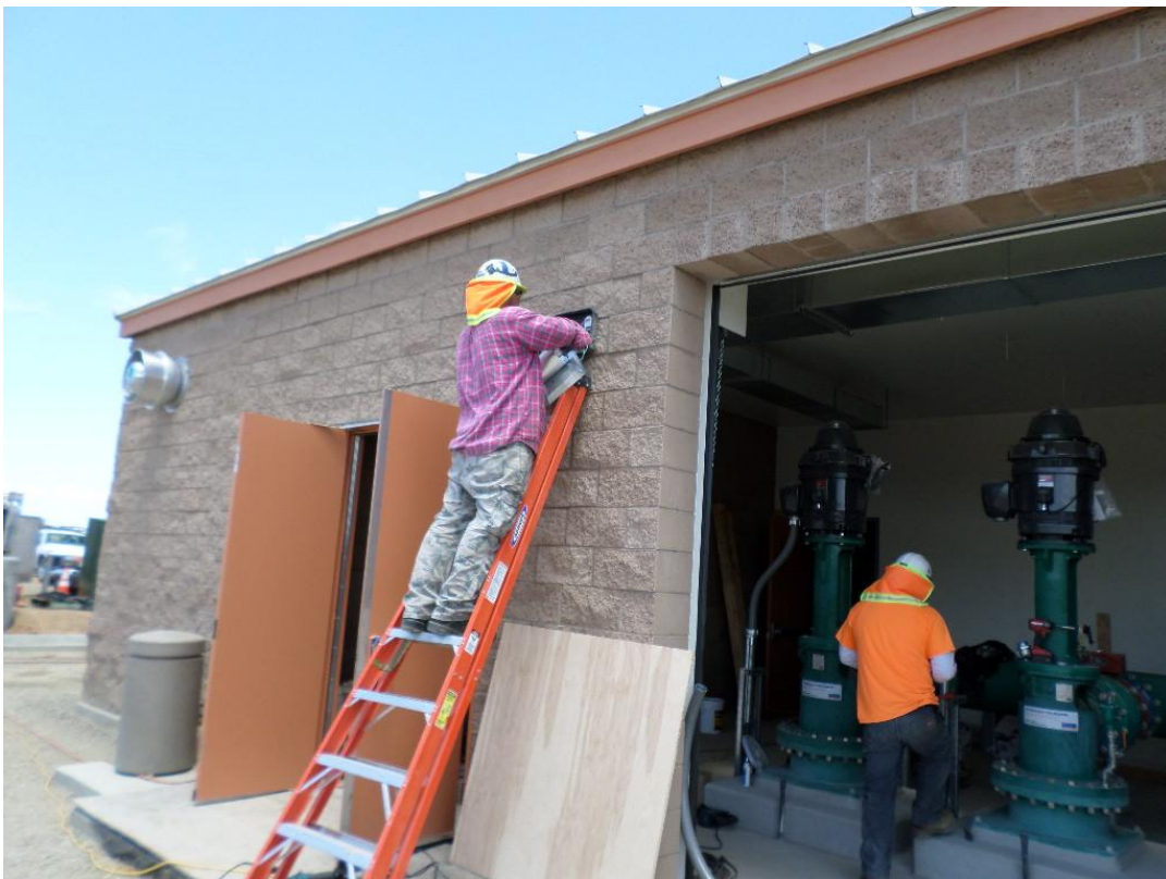
St. Denis Electric installing exterior lights around pump station building.
