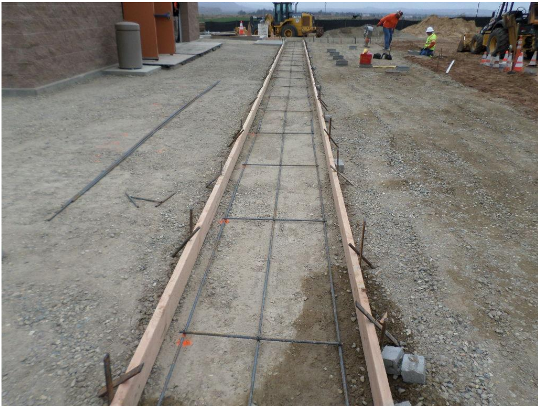
Reinforcing installed at three foot V-ditch.
