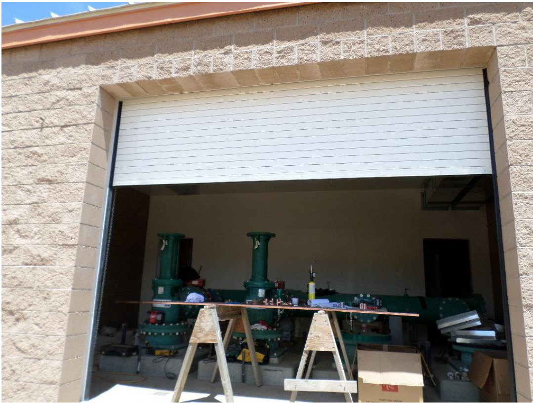
Roll-up door installed for the pump room.
