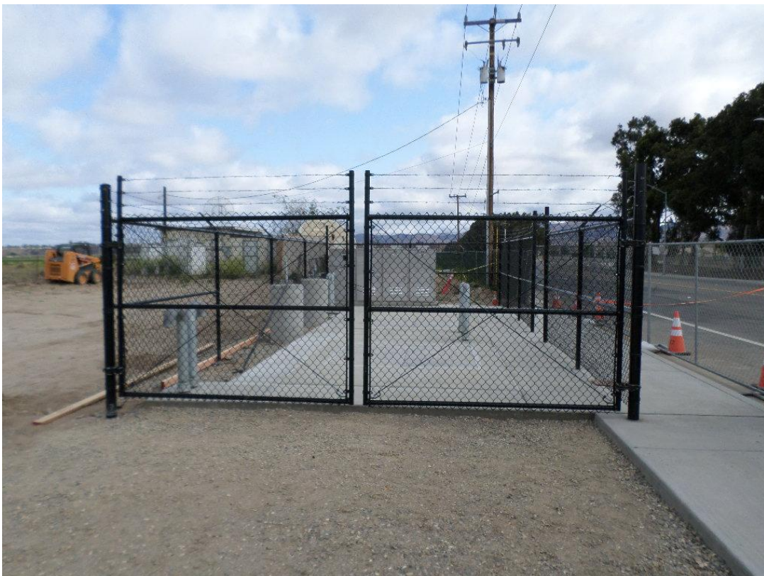
Vehicle access gate installed.
