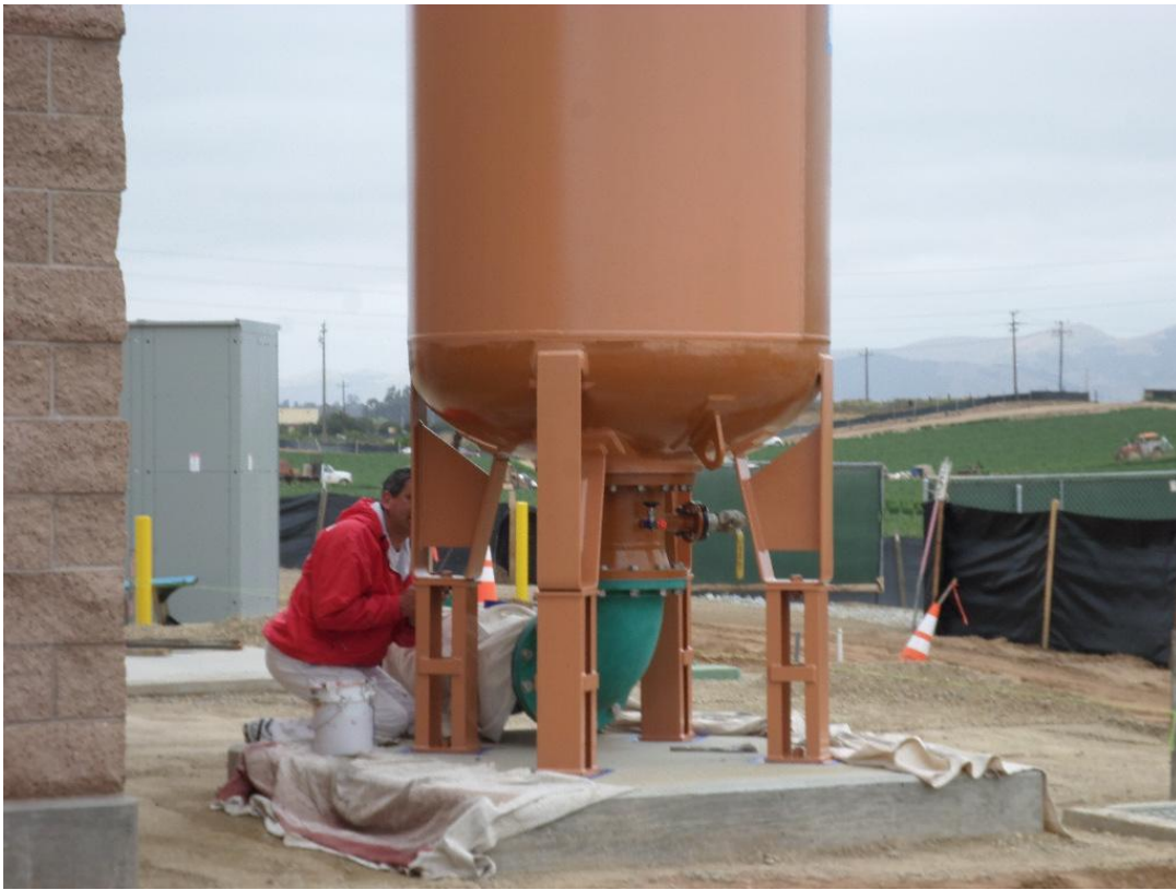
Coast Painting coating supports for surge tank.
