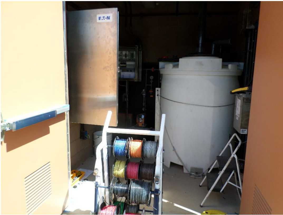
St. Denis Electric pulling wires.
