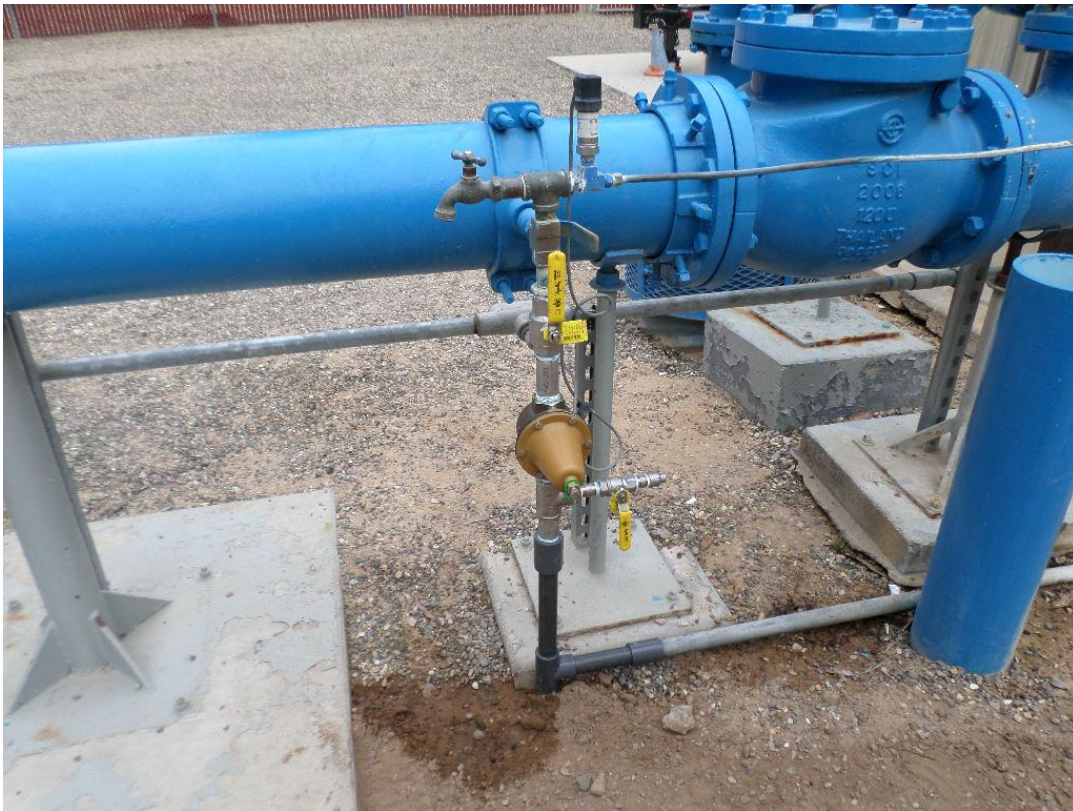
Spiess installing pressure reducer.
