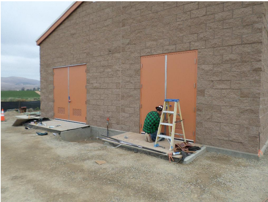
Martin Doors installing hardware on doors.
