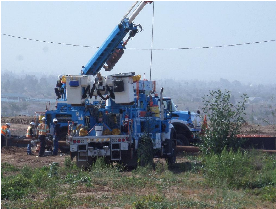
PG&E installing power pole for electrical service to the pump station.
