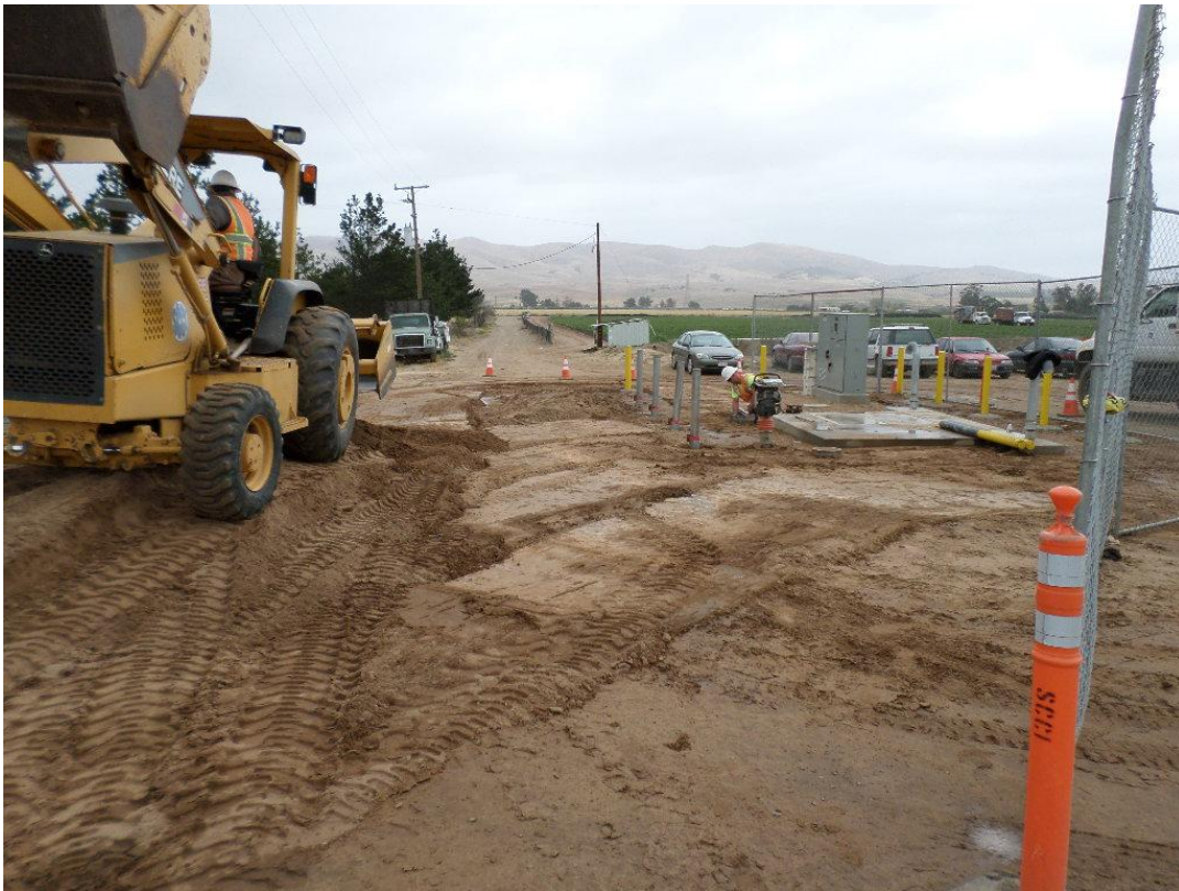
Spieß grading around PRV vault.
