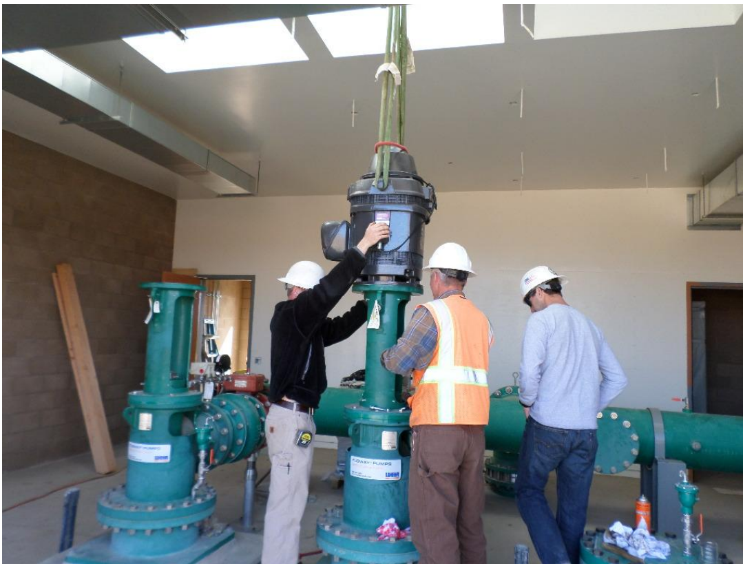
Spiess installing pump motors.
