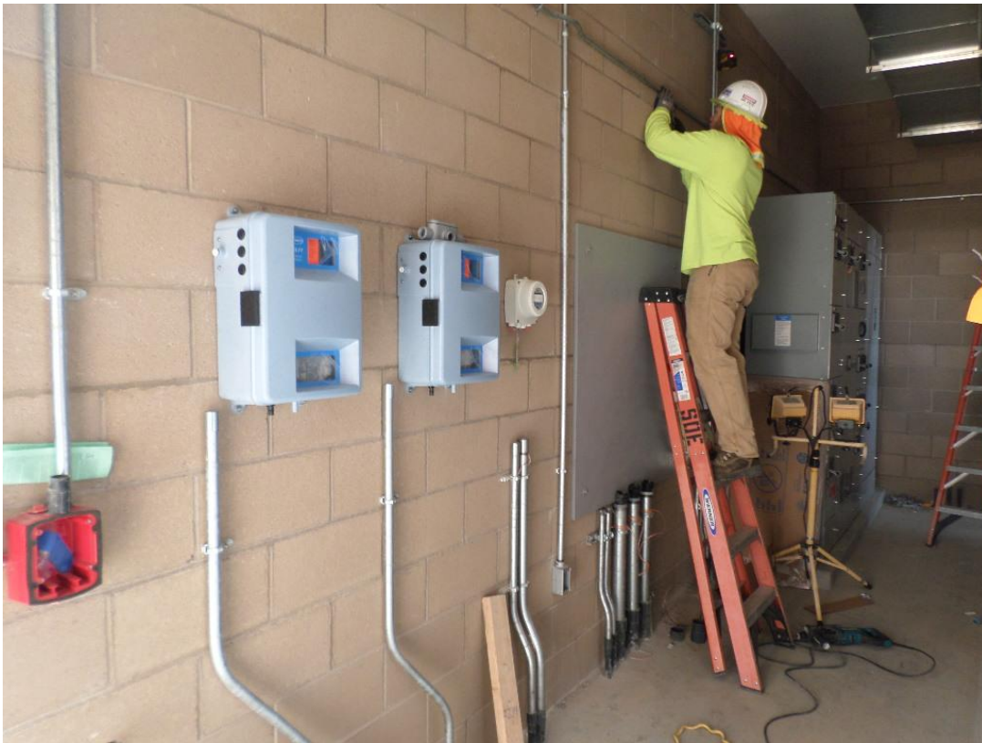
Installing exposed conduit in electrical room.
