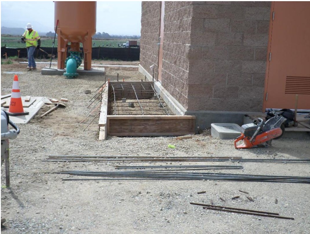
Spies forming sidewalk to electrical room.
