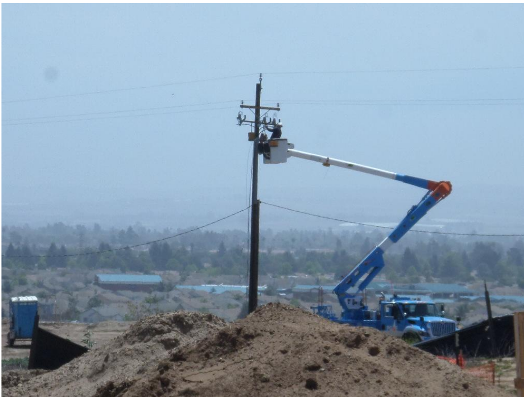
PG&E connecting the main electrical feed at the pole.
