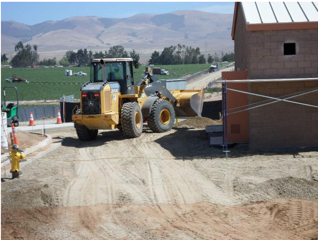
Spiess spreading aggregate base around the building.
