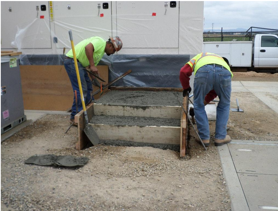
Spieß pouring emergency generator access steps.
