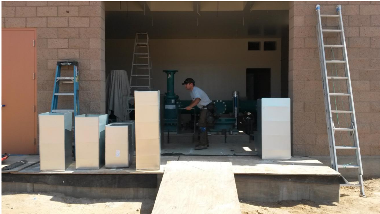
DAHL Air Conditioning installing HVAC ducting inside pump room.
