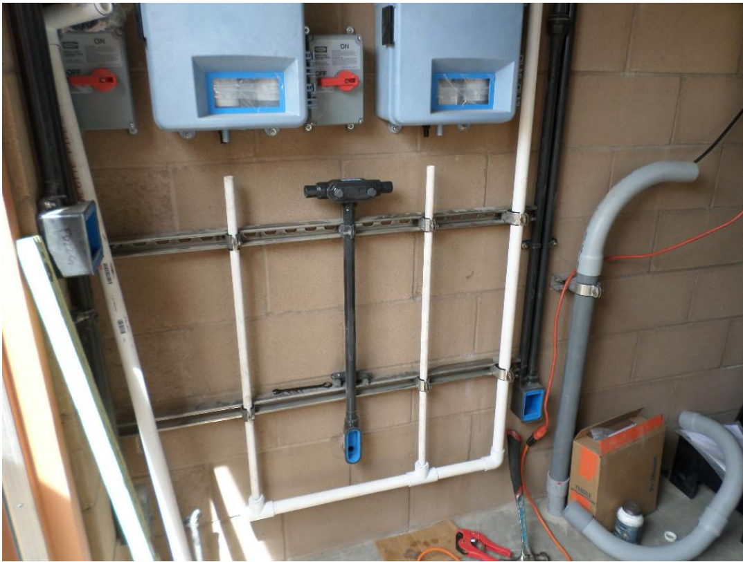
Chemical analyzer piping being installed.
