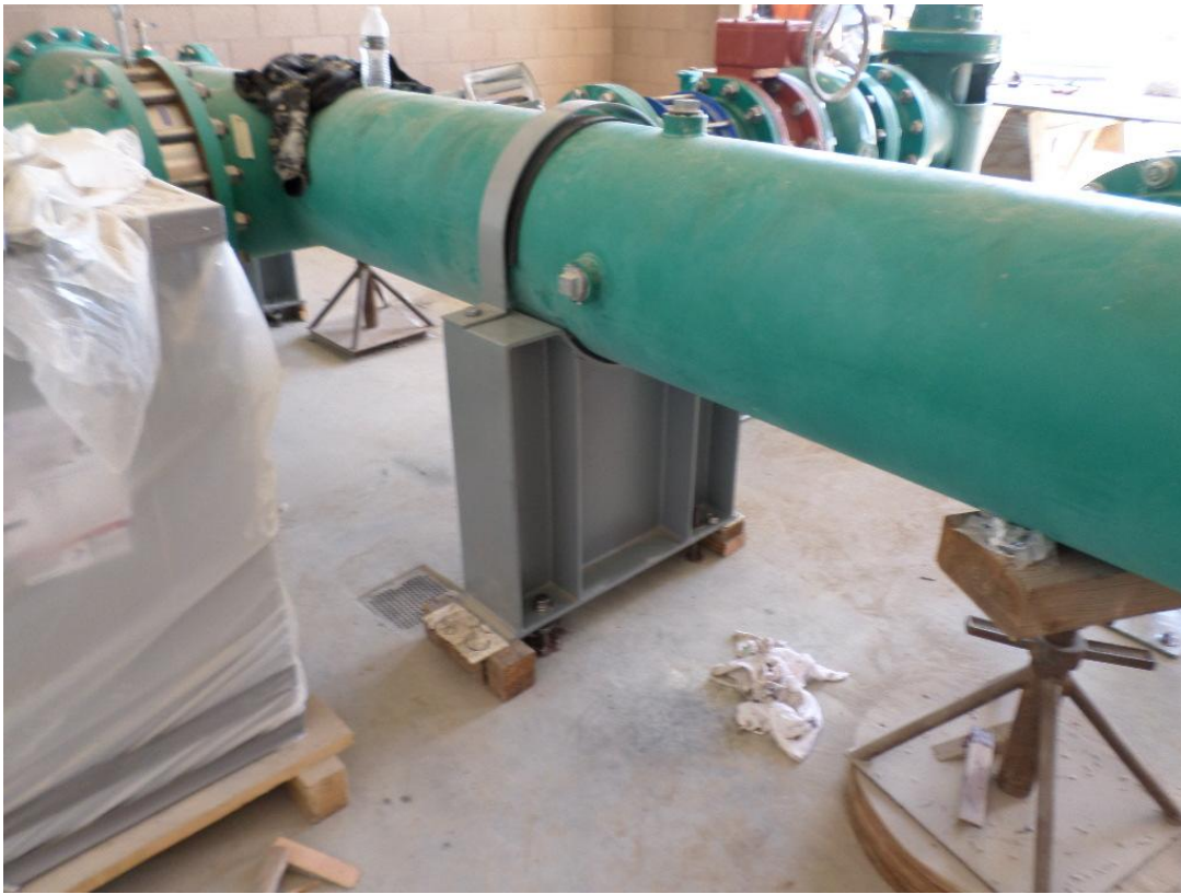
Spiess installing pipe supports in the pump room.
