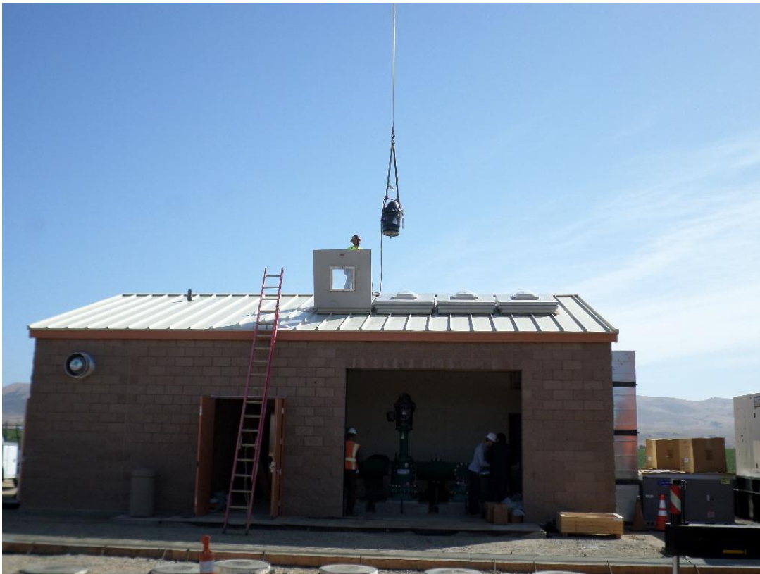
Spiess installing pump motors through access hatches in roof.
