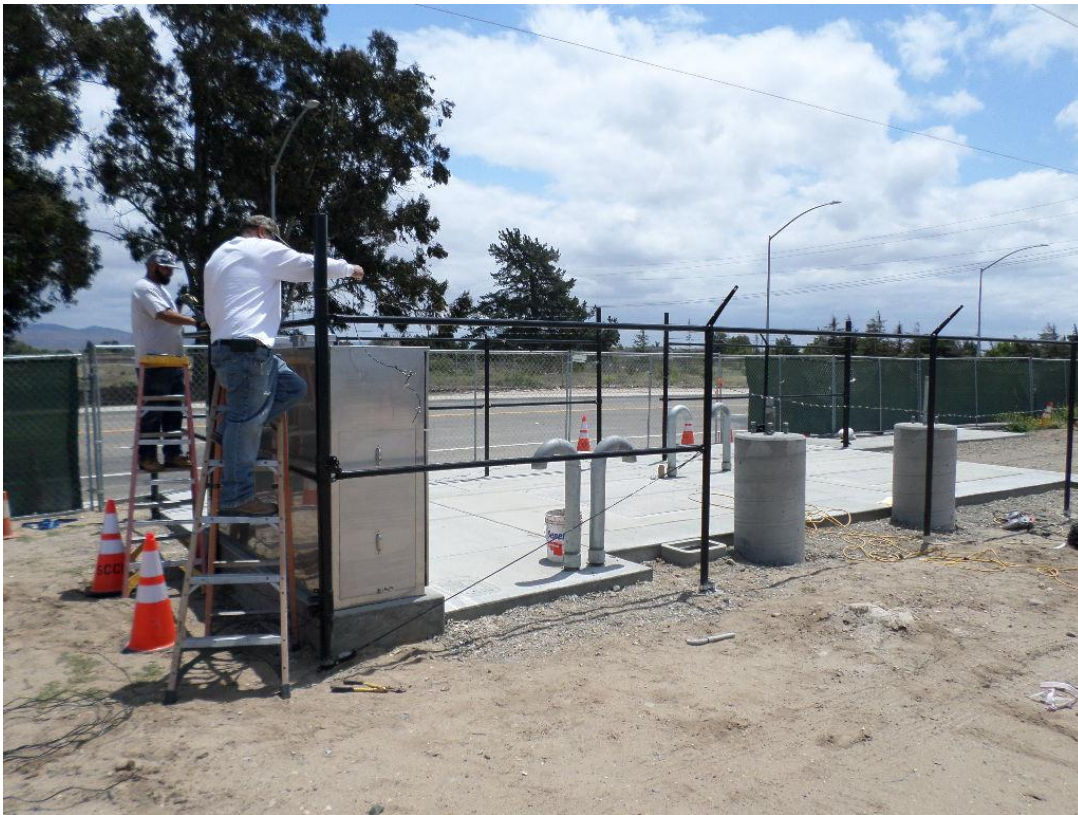
Central Coast Fence installing perimeter fencing.
