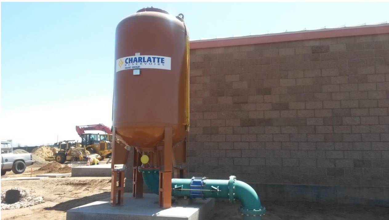
Surge tank anchored.
