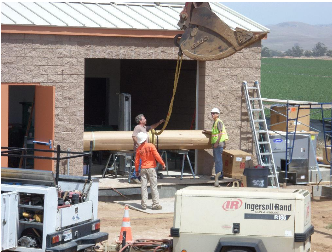
Installing the roll-up door for the pump room.
