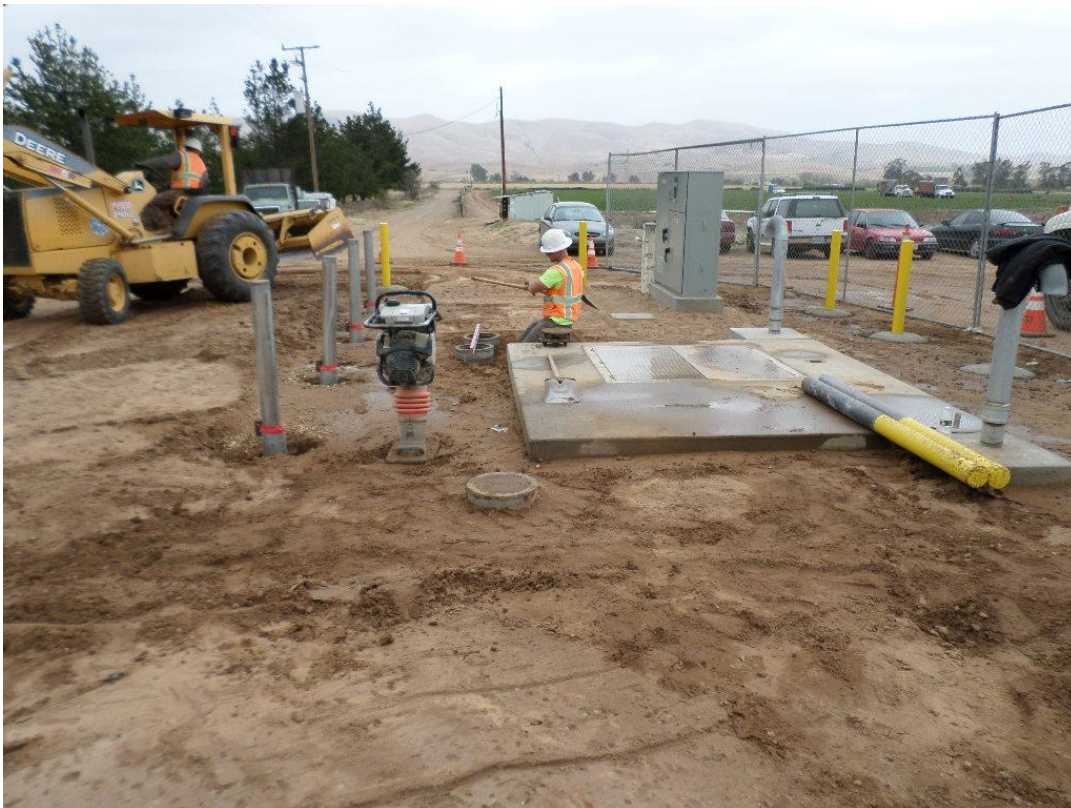
Spieß raising valve cans around PRV vault.
