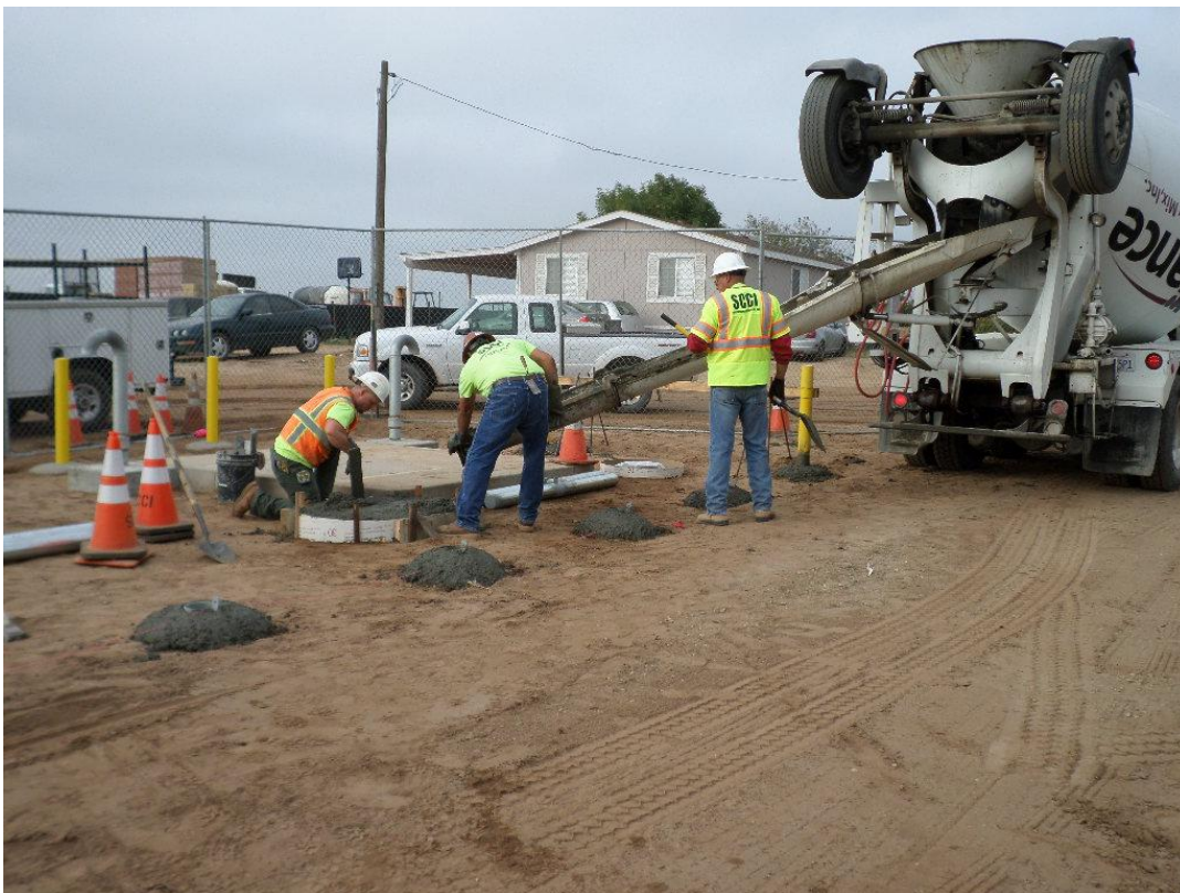
Spies pouring bollards and valve can collars.
