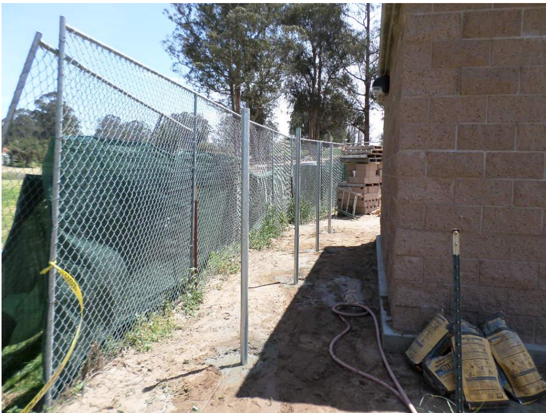
Central Coast Fence installing fence posts.
