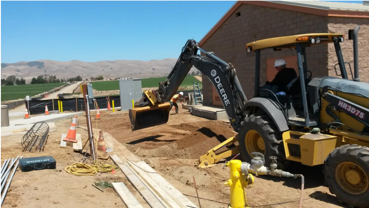
Spiess continuing to remove native material around site in preparation for installation of aggregate Base driveway.
