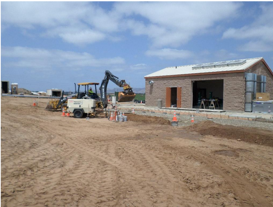
Spies grading around valve cans.
