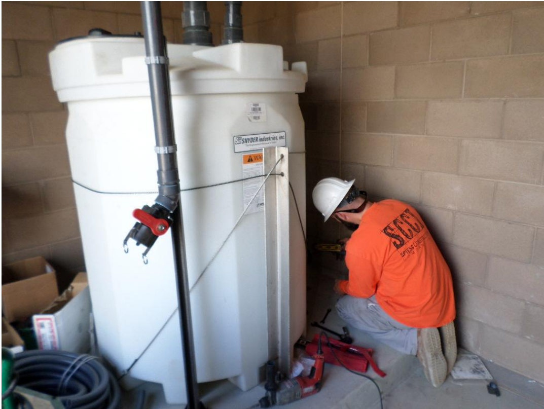
Spiess installing chemical tank piping.
