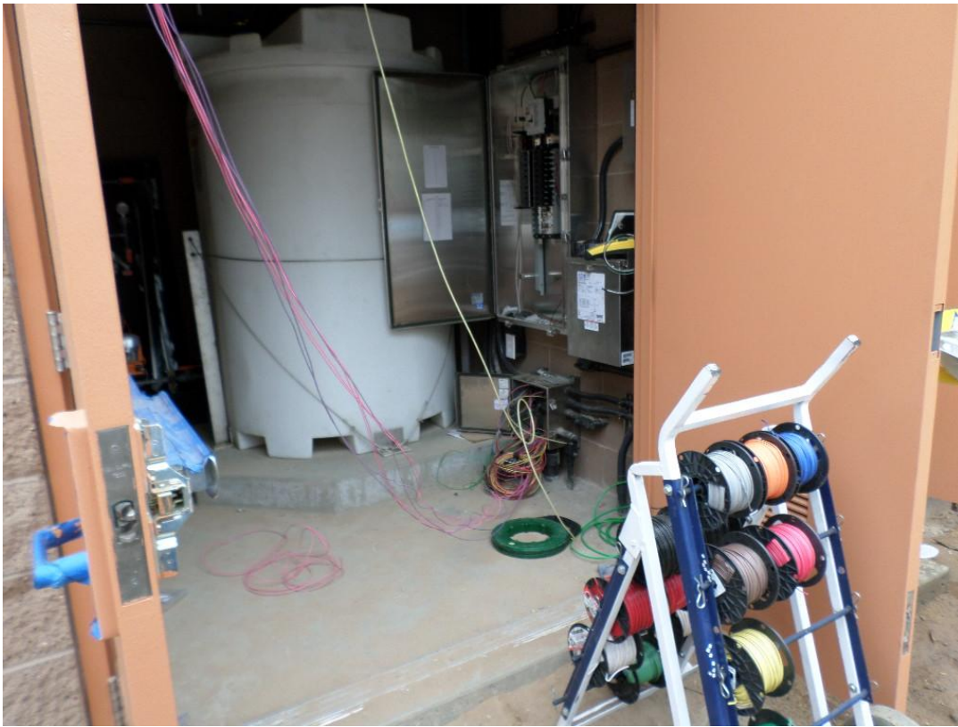
St. Denis Electric pulling wire.
