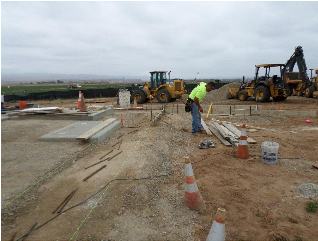
Spies forming three foot V-ditch.
