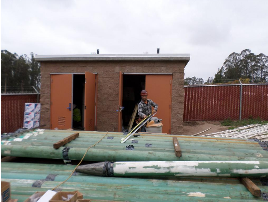
Martin Doors installing hardware on doors.
