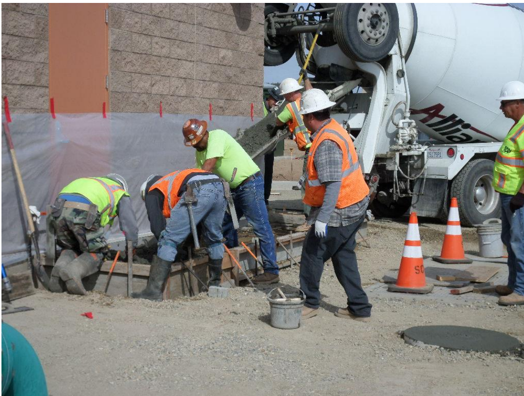
Spies pouring side walk to electrical room.
