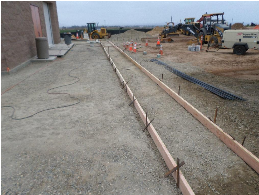
Three foot V-ditch formed.
