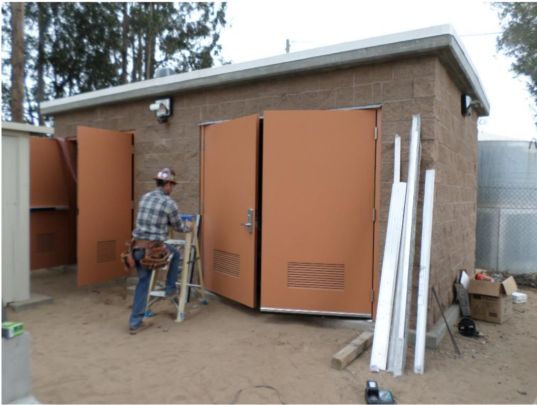
Installing door hardware.
