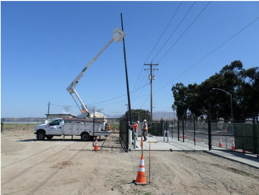
St. Denis Electric installing the SCADA tower.
