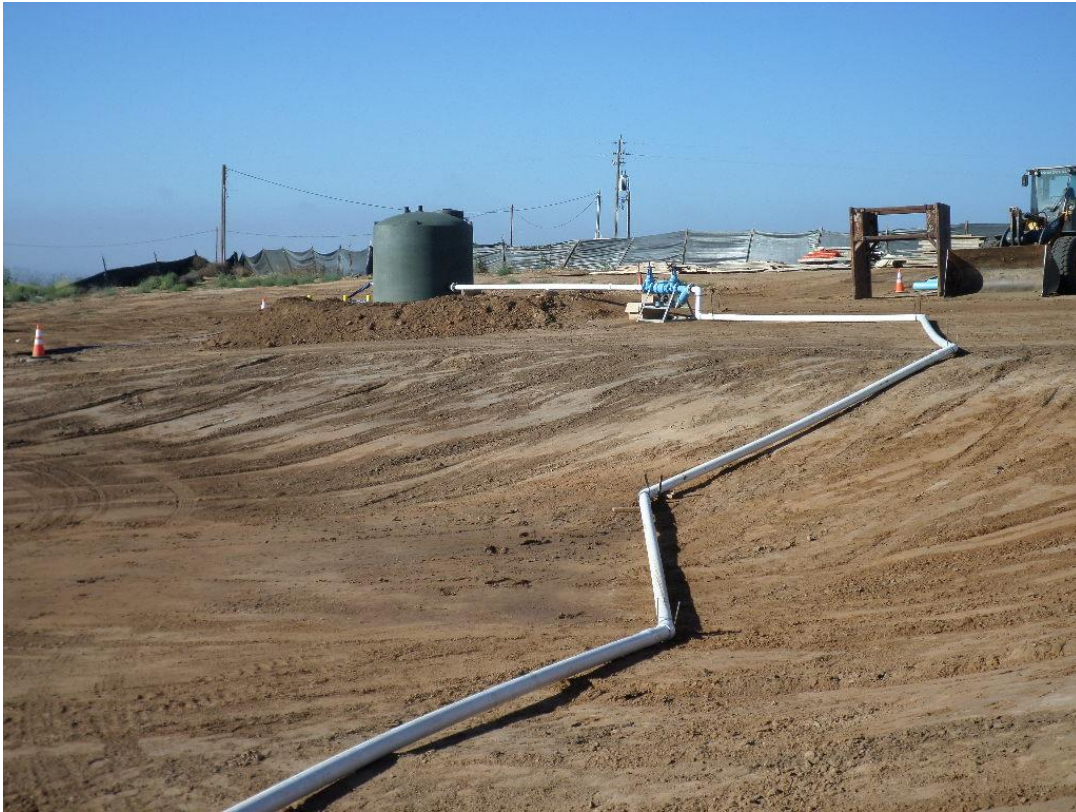
Temporary tank and piping installed in preparation for testing the pump station prior to taking water from the City of Santa Maria.
