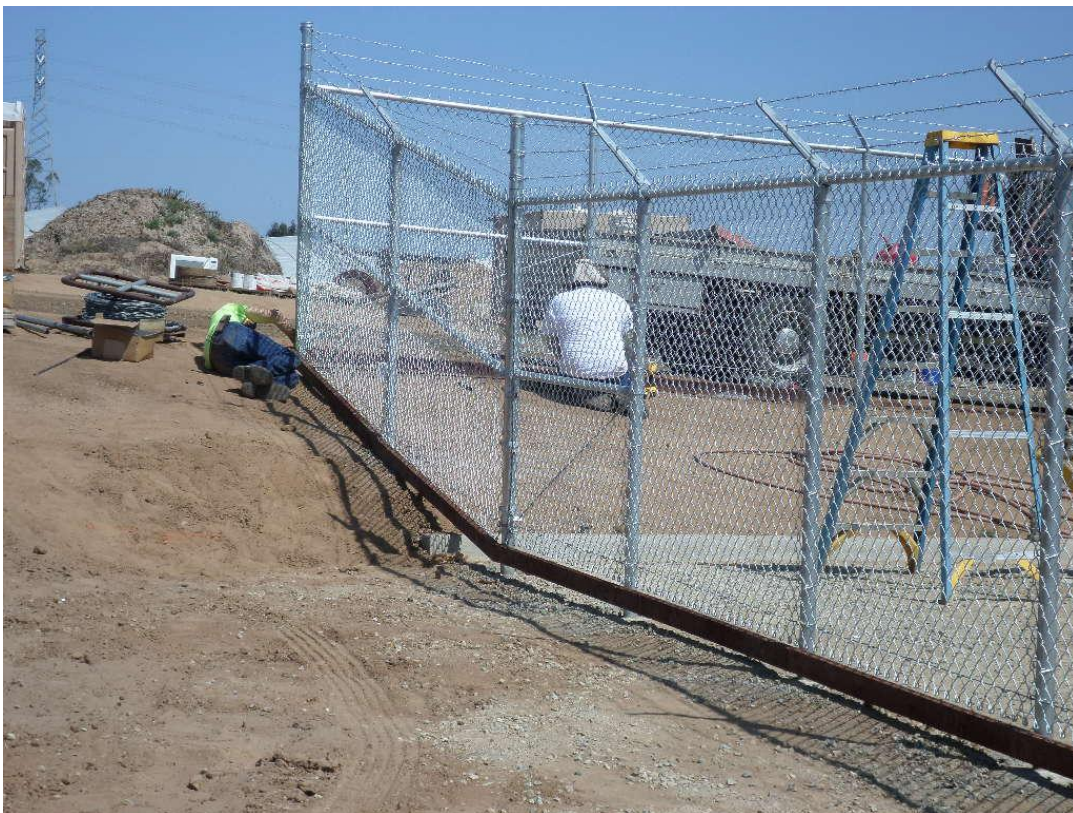
Central Coast Fencing completing fence installation.
