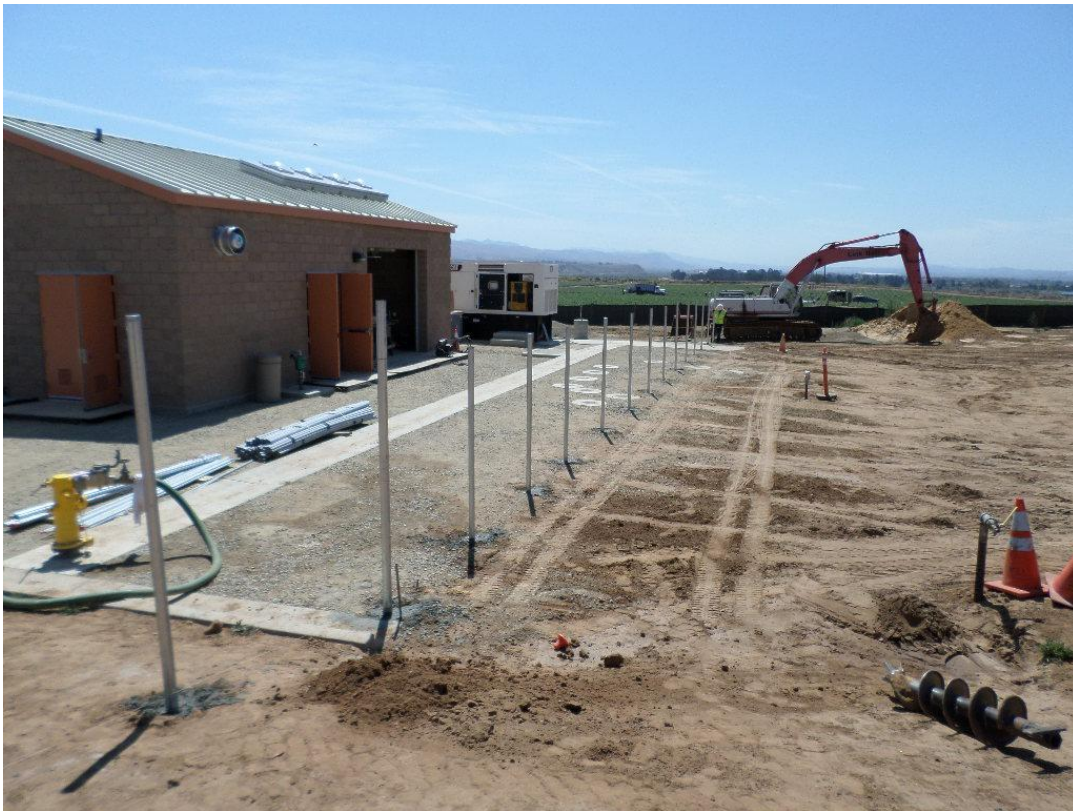
Central Coast Fencing setting fence posts.
