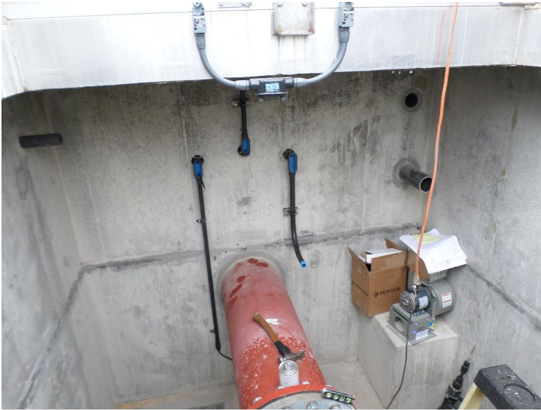
Installing electrical conduit in the vaults.
