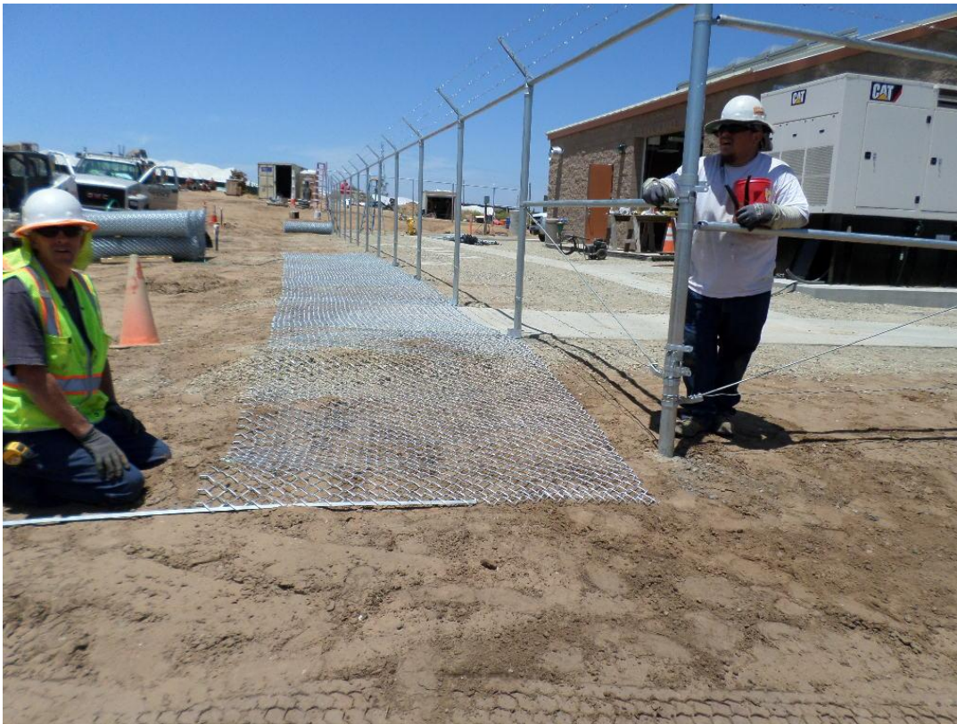
Central Coast Fencing installing fence fabric.
