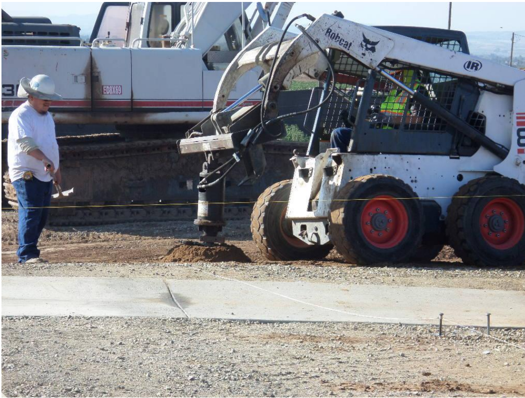
Central Coast Fencing augering fence post holes at the pump station site.
