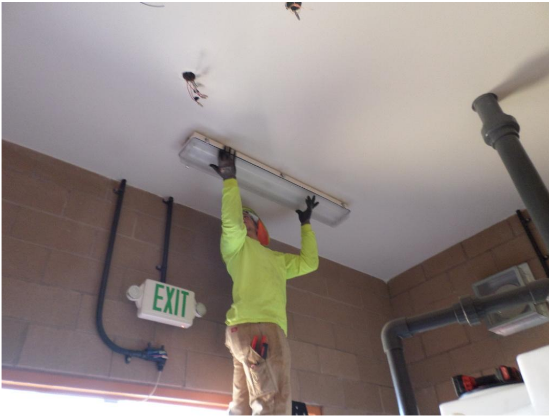
St. Denis Electric installing lights in pump room.
