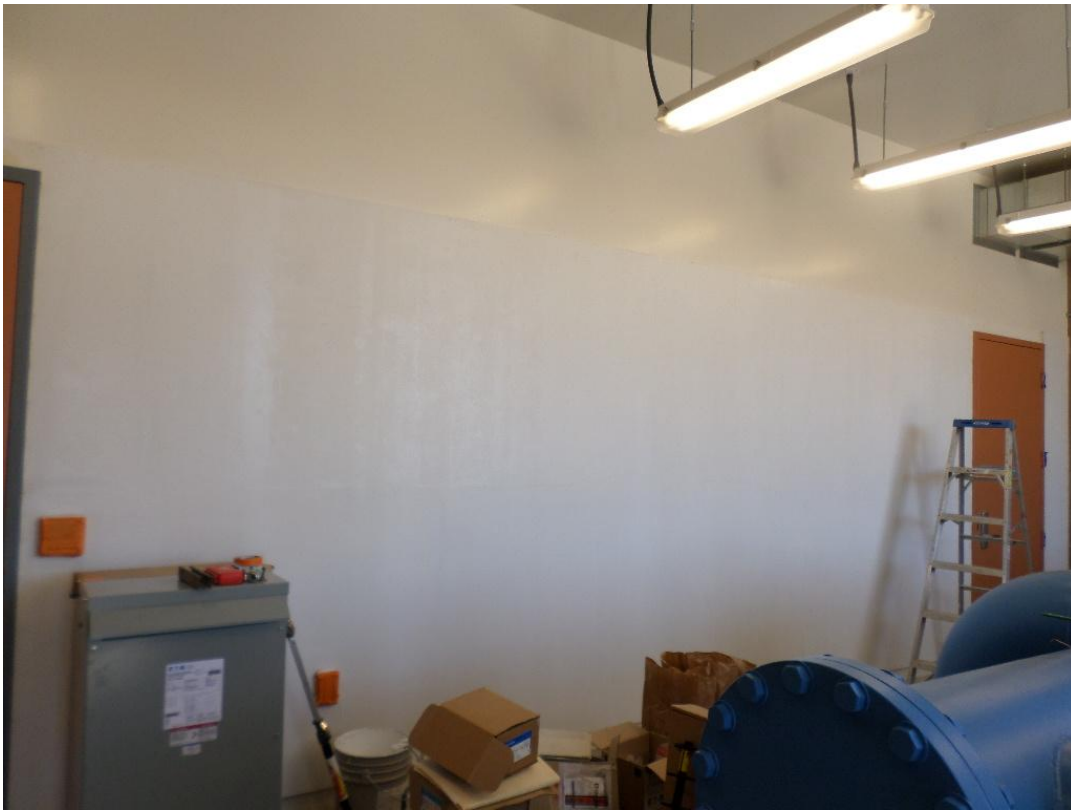
Painting plywood wall inside pump room.
