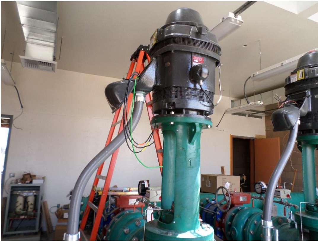
Pulling power wire to the vertical turbine pumps.
