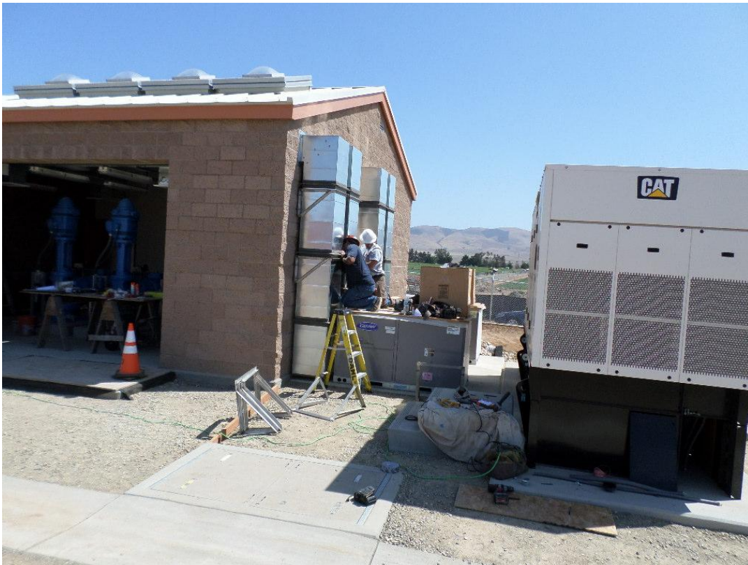
DAHL Air Conditioning installing AC duct supports.
