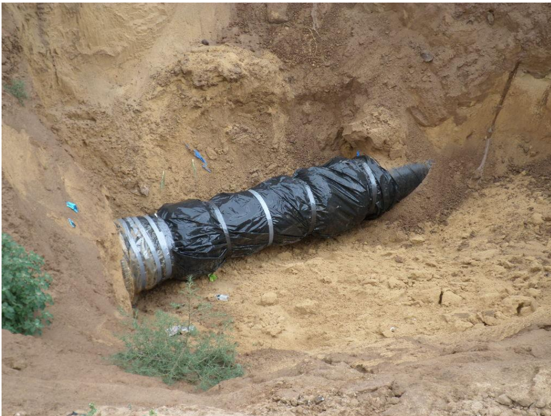
Connection wrapped in plastic and ready for backfill.
