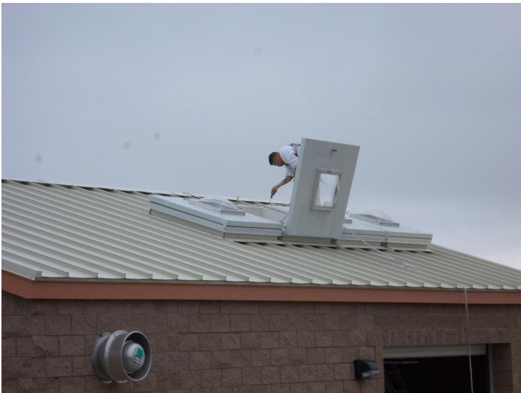
Coast Painting coating roof hatches.
