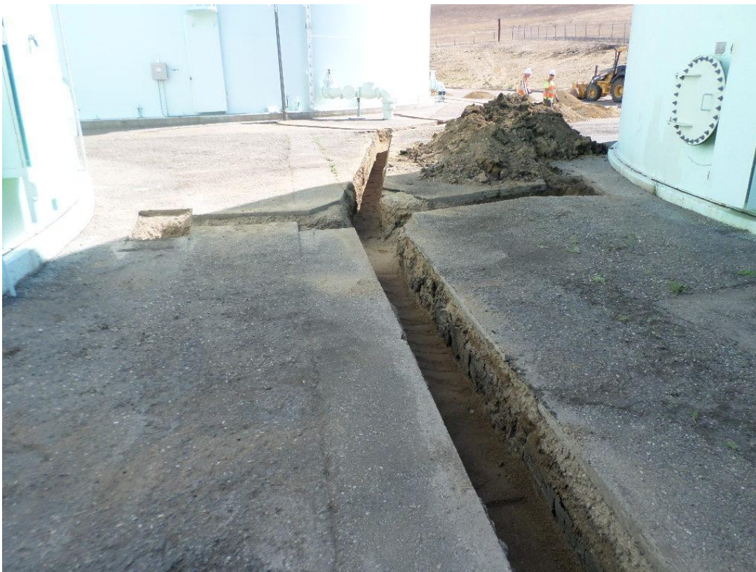
Spiess placing sand in trench at Quad Tanks.
