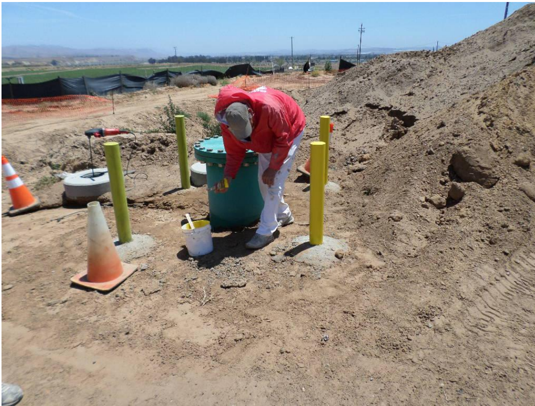
Coast Painting coating bollards.
