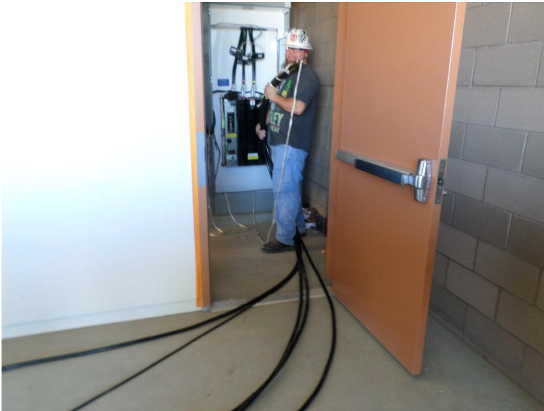
St. Denis Electric pulling wire at the ATS in the electrical room.
