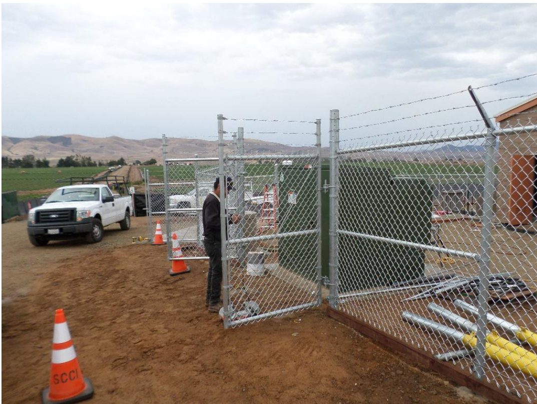
Central Coast Fencing installing access gate for PG&E at transformer.
