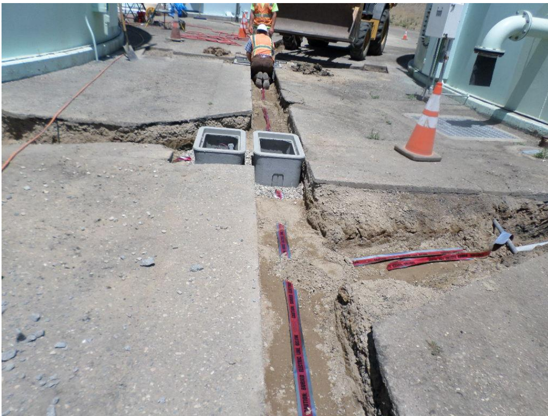
Pull boxes being installed at the Quad Tanks.
