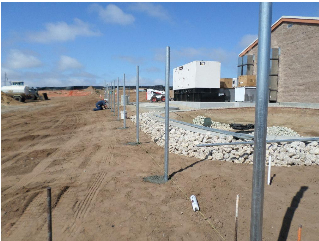
Setting fence posts.
