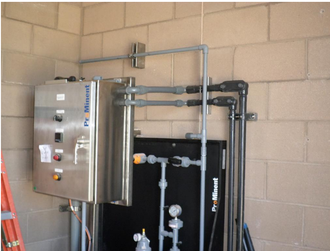
Spiess installing chemical feed pump piping.
