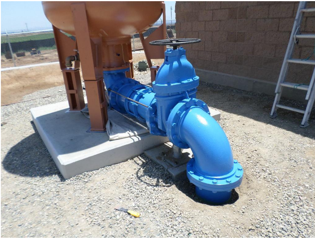
Coast Painting coating the piping and valve at the surge tank.
