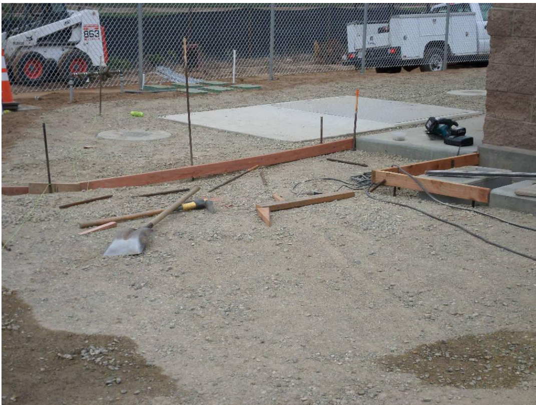
Spieß installing border for pavement for pump station driveway.
