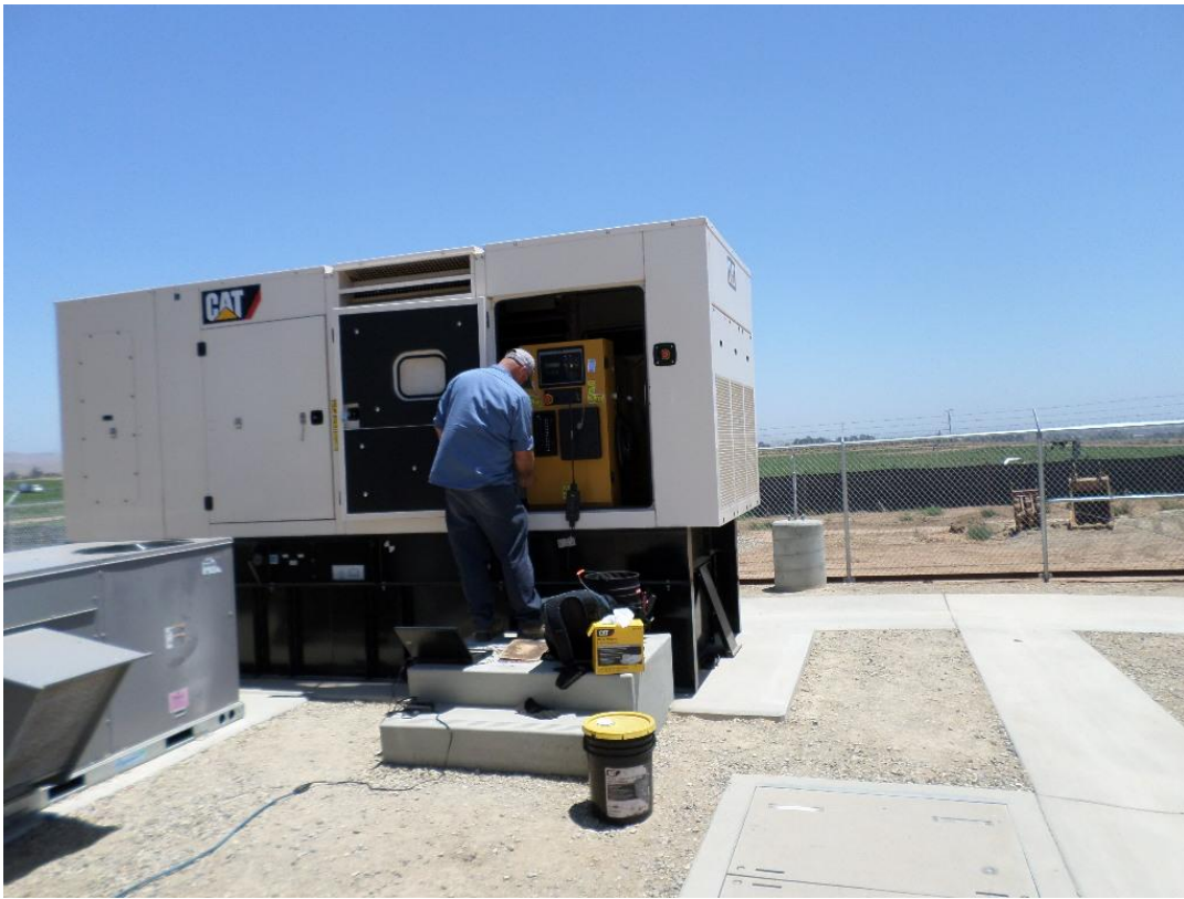
Setting up Emergency Generator at pump station.
