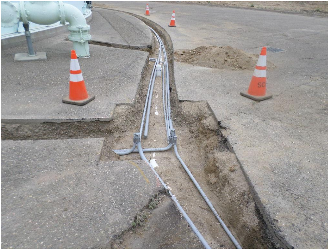
Conduit installation at the Quad Tanks.
