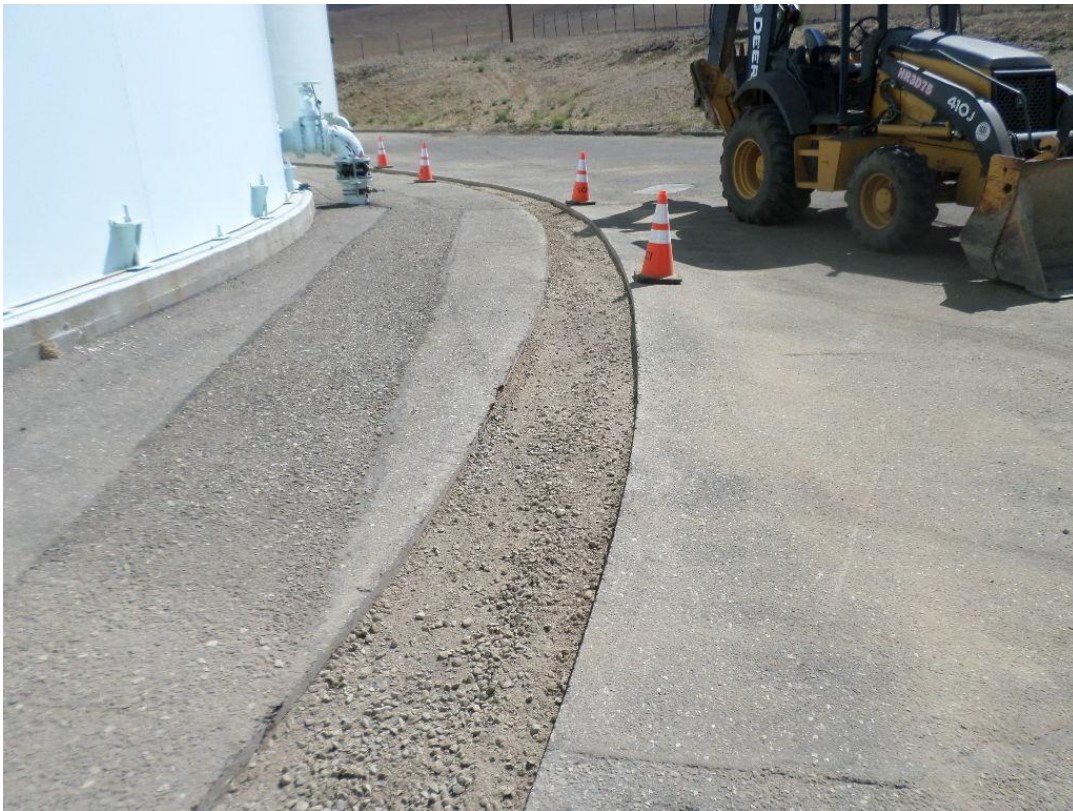
Spiess installing base in trench in preparation for paving.
