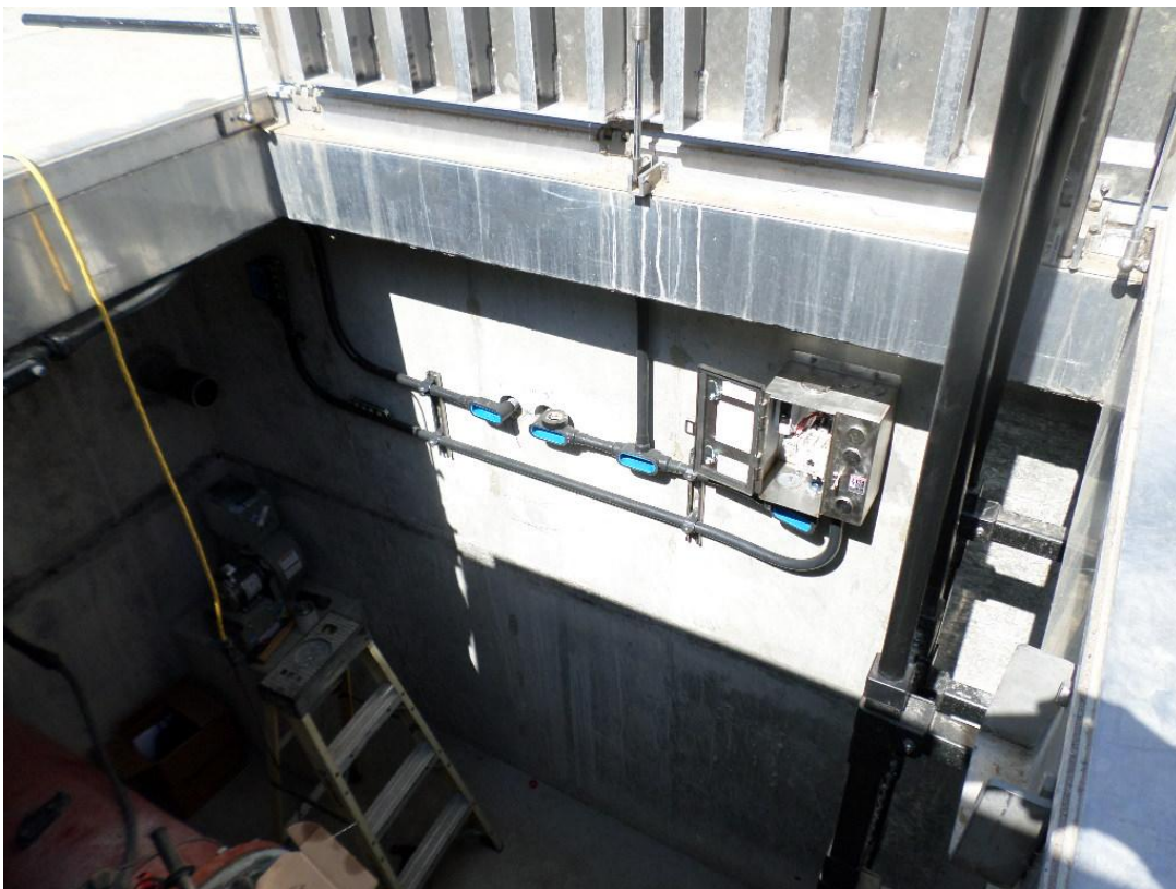
Installing electrical conduit in the vaults.
