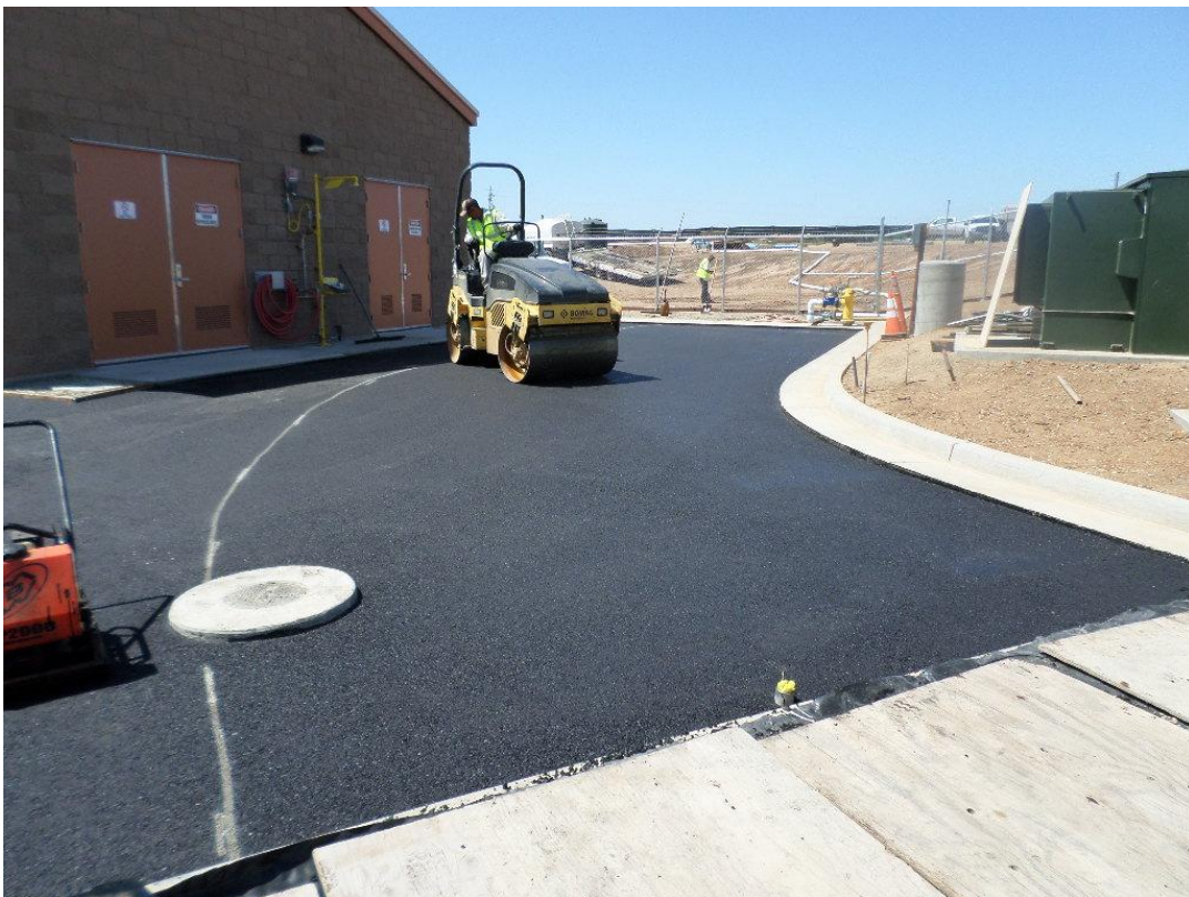
Toste Grading and Paving rolling first lift of asphalt for pump station driveway.
