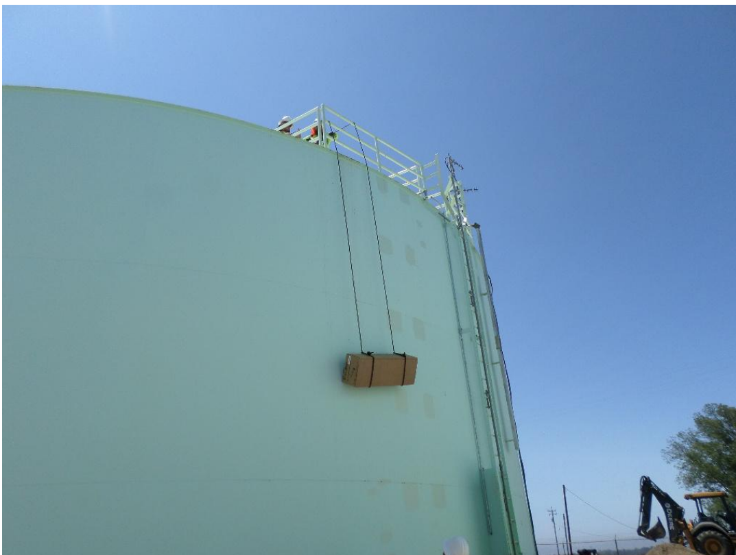
Spiess staging materials for mixer installation at the Quad Tanks.
