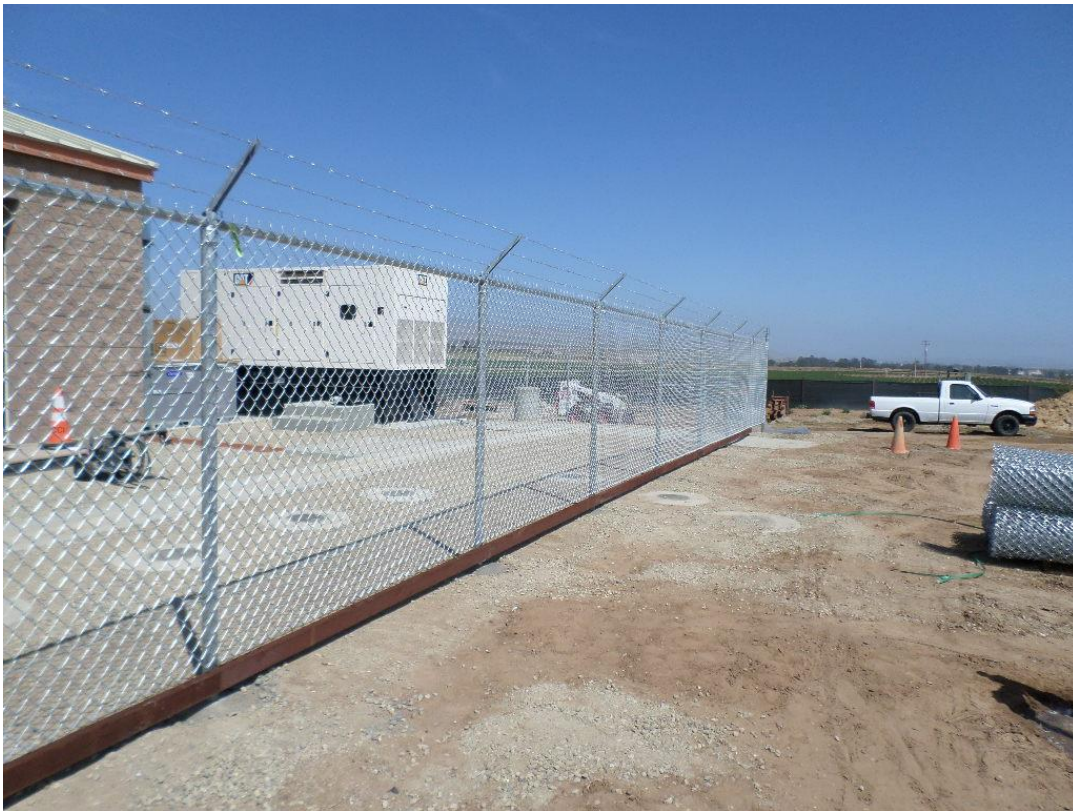
Fence installed at the pump station.
