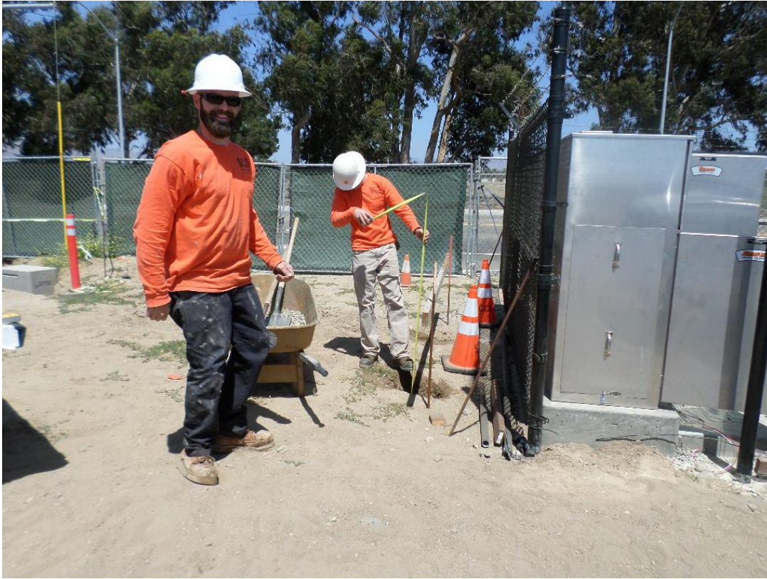
Spiess installing bollards.
