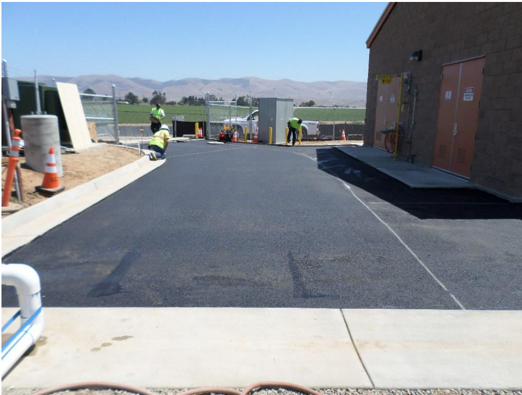
Toste Grading and Paving laying out drainage swale for pump station driveway.
