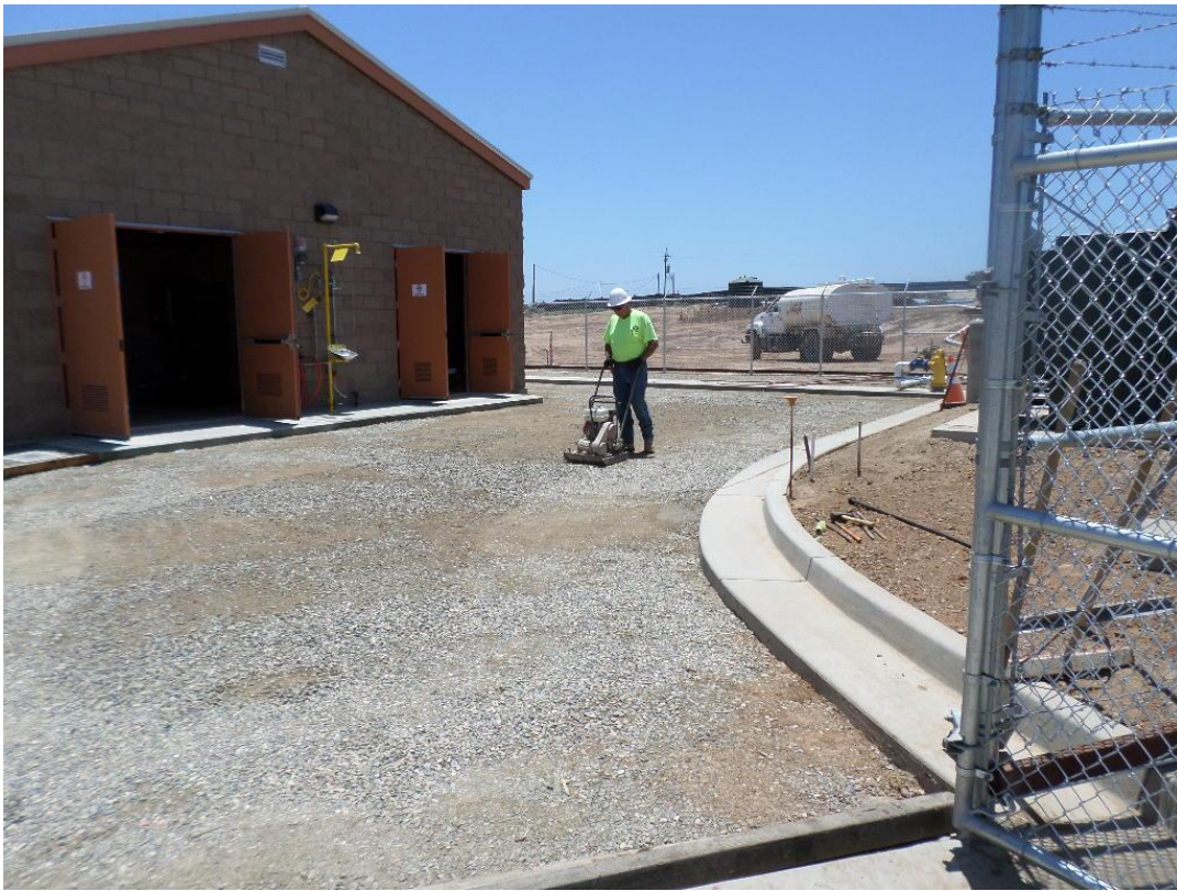
Spieß compacting base in preparation for driveway paving.
