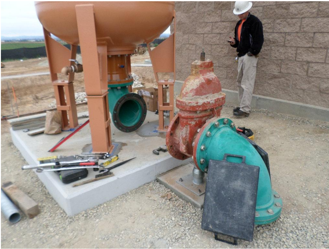
Spiess installing the valve at the surge tank.
