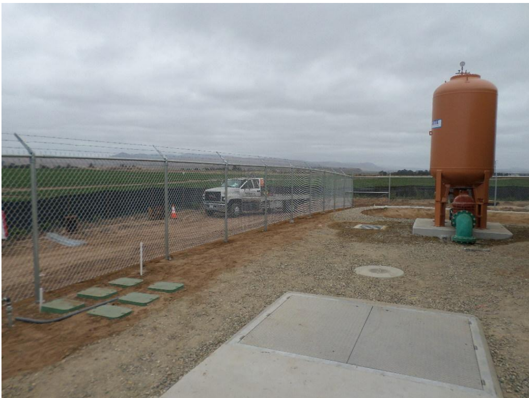
Central Coast Fencing completing fencing installation.
