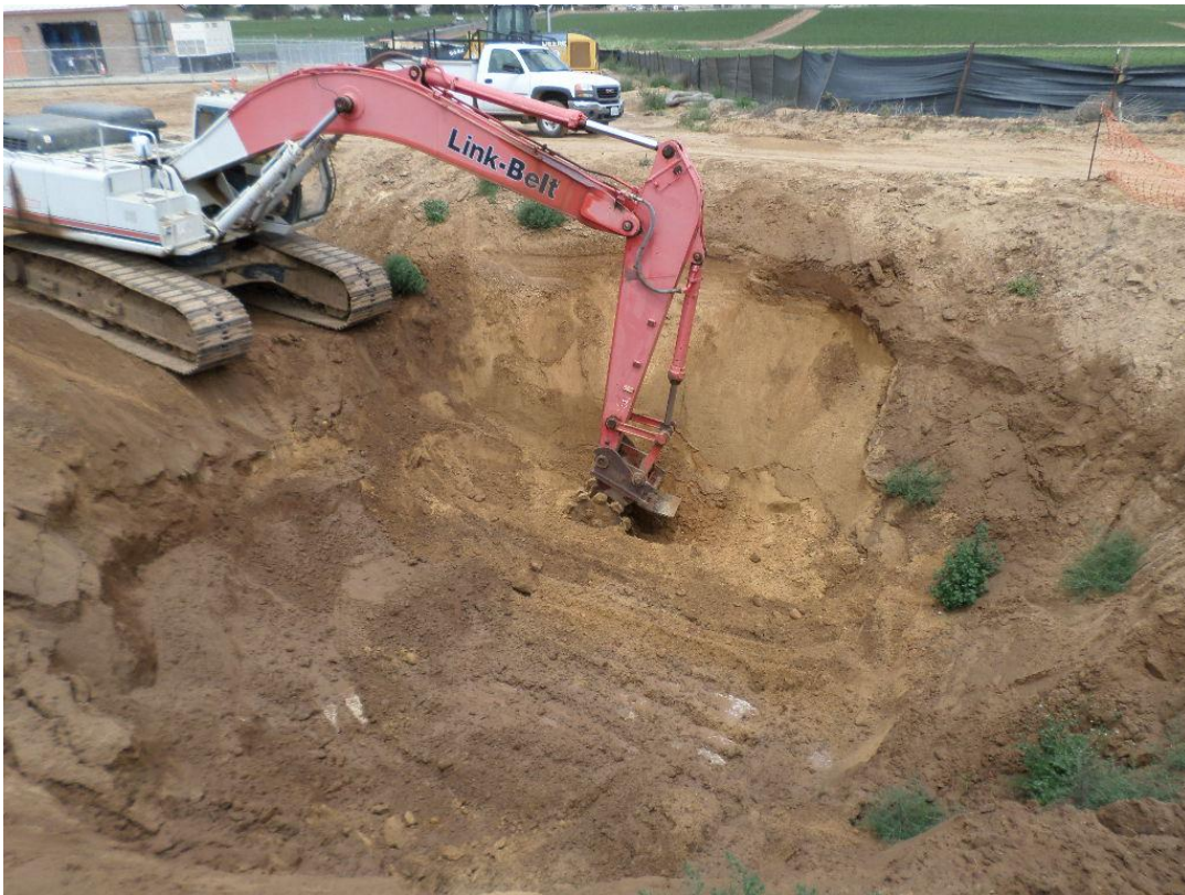
Spiess backfilling pipe connection.
