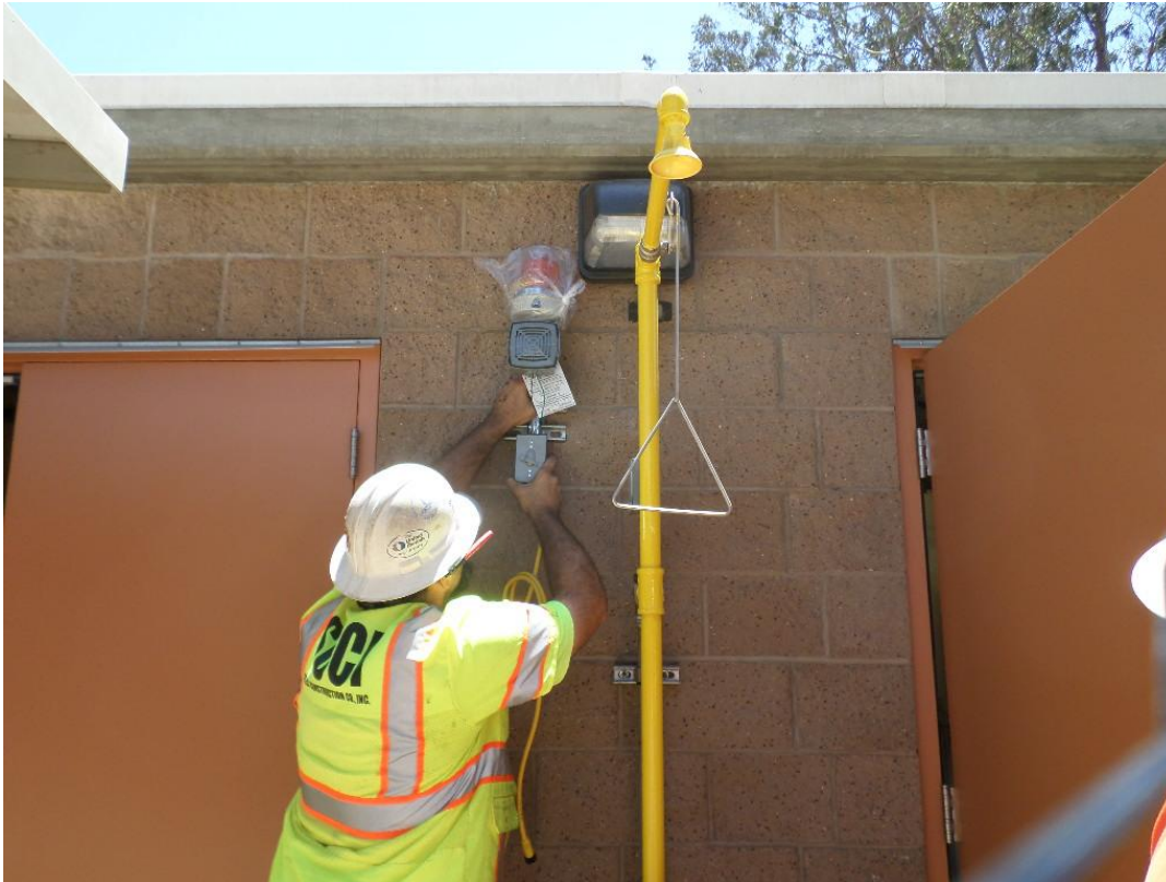
Spiess installing the emergency eye wash station.
