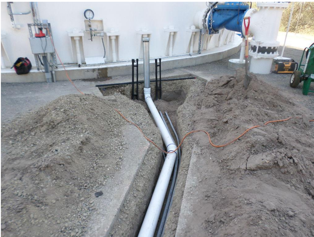
Drain line and conduit being installed at the Standpipe Tank.
