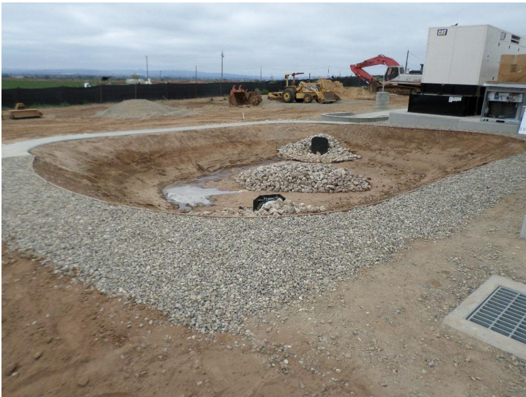
Spiess spreading \frac{3}{4} -inch rock around the retention basin.
