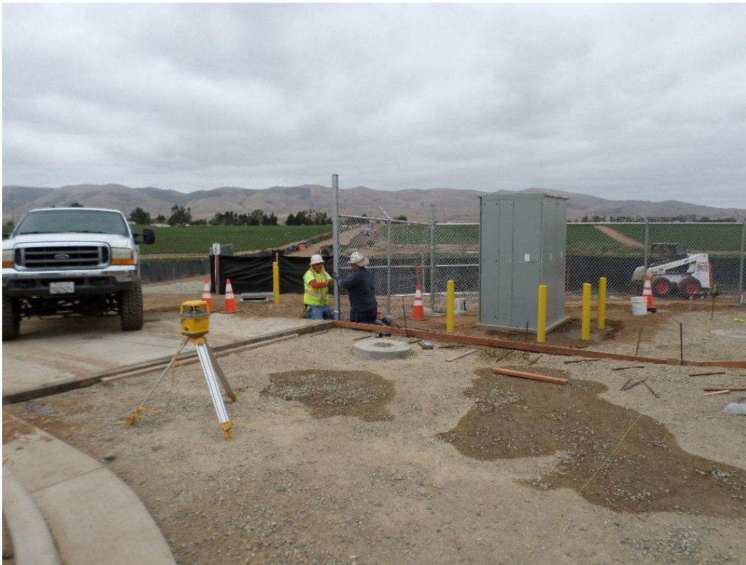
Central Coast Fencing completing fence installation.
