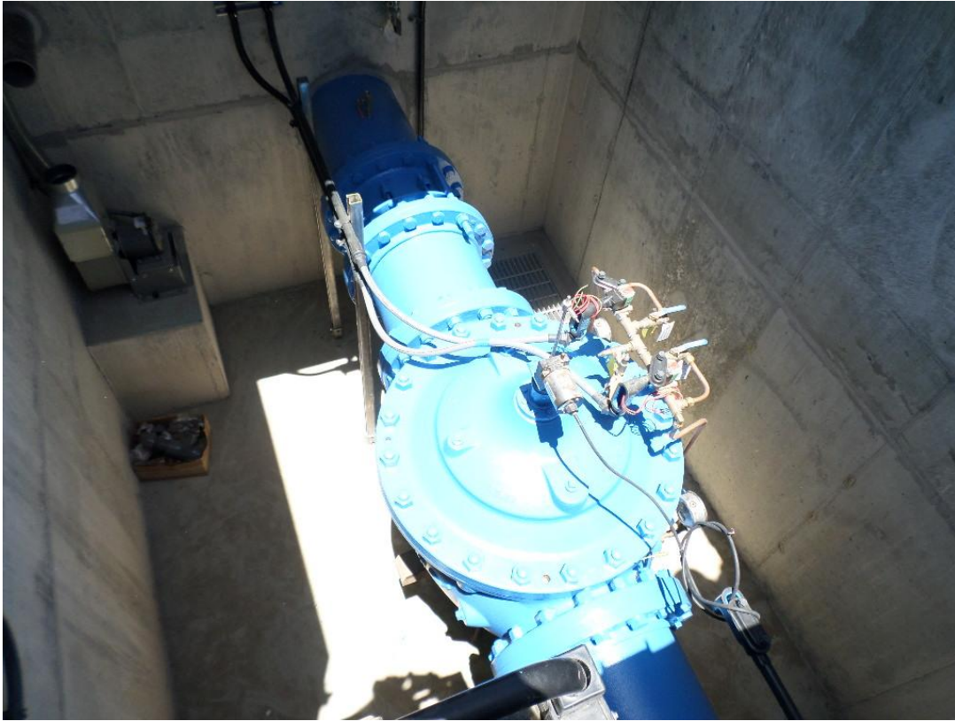
Coast Painting coating the pipes and appurtenances inside the vaults.
