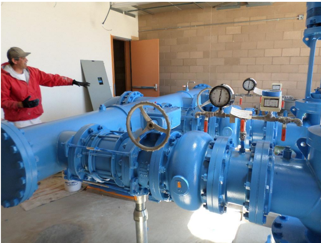
Coast Painting coating discharge piping inside the pump station.
