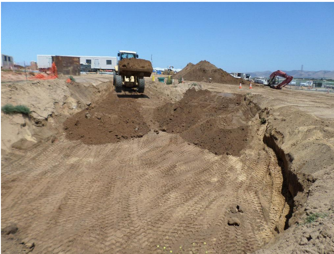
Spiess backfilling connection of pump station to HDPE pipe.
