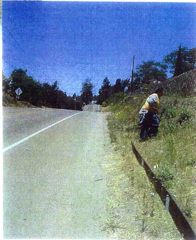
Photo 8: Orchard Avenue looking North along Pipeline Route
