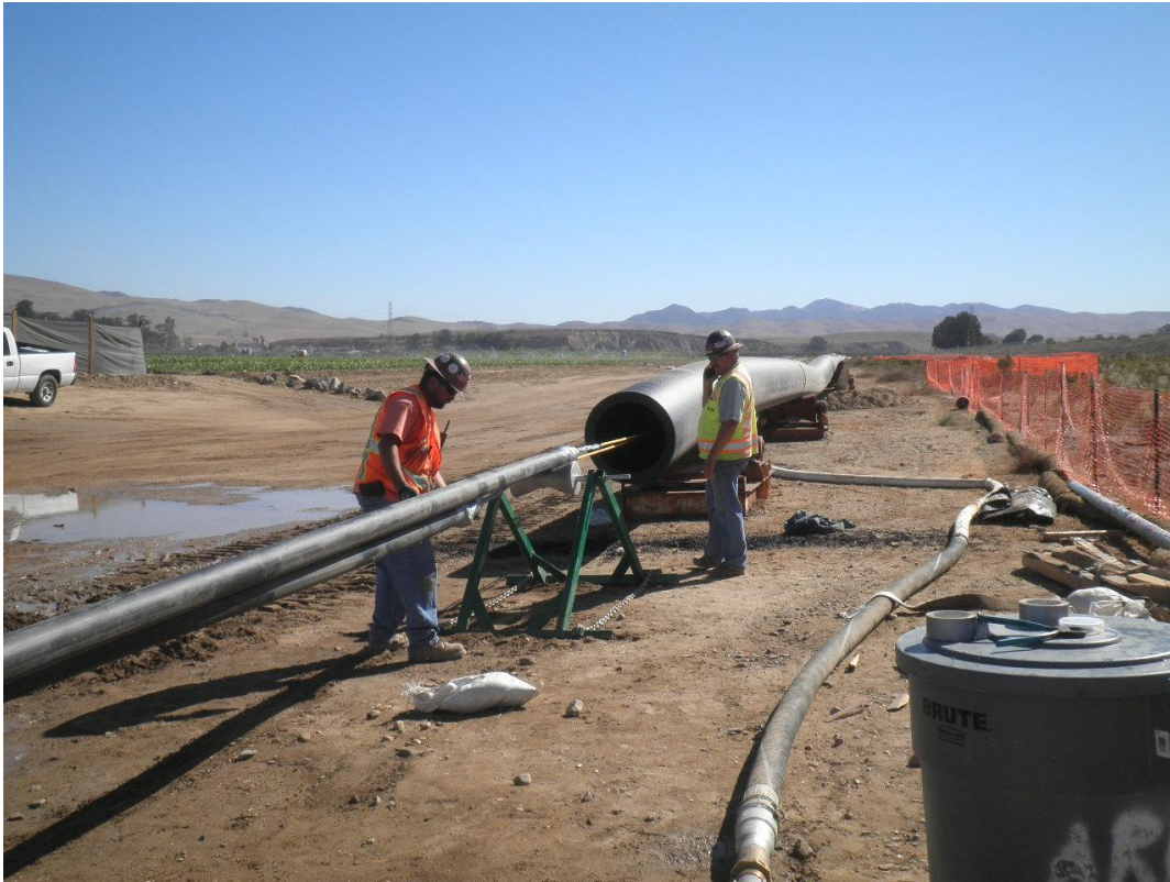
ARB positioning the two 4-inch pipes for pulling into the HDPE pipe.
