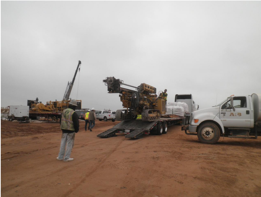
GeoGrout mobilizing one of their drill rigs to the north site on October 23.
