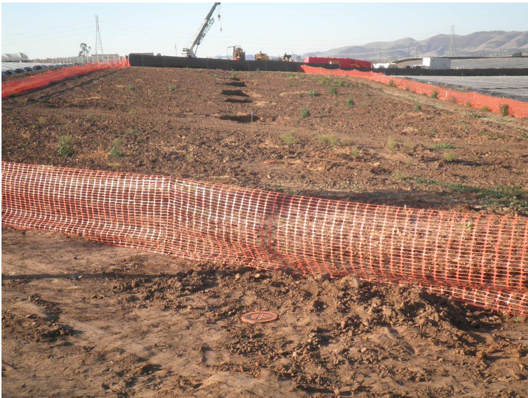
Settlement monitors installed by ARB to monitor further settlement closer to the edge of the bluff.
