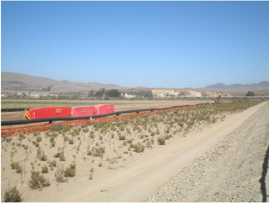
Water tanks (20,000 gallon) mobilized for hydrostatic pressure test of HDPE pipe.
