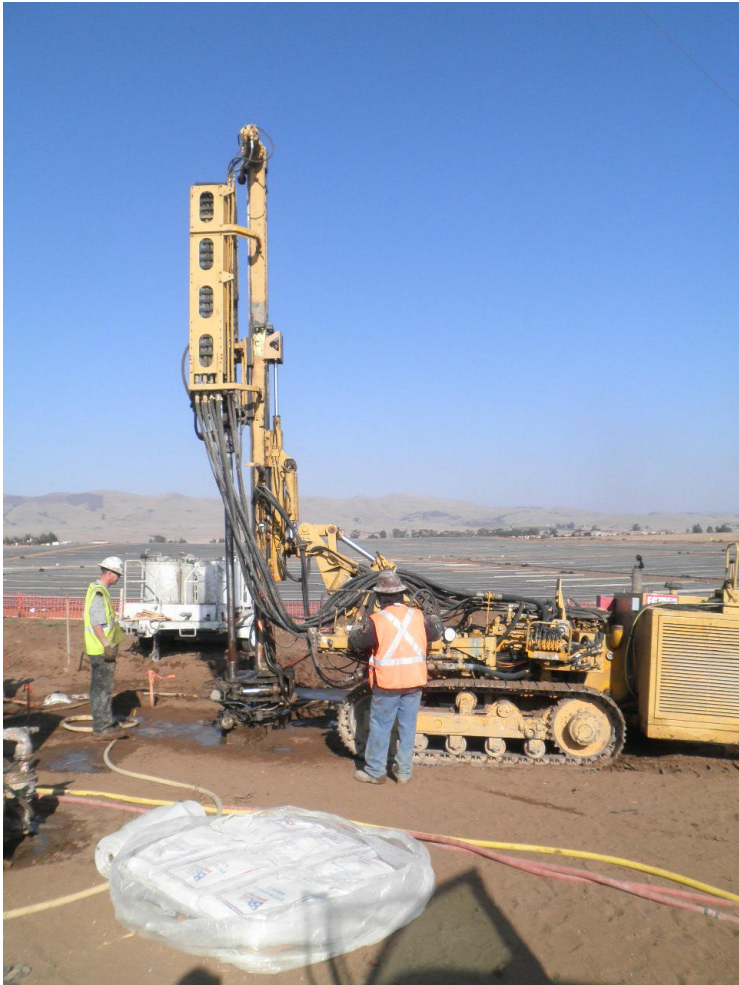
GeoGrout continuing permeation grouting injections.
