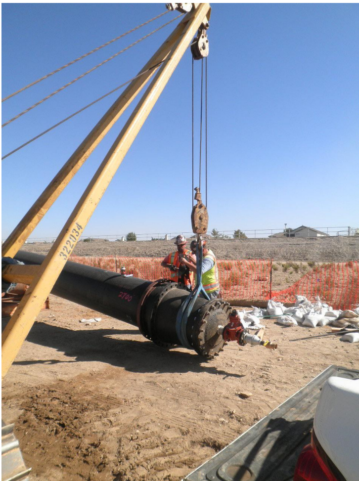
ARB installing welded flanged adapter and DIP reducer with pressure test fitting to the west end of the HDPE pipe.
