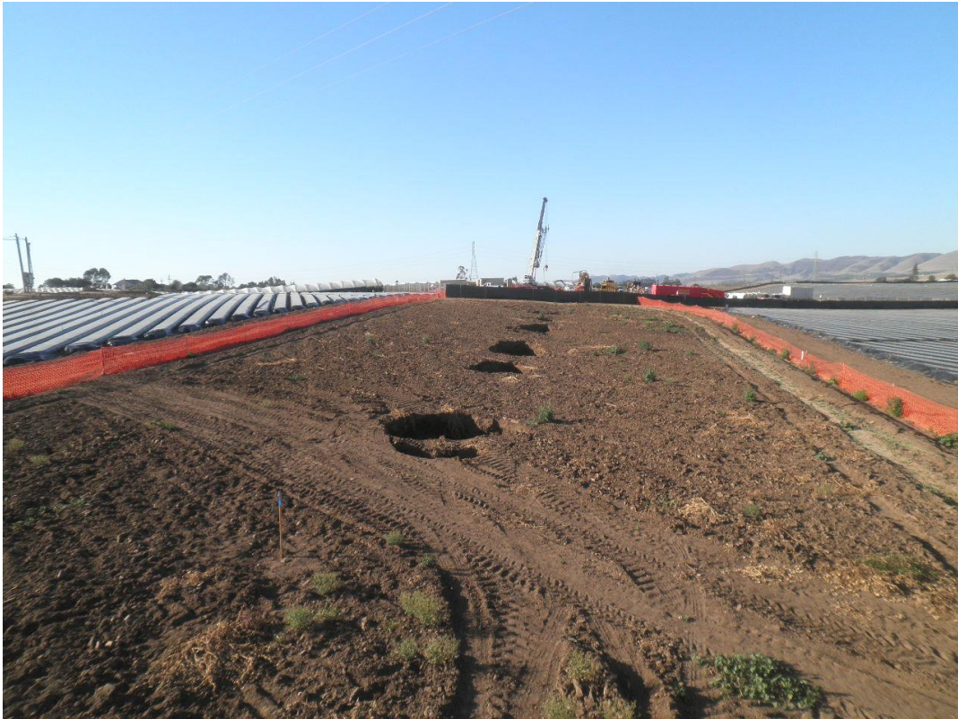
Sink holes when initially discovered on October 14.
