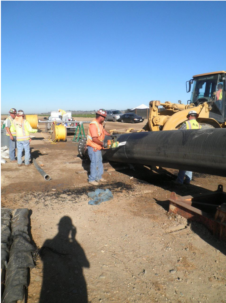
Removing flanged adapter and DIP reducer from west end of pipe after hydrostatic pressure test.
