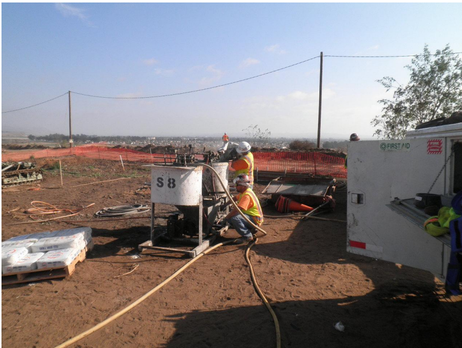
ARB personnel assigned to work with GeoGrout mixing cement grout.
