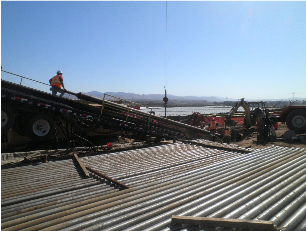
ARB inserting 12-inch casing into hole to help free 36-inch drill.
