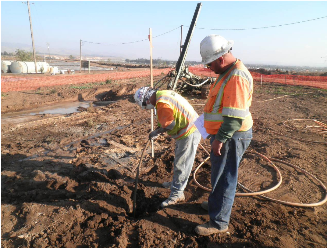
GeoGrout backfilling drill hole with cement grout.
