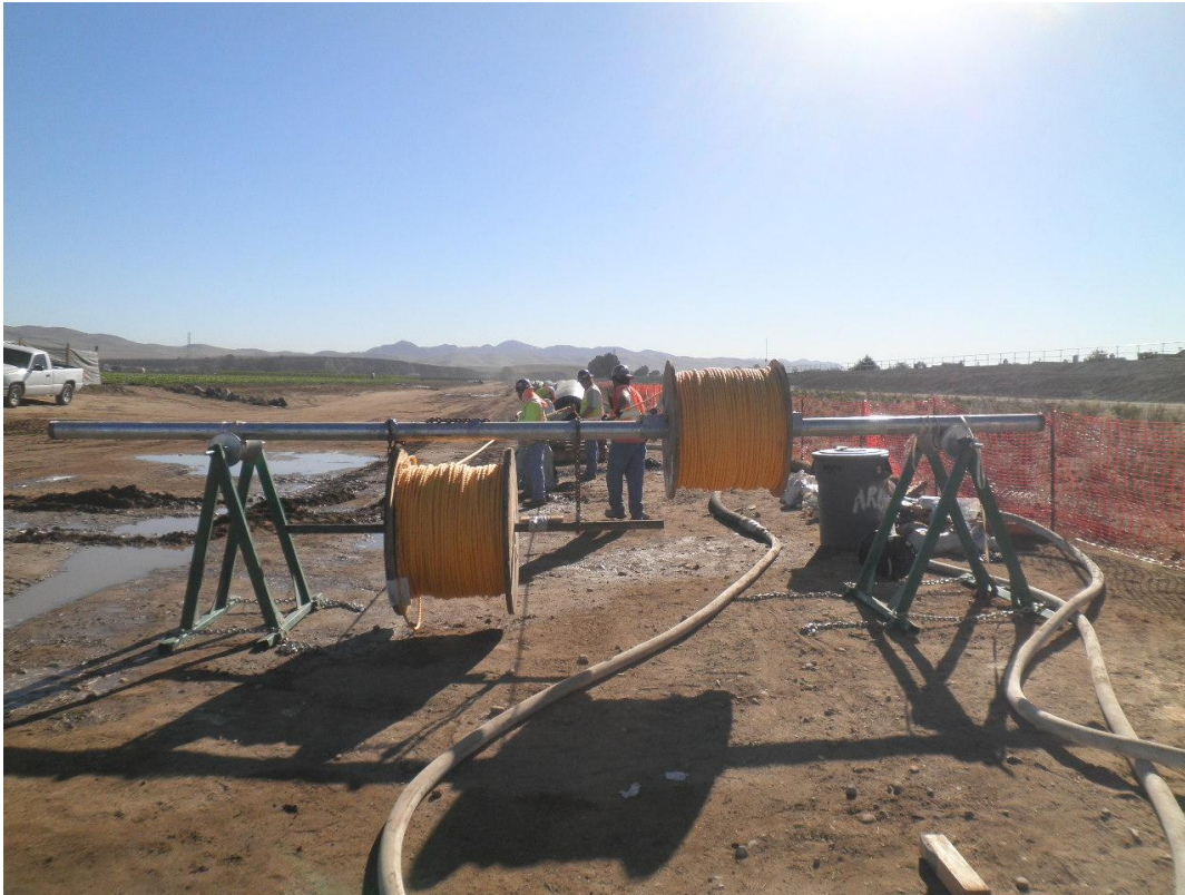
ARB feeding rope into HDPE pipe from west end.
