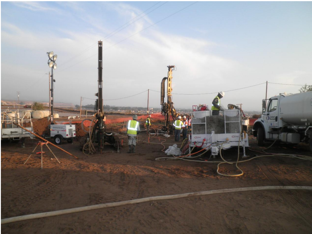
Two GeoGrout drills completing first permeation grout injections.
