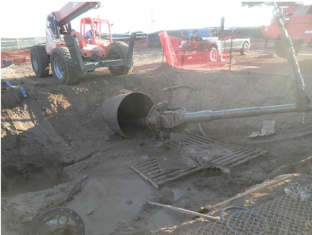
ARB removing 36-inch drill after it became stuck due to material settlement during the second reaming pass on October 16.
