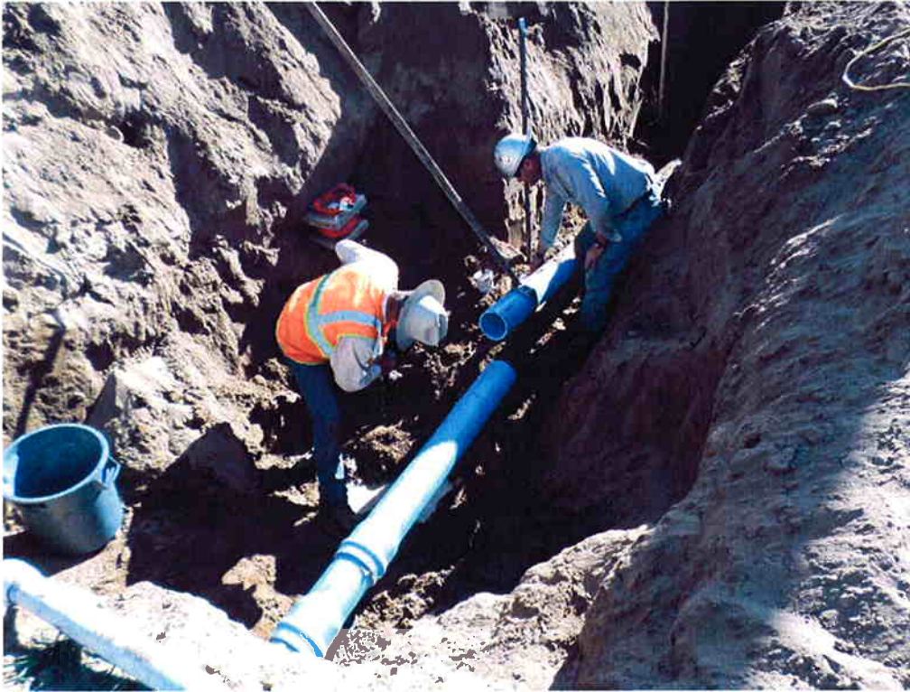
Cushman tying in the 6-inch water line.
