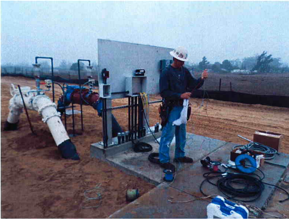
Bergelectric terminating wires at control panel.
