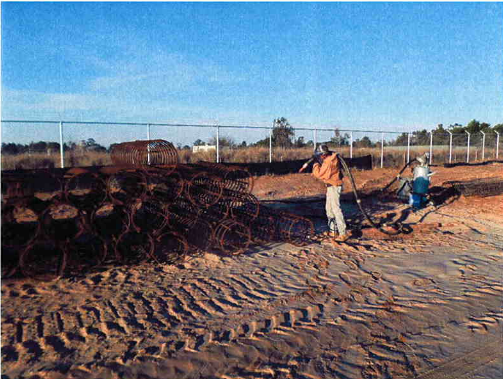
Cushman sandblasting rebar for street light bases.
