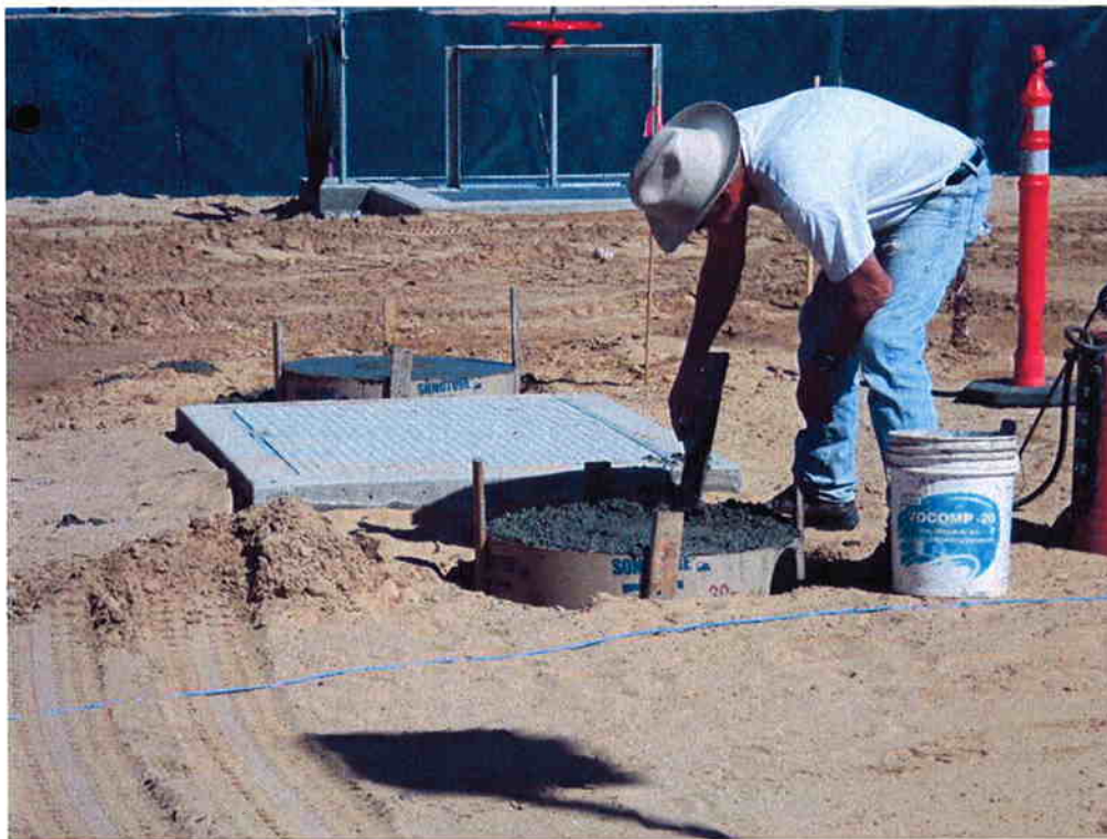
Cushman pouring collars at valve cans.
