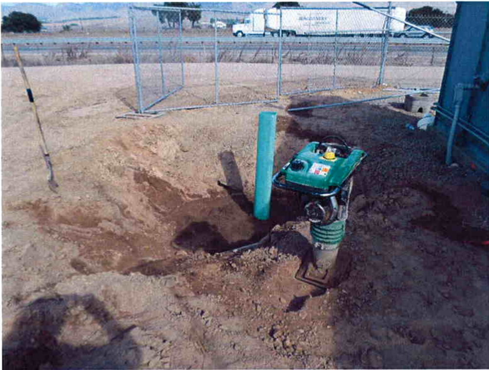
Cushman compacting 6-inch valve can.
