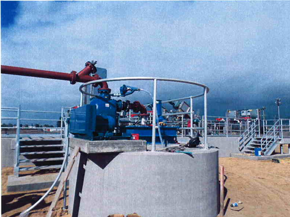
Cushman completing handrail installation at the headworks.
