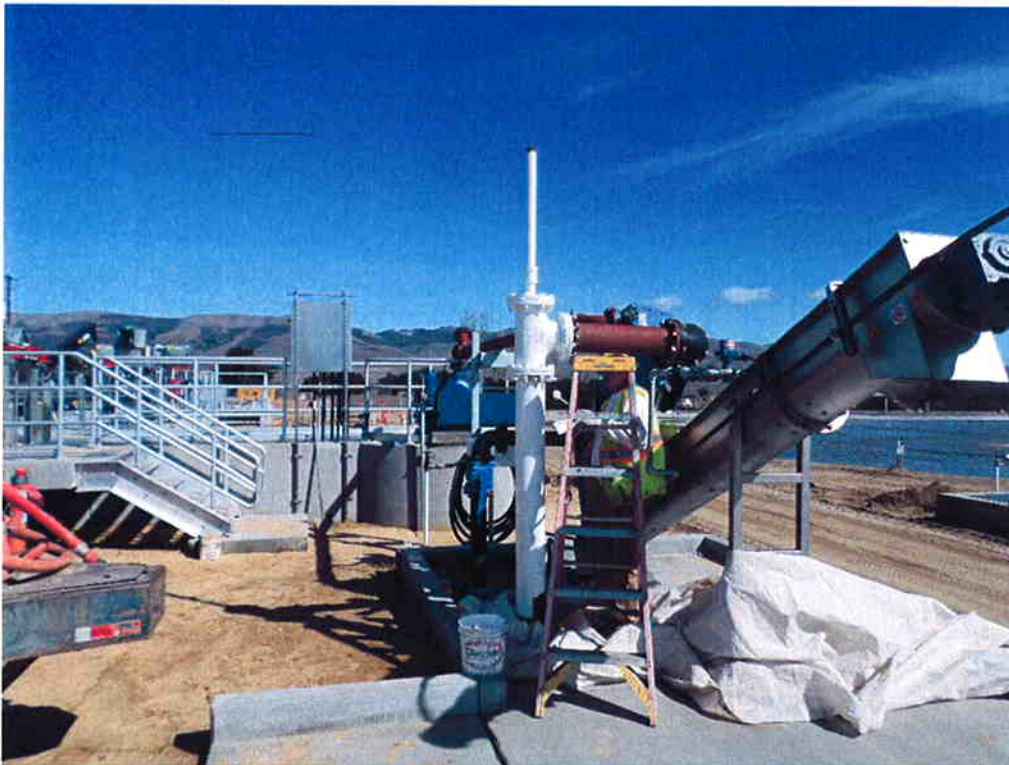
KNK Coating applying prime coat to grit piping.
