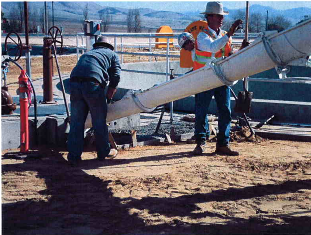
Cushman pouring concrete for hose bib pads.
