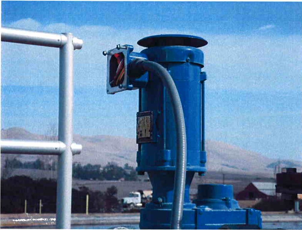
Bergelectric terminating wires to grit motor.
