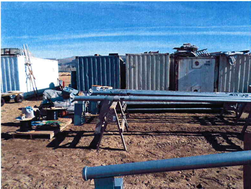
Cushman assembling street light poles.
