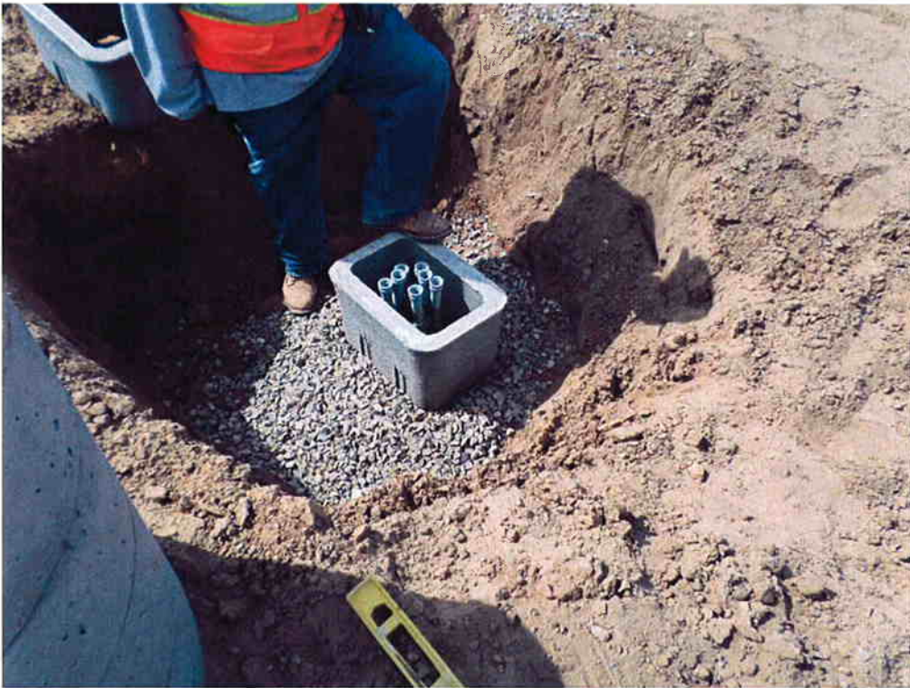
Bergelectric installing street light pull boxes.
