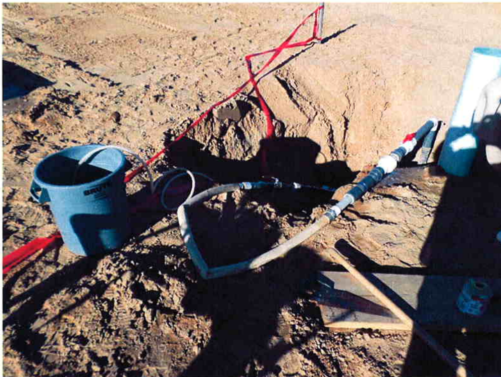
Cushman disinfecting the 2-inch potable water line.
