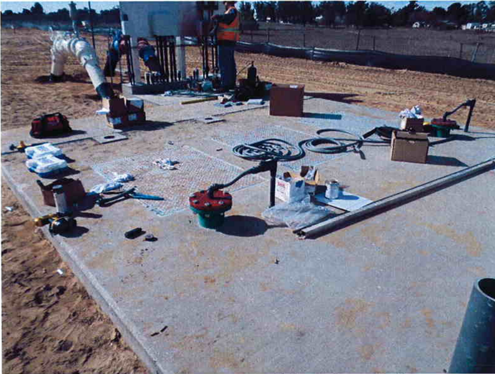
Bergelectric installing level sensors at the Influent Pump Station.
