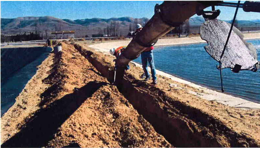
Cushman pouring red slurry over conduit for street lights.
