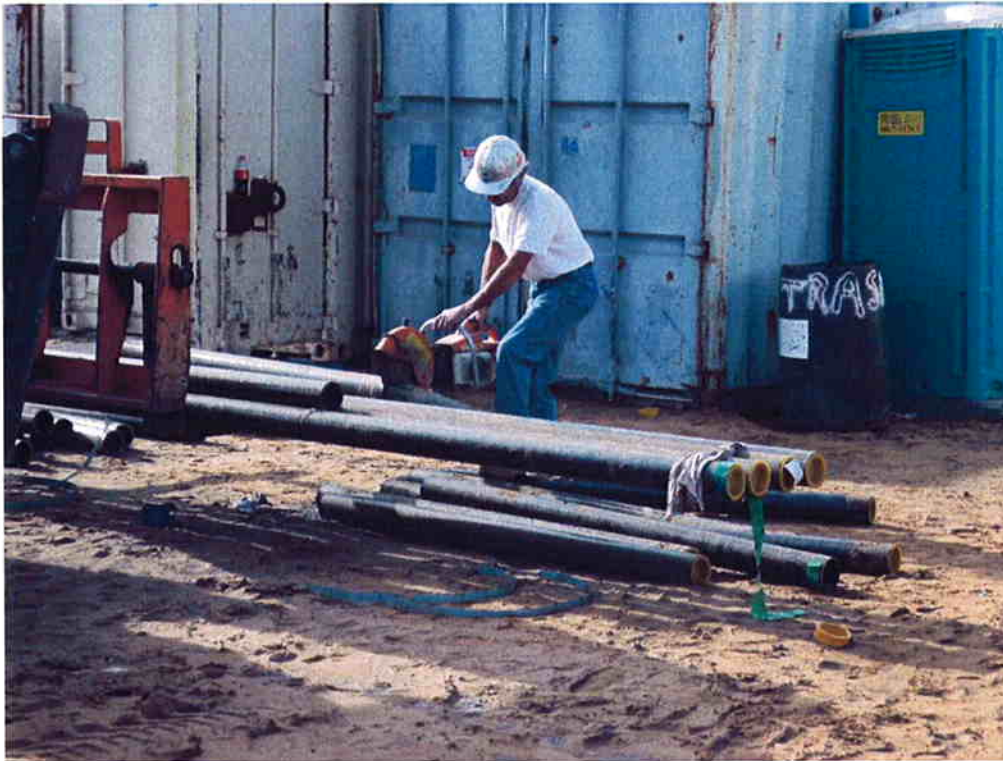
Cushman cutting pipe into bollards.
