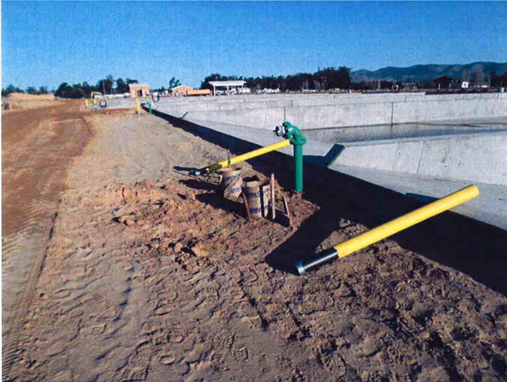
Cushman installing bollards at the drain pipes.
