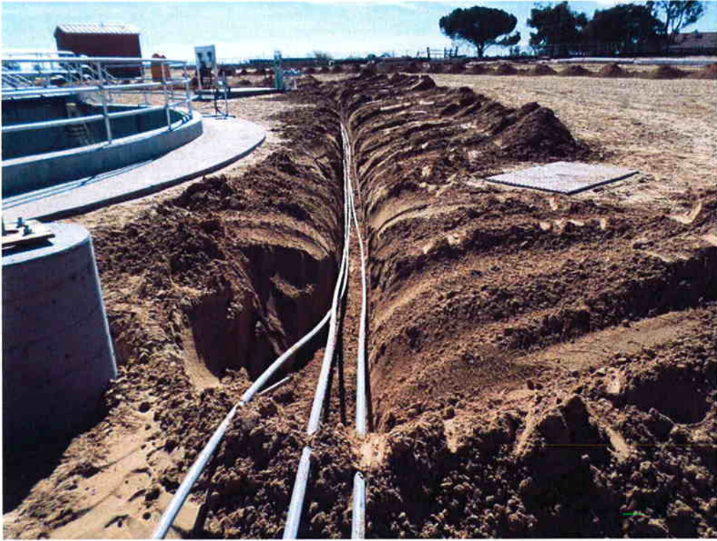
Bergelectric installing street light conduit.
