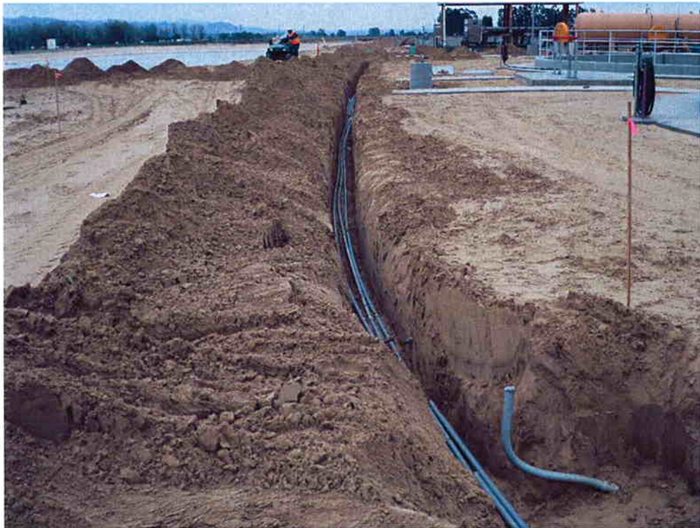
Bergelectric installing street light conduit.
