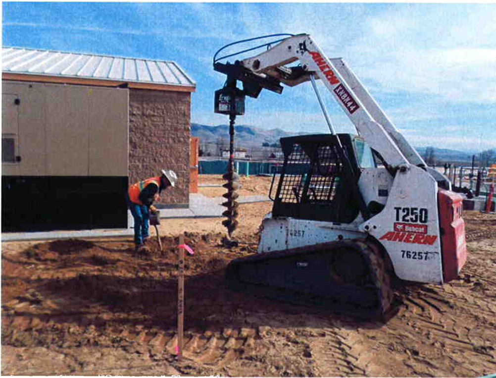
Cushman boring holes for bollard installation.
