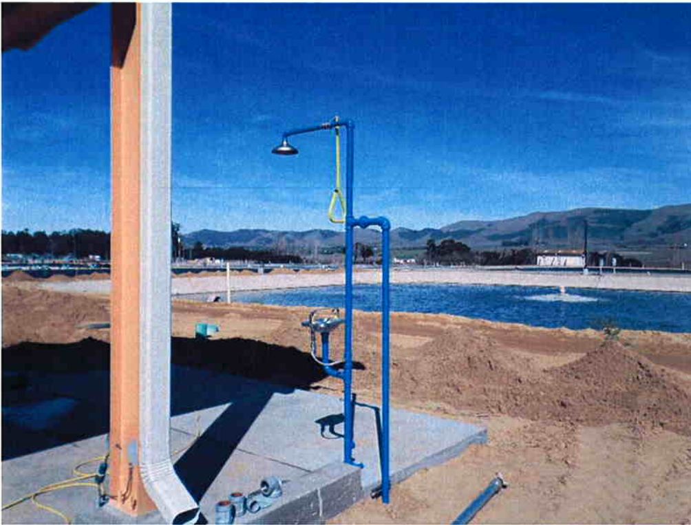
Eye wash station installed at the Sludge Thickening Structure.
