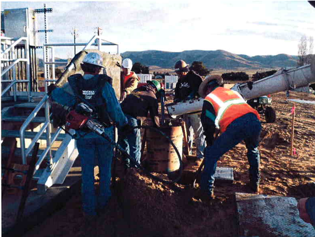
Cushman placing concrete at street light bases.
