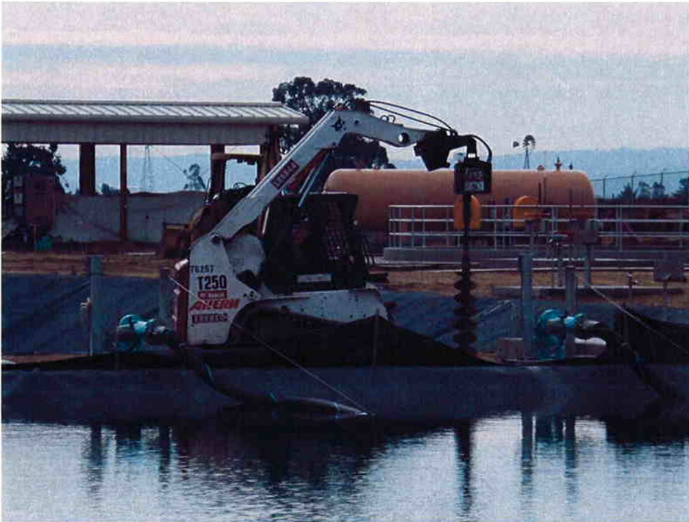
Cushman boring holes for street light bases between Aeration Basin #1 and the Emergency Basin.
