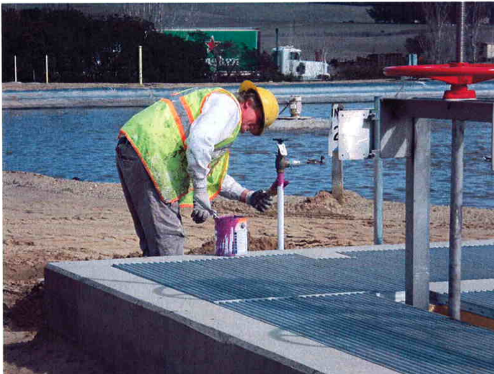
KNK Coatings painting non potable water piping.
