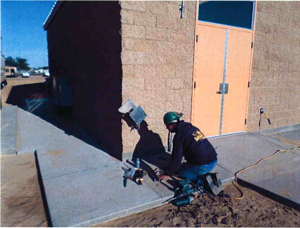
Cushman installing hose racks.
