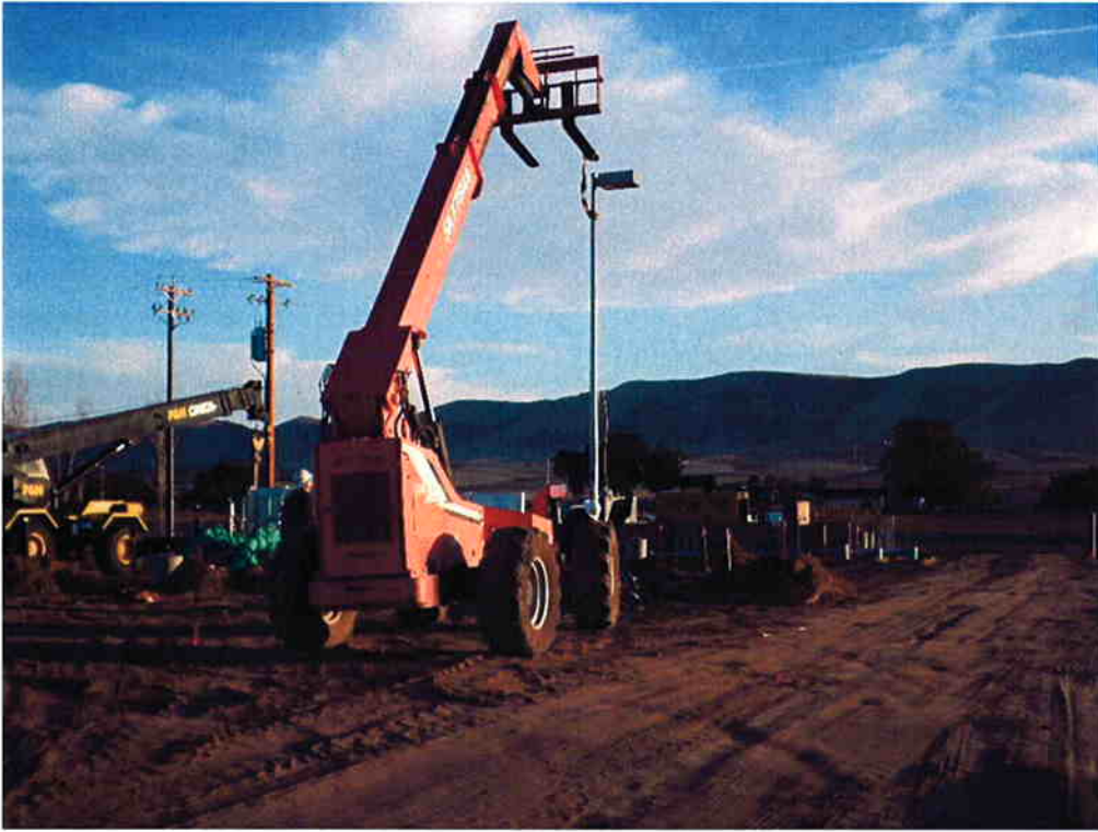
Cushman installing light posts on for street lights.
