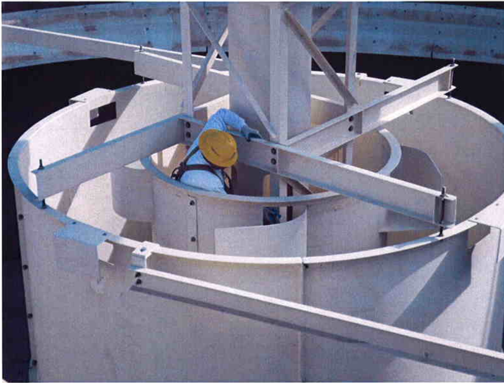
KNK Coating recoating where corrosion was removed on Clarifier #2 mechanism.
