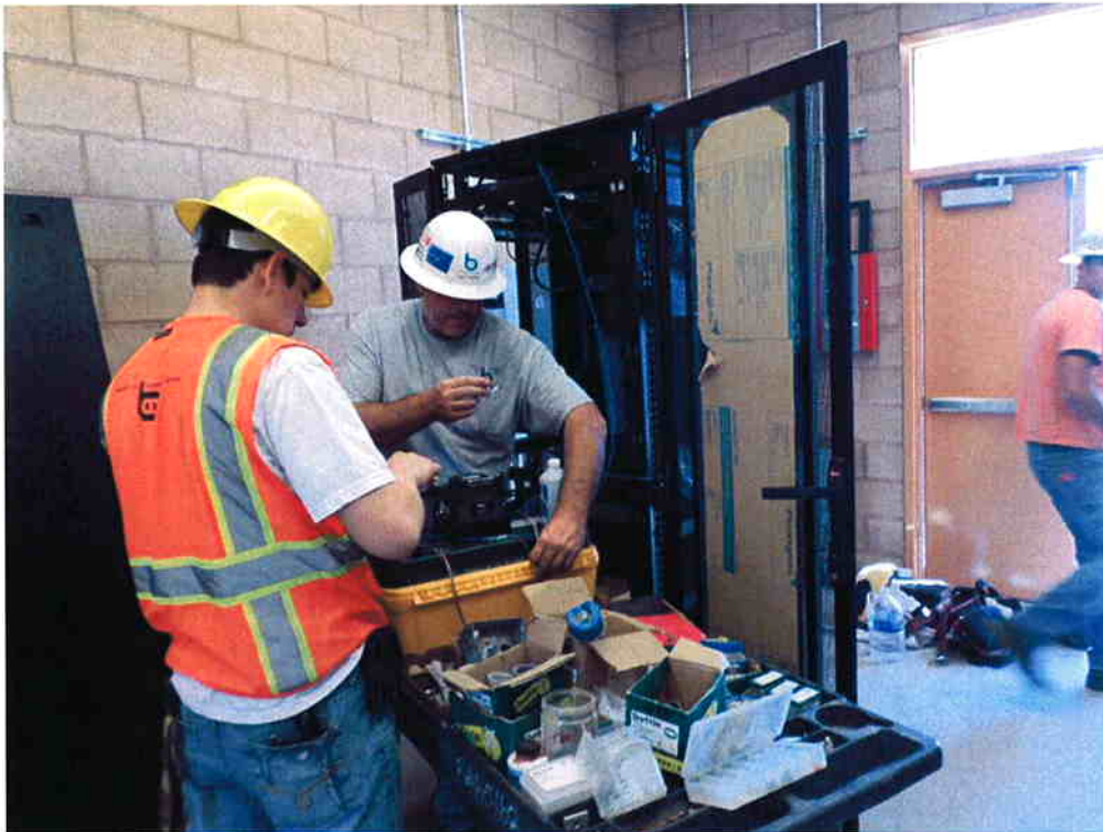
Cushman terminating the new fiber optic line.
