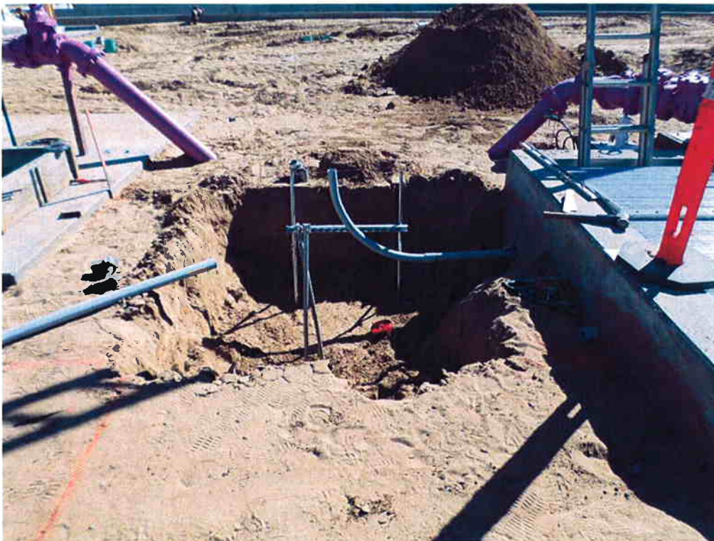
Bergelectric installing conduit for the processed water sampler.
