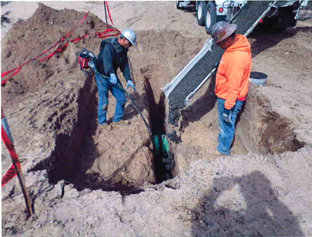
Cushman pouring concrete collar around pipe between Infiltration Ponds 1 & 2.
