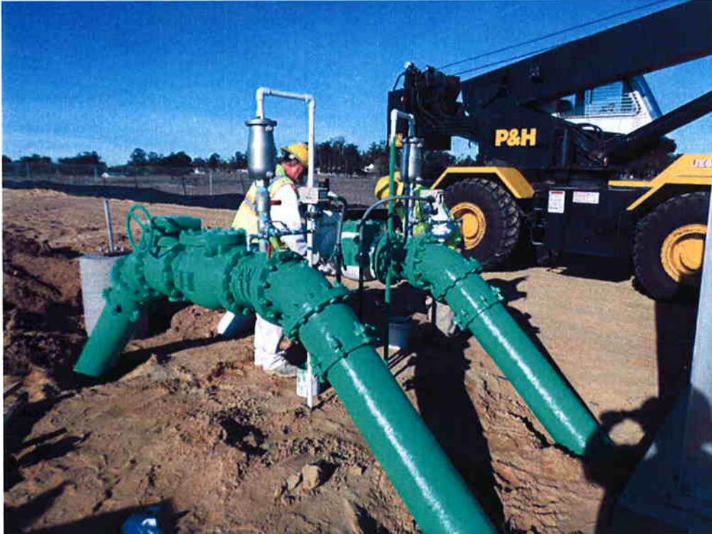
KNK Coating applying finish coat to piping leaving Influent Pump Station.
