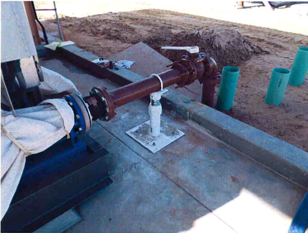
Cushman installing pipe support at WAS piping.
