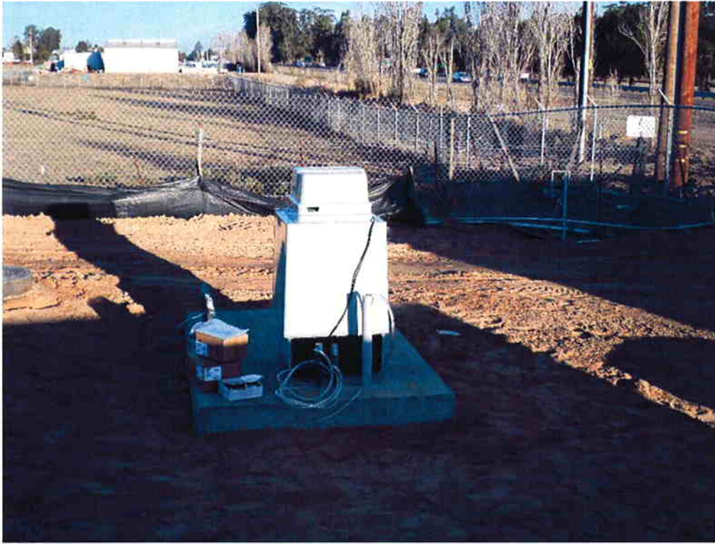
Installing influent pump sampler.
