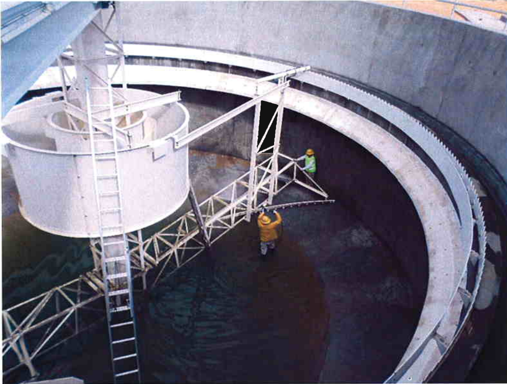
Draining and power washing inside Clarifier #2 in preparation for repair of corroded areas.
