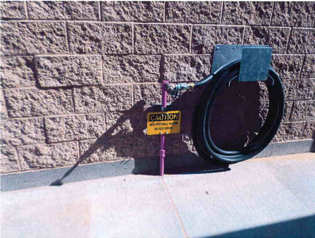
Non-potable water signs installed.
