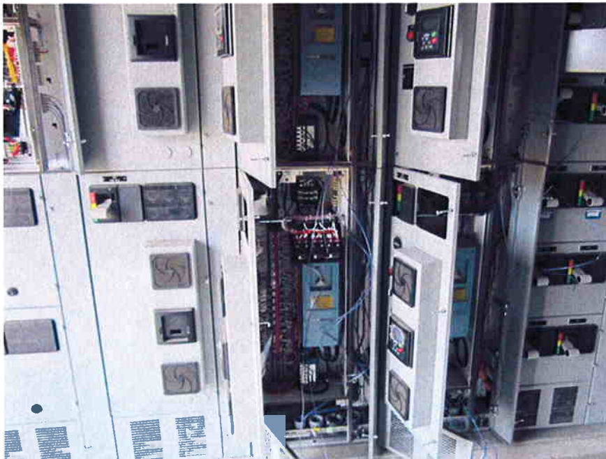
Bergelectric pulling wires inside MCC panels.
