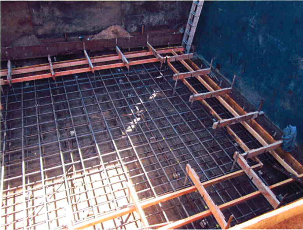
Forms and reinforcing for the slab.
