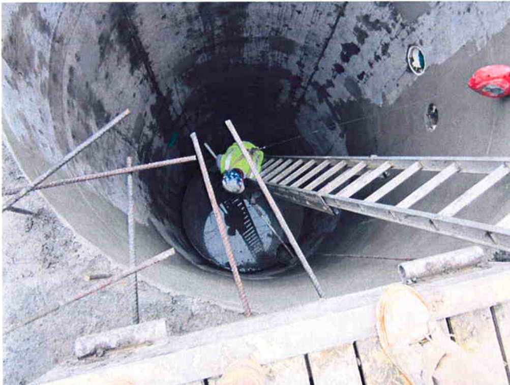
KNK Coating applying Xypex to the inside of the Scum Well.
