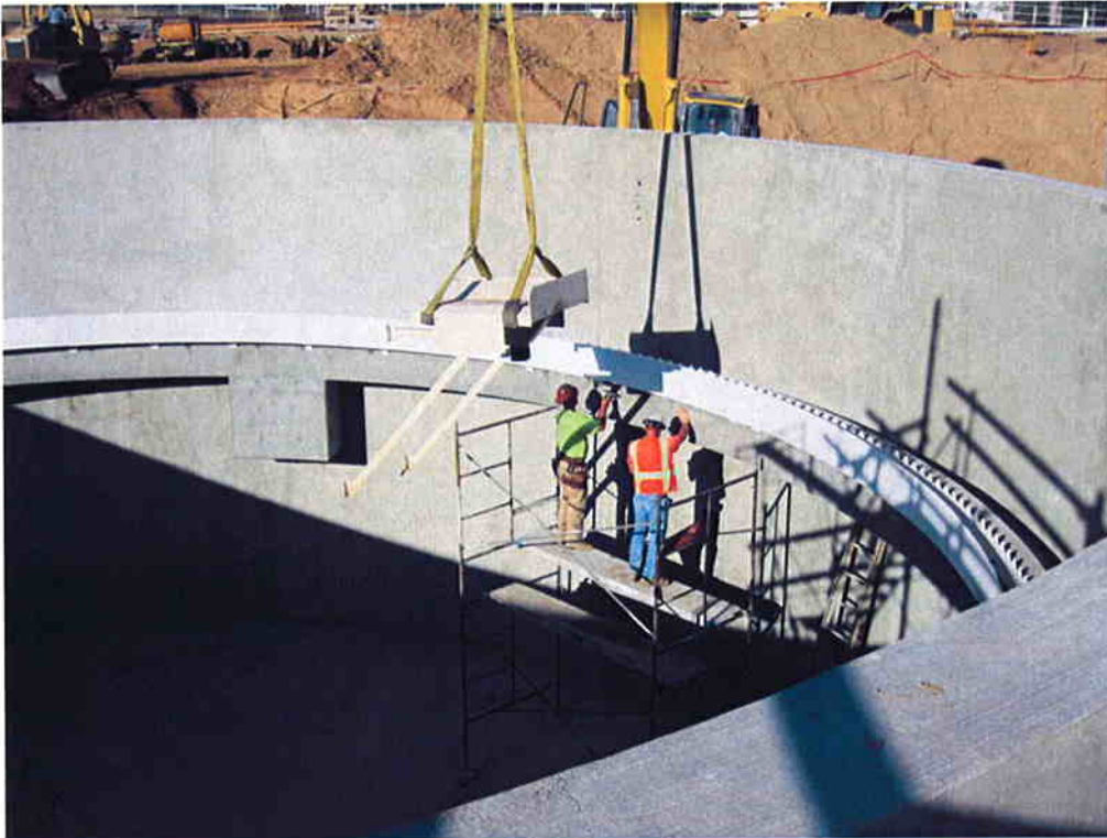
Cushman installing the scum trough inside Clarifier #1.
