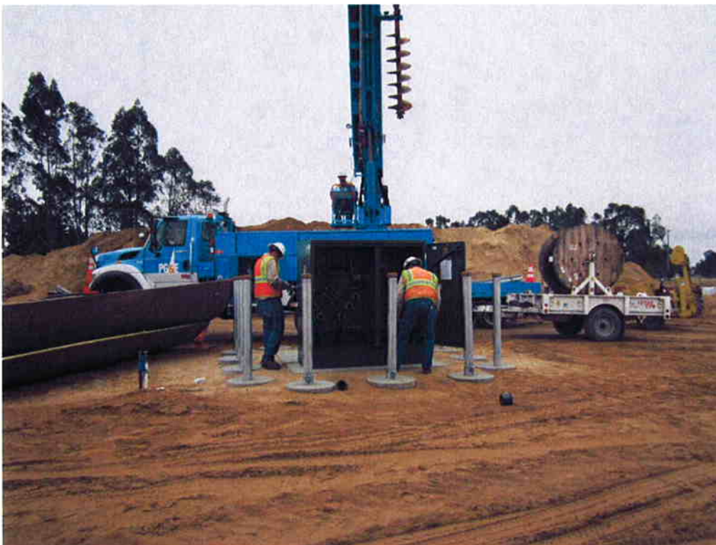
PG&E setting new transformer.
