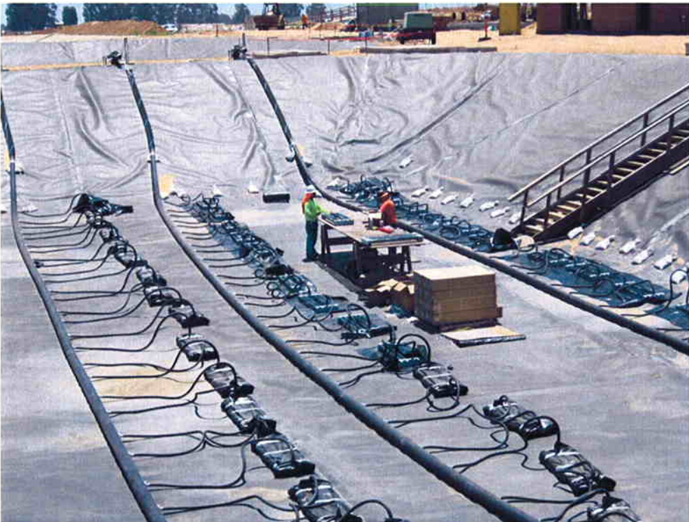
Cushman assembling the biofusers for the Biolac system.
