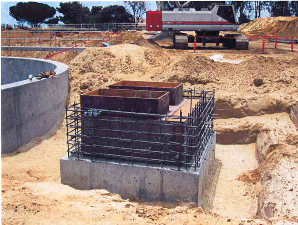
Forming the top of RAS/WAS Pump Station #2.
