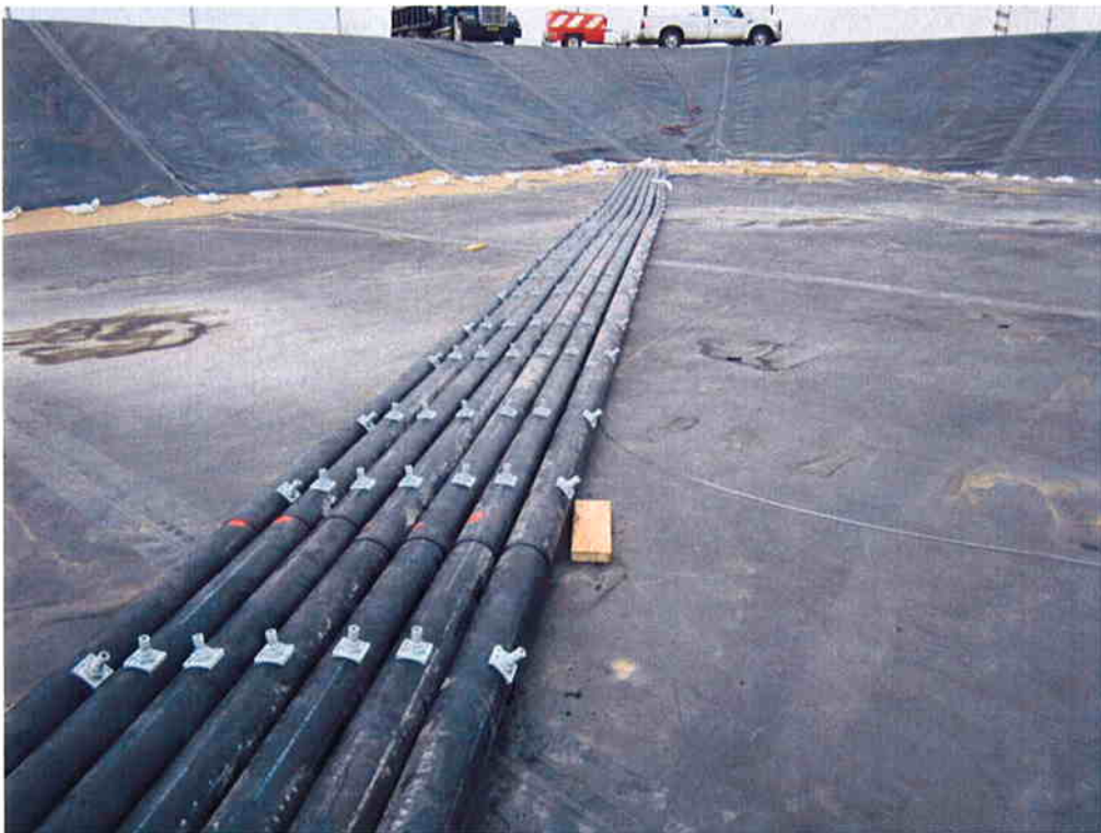
HDPE pipe welding complete and nipples installed on pipe.
