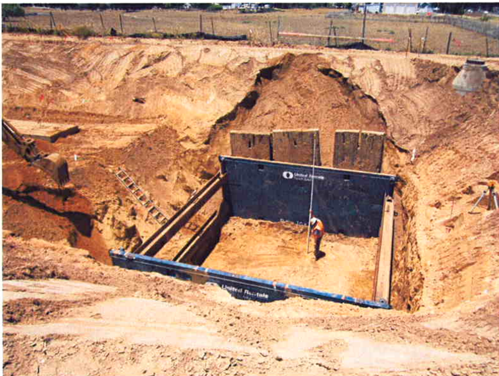
Installing first level of shoring.
