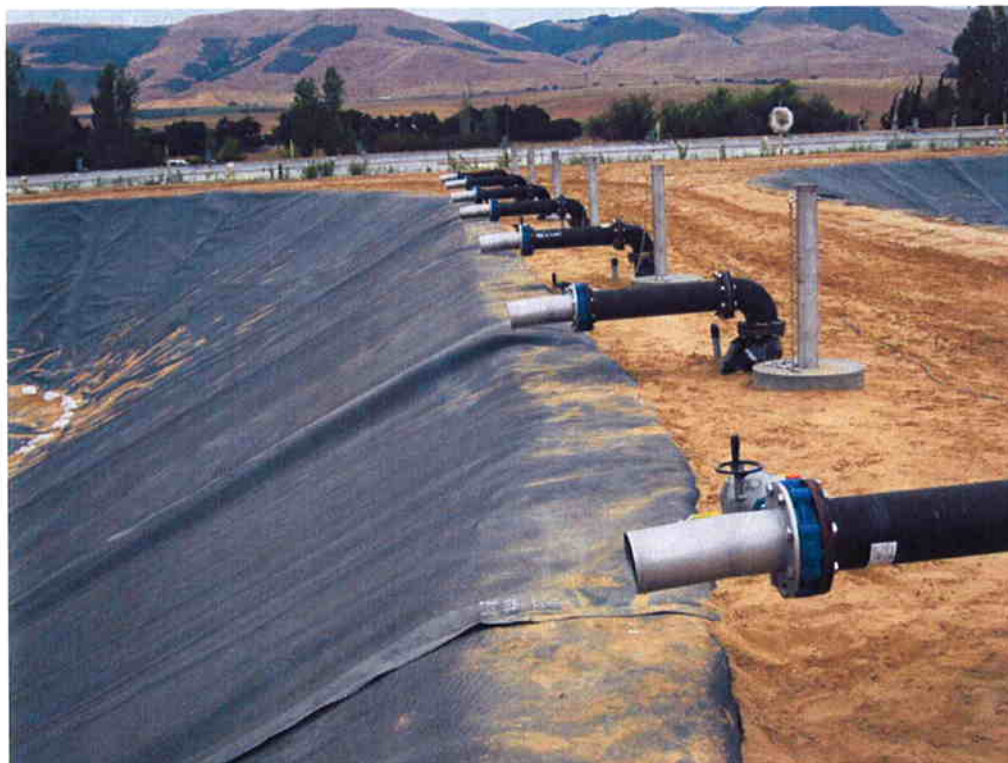
AR piping with valves and posts installed.
