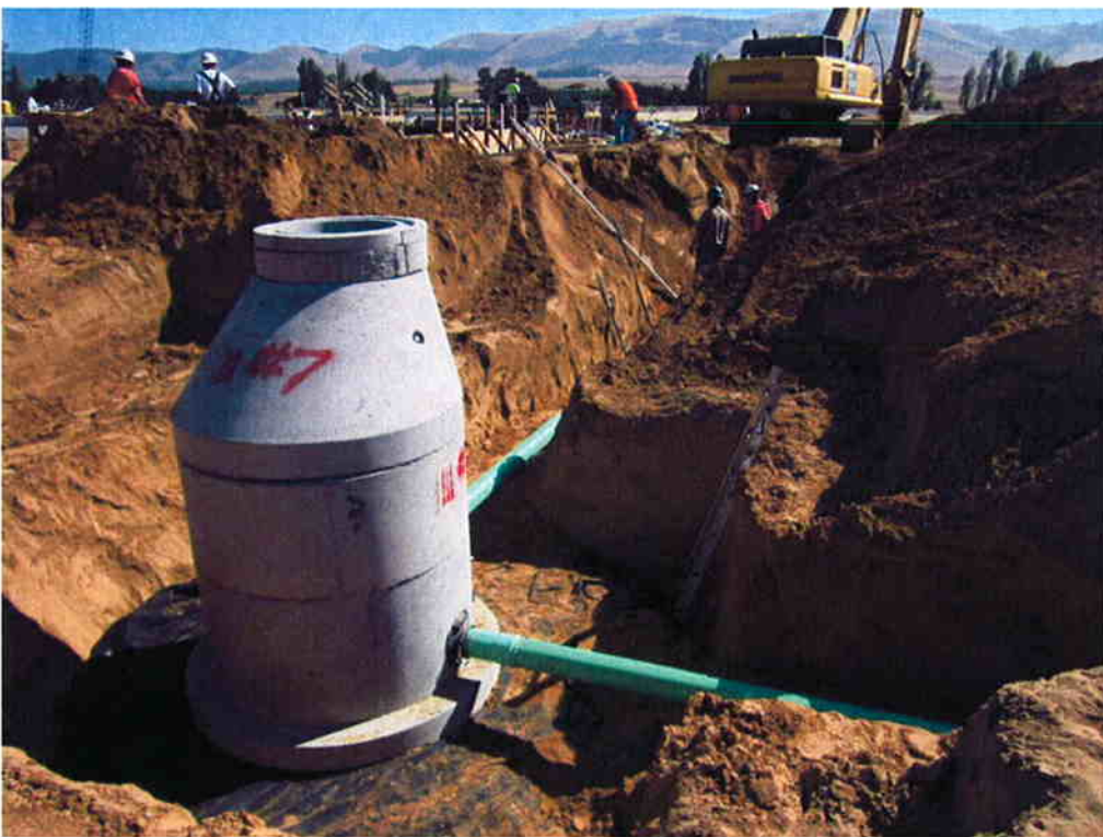
Cushman installing Manhole #7 and 6" DR piping.
