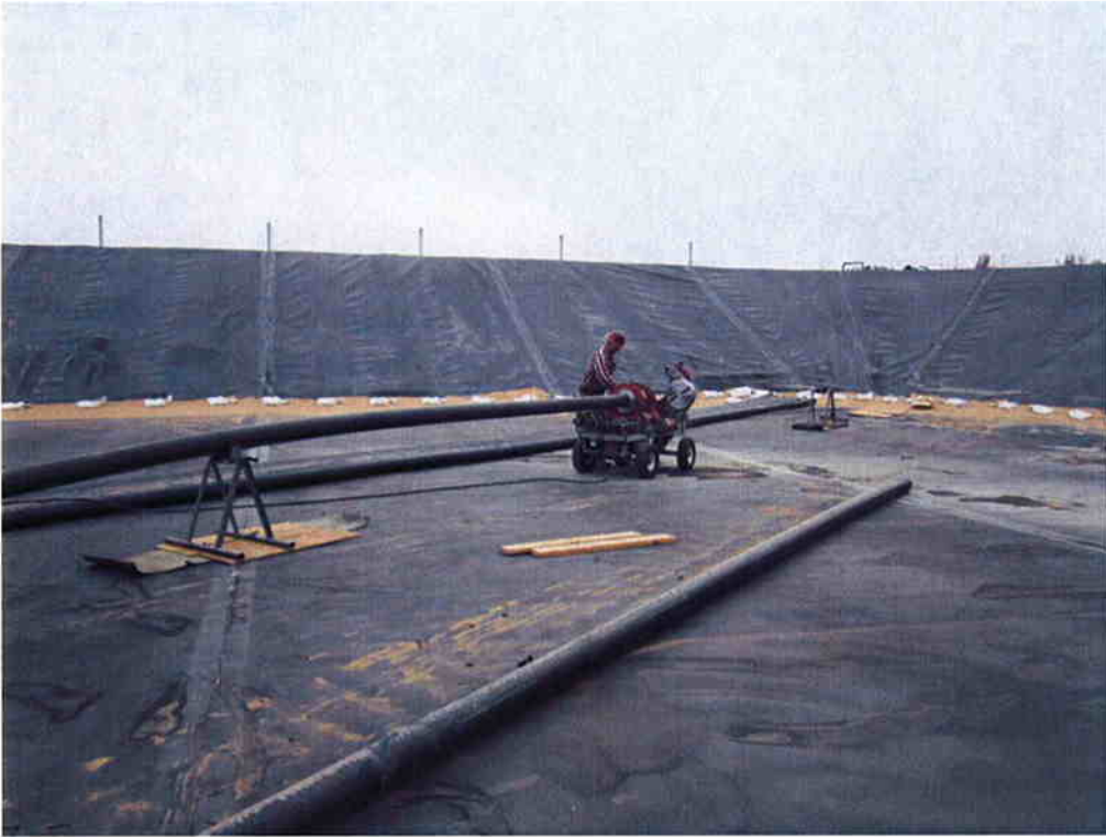
Cushman heat welding HDPE pipe for biofilters.
