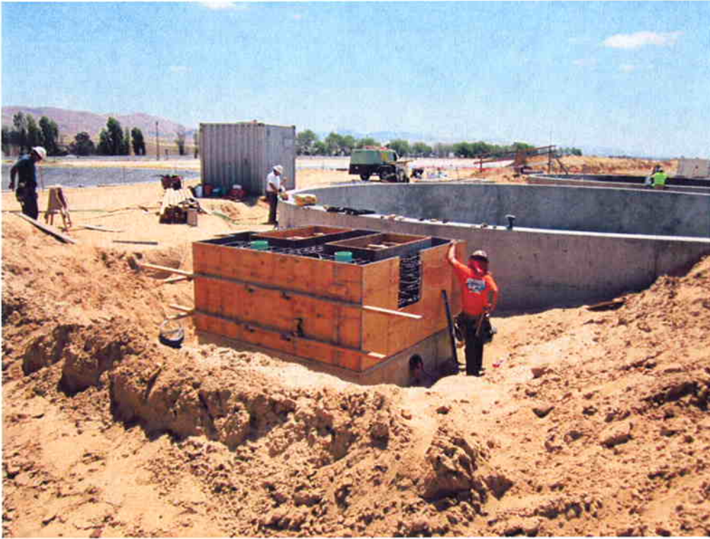
Forming the top of RAS/WAS Pump Station #2.
