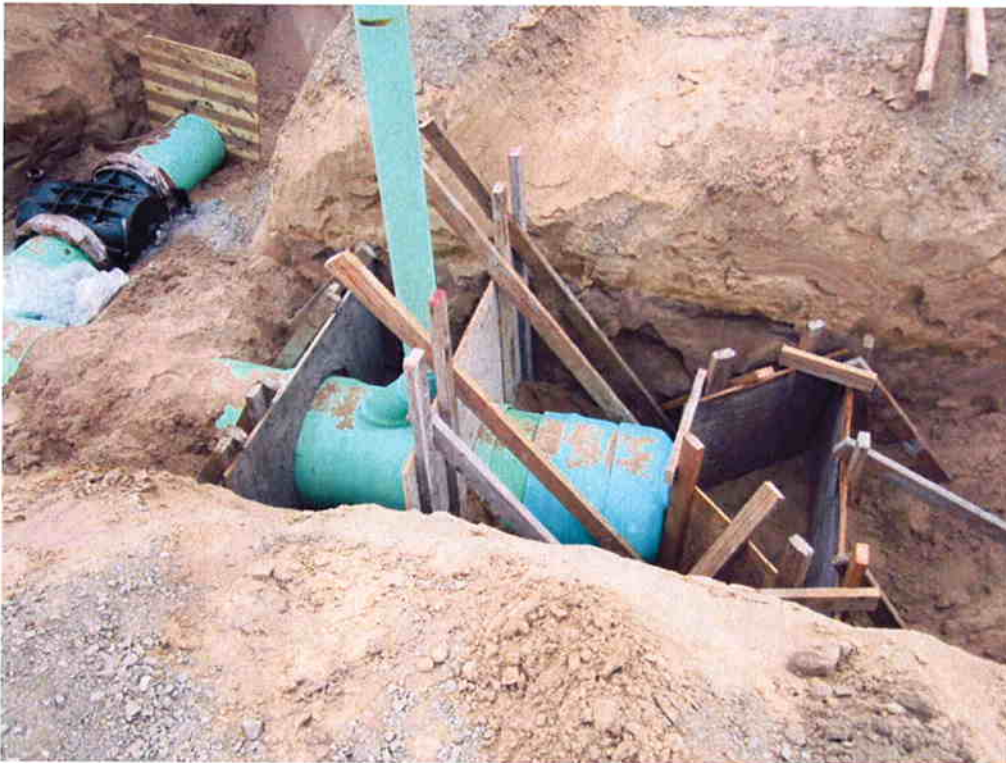
Forms for pouring thrust block at a tee on the 24" SE2 pipe.
