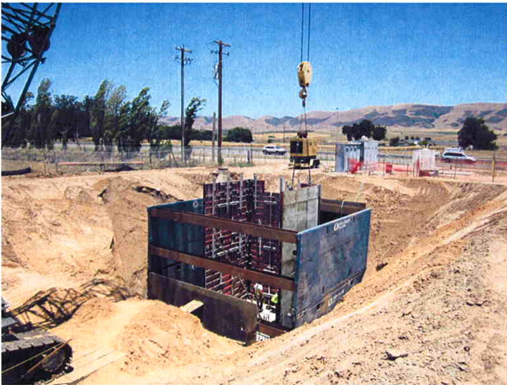
Installing interior wall forms.
