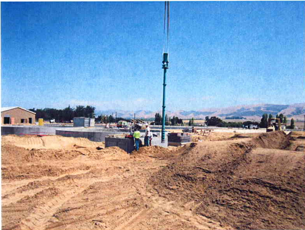
Installing vertical turbine pump shafts inside the Process Water Pump Station.
