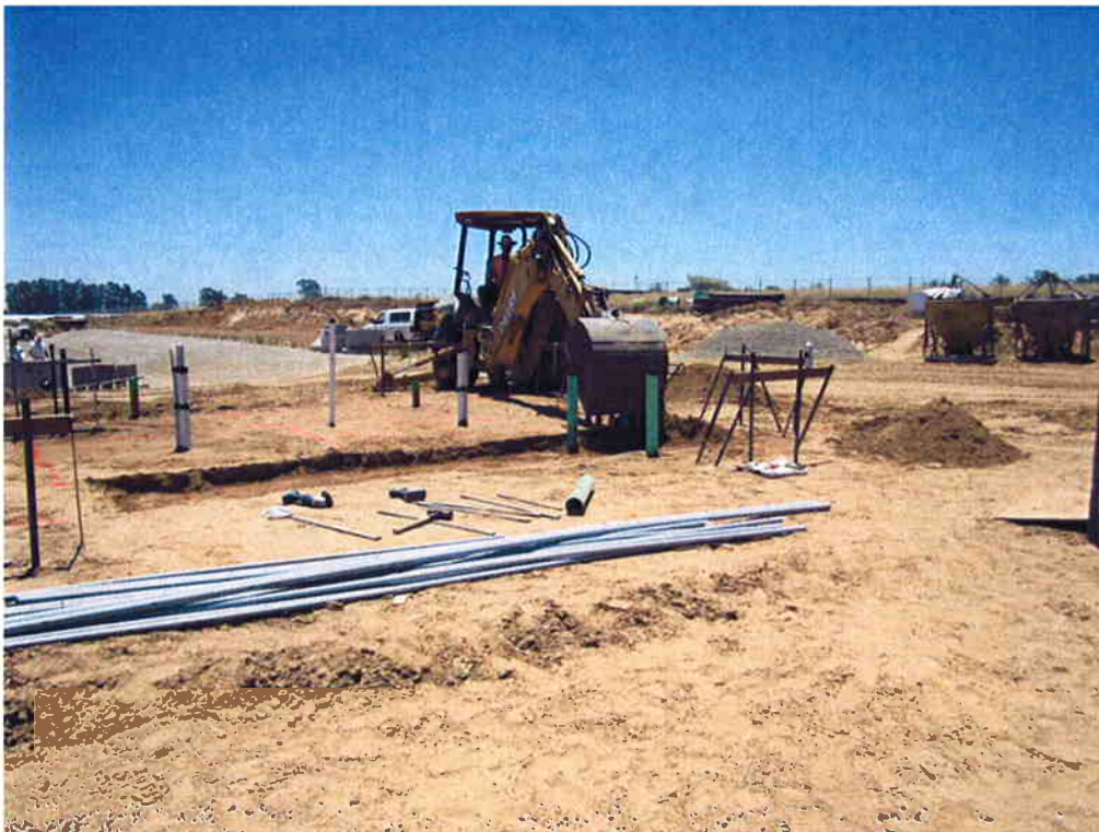
Cushman excavating for the footings of the Sodium Hypochlorite Storage building.
