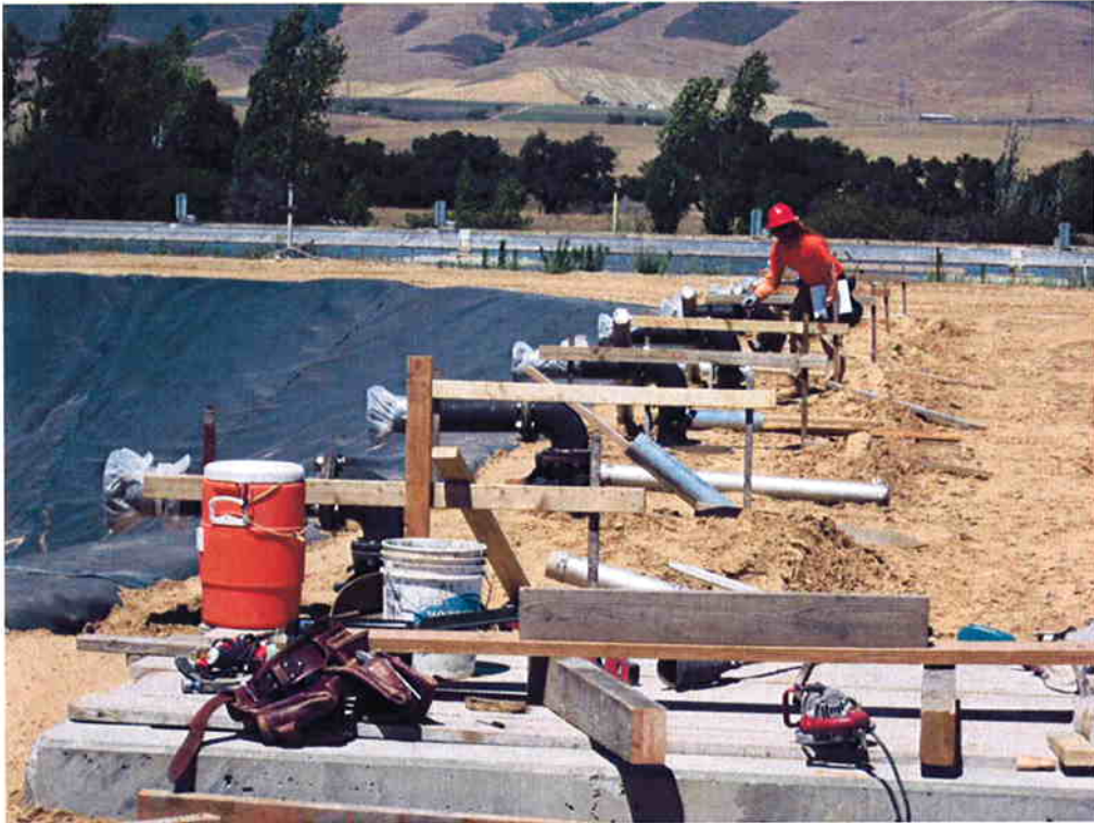
Installing anchor posts for the biofusers.
