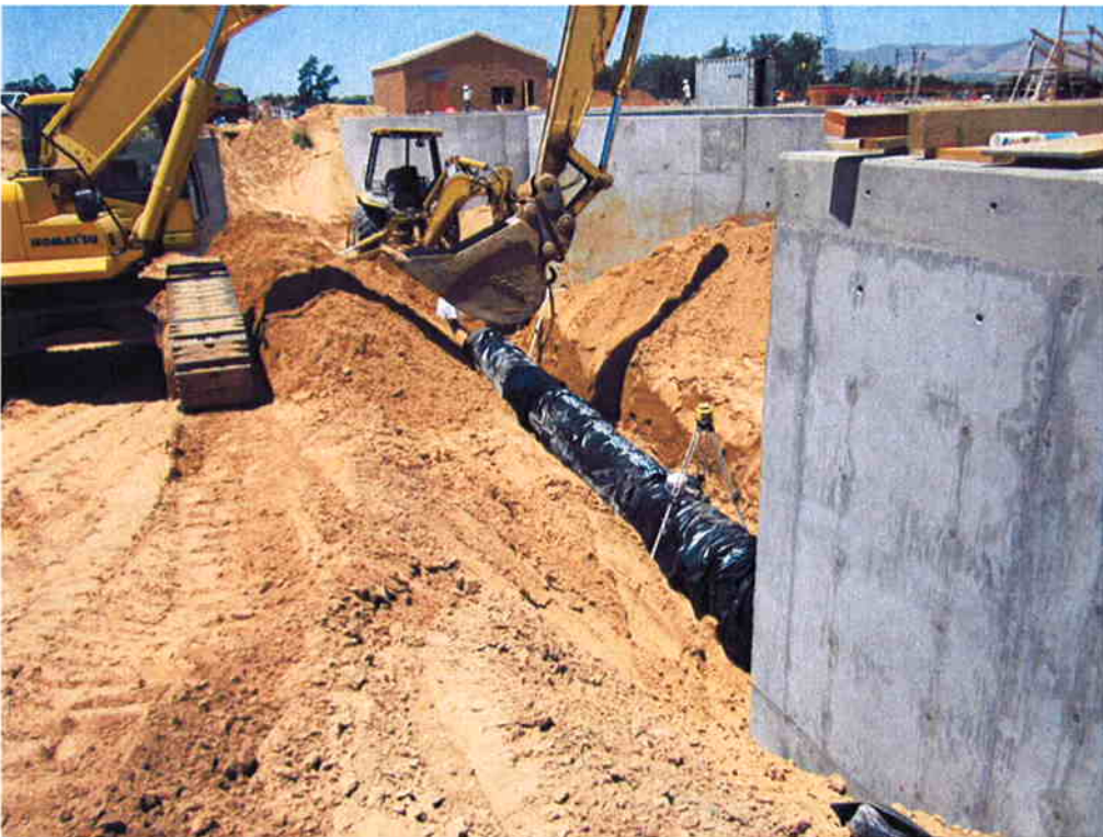
Cushman installing the 16" SE1 piping between the Process Water Pump Station and Clarifier #1.
