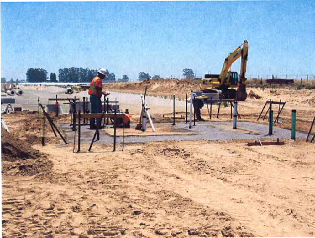
Compacting the base for the footings of the Sodium Hypochlorite Storage building.
