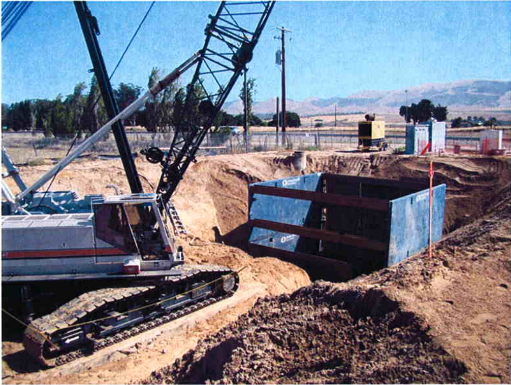
Installing second level of shoring.
