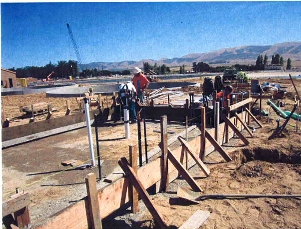
Cushman preparing forms for the Sodium Hypochlorite Storage building foundation.
