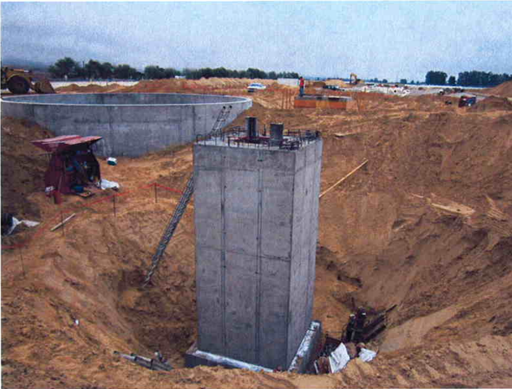
Scum Well wall forms removed.
