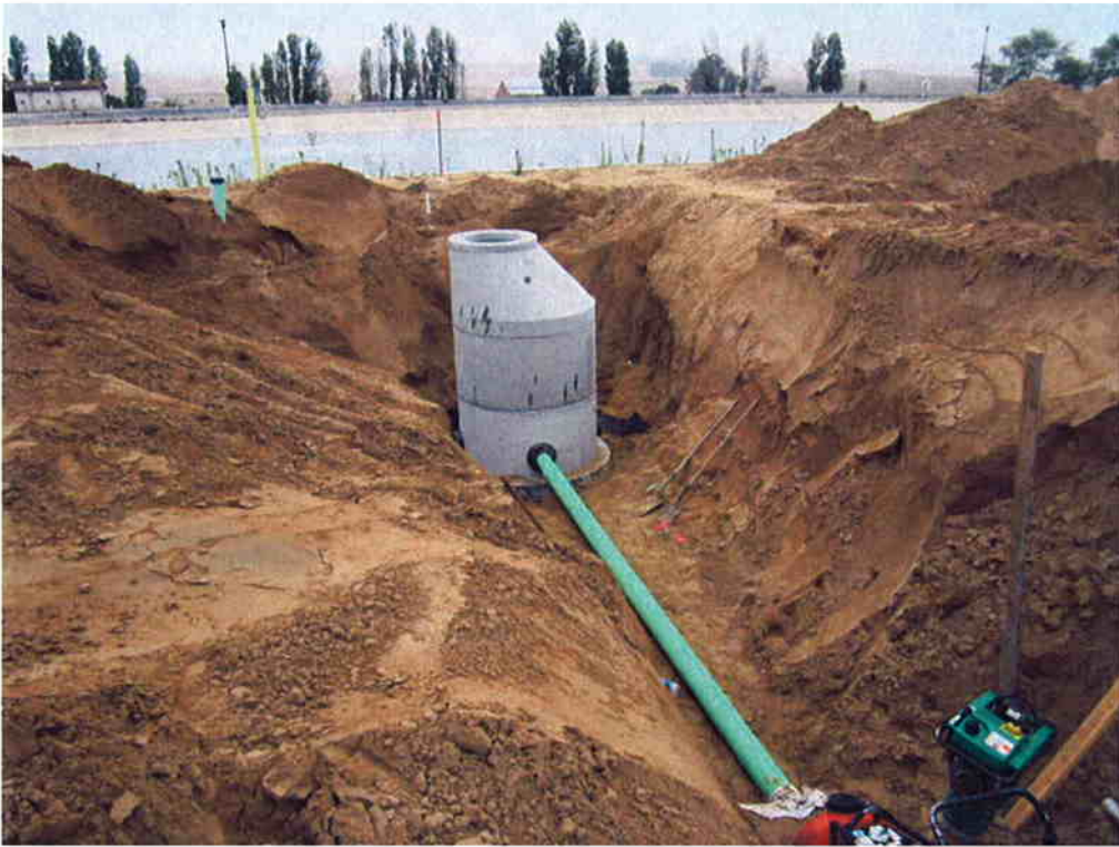
Manhole #6 installed with 6" DR piping to Manhole #7.
