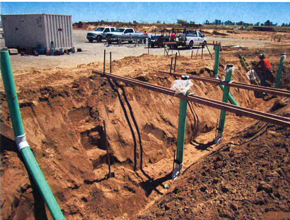
Installation of 6" DR piping from Manhole #6 to the Sludge Thickening Building.
