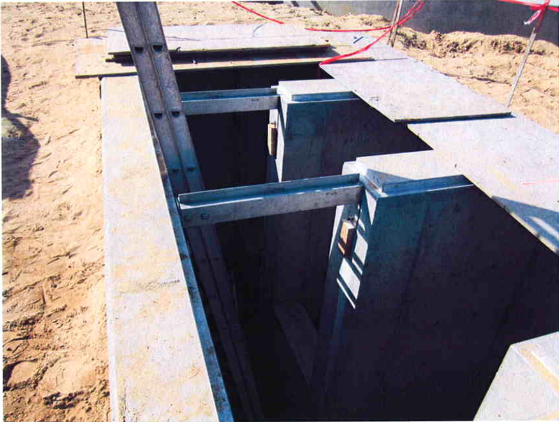
Installing beams for grating support at Distribution Box #2.
