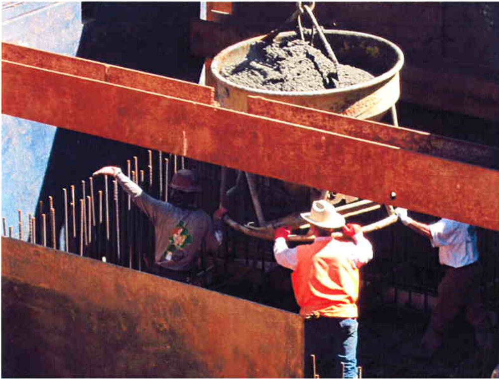
Pouring concrete for the slab.
