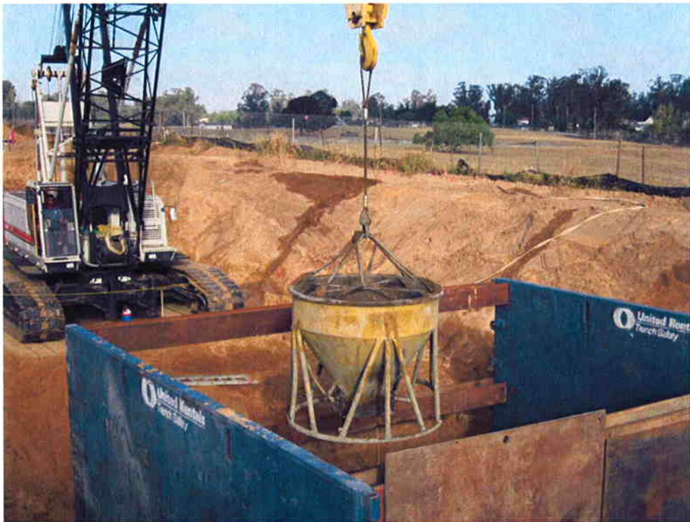
Installing base material.
