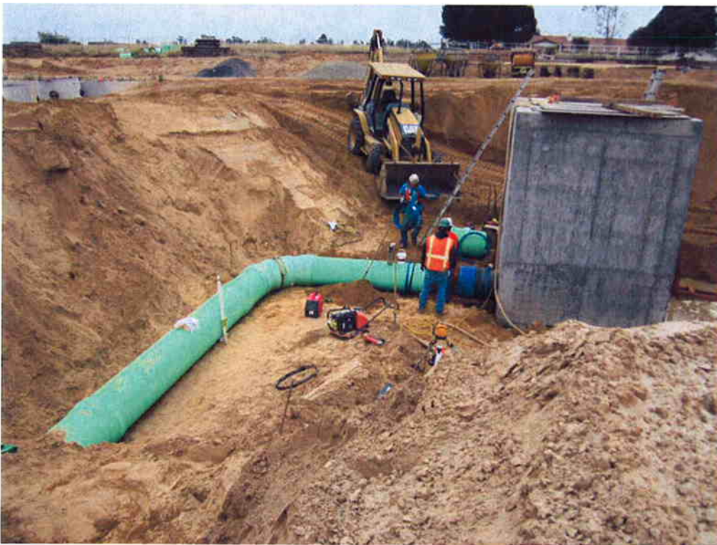
Connecting the 24" SE2 piping to the Process Water Pump Station.
