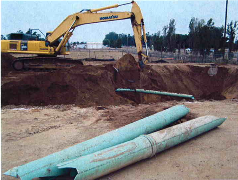
Excavating for influent pump station. Cushman found unidentified 10" PVC C-900 pipe.
