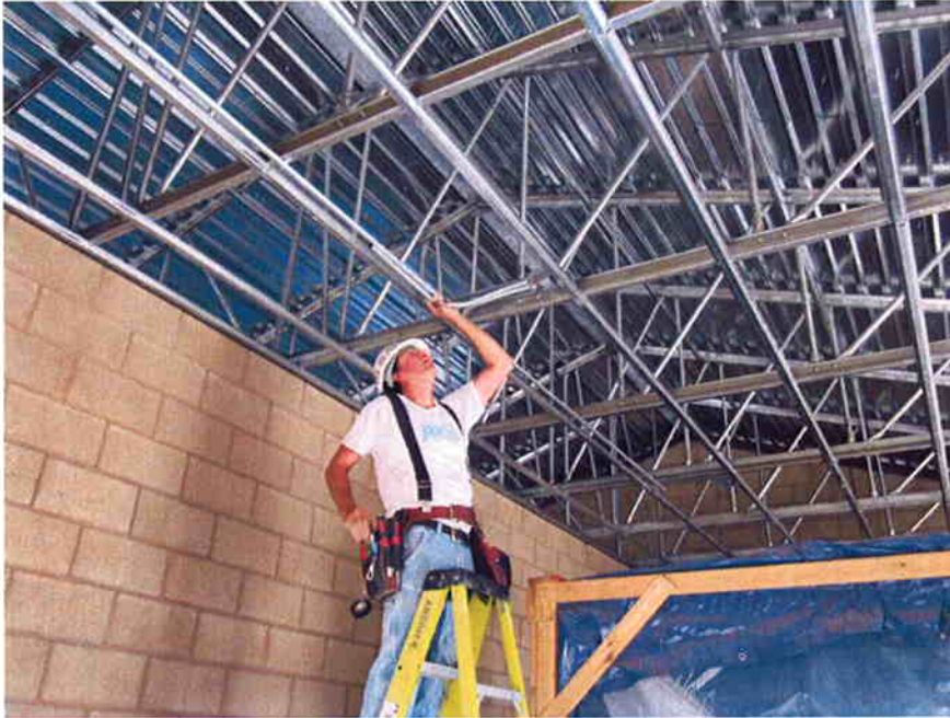
Bergelectric installing lighting conduit.
