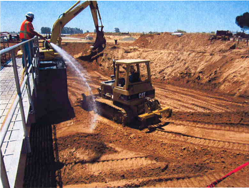
Backfilling around the Scum Well.
