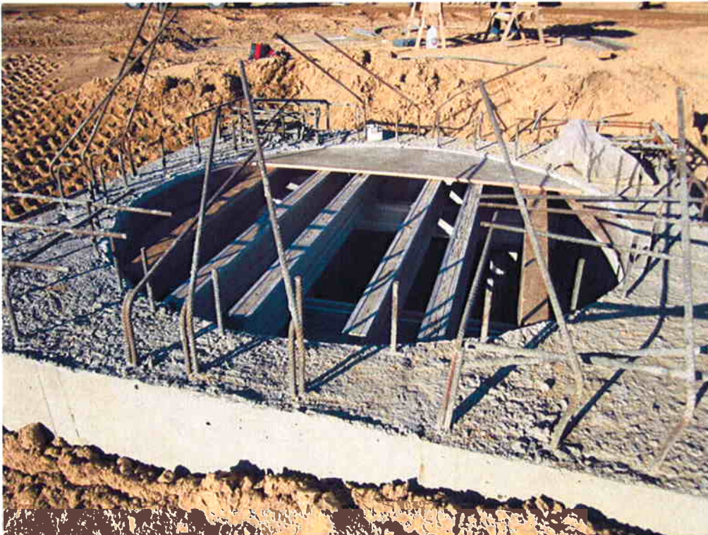
Cushman installing forms for pouring the top of the Scum Well.
