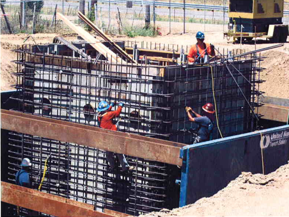
Installing rebar for walls.
