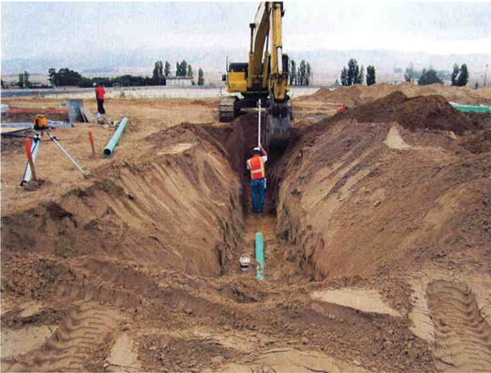
Excavating for the 6" DR pipe.
