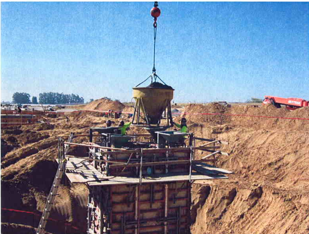
Cushman pouring the Scum Well walls.
