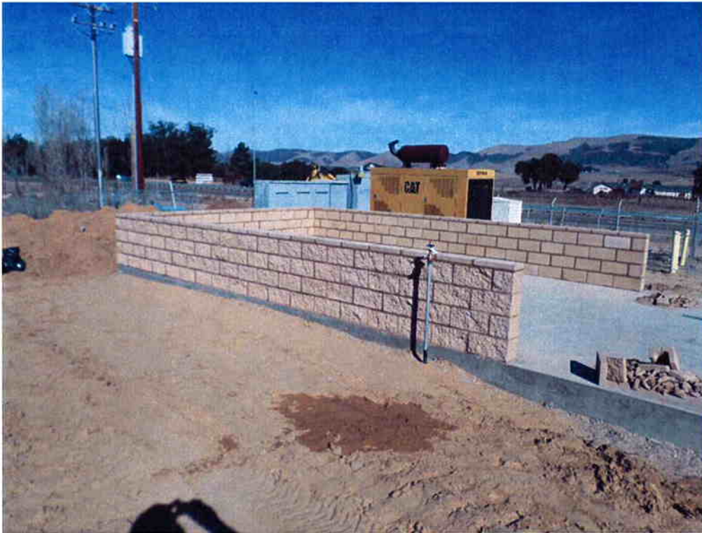
Truck wash down station wall completed.
