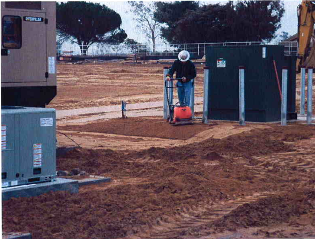
Cushman grading around the Electrical/Blower Building.
