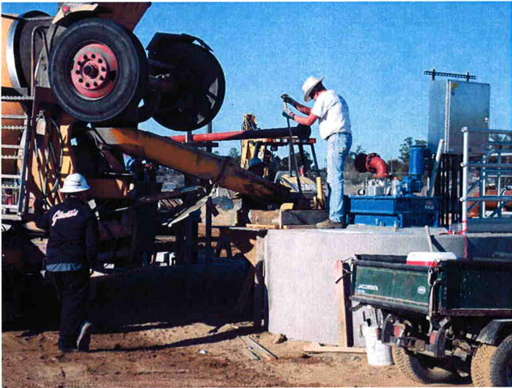
Cushman pouring the pad for the Grit Pump.
