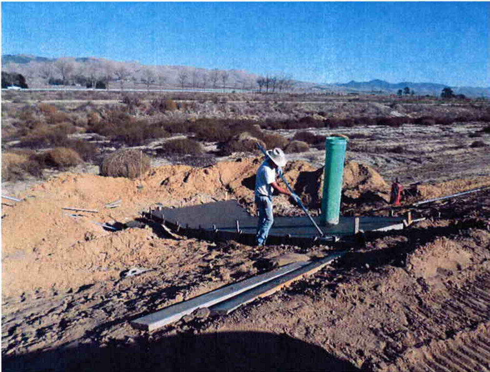
Cushman pouring the concrete pad at the overflow in Infiltration Pond #3.
