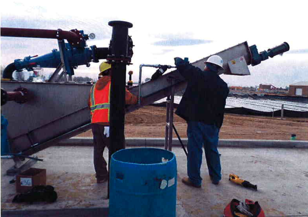
Bergelectric installing conduit to the solenoid valve at the Grit Classifier.
