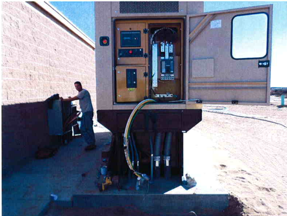
Bergelectric pulling generator feed cables at the new Emergency Generator.
