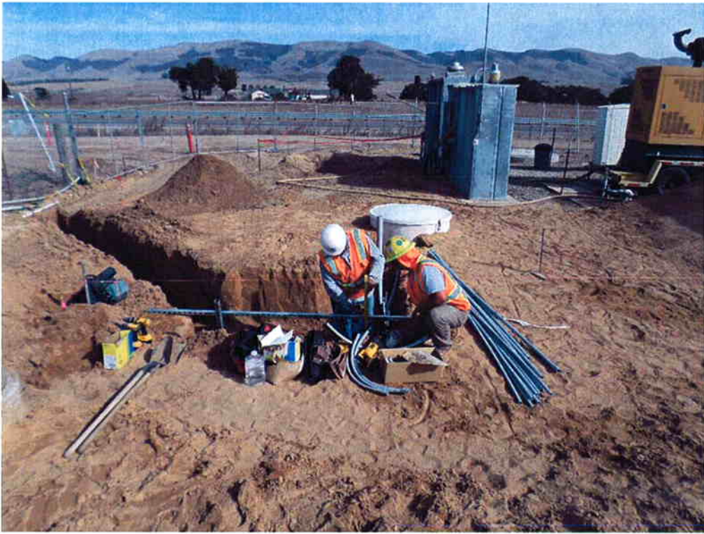
Bergelectric installing conduit at the Influent Sampler.
