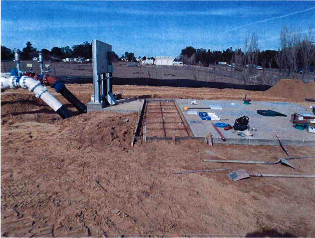
Forms and rebar for sidewalk between the control panel pad and the Influent Pump Station.
