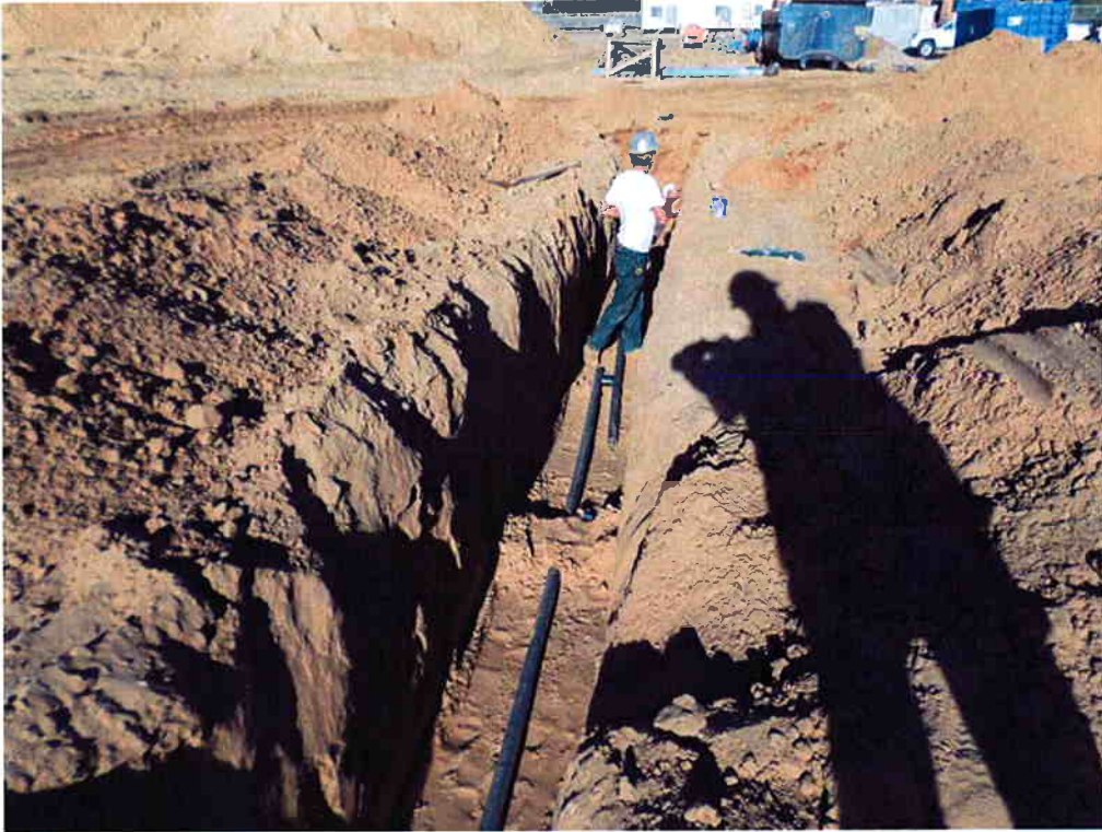
Cushman installing 2-inch non-potable water line.
