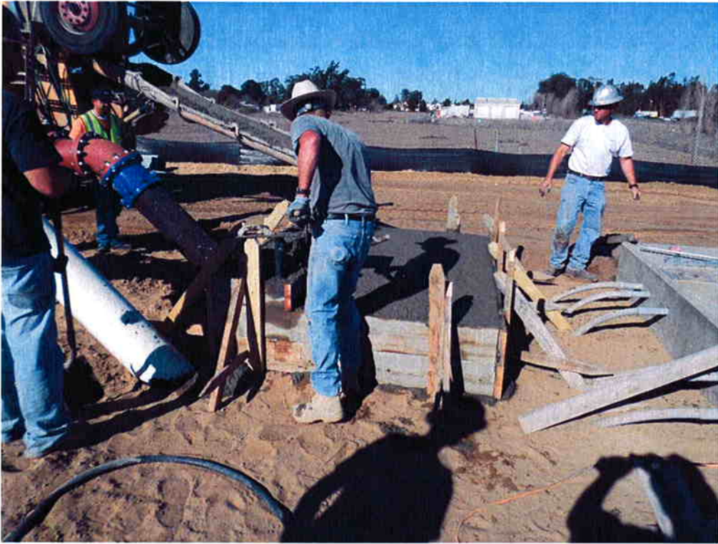
Cushman pouring concrete at the control panel pad for the Influent Pump Station.
