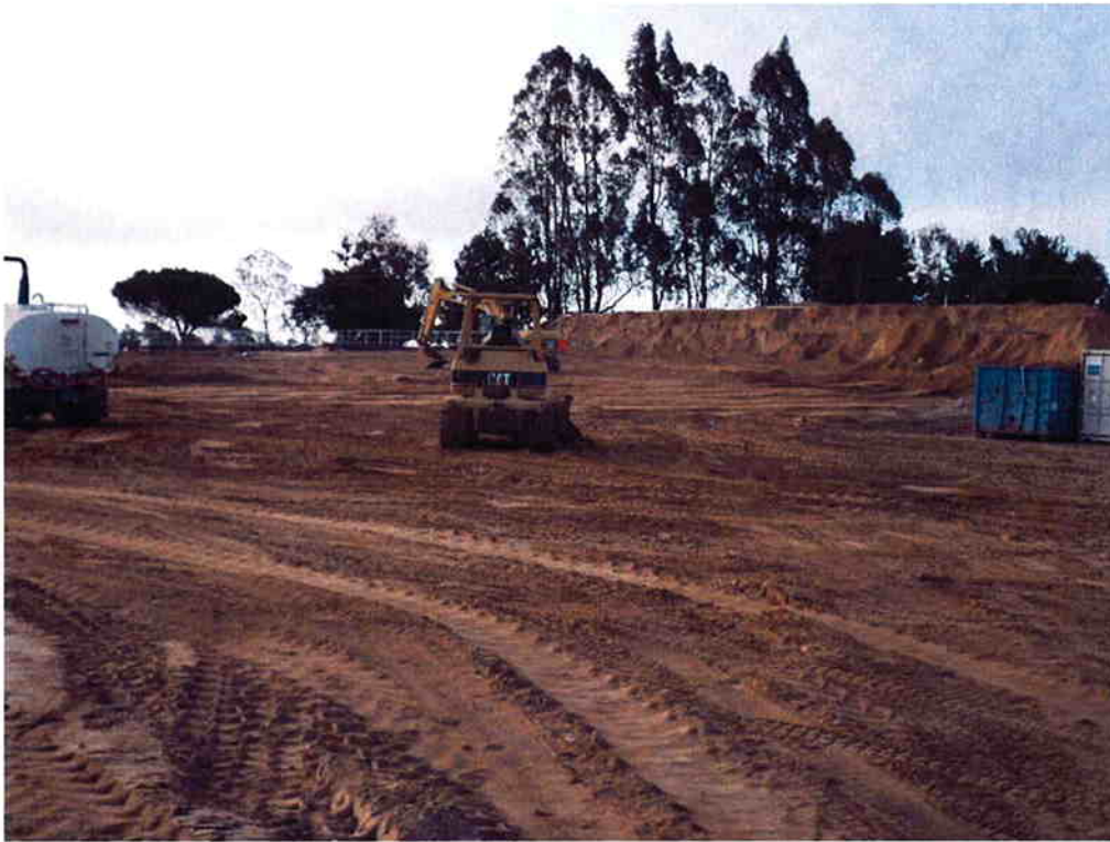
Cushman performing site grading to the north west of the Electrical/Blower Building.
