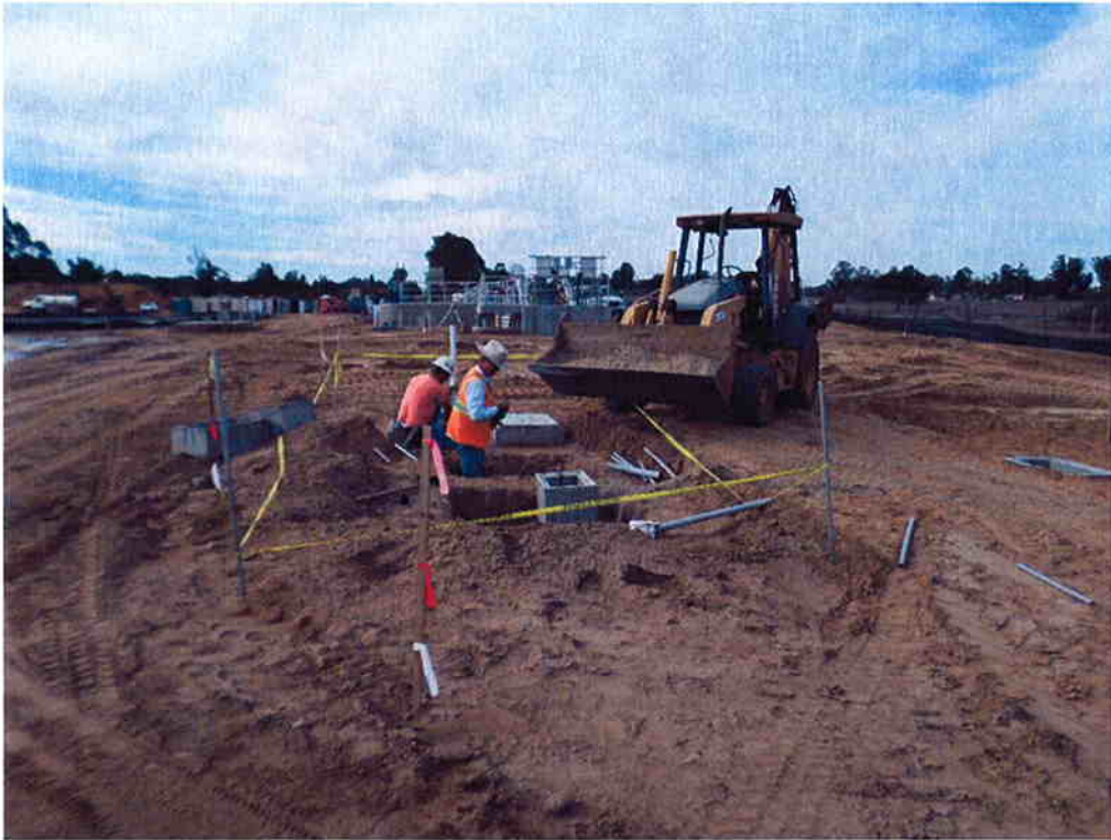
Cushman and Bergelectric setting boxes for PB01.
