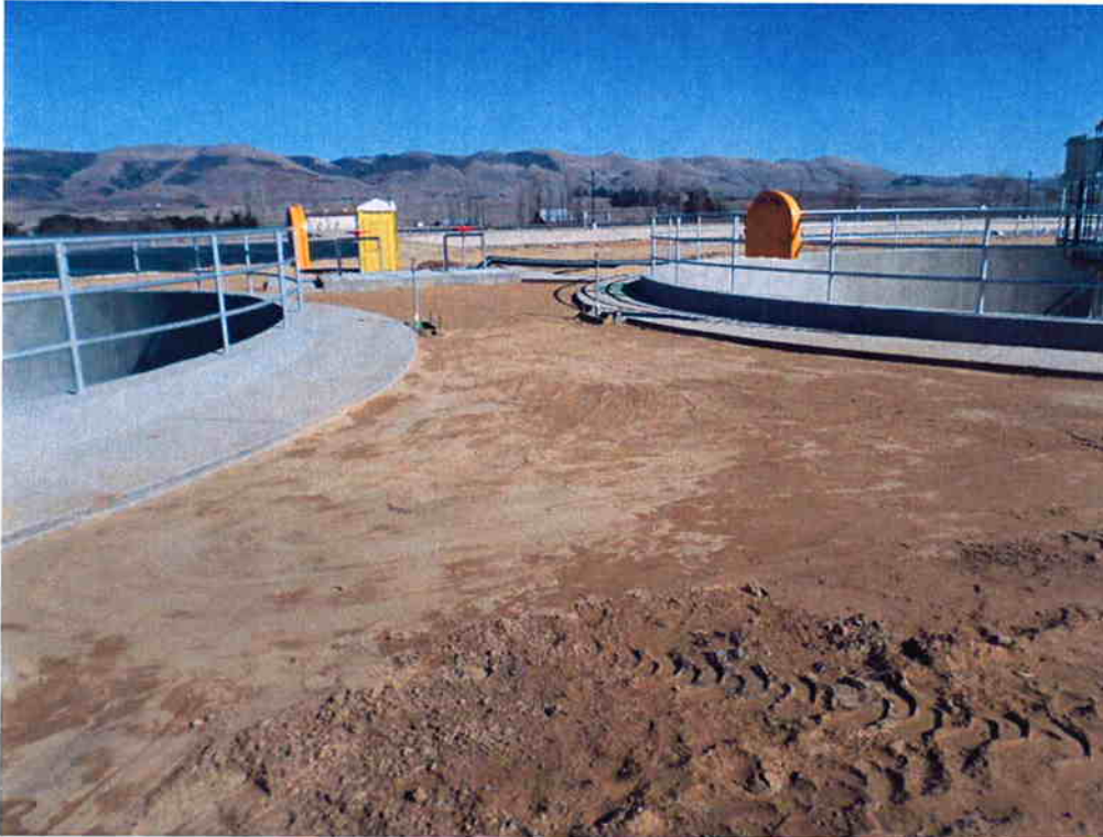
Grading between the clarifiers.
