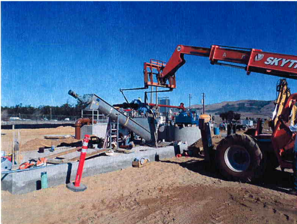
Cushman installing the piping from the Grit Pump to the Grit Classifier.
