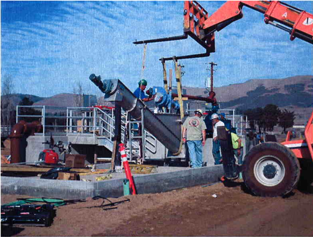
Cushman installing the Grit Pump for the Grit Classifier.
