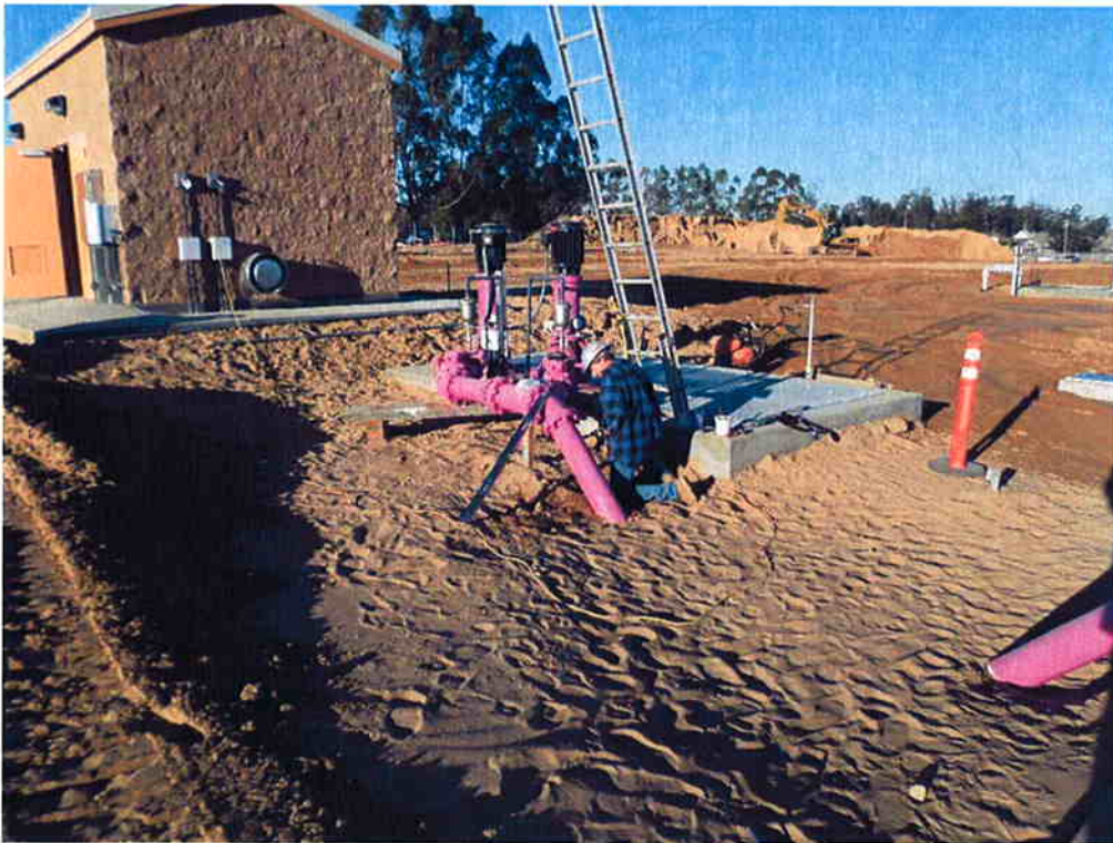
Cushman installing the chemical injection post and assembly.
