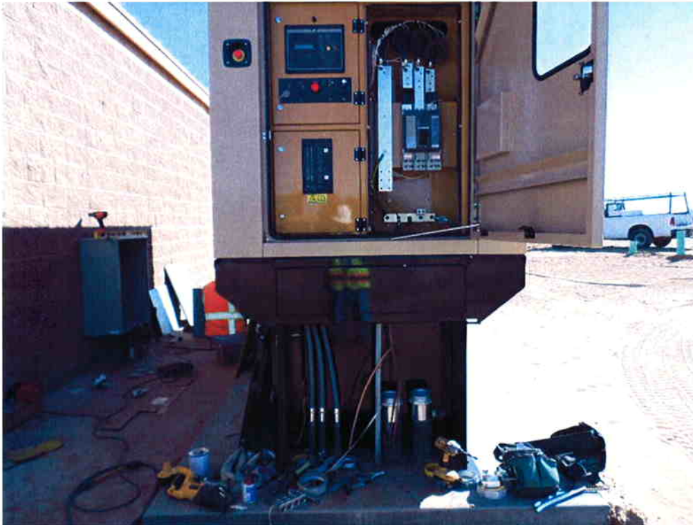
Bergelectric installing conduit and terminating at the new Emergency Generator.
