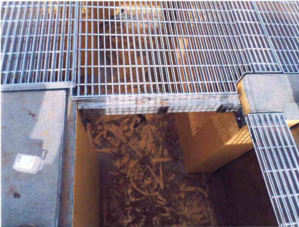
Cushman installing grating support beams.
