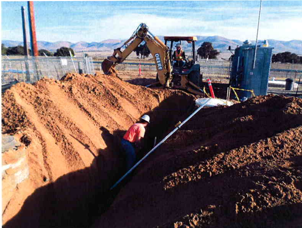
Cushman installing the 6-inch potable water line.
