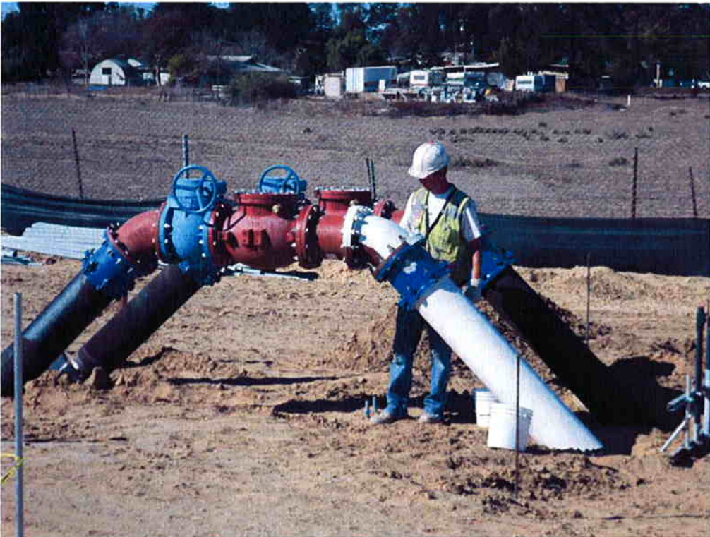
KNK Coating applying primer to the RW piping between the Influent Pump Station and the Headworks.
