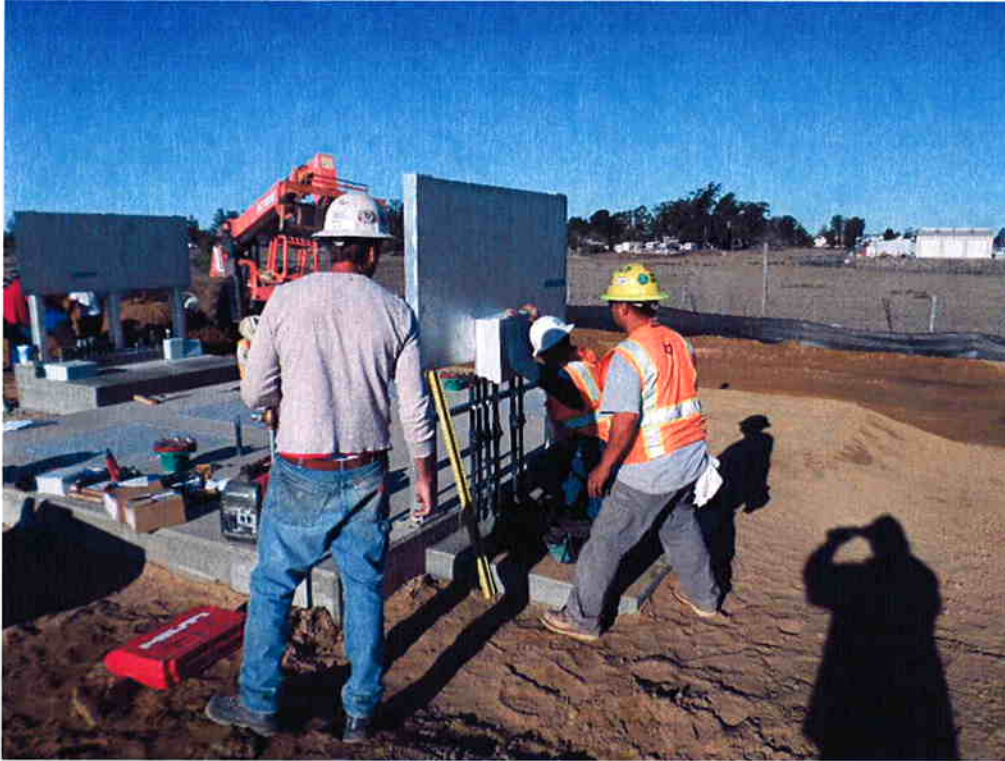
Bergelectric installing the aluminum stand and conduit for the control panel at the Influent Pump Station.
