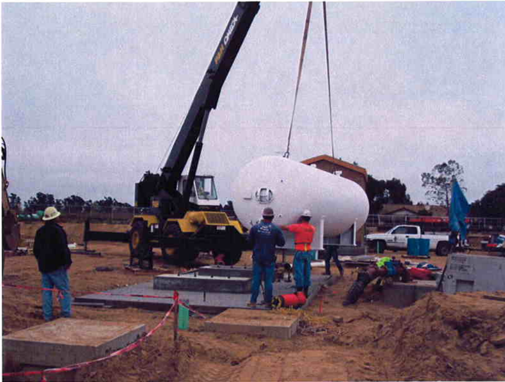
Cushman mounting hydropneumatic tank on supports.
