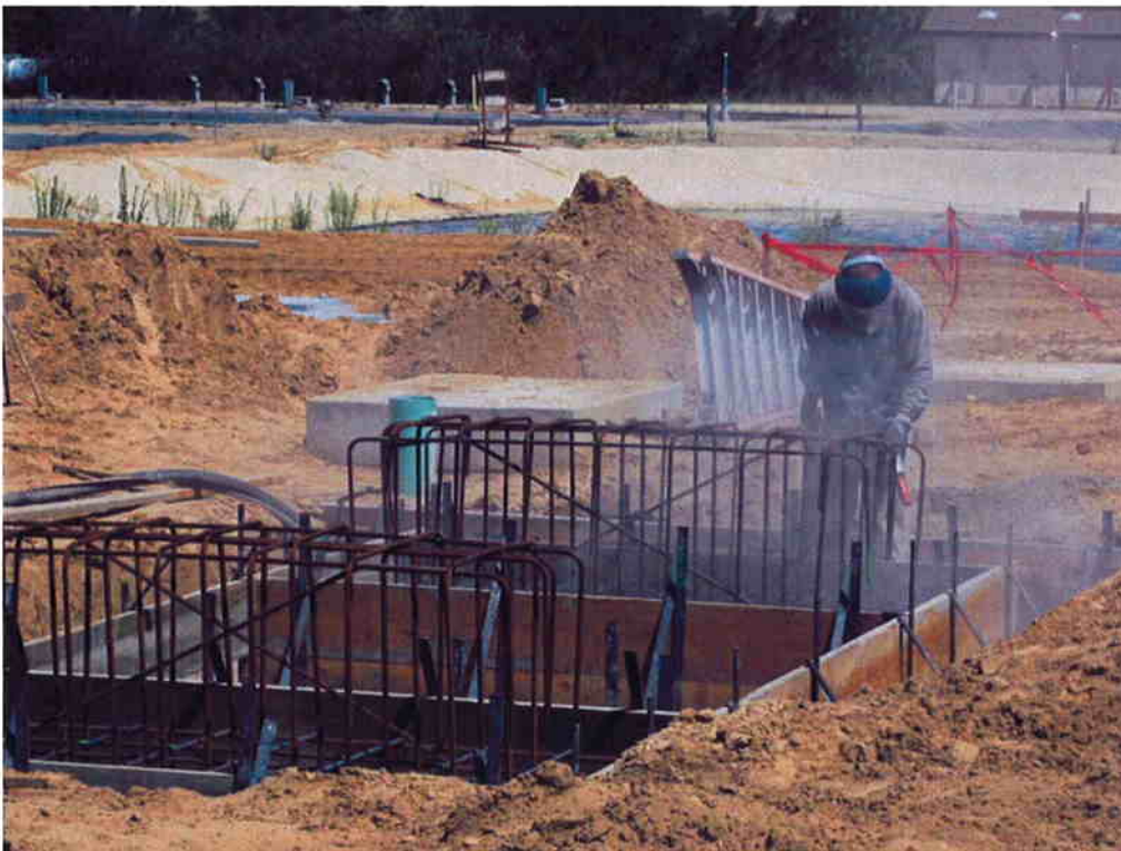
Sandblasting foundation for hydropneumatic tank supports.
