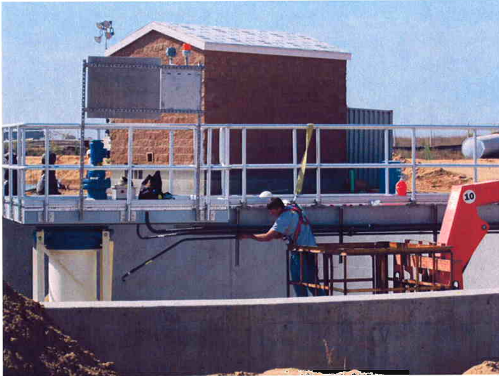
Bergelectric installing PVC rigid coated conduit at Clarifier #1.
