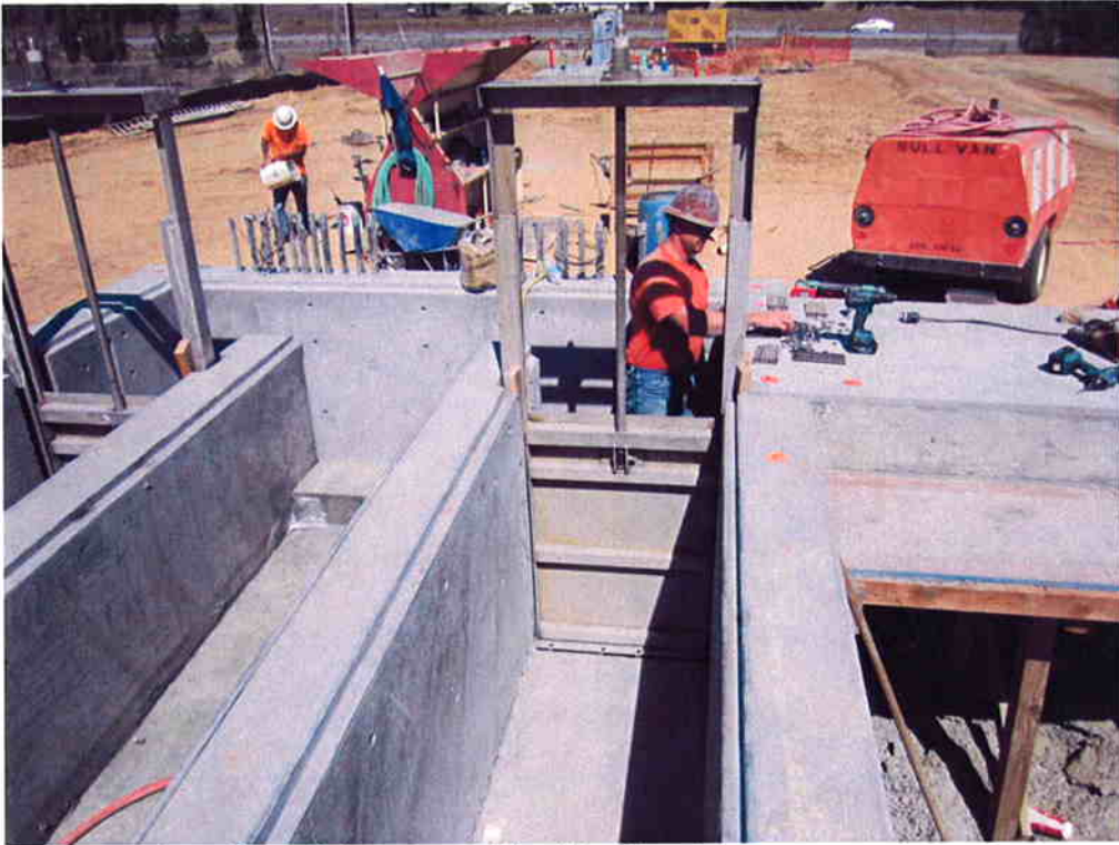
Cushman installing slide gates at the Headworks.
