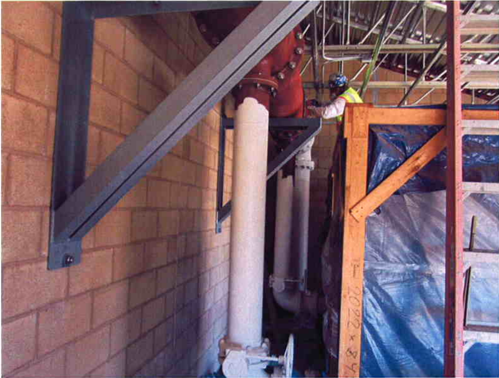
KNK Coating priming AR piping in Blower Room of Electrical/Blower Building.
