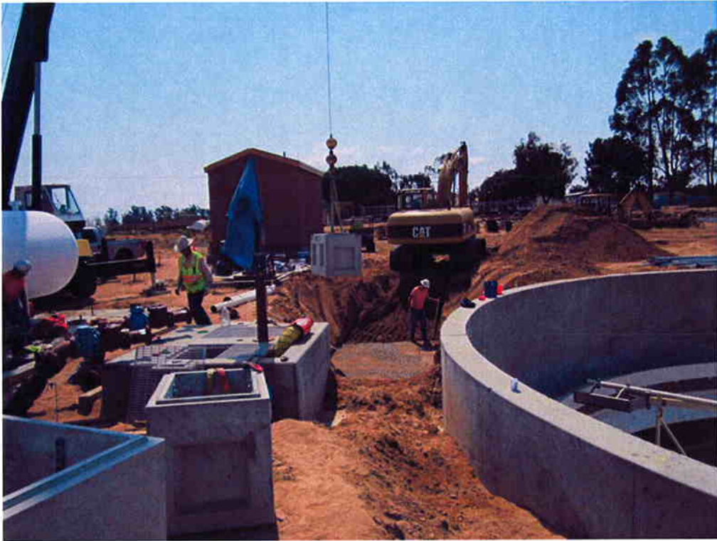
Bergelectric and Cushman installing Pull Box 20.
