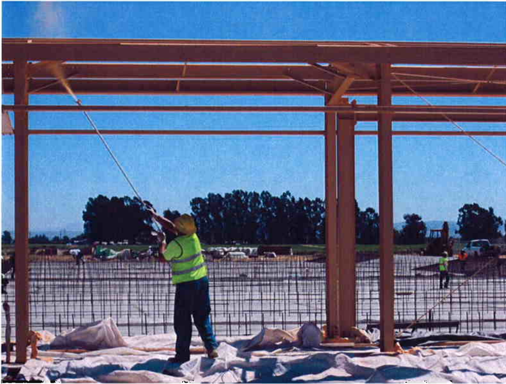
KNK Coating applying finish coat to the Sludge Thickening Building.
