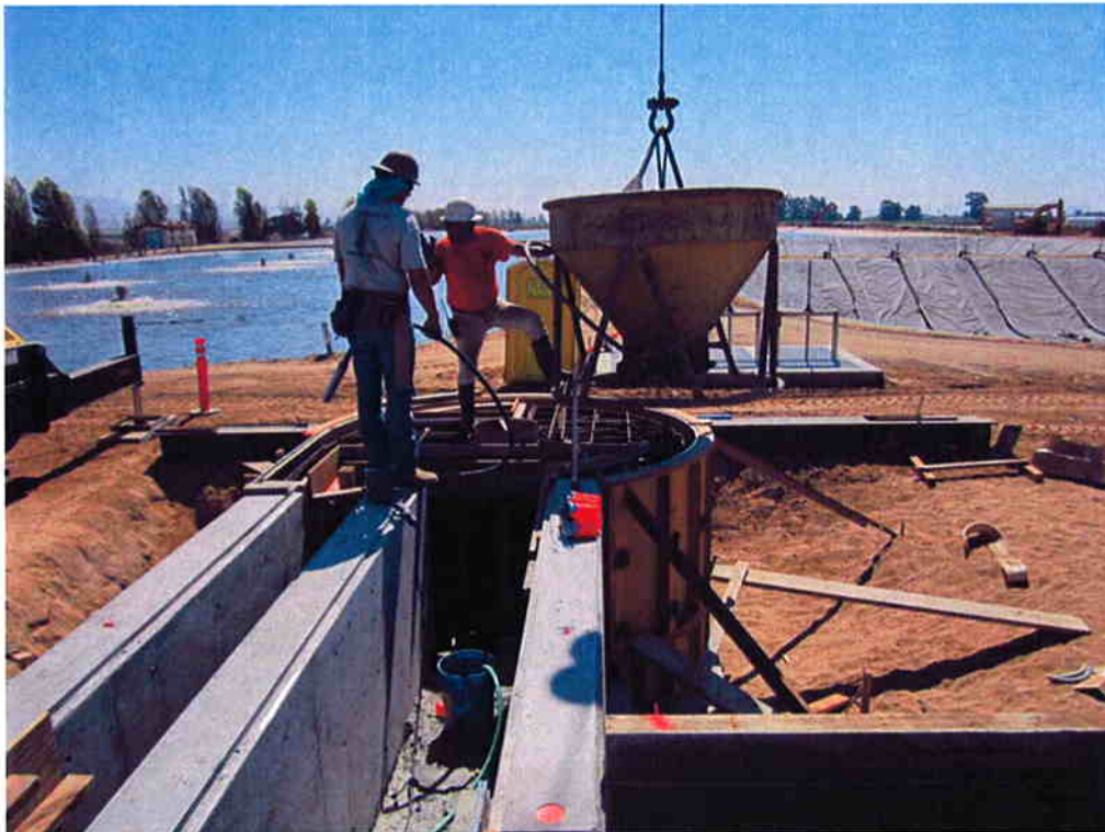
Cushman pouring the Grit Chamber structure.
