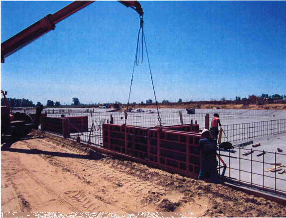
Cushman setting forms for intersections of divider walls at the Sludge Drying Beds.
