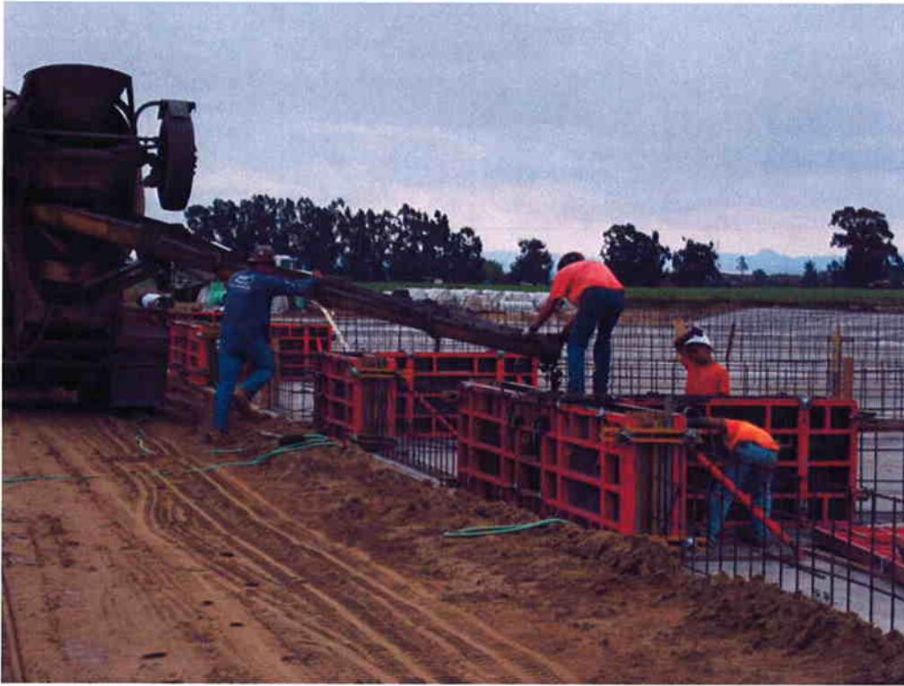
Cushman pouring divider wall intersections at Sludge Drying Beds.
