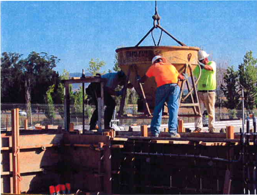
Cushman pouring channel walls to the Vortex Grit Tank.
