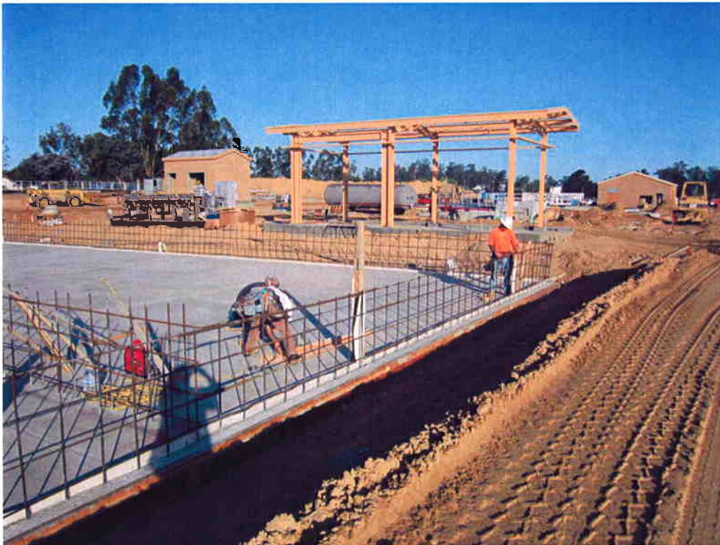
Cushman installing wall construction joints with water stop at Sludge Drying Bed #1.
