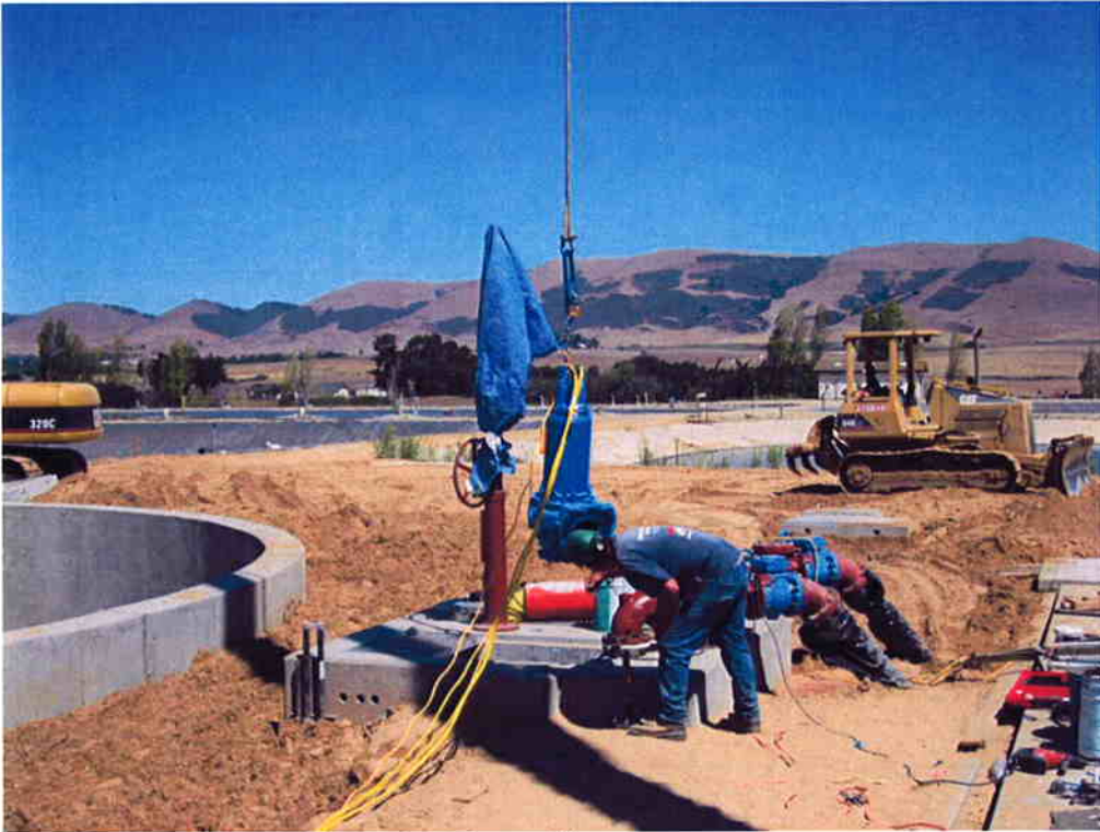
Cushman installing RAS/WAS Pump #1.
