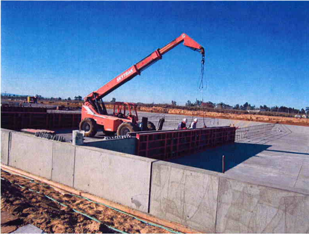
Cushman setting reusable forms for divider walls at the Sludge Drying Beds.
