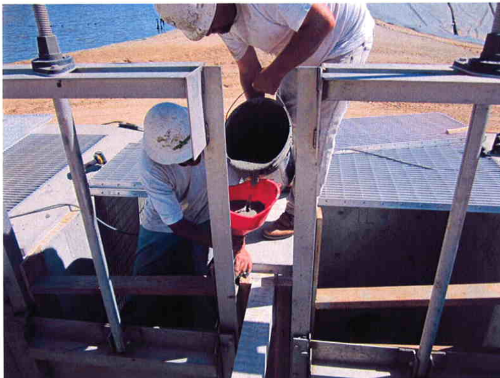
Cushman grouting the slide gates at Distribution Box #1.
