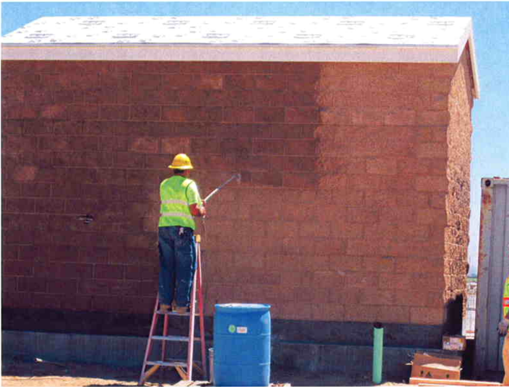
KNK Coating applying Bloc Seal to the outside of the Sodium Hypochlorite Storage Building for waterproofing.
