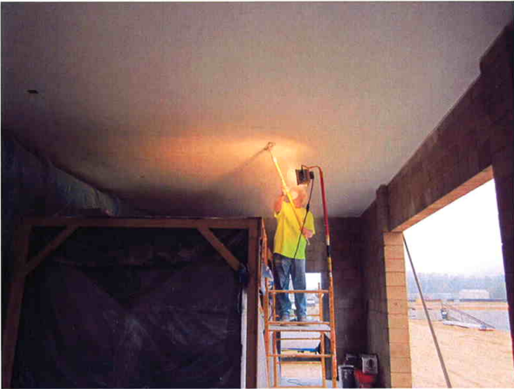
AIT sanding the smooth coating on the ceiling inside the Blower Room of the Electrical/Blower Building.
