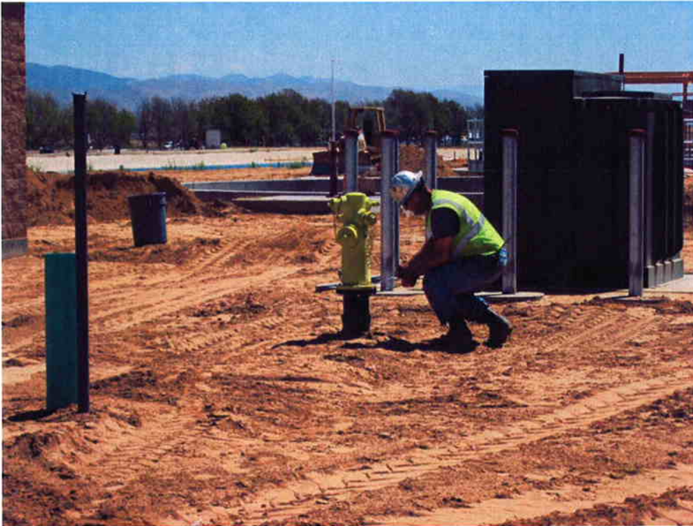
Cushman installing the fire hydrant near the Electrical/Blower Building.
