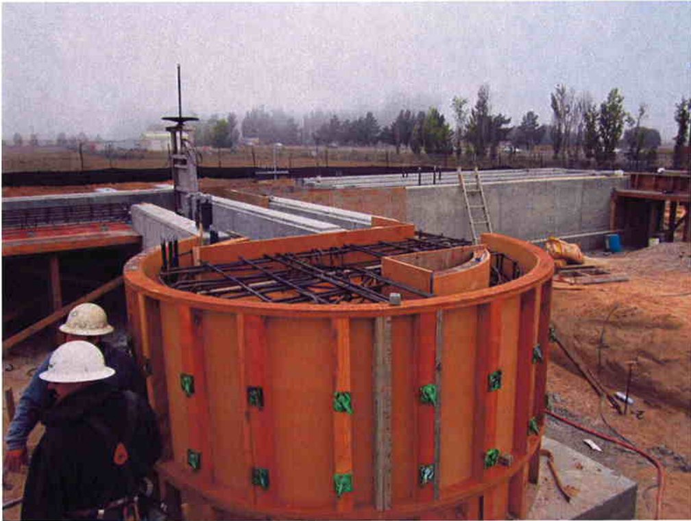
Completing forms for the Grit Chamber.
