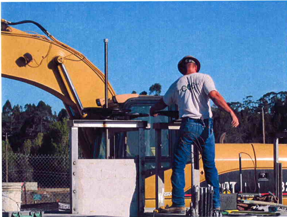
Cushman installing slide gate hand operators at the Headworks channels.
