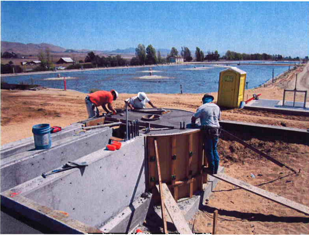
Cushman finishing the surface of the Grit Chamber.
