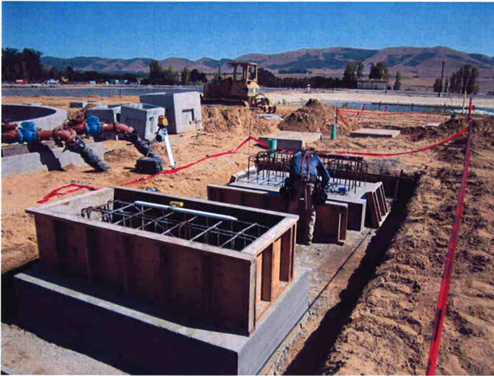
Cushman forming hydropneumatic tank supports.
