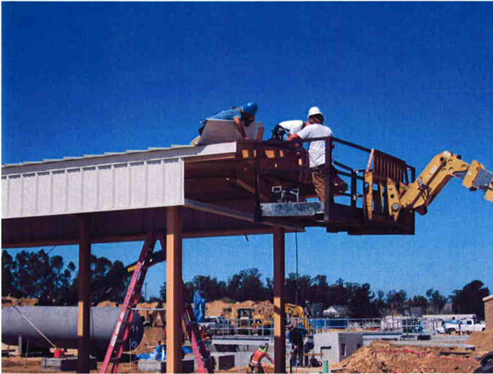
Dueck Roofing installing the shade canopy at the Sludge Thickening Building.
