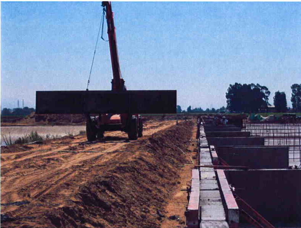
Cushman relocating reusable forms from the west wall concrete pours to the divider walls at the Sludge Drying Beds.
