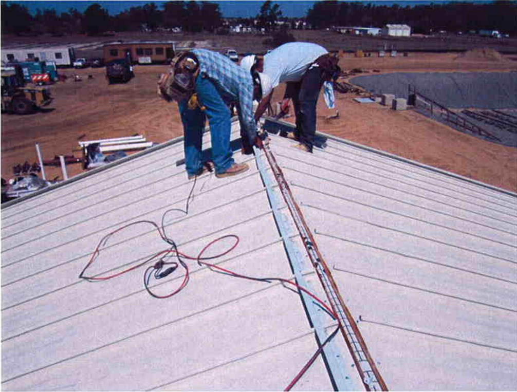
Dueck Roofing installing the ridge on the Electrical/Blower Building.
