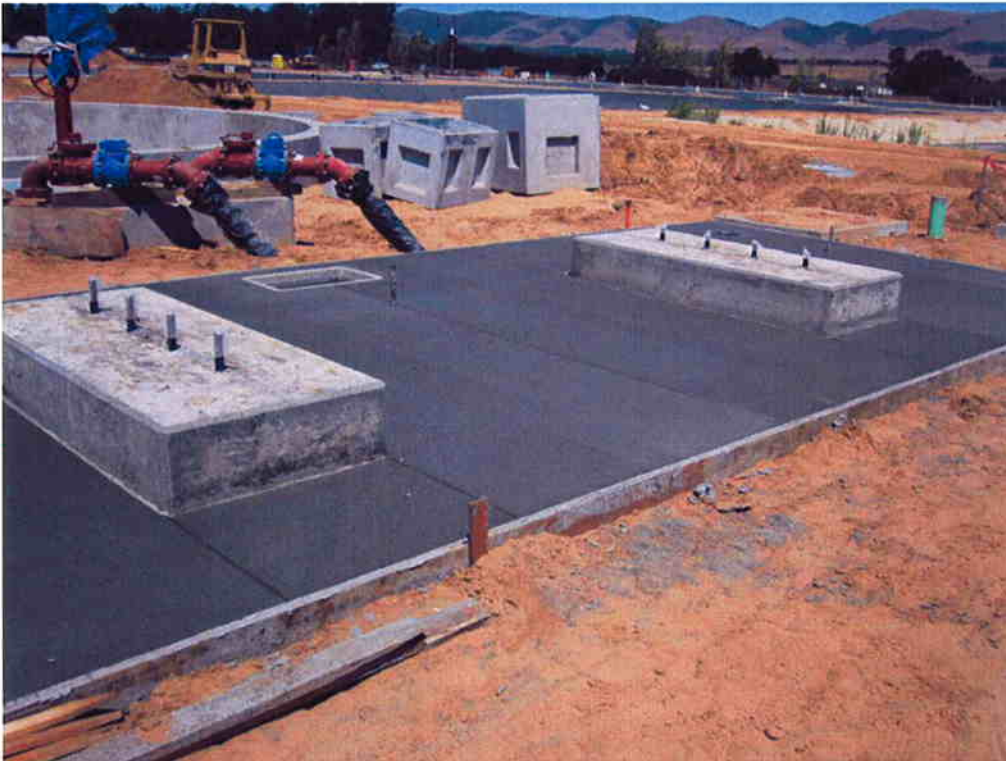
Hydropneumatic tank slab finished.
