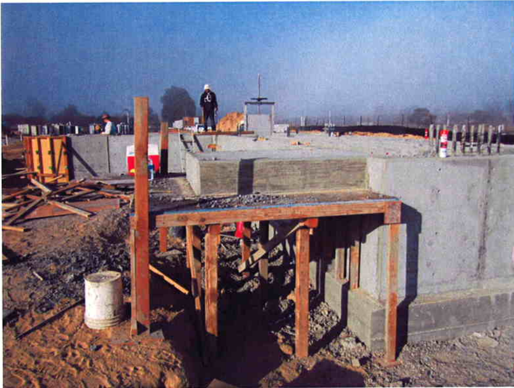
Cushman pouring stair landings at Headworks.
