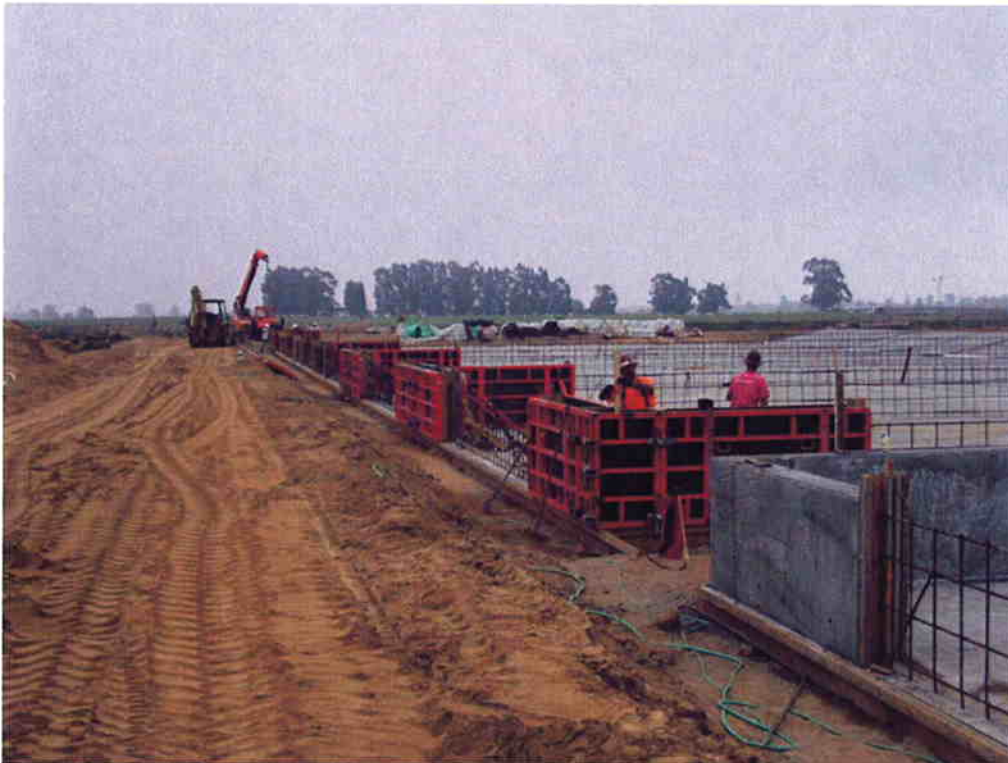
Cushman removing forms for divider wall intersections from the first pour and relocating and installing them for the next pour at the Sludge Drying Beds.
