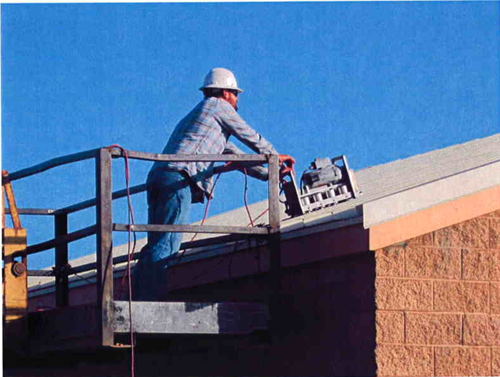
Dueck Roofing completing mechanical seam roof at Electrical/Blower Building.
