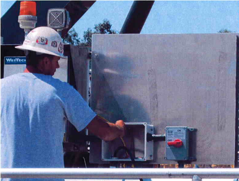
Bergelectric pulling wire to the local control panel at the clarifiers.
