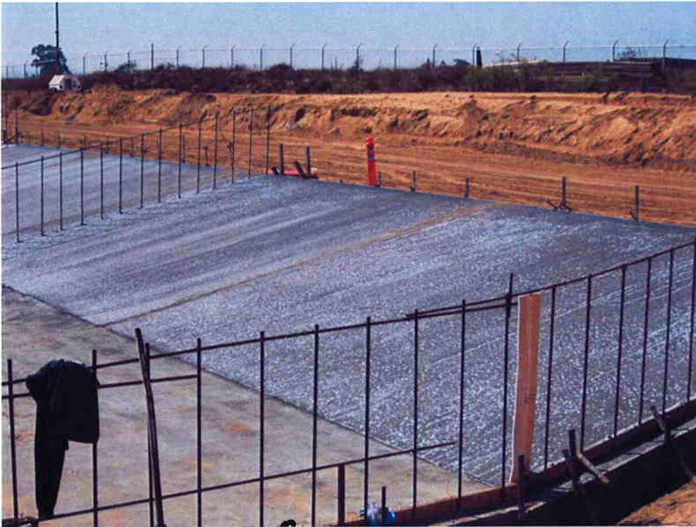
Sludge Drying Bed ramp pours complete and concrete cure applied.
