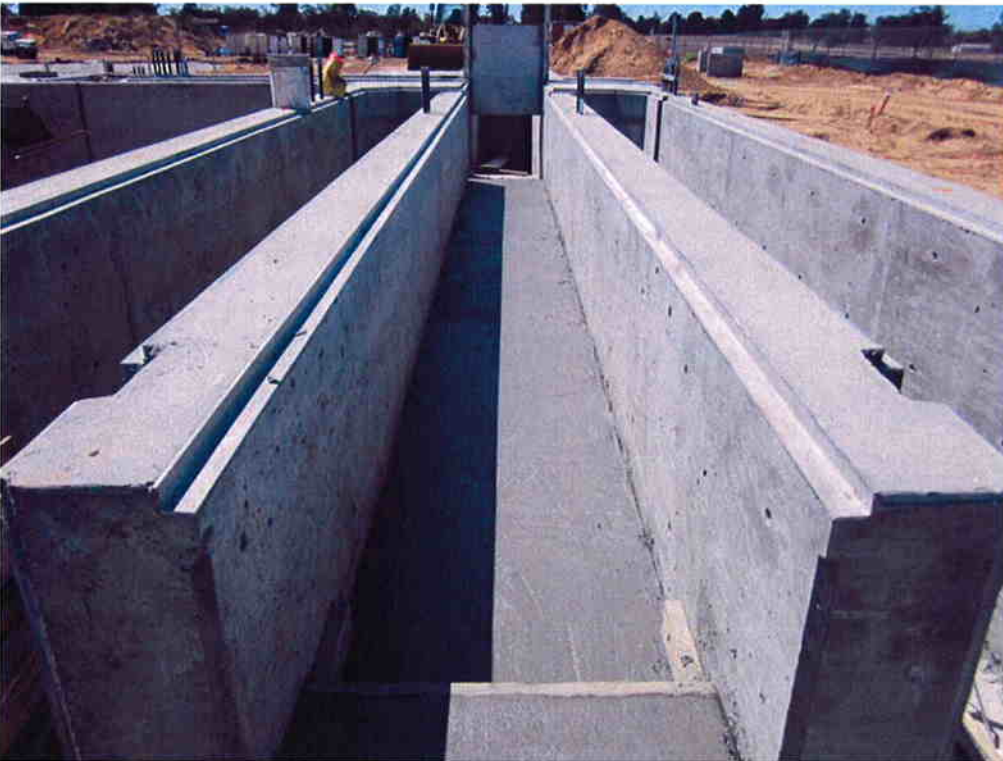
Concrete fill poured at the overflow channel of the Headworks.
