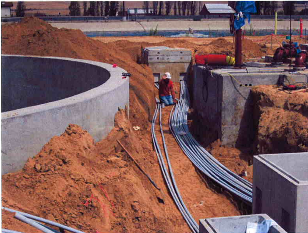
Bergelectric installing Duct Bank 12 (DB 12).
