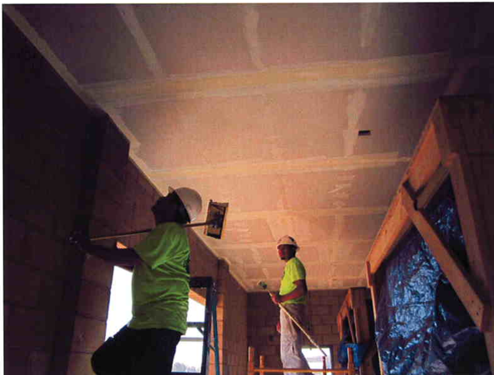
AIT taping drywall in the Blower Room at Electrical/Blower Building.
