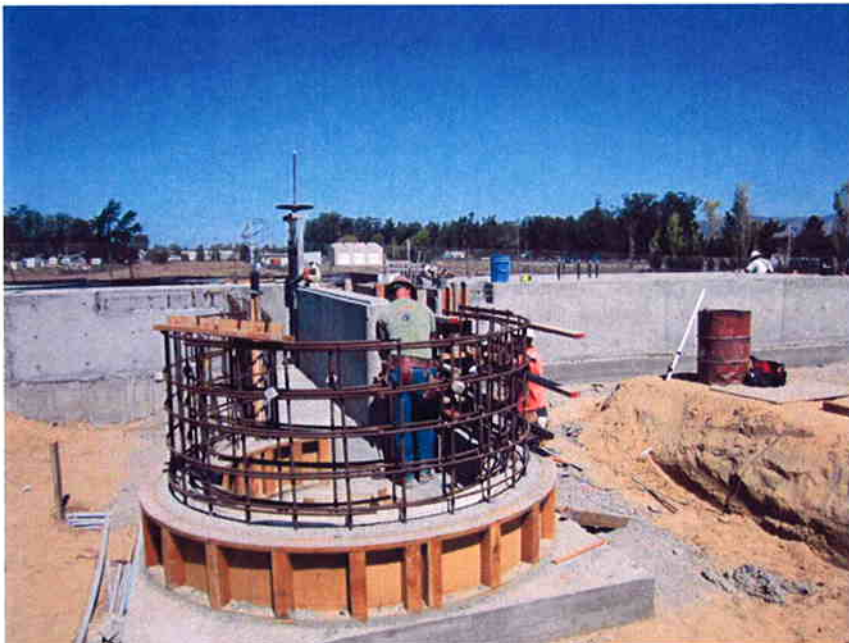
Cushman forming Grit Chamber walls.
