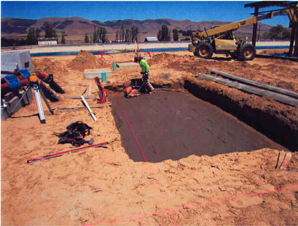
Cushman compacting base material under hydropneumatic tank foundation.
