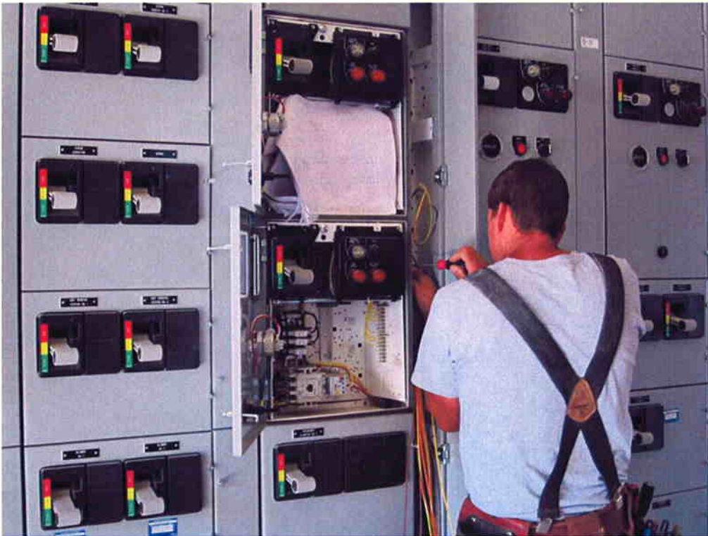
Bergelectric terminating clarifier wires at MCC room in Electrical/Blower Building.
