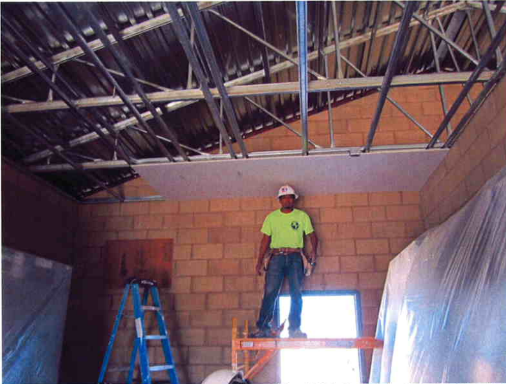
AIT installing sheet rock on the ceiling of the MCC Room in the Electrical/Blower Building.
