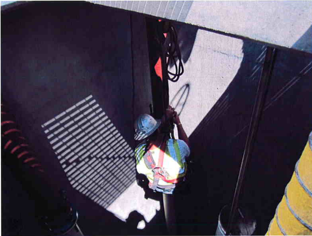
Cushman installing RAS/WAS piping inside RAS/WAS Pump Station #1.
