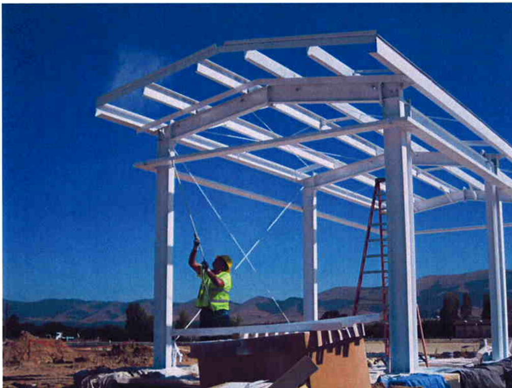
KNK Coating applying primer to the Sludge Thickening Building.
