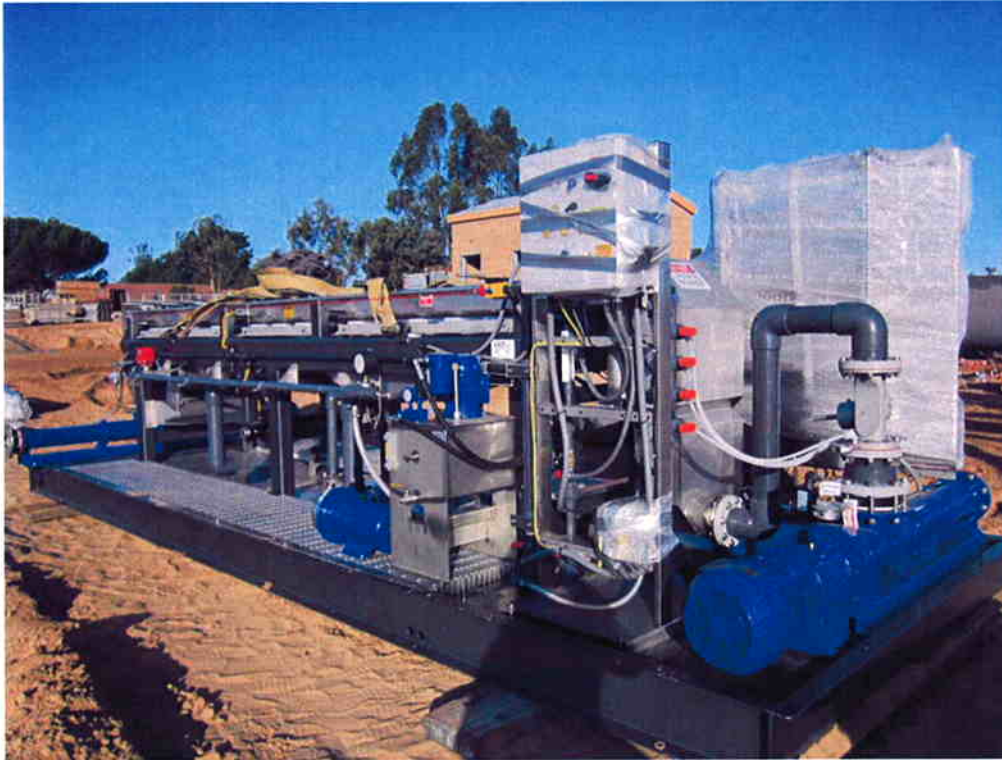
Sludge thickening equipment delivered to site.
