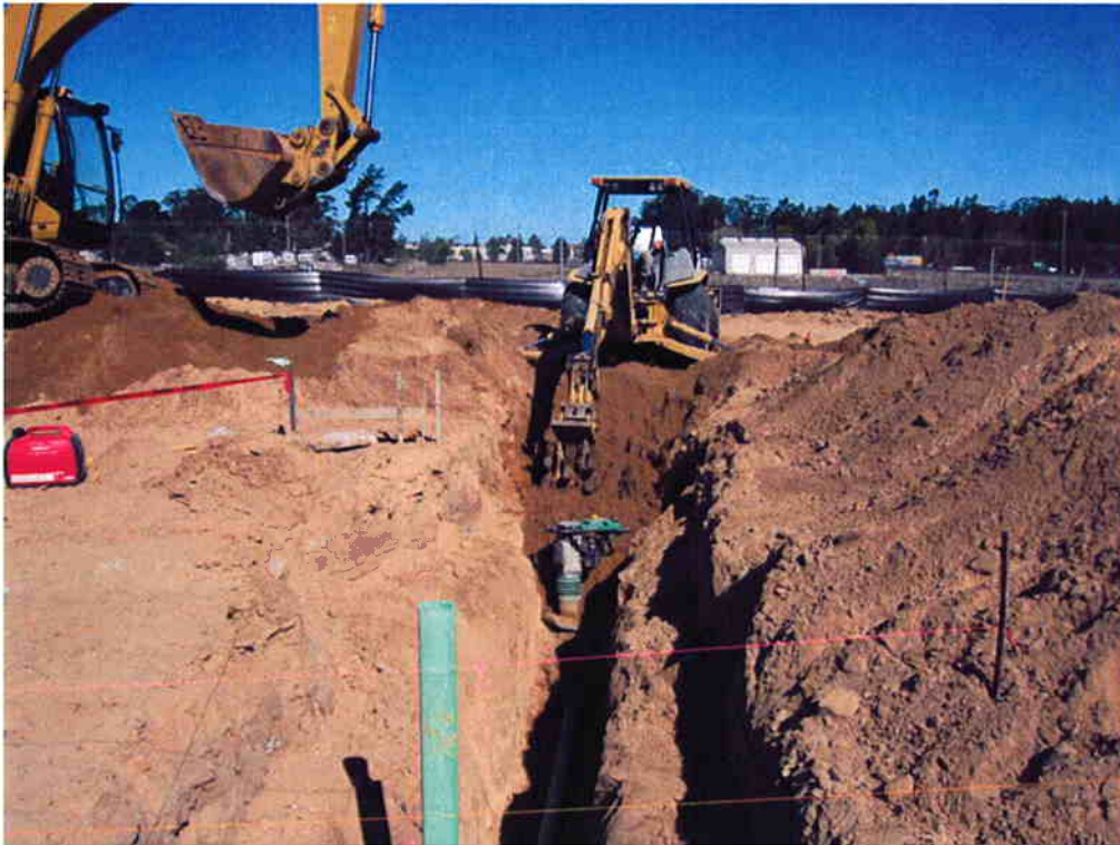
Cushman installing 4-inch DR piping along the Grit Classifier.
