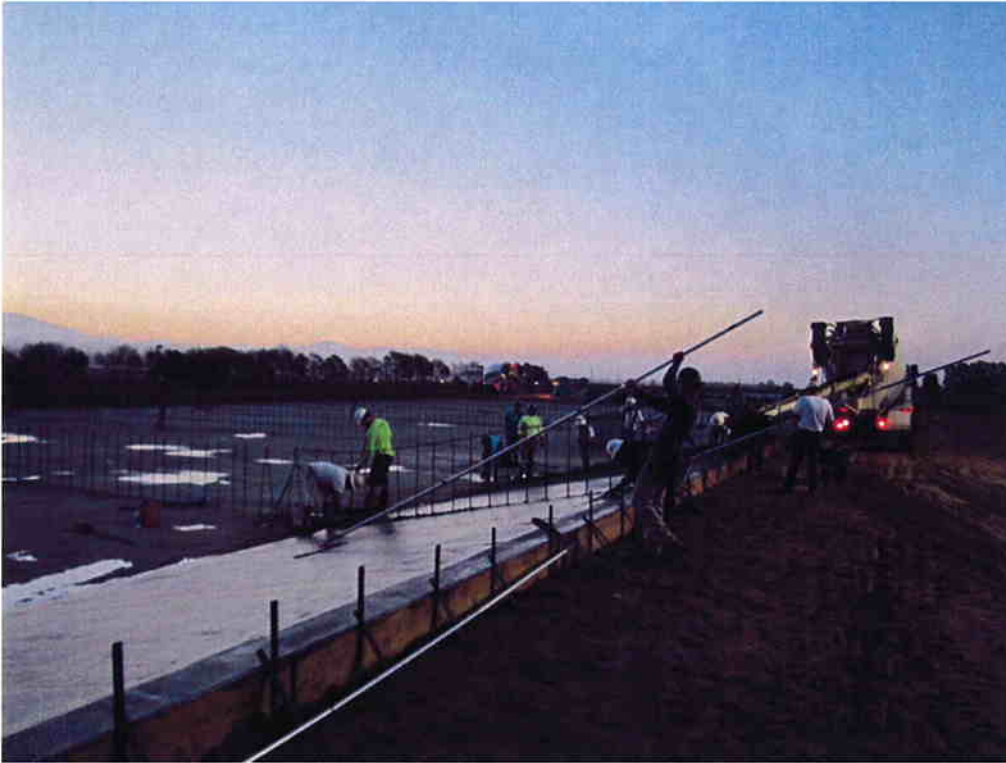
Cushman completing concrete pours of the ramps to the Sludge Drying Beds.
