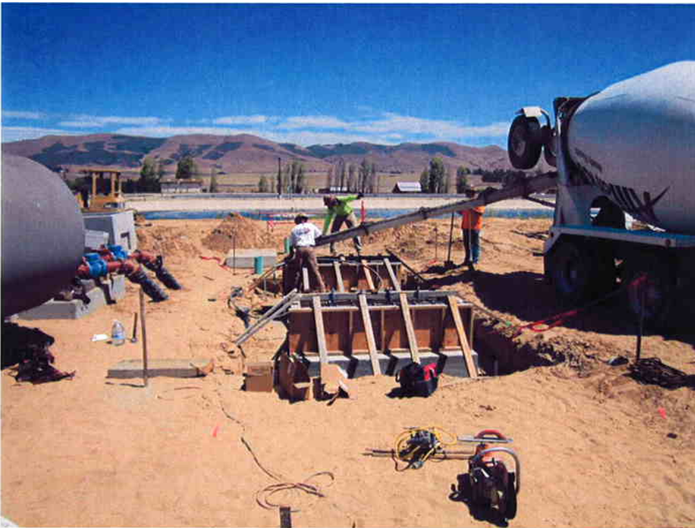
Cushman pouring the hydropneumatic tank supports.
