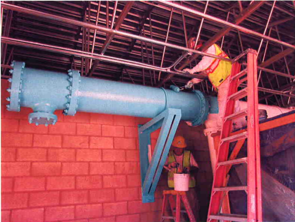
KNK Coating putting finish coat on AR piping in Blower Room of Electrical/Blower Building.
