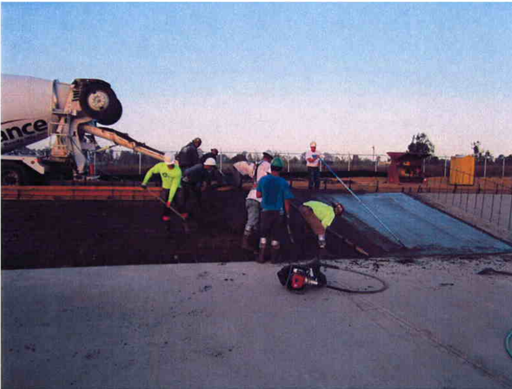
Cushman making final pour of the ramps for the Sludge Drying Beds.
