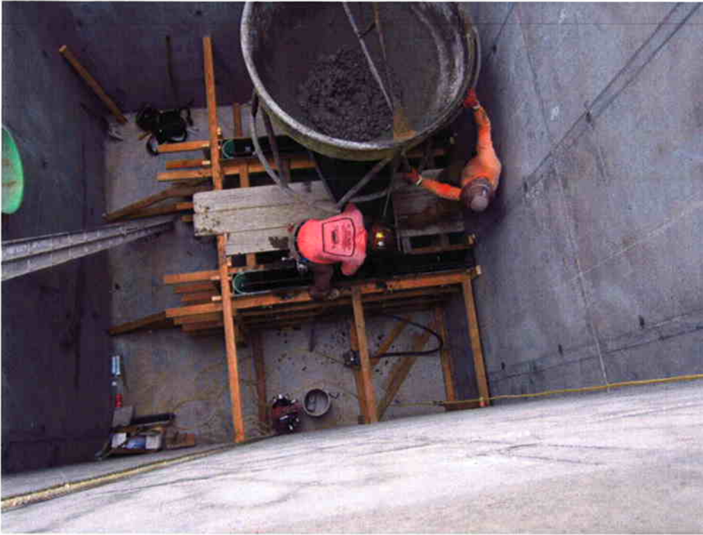
Pouring the dividing walls for the prerotation basins in the Influent Pump Station.
