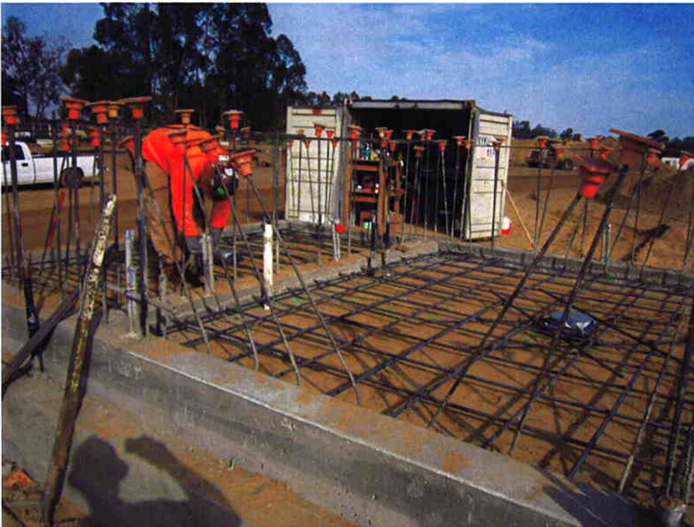
CMC Rebar tying reinforcement for slab at Sodium Hypochlorite Building.
