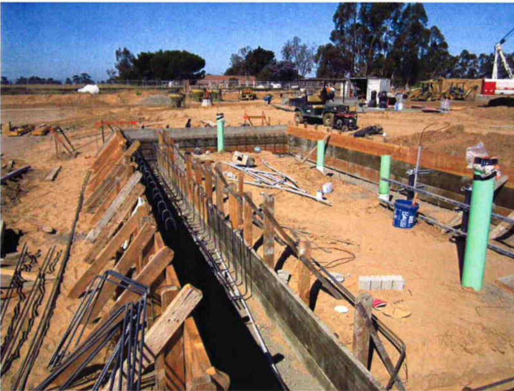
Reinforcement installation for the Sludge Thickening System footing.
