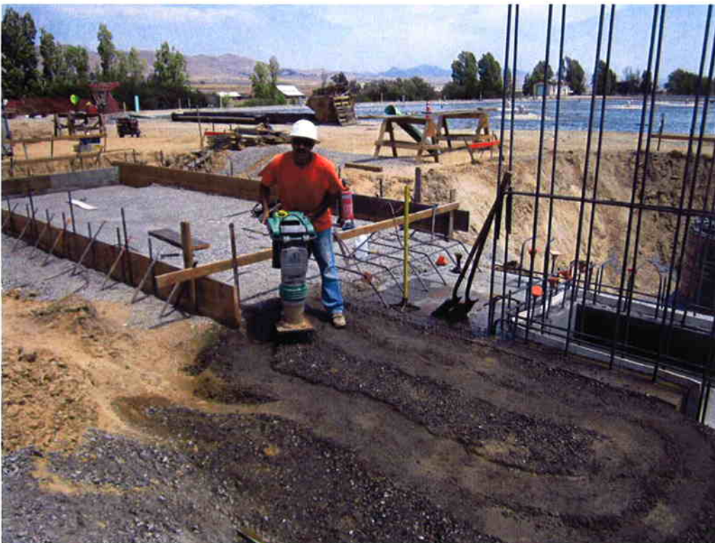
Compacting base under the upper headworks.
