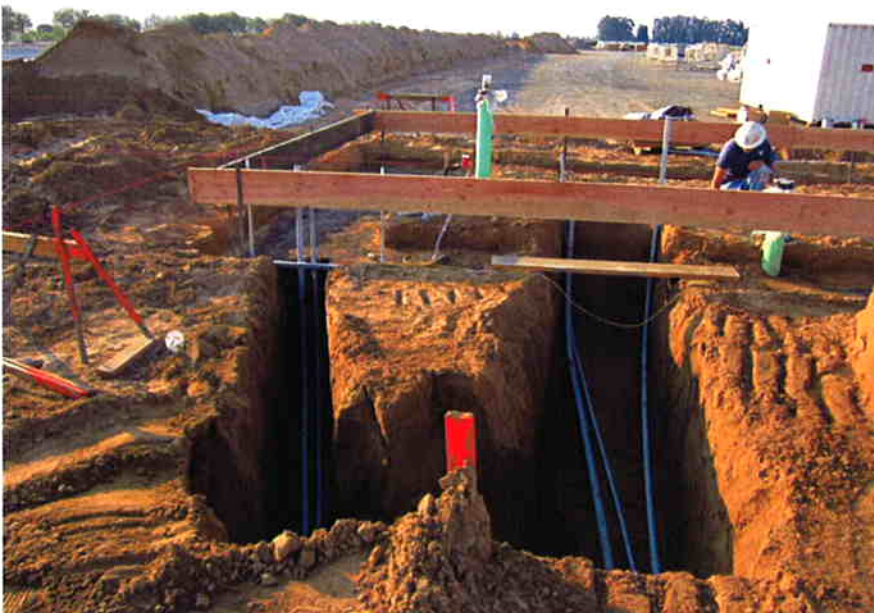
Bergelectric installing conduits under the foundation at Sludge Thickening System.
