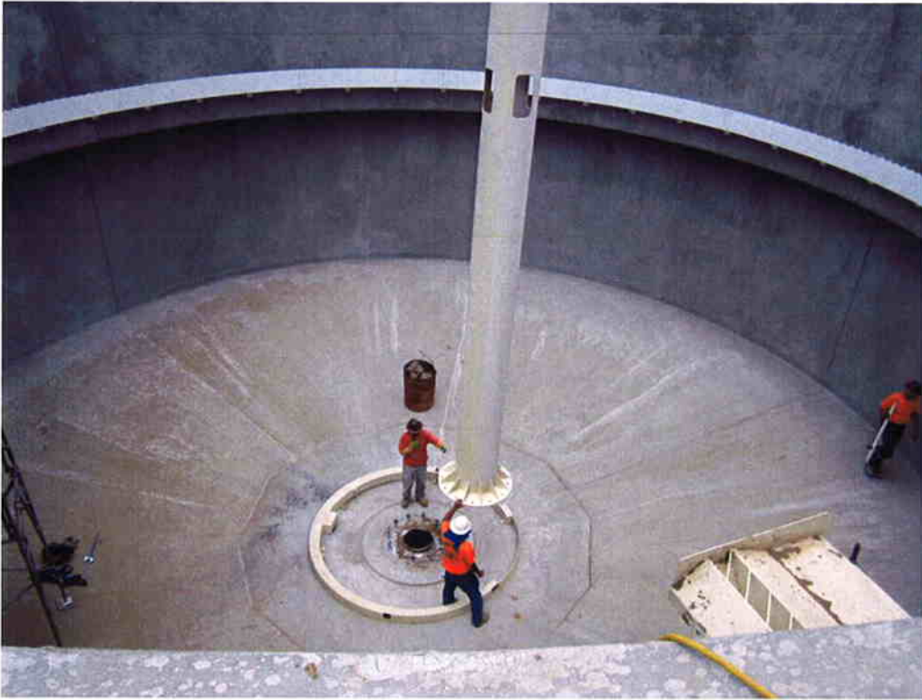
Installing center column inside Clarifier #2.
