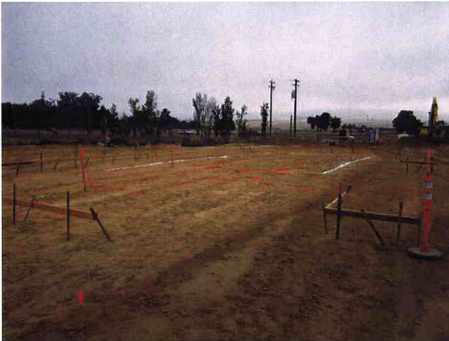
Laying out the headworks and grit removal system.
