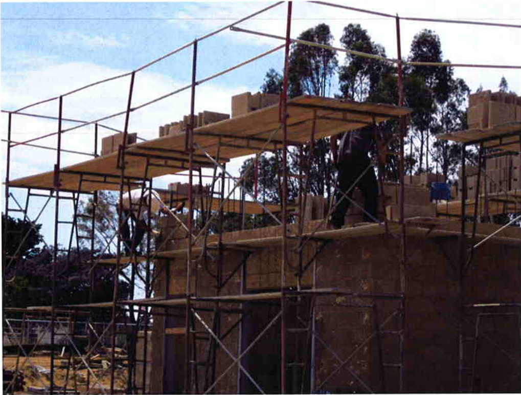
Building corner leads at the Sodium Hypochlorite Building.
