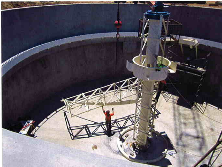
Installing mechanisms inside Clarifier #1.
