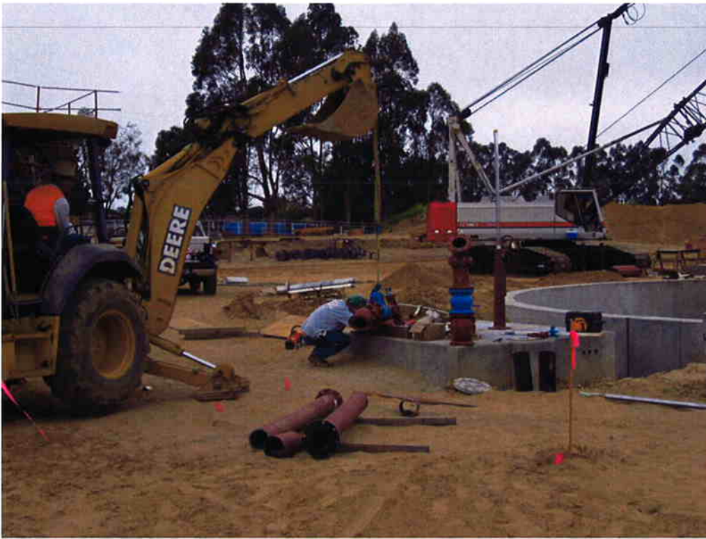
Cushman installing piping at RAS/WAS Pump Station #1.
