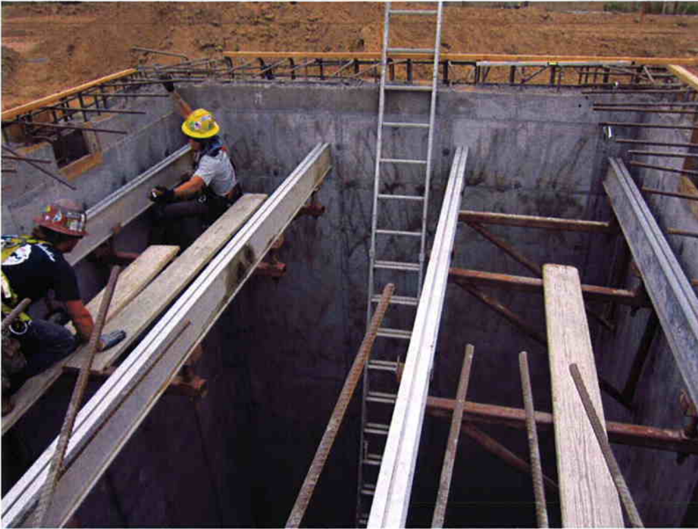
Installing supports for shoring to prepare for deck pour at Influent Pump Station.
