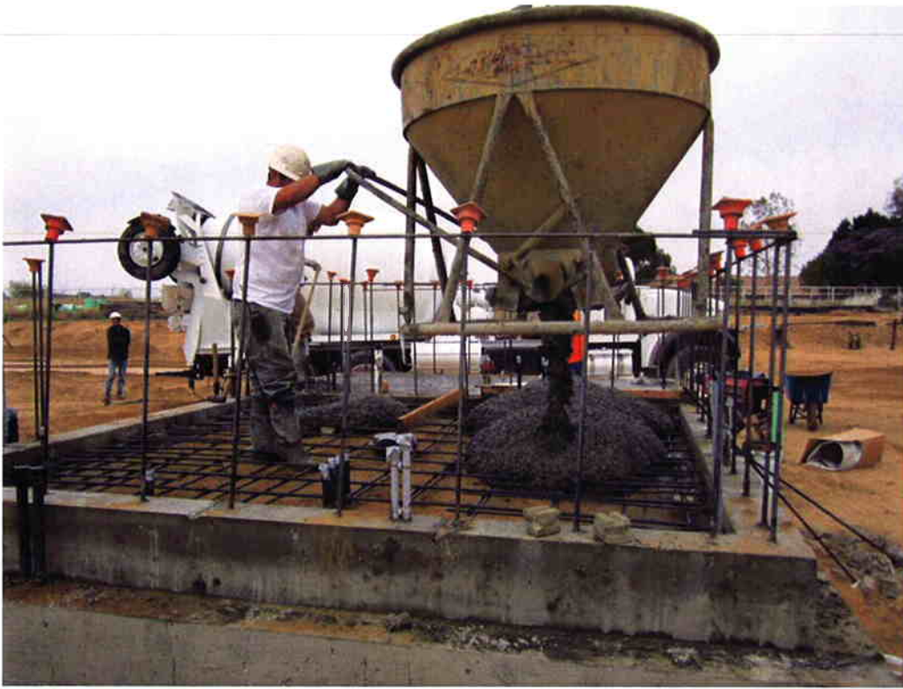
Pouring slab of the Sodium Hypochlorite Building.
