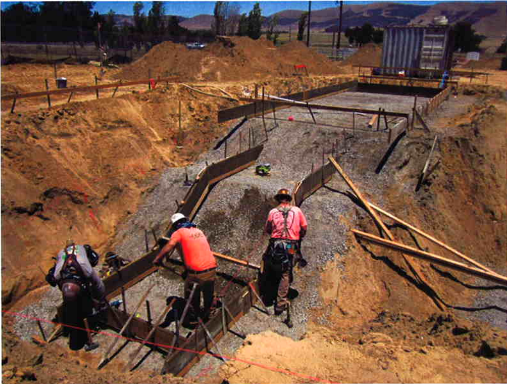
Forming lower level of headworks.
