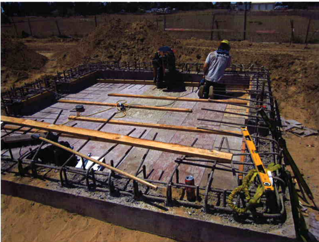
Setting shoring for pouring the deck of the Influent Pump Station.
