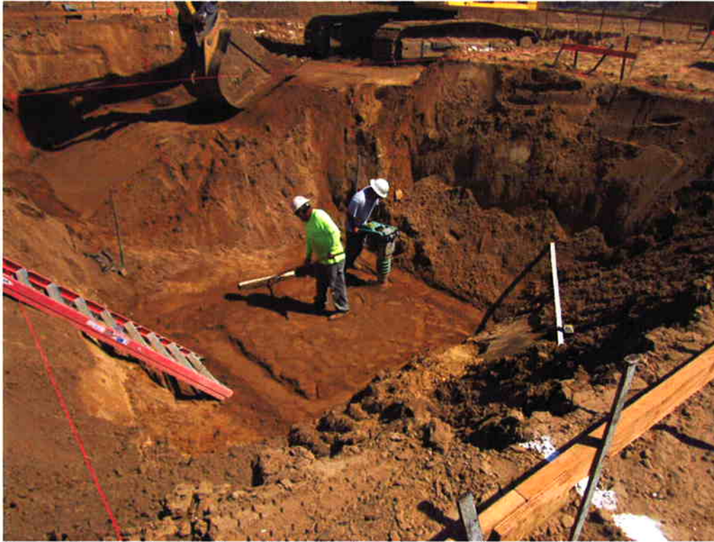
Excavating for the headworks and grit removal system.
