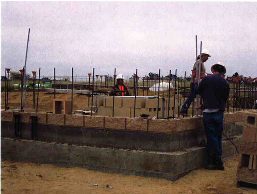
Beinscroth Masonry placing first course of block at the Sodium Hypochlorite Building and Bergelectric installing conduit running through the walls.
