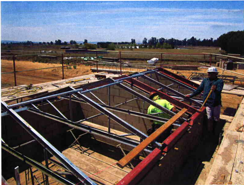
Cushman installing the metal roof trusses at the Sodium Hypochlorite Building.
