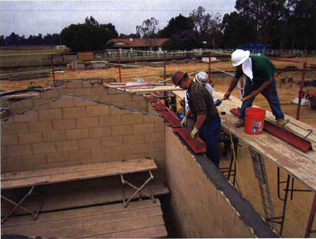
Cushman setting steel channels at Sodium Hypochlorite Building.
