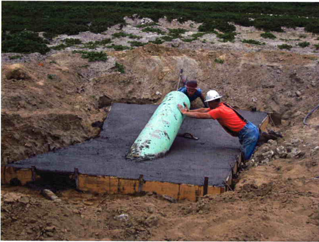
Pouring the inlet structure slab at Pond 1.
