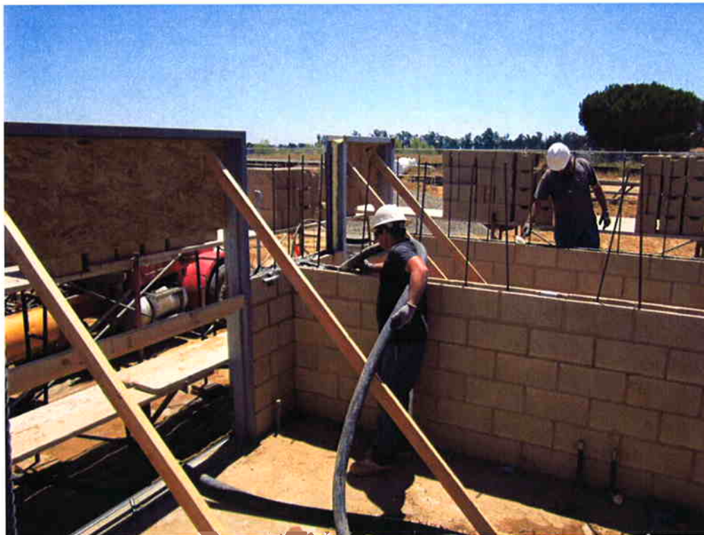
First grout pour at the Sodium Hypochlorite Building.
