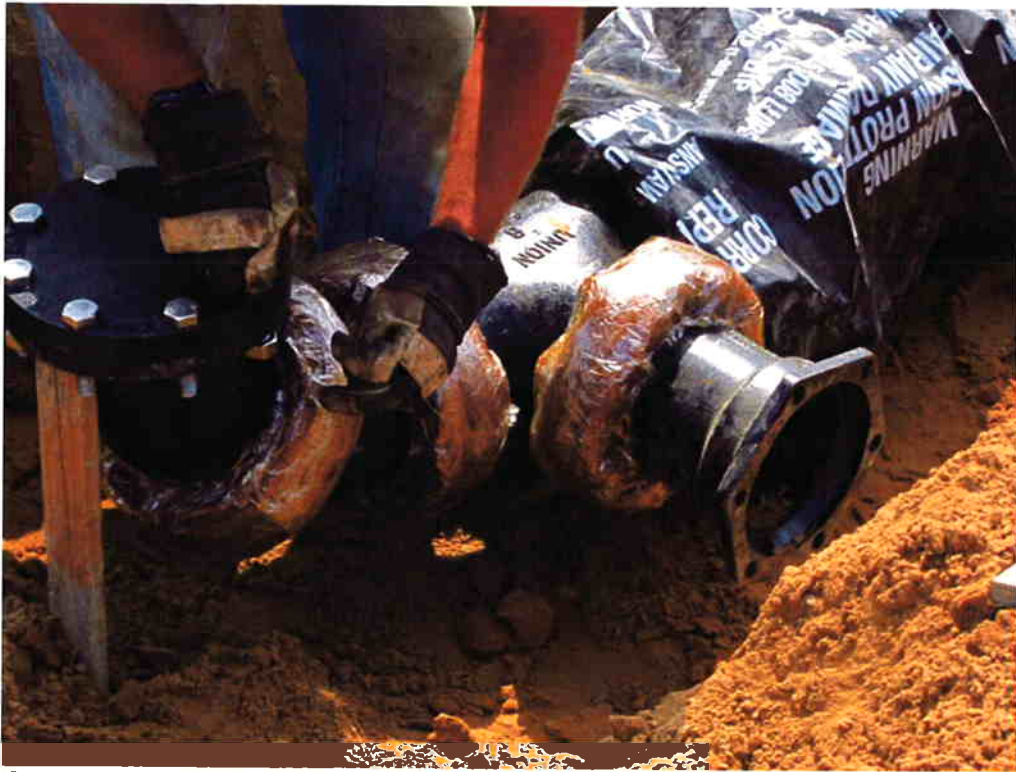
Cushman installing fittings on the 6-inch TWAS pipe.
