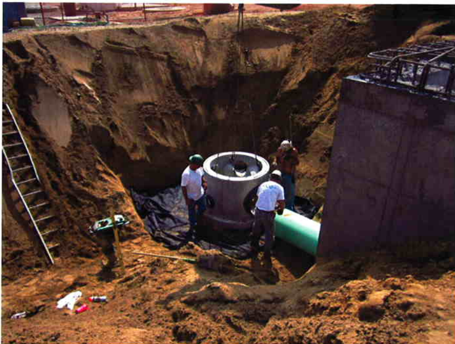
Cushman setting Manhole #1 and connecting piping to the Influent Pump Station.
