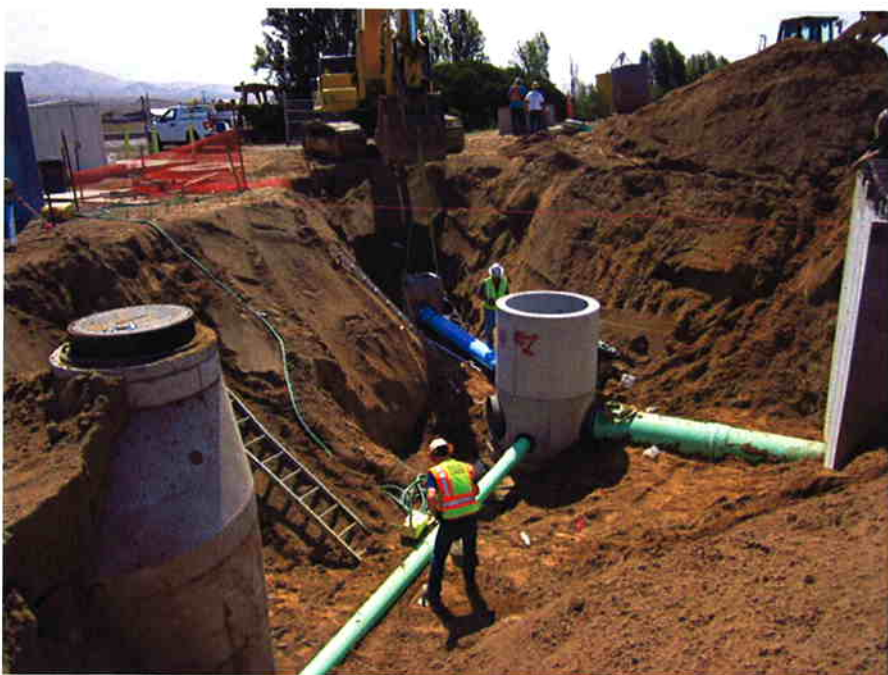
Cushman installing Manhole #1 and piping.
