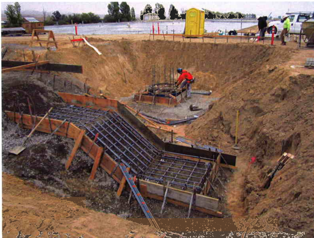
Reinforcing being installed at lower headworks and grit removal chamber.
