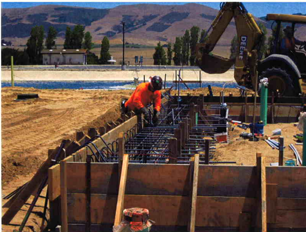
Tying more reinforcing in the footing for the Sludge Thickening System.
