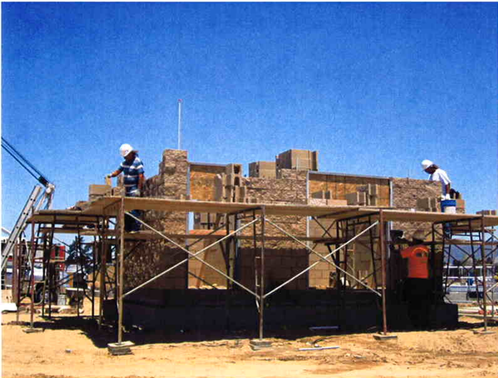
Beinscroth Masonry placing CMU at Sodium Hypochlorite Building.
