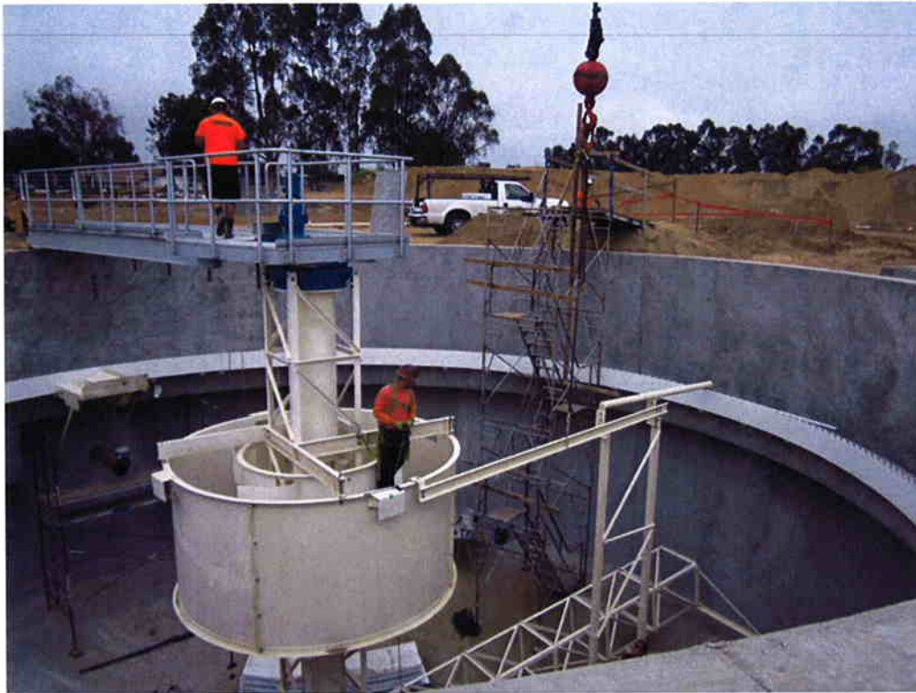
Installing mechanisms inside Clarifier #2.
