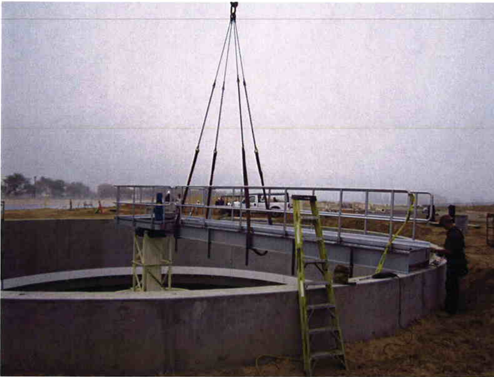
Installing the bridge for Clarifier #1.
