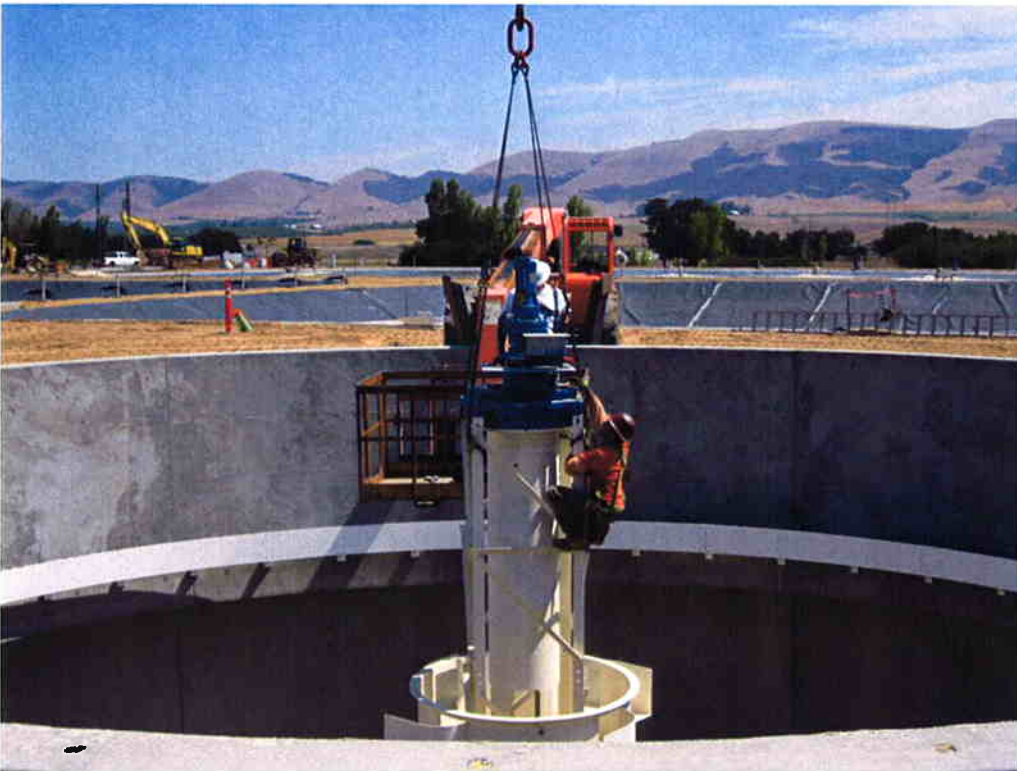
Installing motor for mechanisms inside Clarifier #2.
