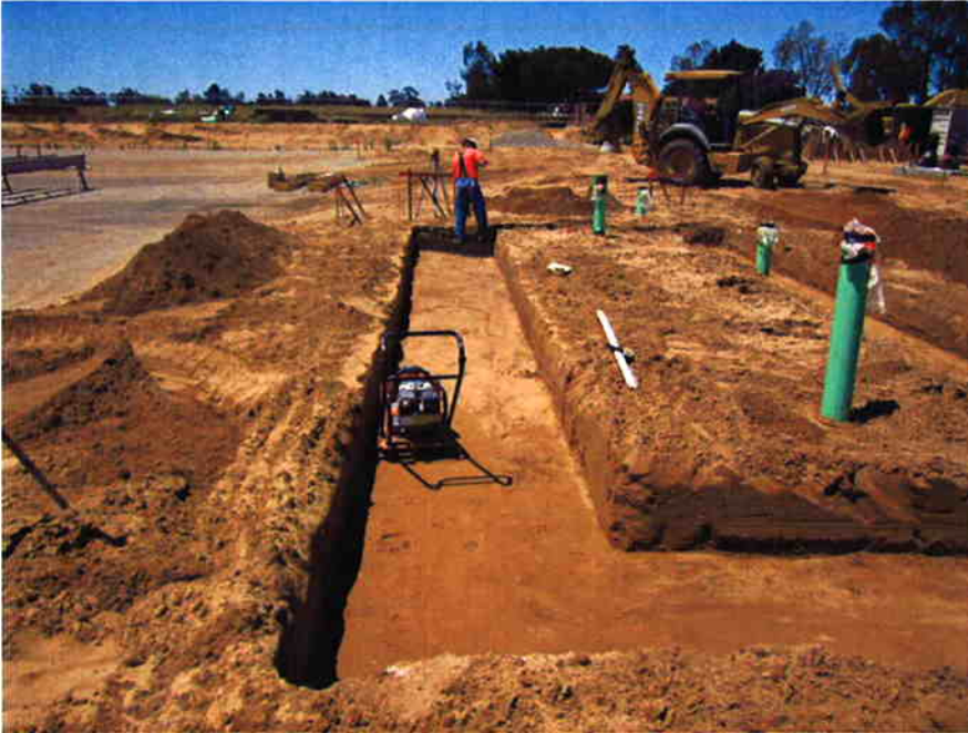
Cushman installing base at for footing at Sludge Thickening System.
