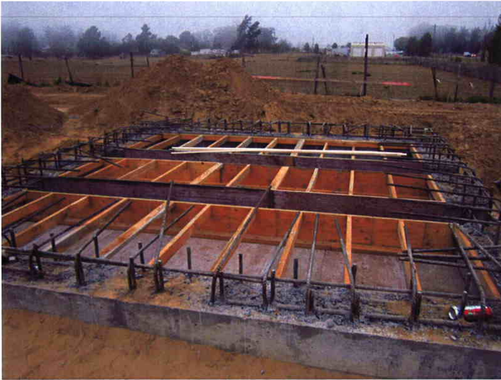
Forming deck of Influent Pump Station.
