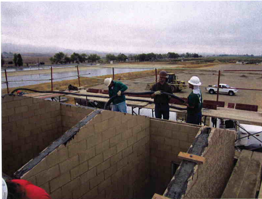
Last grout pour at Sodium Hypochlorite Building.
