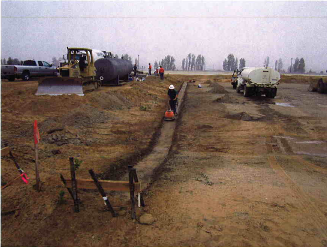
Cushman excavating and compacting the wall line along Sludge Drying Bed #1.
