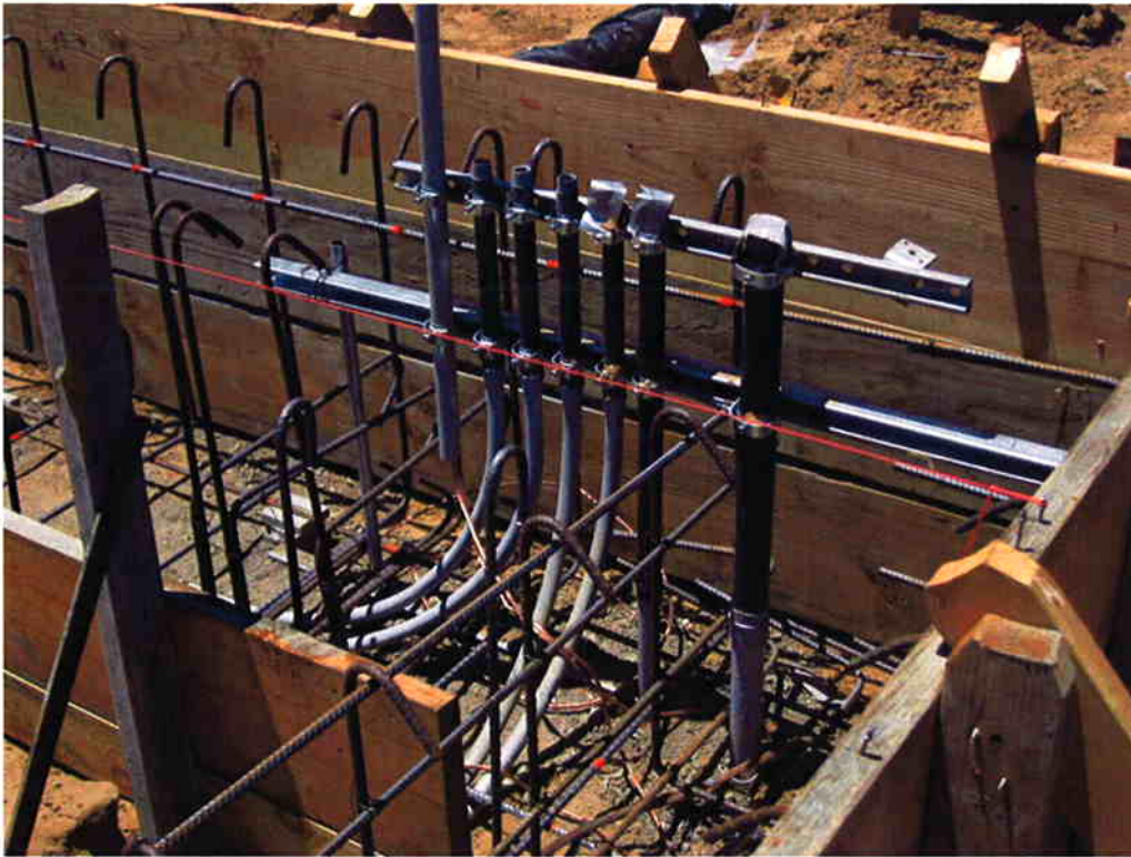
Underground conduit installed in the Sludge Thickening System footing.
