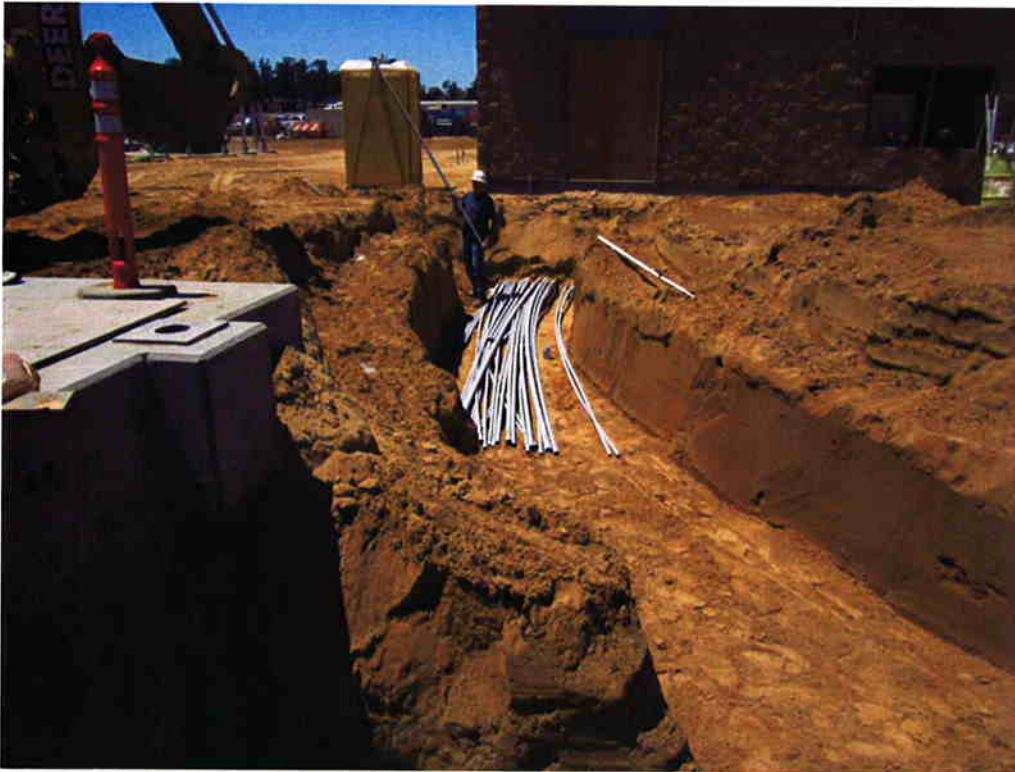
Bergelectric installing Duct Bank #25 from the Electrical/Blower Building.
