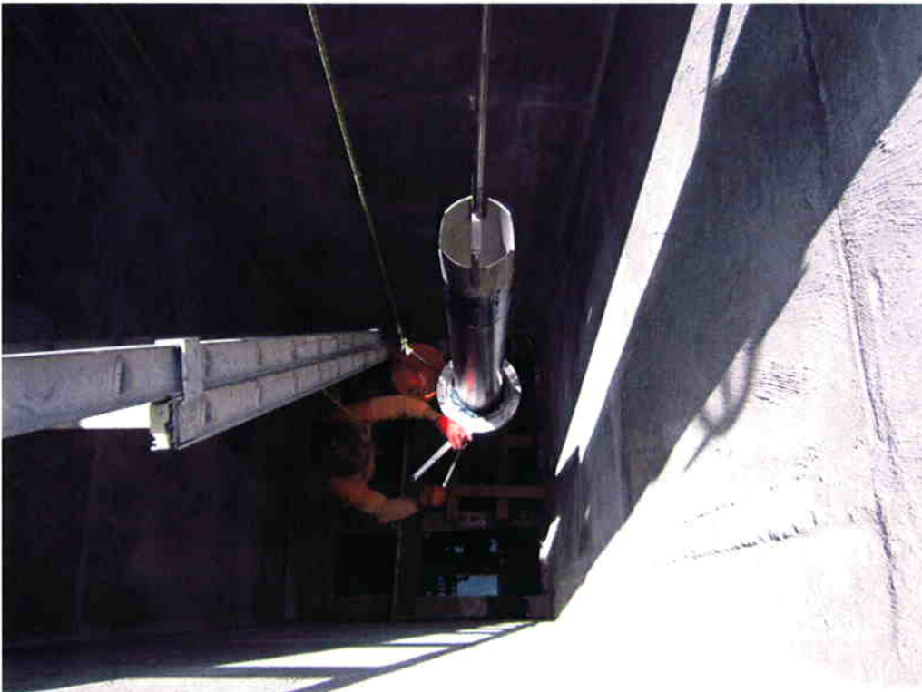
Cushman installing the telescoping valve inside RAS/WAS Pump Station #1.
