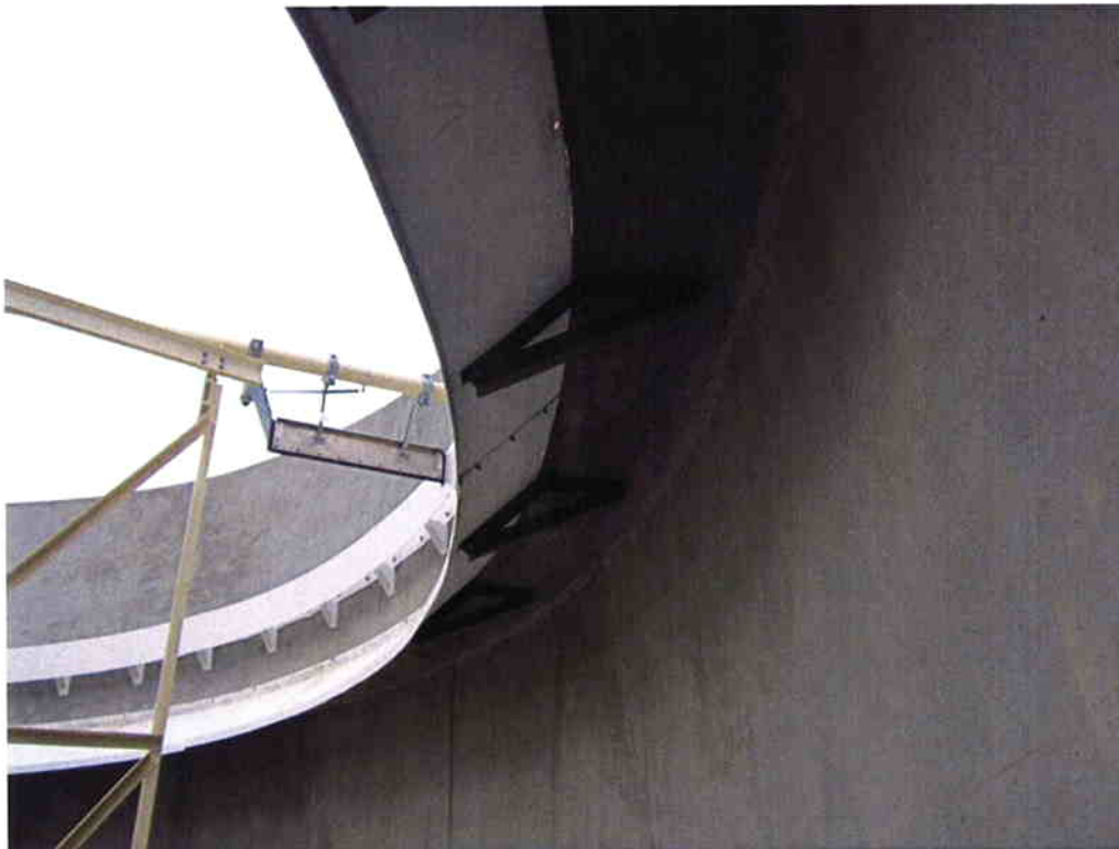
Installing the peripheral baffle inside Clarifier #2.
