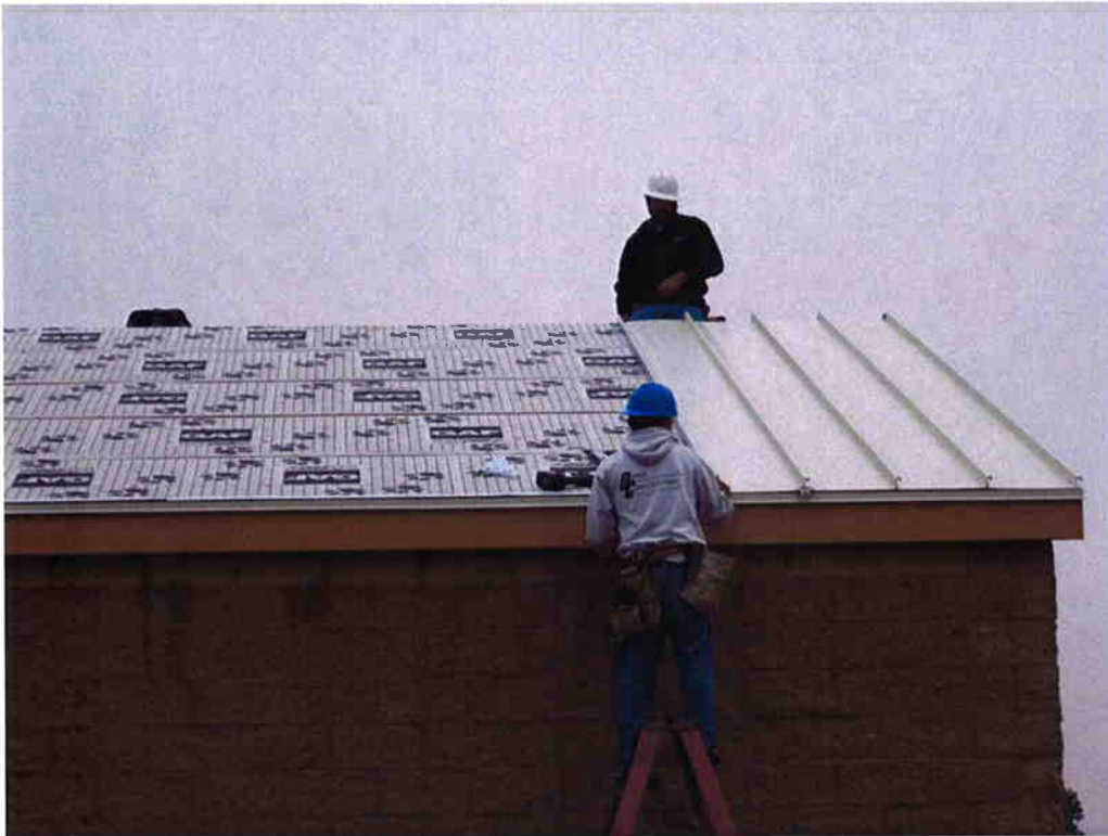
Subcontractor Dueck Roofing installing standing seam roof on Electrical/Blower Building.
