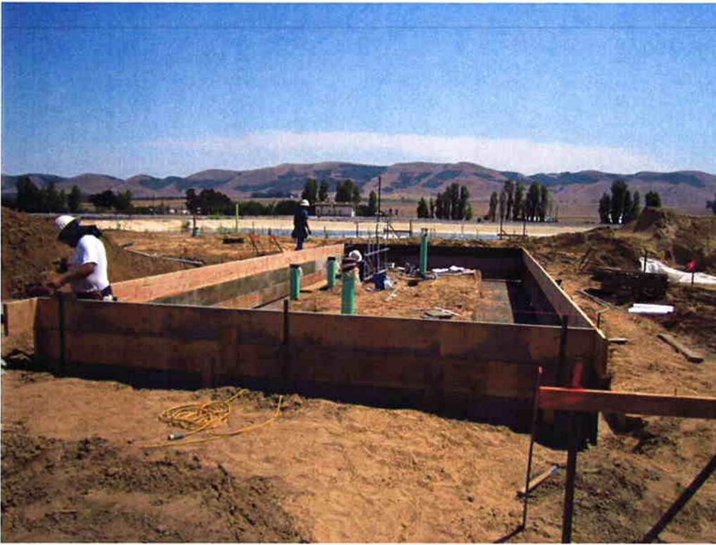
Cushman forming footing for the Sludge Thickening System.
