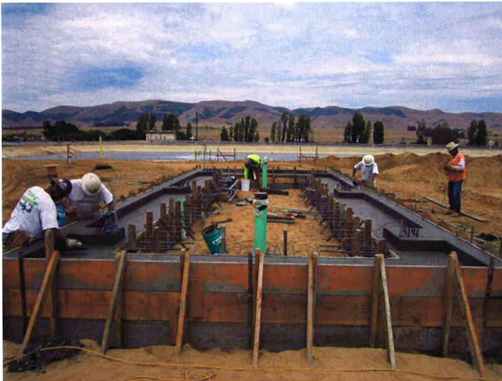
Cushman finishing the footing for the Sludge Thickening System.
