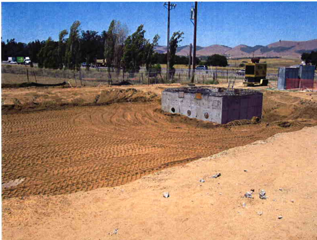
Backfilling around Influent Pump Station.
