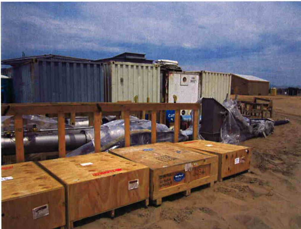
Receipt of screw conveyor and grit classifier.
