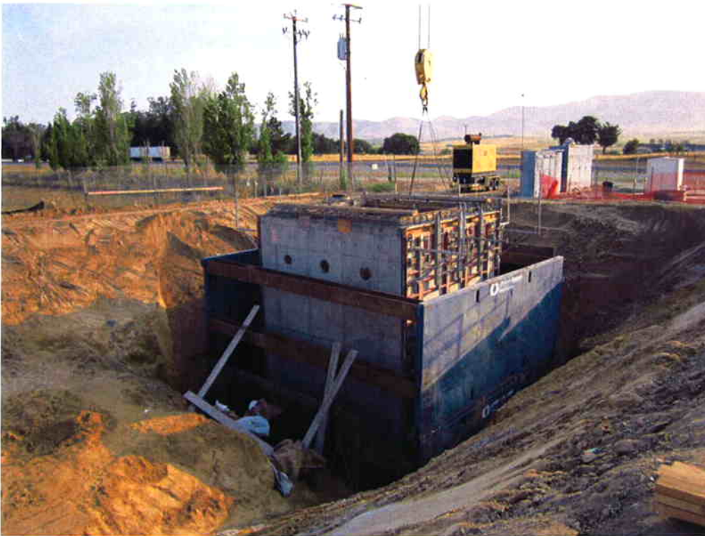
Stripping forms at the Influent Pump Station after the wall pour.
