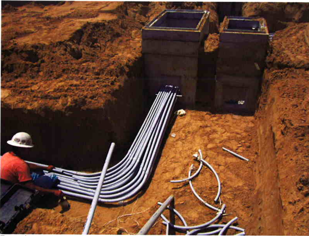
Bergelectric installing Duct Bank #22.
