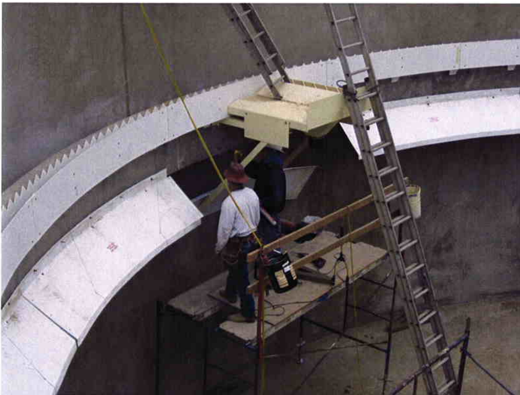
Installing the peripheral baffle inside Clarifier #1.
