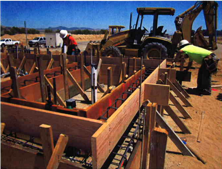
Cushman forming the starter wall for Sodium Hypochlorite Building.
