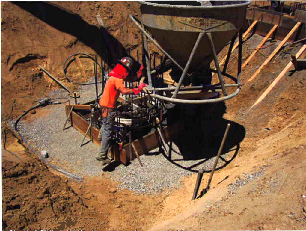
Pouring the foundation for the grit removal system.
