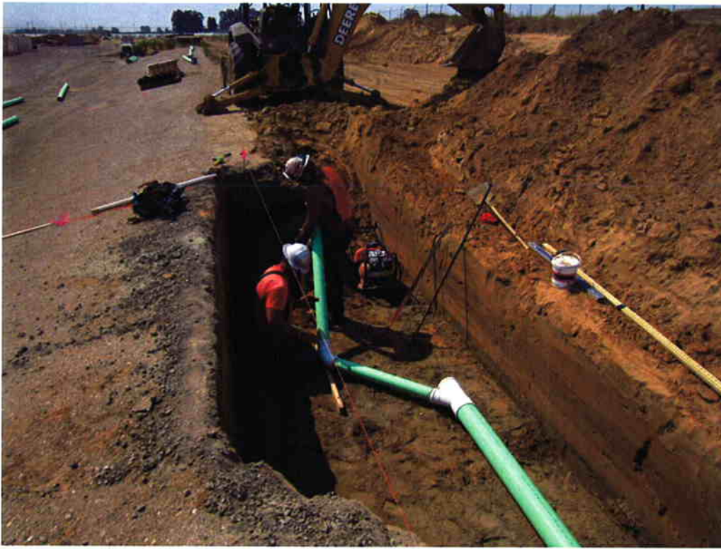
Cushman installing the 6-inch TWAS west of the Sludge Drying Beds.
