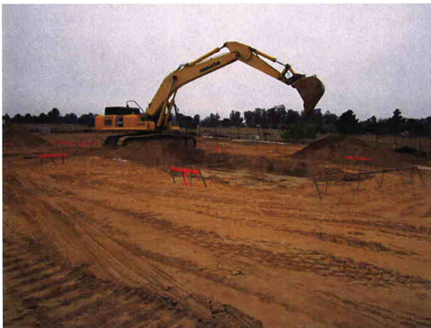
Excavating for headworks and grit removal system.
