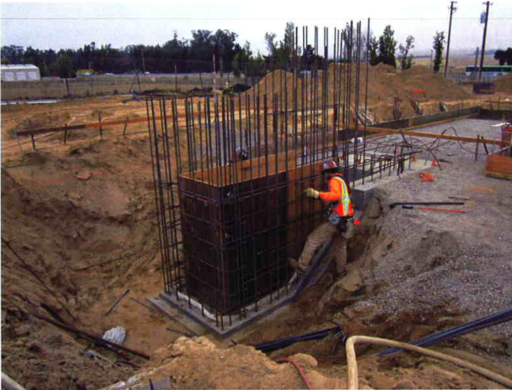
Forming the walls for the lower headworks.
