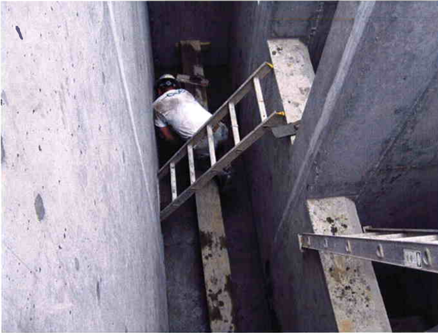
Cushman placing concrete fill inside Distribution Box #2.
