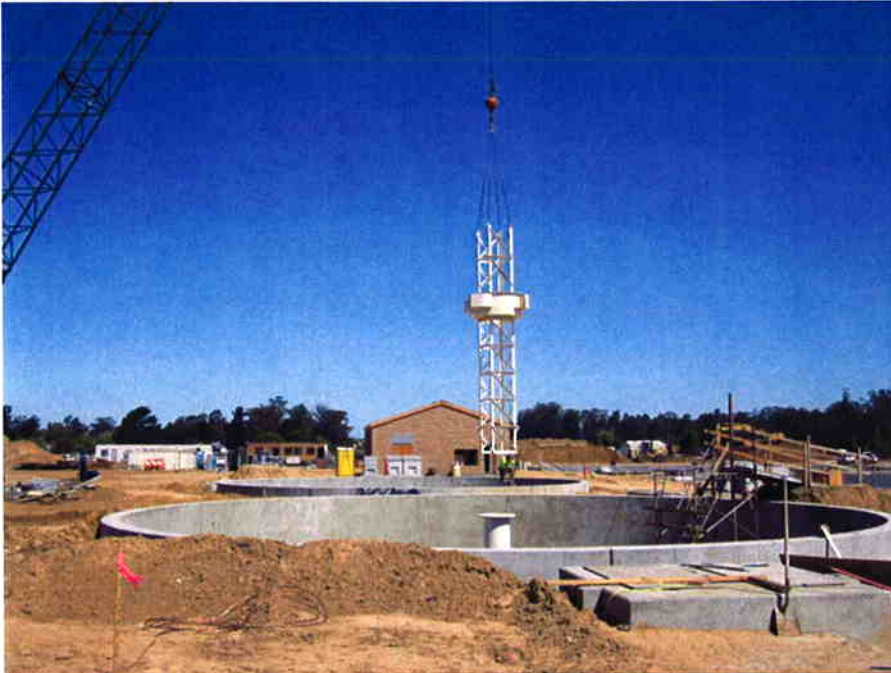
Installing mechanisms inside Clarifier #1.
