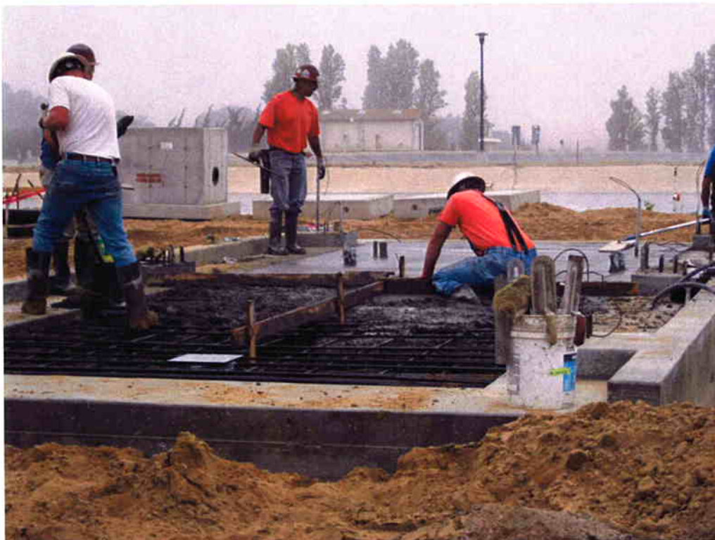
Cushman pouring concrete for Sludge Thickening slab.
