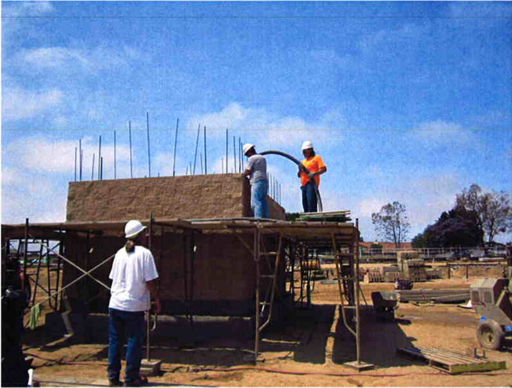
Installing reinforcing and pouring grout at the Sodium Hypochlorite Building.
