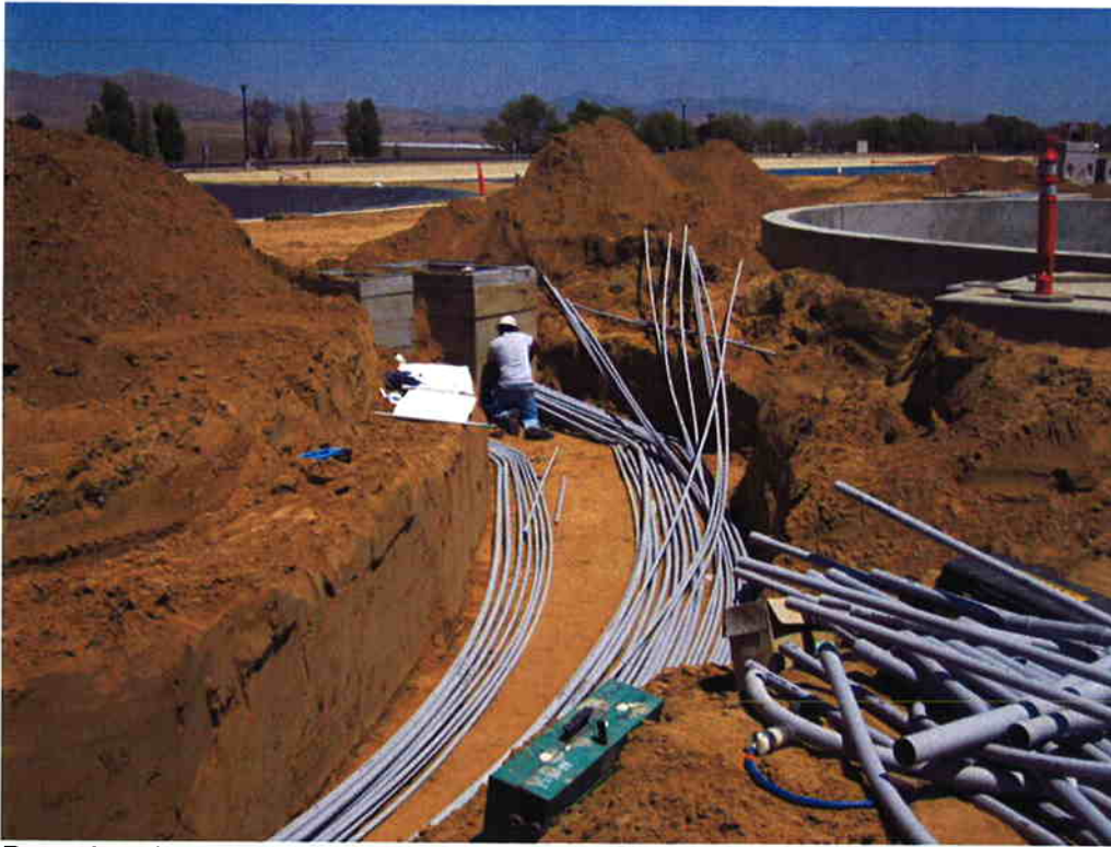
Bergelectric installing Duct Bank #25 into Pull Box #25.
