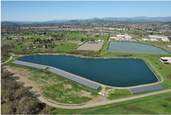
First PV System Installed on the Face of a Dam: Sonoma County Water Agency (600 kW)
