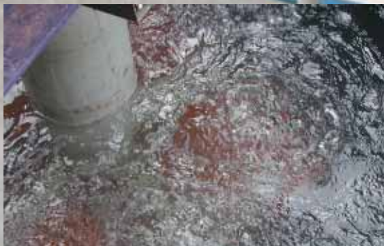
A new circular, vortex grit trap that introduces air floatation to enhance the in-tank classification of the mineral solids.
