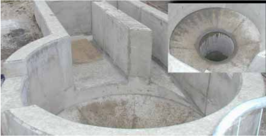
Civil construction and installation.
