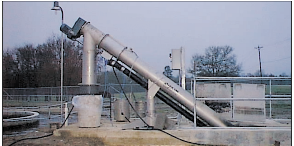
Combines screening, conveying and dewatering into one reliable, automatic, cost-efficient system.
