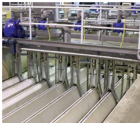
AquaDiamond® backwash assembly and laterals.
