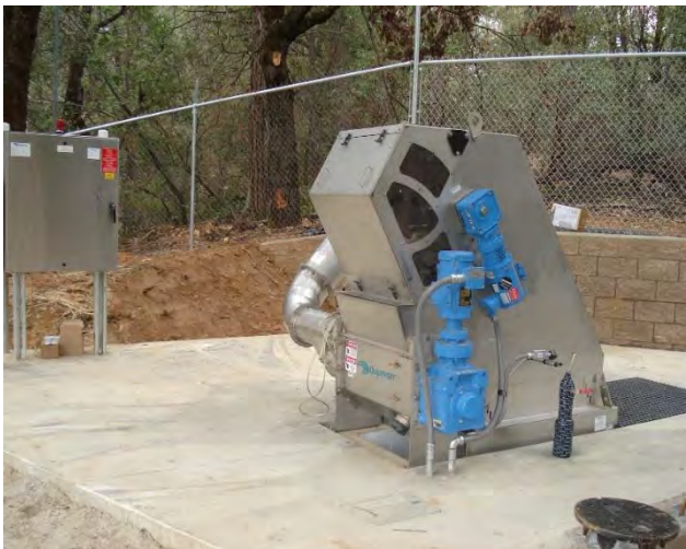
Duperon Low-Flow FlexRake® and washer compactor
