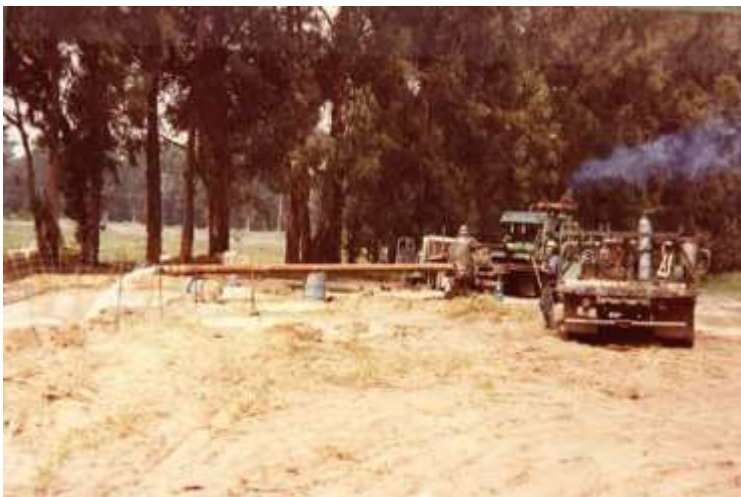
Construction at Eureka well site, the District's largest production well, circa 1979
