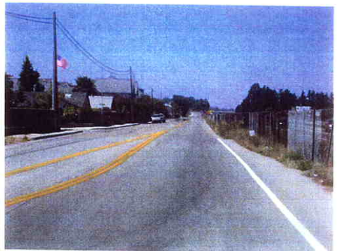
Southland Street and South Frontage Road
