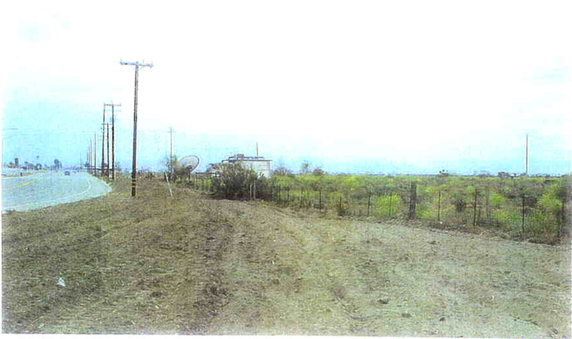
Photo 4: Blosser Road looking South Pump Station No. 1, Site 2
