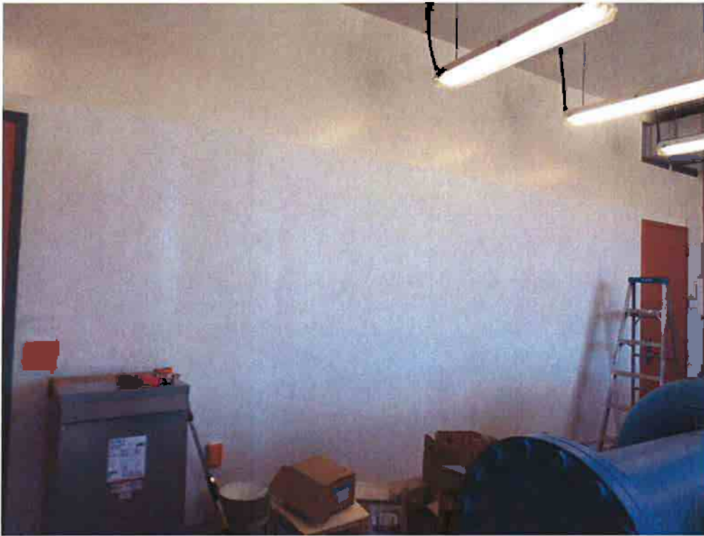
Painting plywood wall inside pump room.
