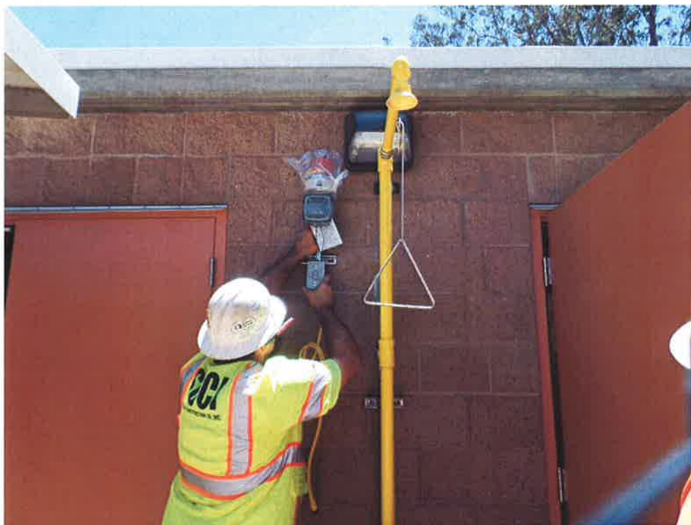
Spiess installing the emergency eye wash station.
