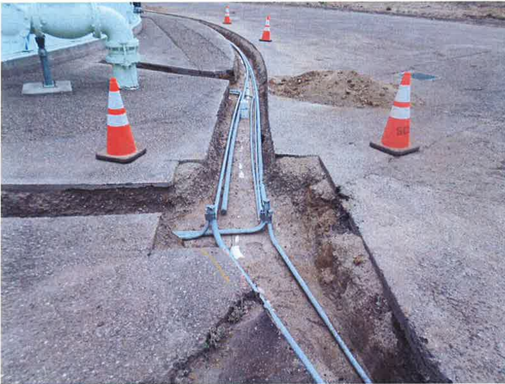
Conduit installation at the Quad Tanks.
