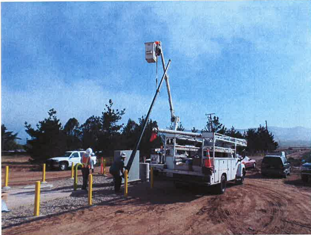
St. Denis Electric installing the SCADA tower at the PRV vault.
