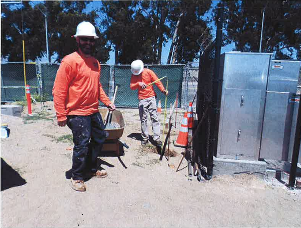
Spieß installing bollards.
