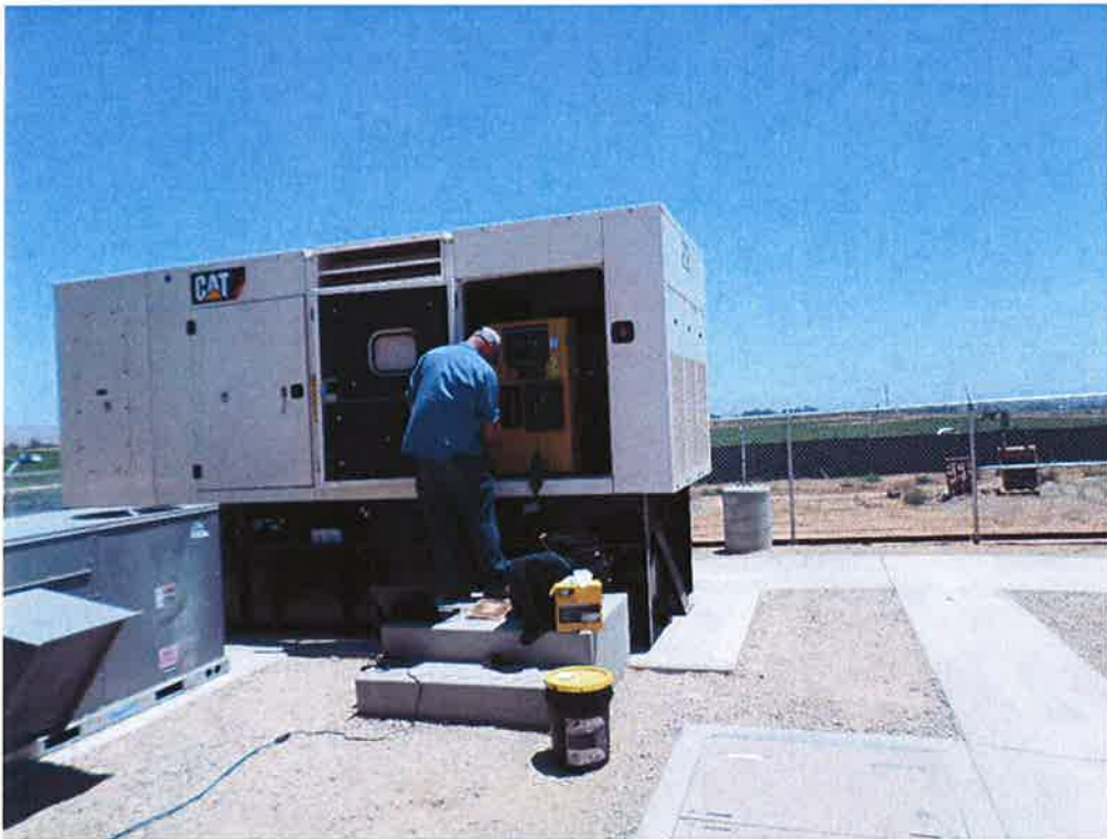
Setting up Emergency Generator at pump station.
