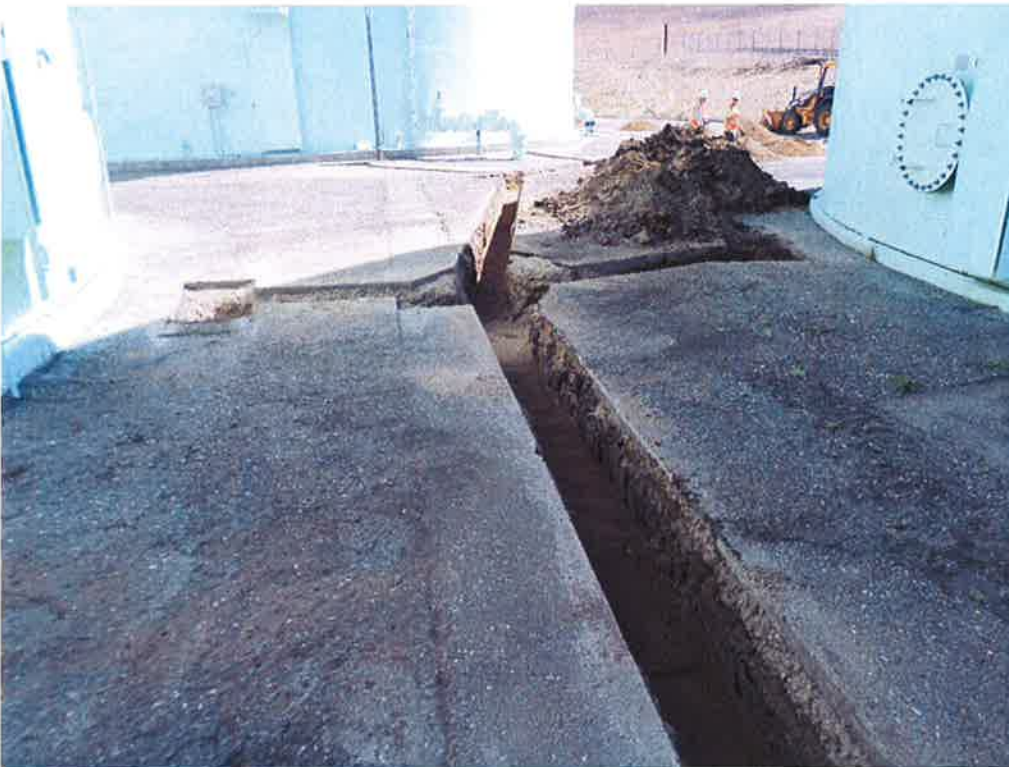
Spiess placing sand in trench at Quad Tanks.
