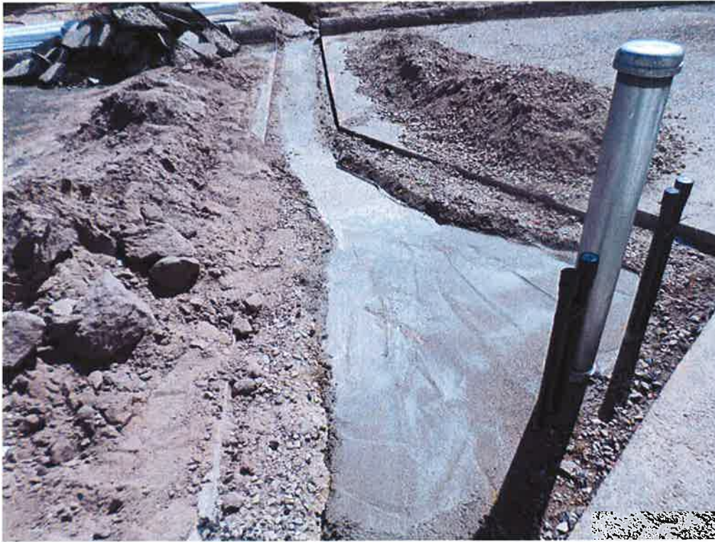
Slurry poured over the 4-inch drain line and conduits at the Standpipe Tank.
