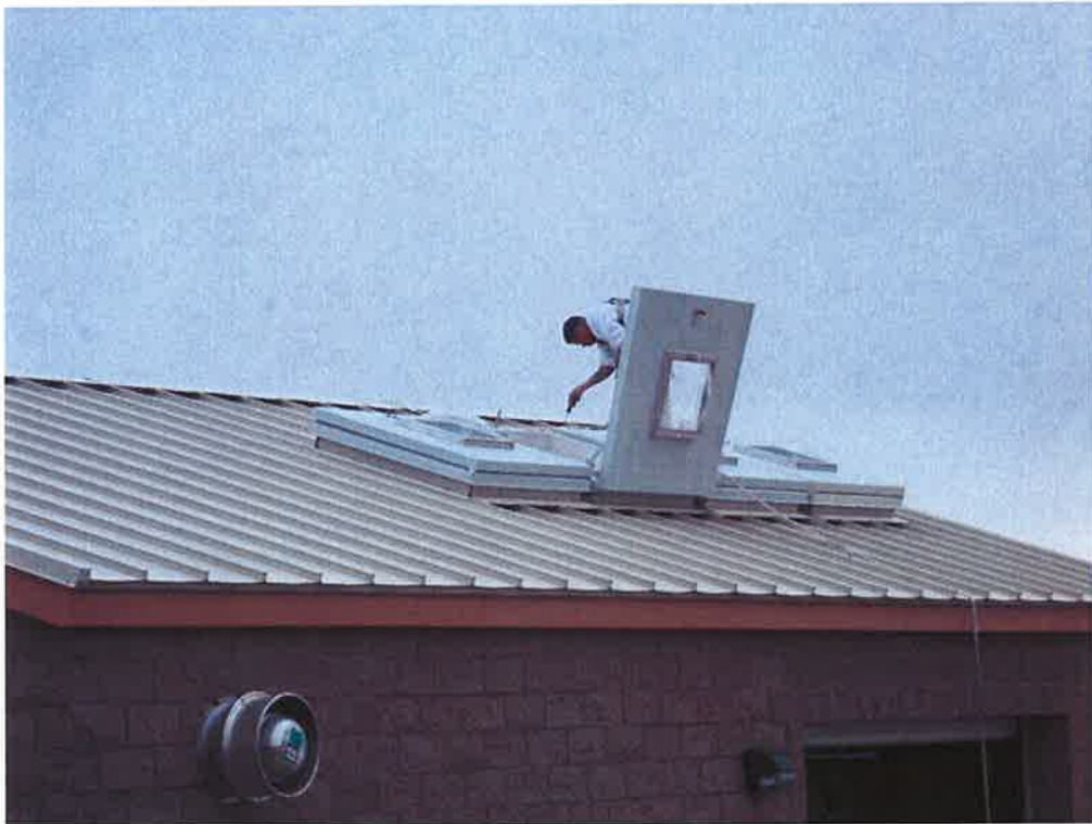
Coast Painting coating roof hatches.
