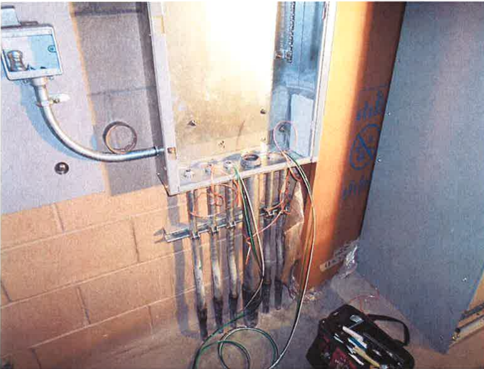
St. Denis Electric pulling power conductors in electrical room.
