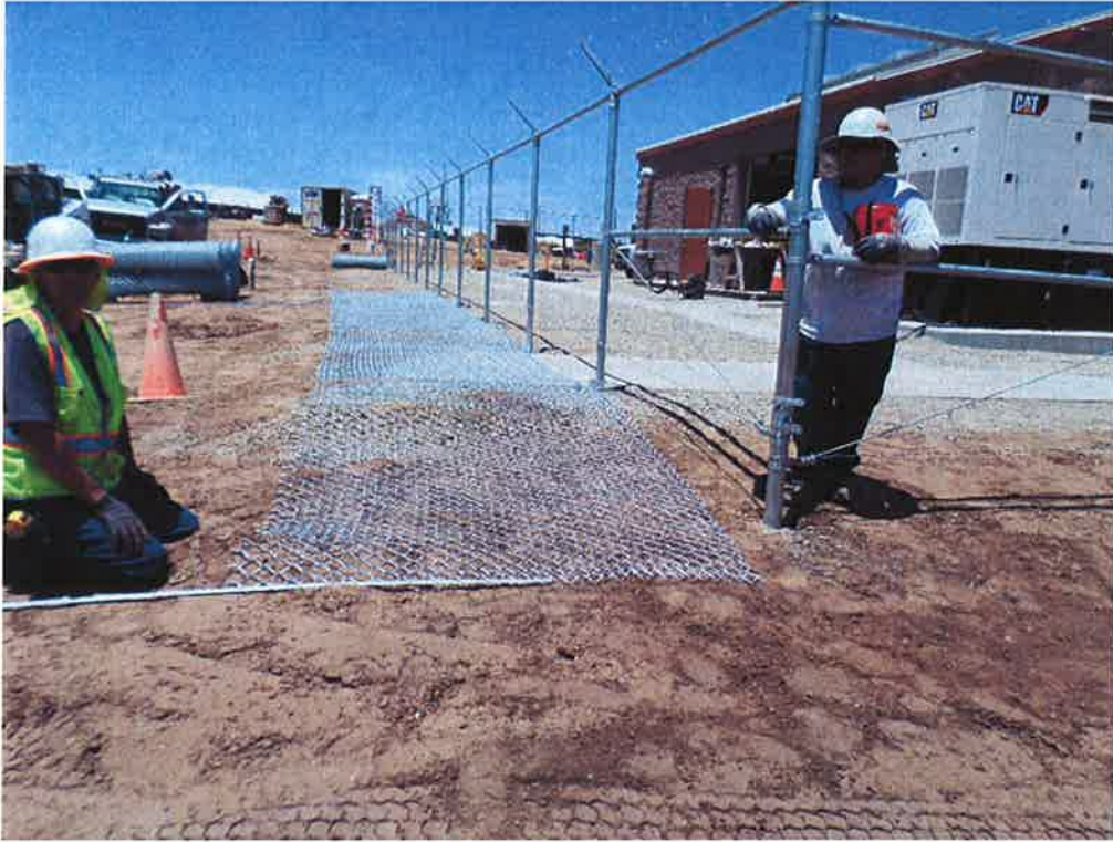
Central Coast Fencing installing fence fabric.
