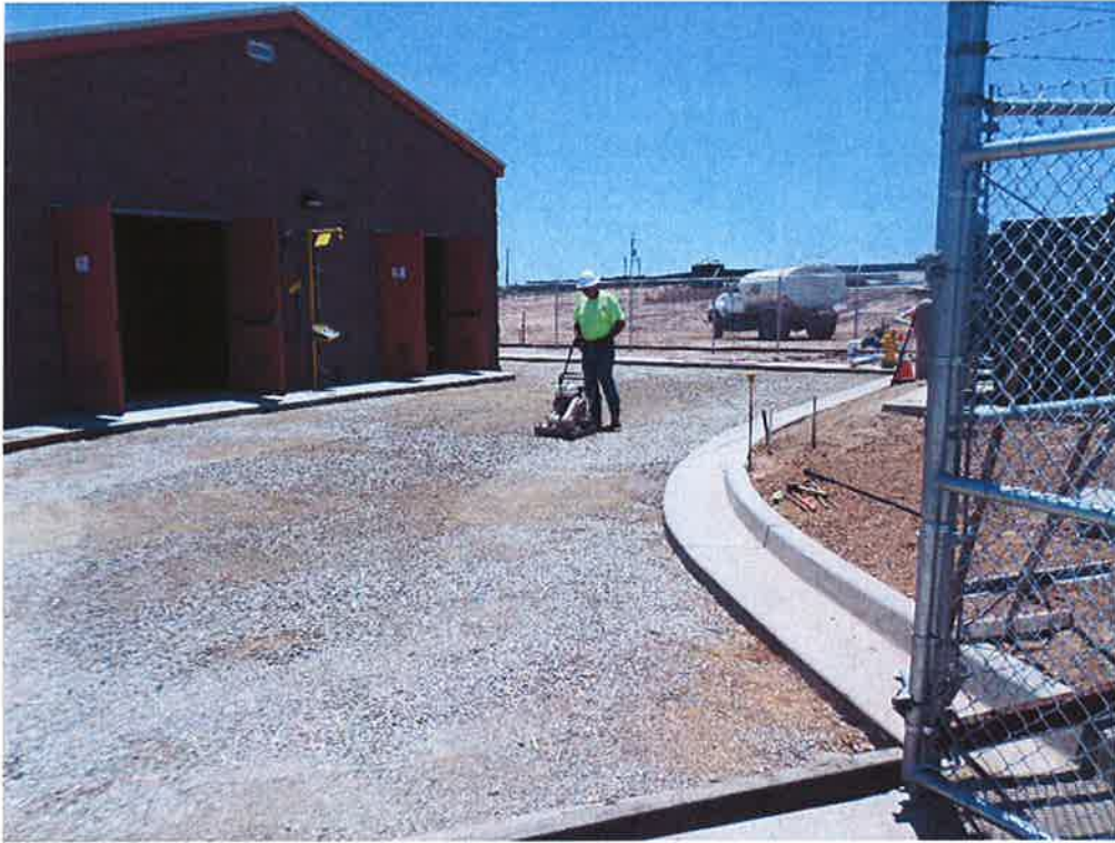
Spiess compacting base in preparation for driveway paving.
