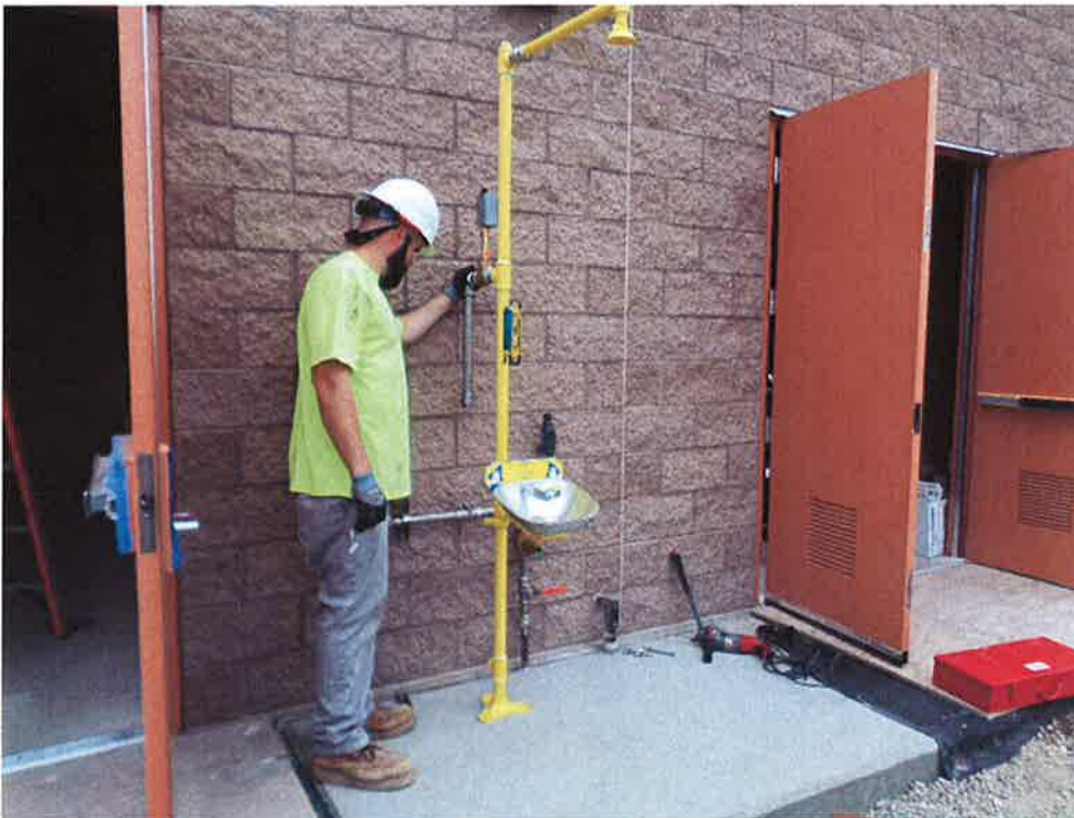
Spiess installing emergency eyewash station.
