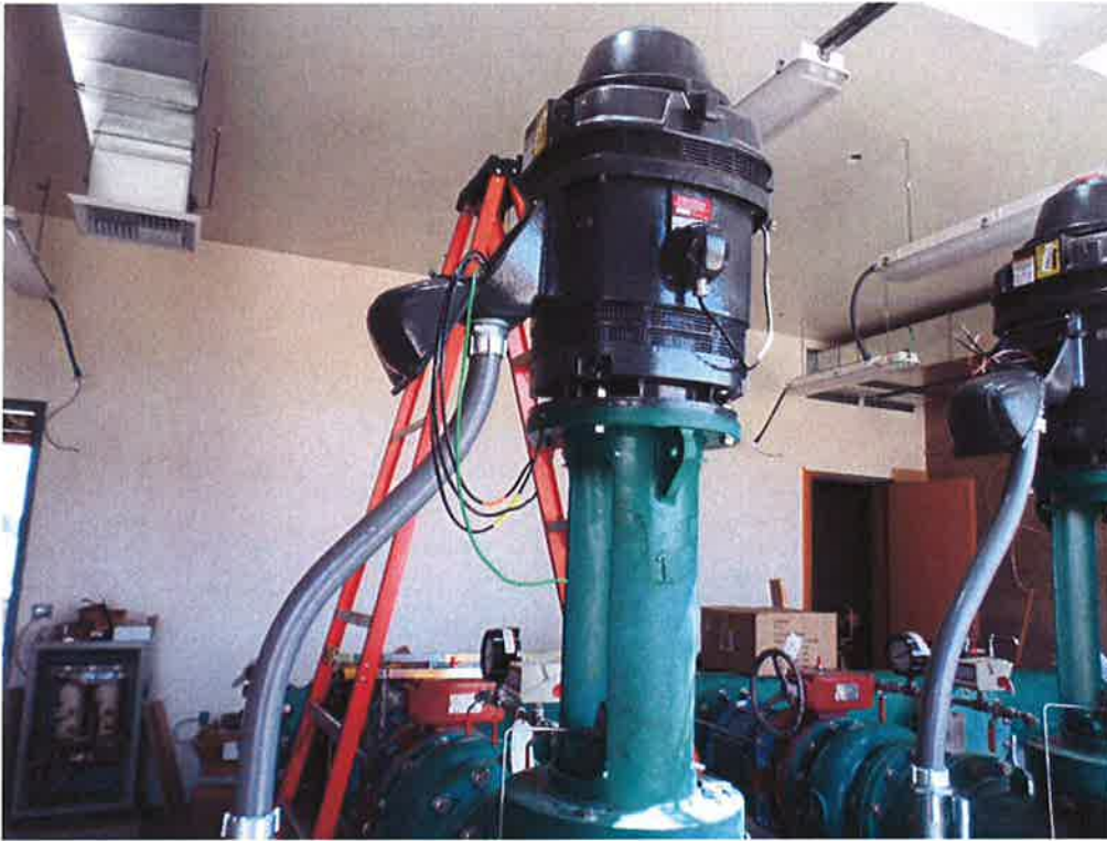
Pulling power wire to the vertical turbine pumps.
