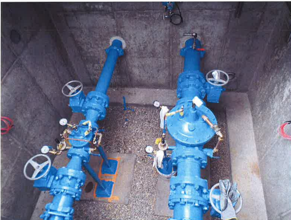
Coast Painting coating pipes inside the PRV vault.
