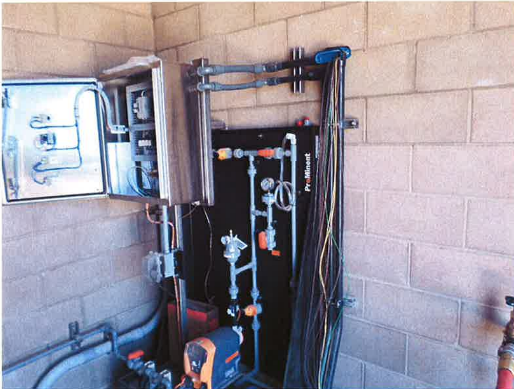
St. Denis Electric pulling wire to the chemical feed pumps.
