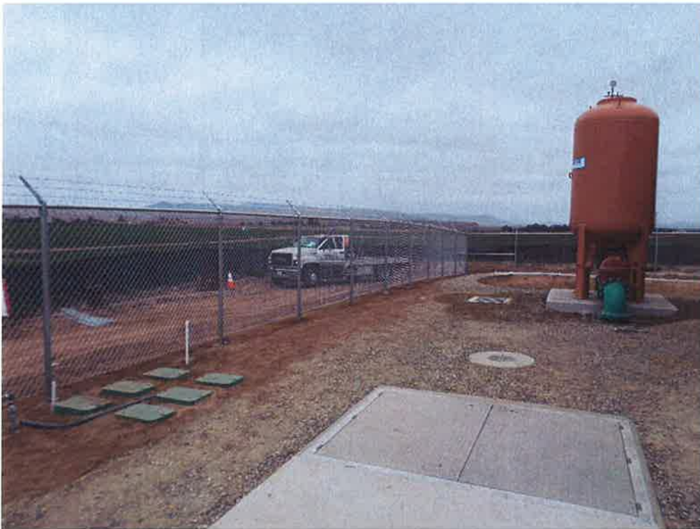
Central Coast Fencing completing fencing installation.
