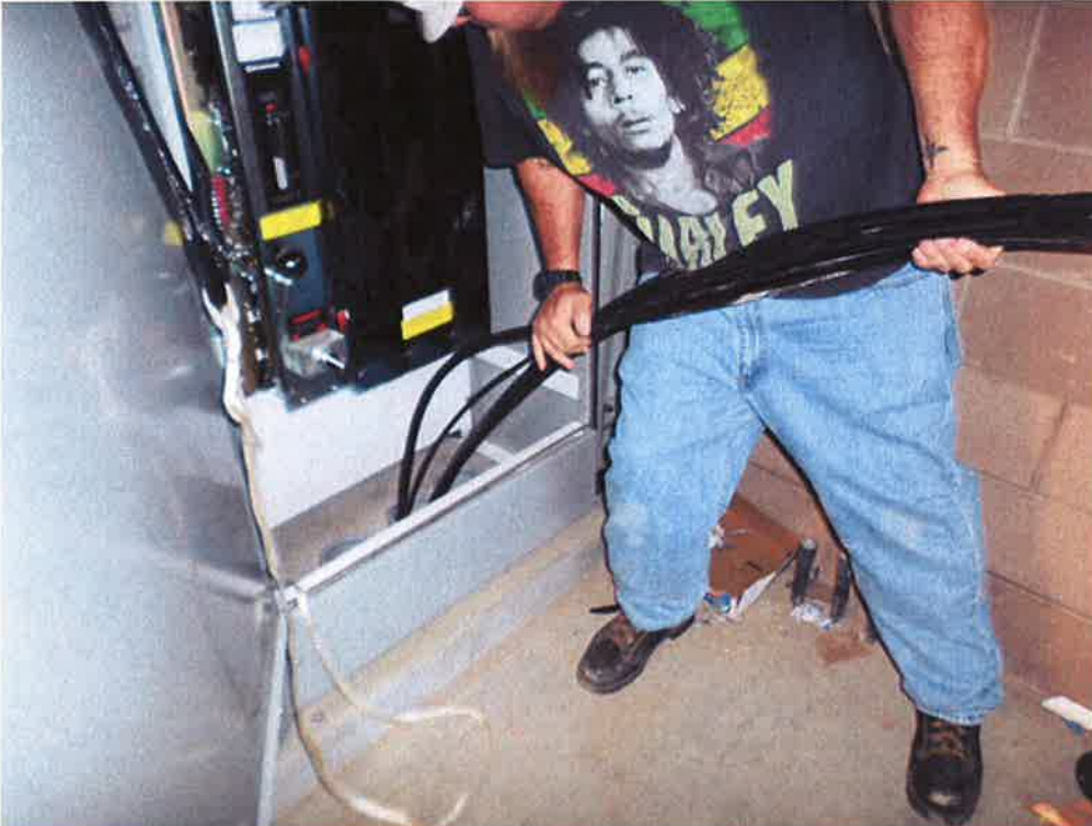
Pulling the wire at the ATS in the electrical room.
