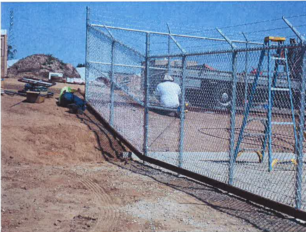
Central Coast Fencing completing fence installation.
