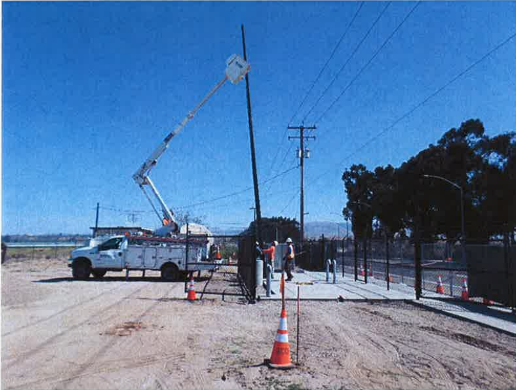
St. Denis Electric installing the SCADA tower.
