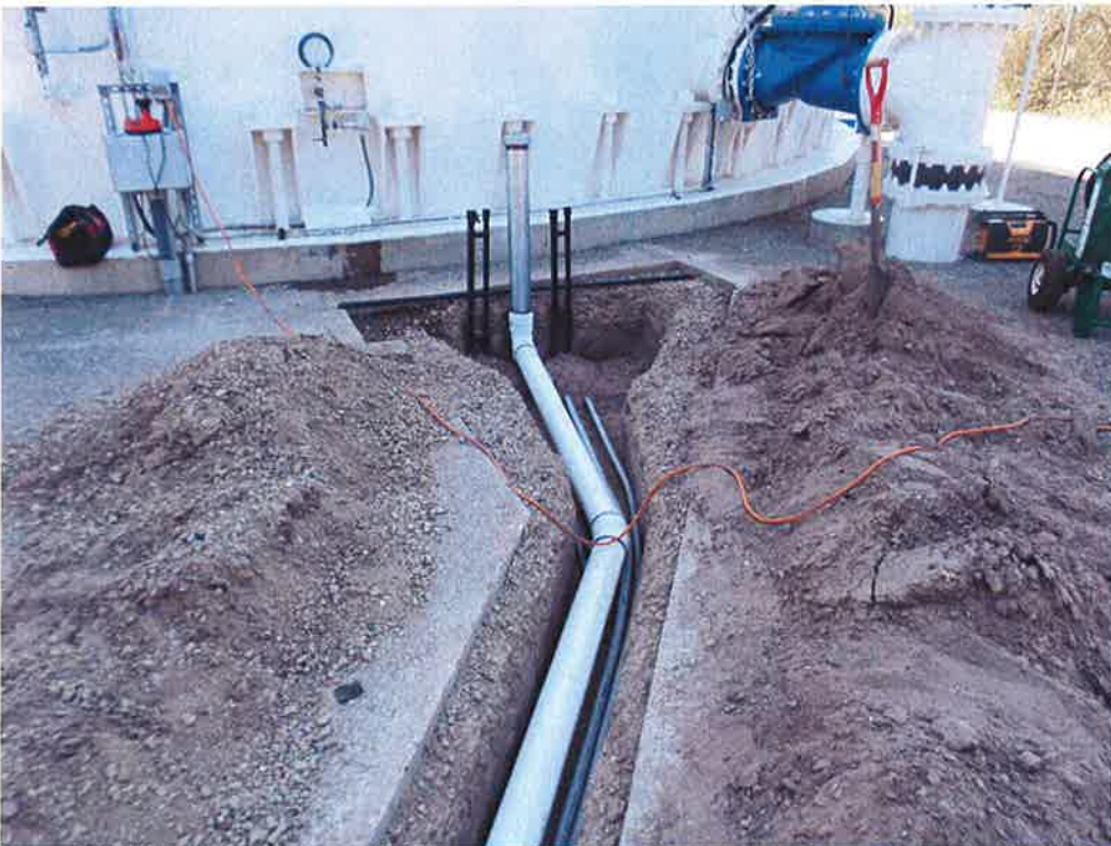
Drain line and conduit being installed at the Standpipe Tank.
