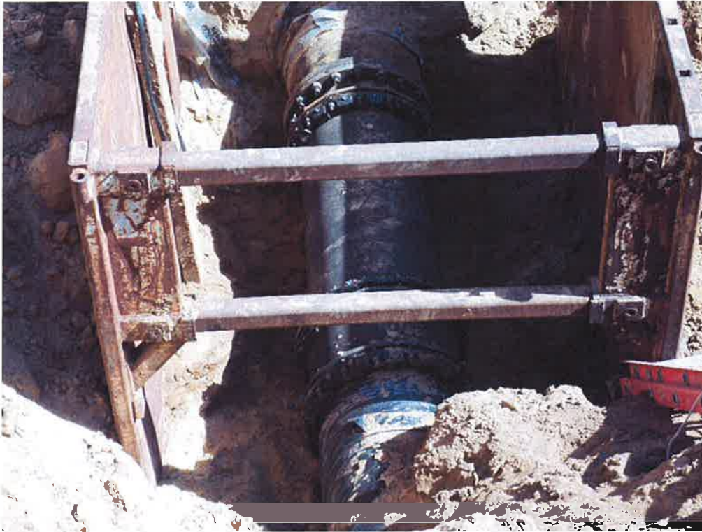
Connection of the 24-inch DIP to the HDPE pipe from Bid Package #1 completed.
