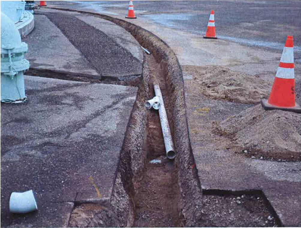
Spies installing the 4-inch drain line at the Quad Tanks.
