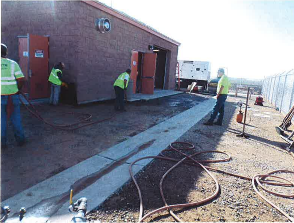
Toste Grading and Paving preparing base for asphalt.
