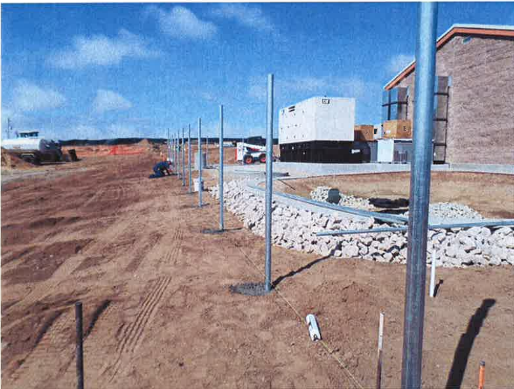
Setting fence posts.
