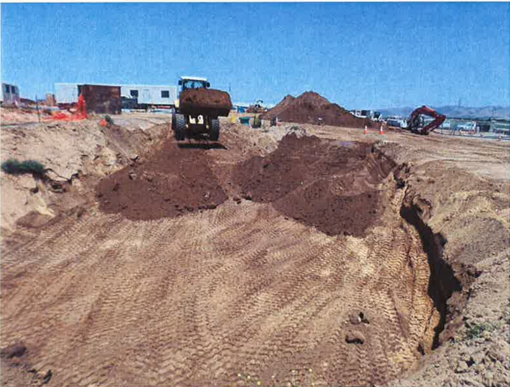
Spiess backfilling connection of pump station to HDPE pipe.
