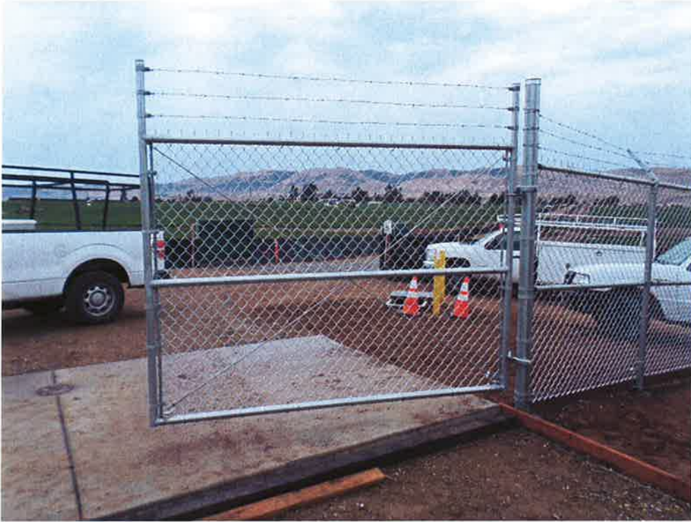
Central Coast Fencing installing 8-foot site access gates.
