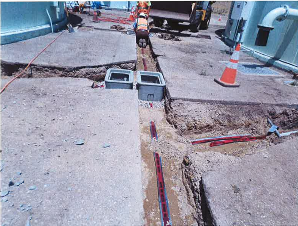
Pull boxes being installed at the Quad Tanks.
