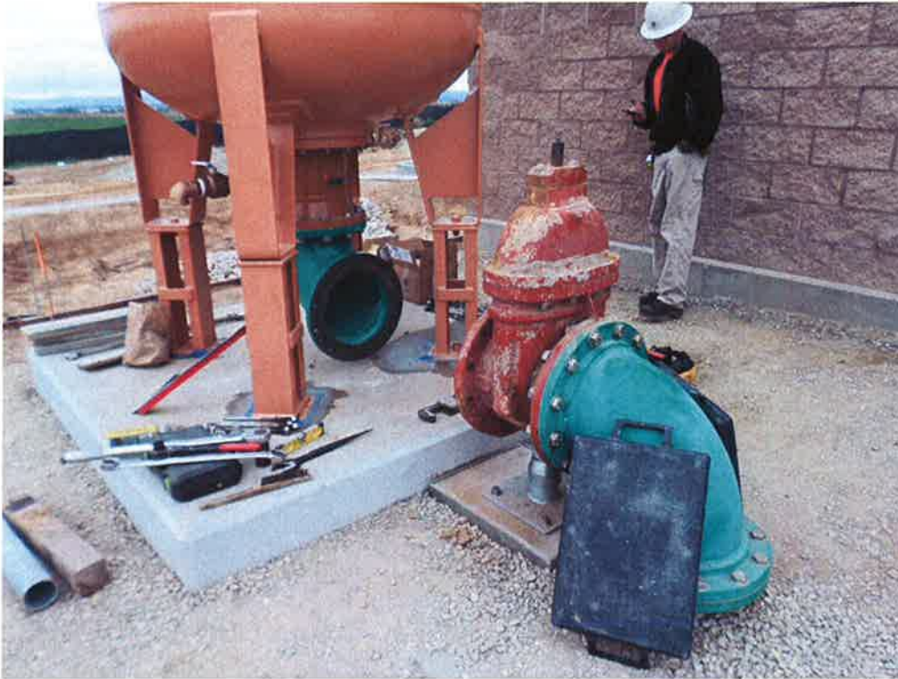
Spies installing the valve at the surge tank.
