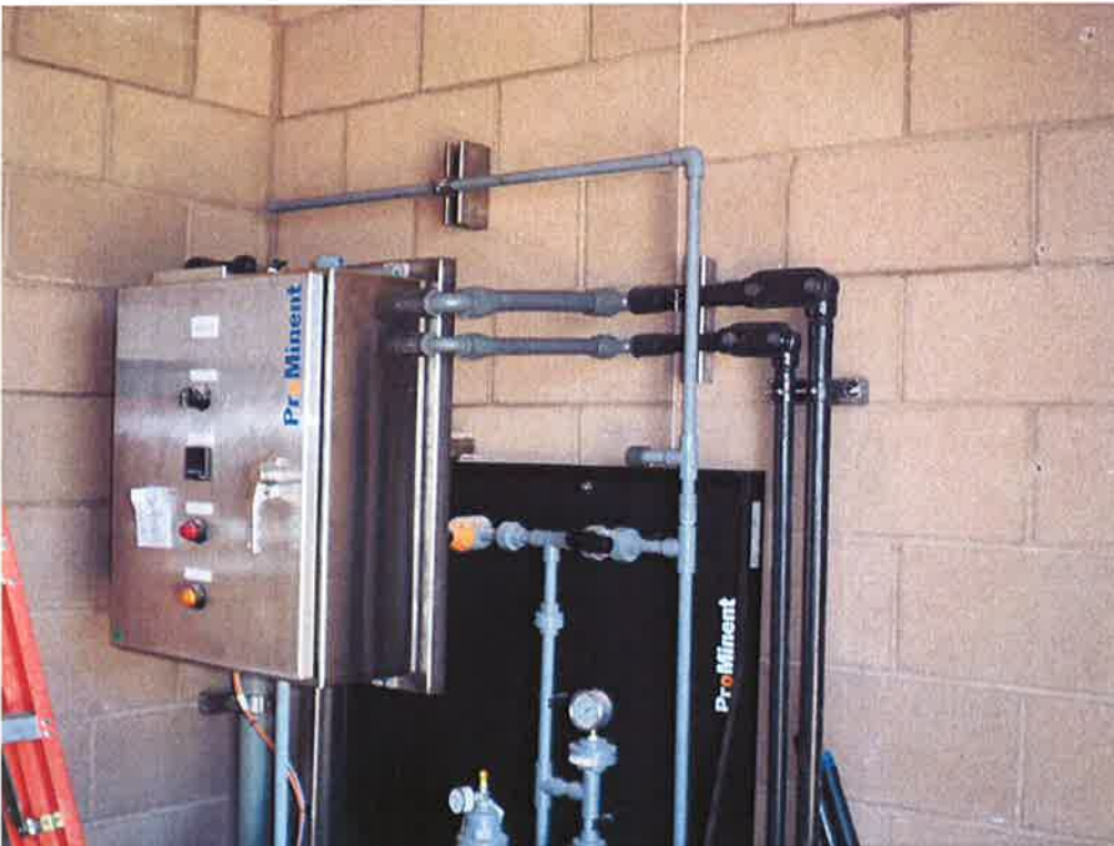
Spiess installing chemical feed pump piping.
