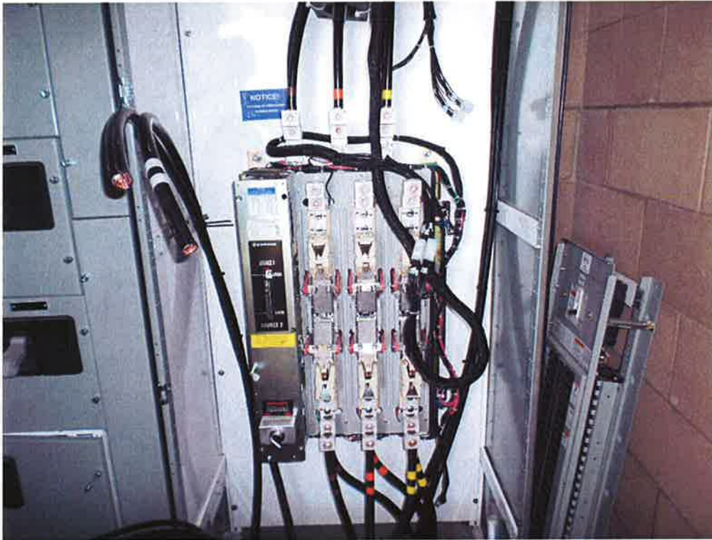
St. Denis Electric terminating the main feed at the ATS.
