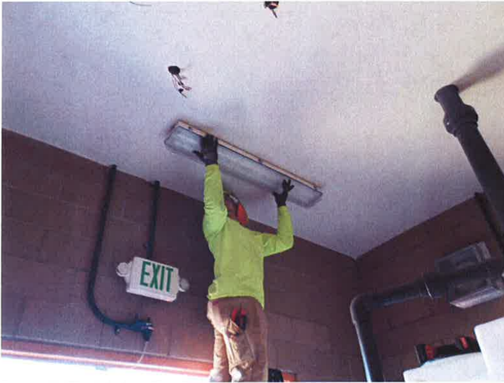
St. Denis Electric installing lights in pump room.
