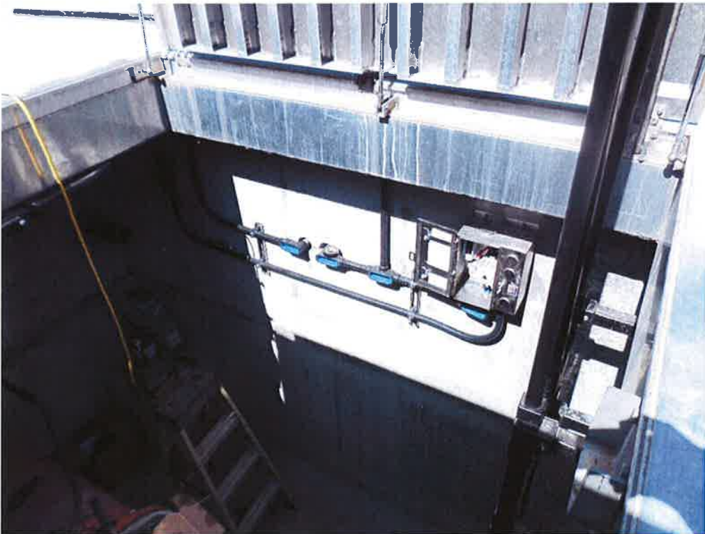
Installing electrical conduit in the vaults.
