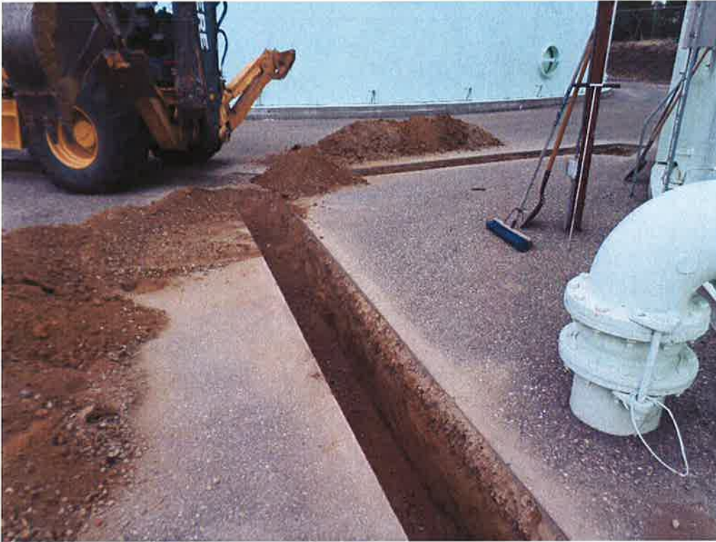
Spiess excavating trench to prepare for installation of drain line and conduits at the Quad Tanks.
