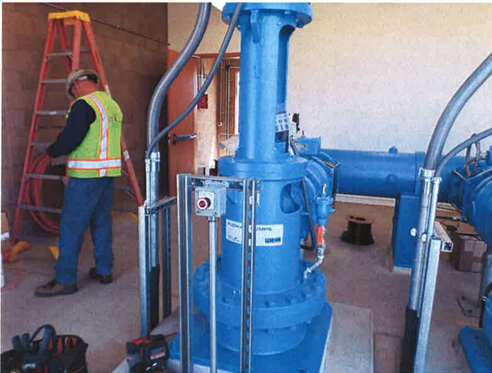
Installing emergency stop buttons (E-stops) at the vertical turbine pumps.
