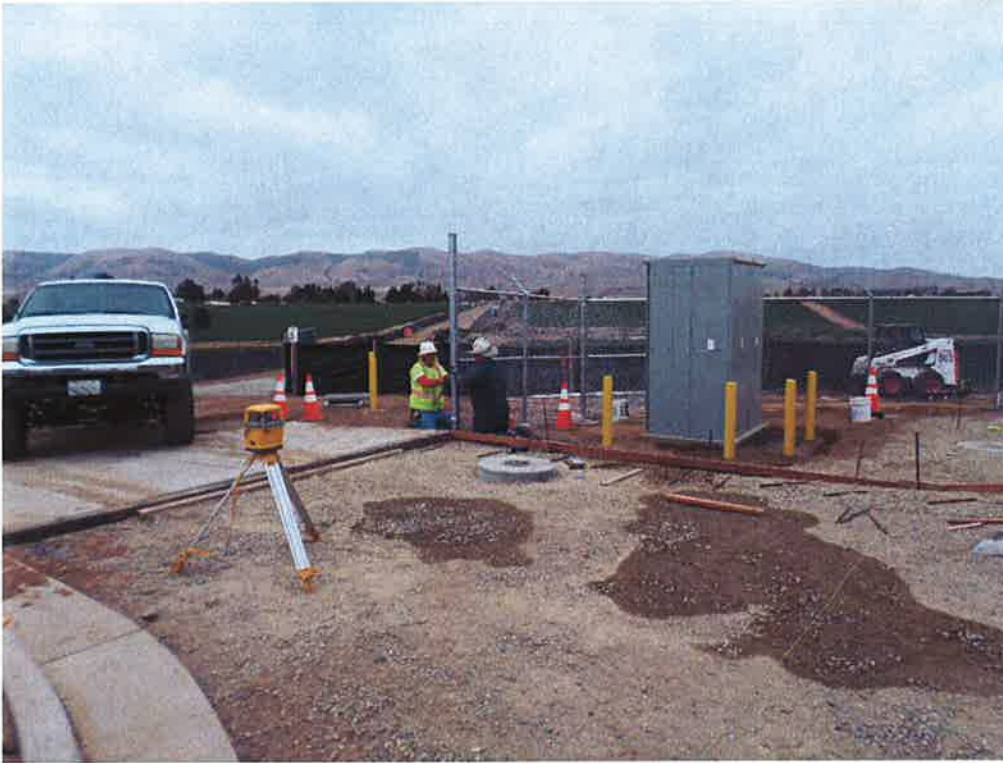
Central Coast Fencing completing fence installation.
