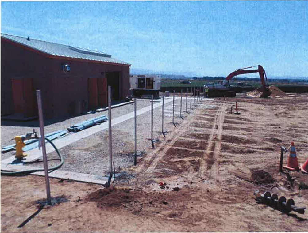
Central Coast Fencing setting fence posts.
