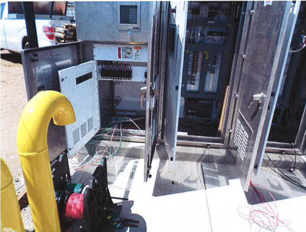
St. Denis Electric pulling wire to electrical and control panels.
