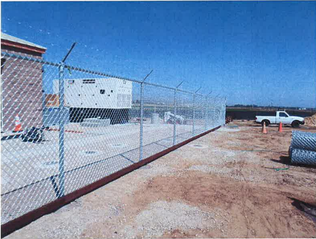
Fence installed at the pump station.
