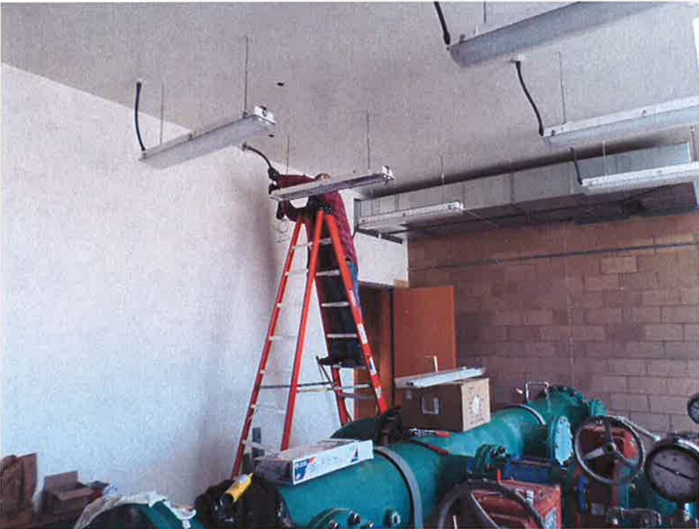
St. Denis Electric installing lighting pigtails in pump room.
