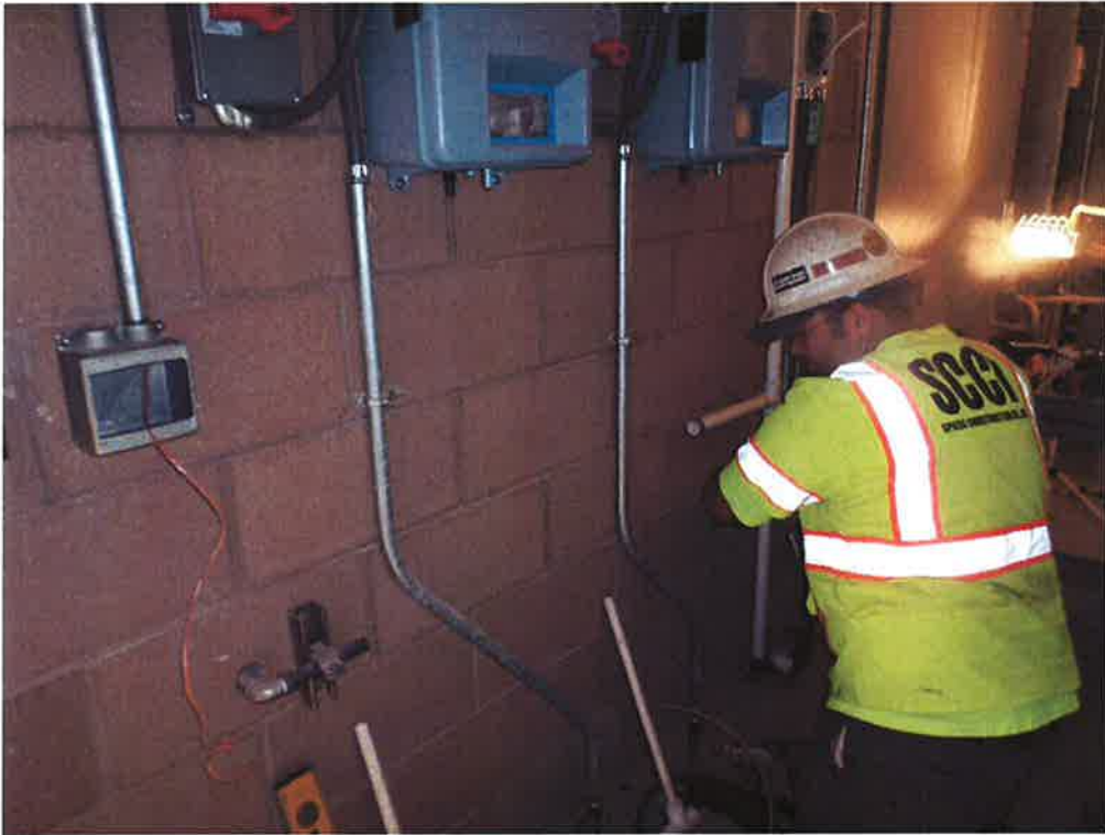
Spieß installing chlorine analyzer piping.
