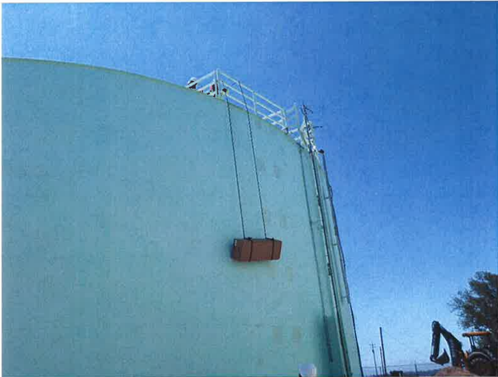
Spies staging materials for mixer installation at the Quad Tanks.
