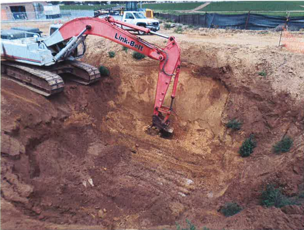
Spiess backfilling pipe connection.
