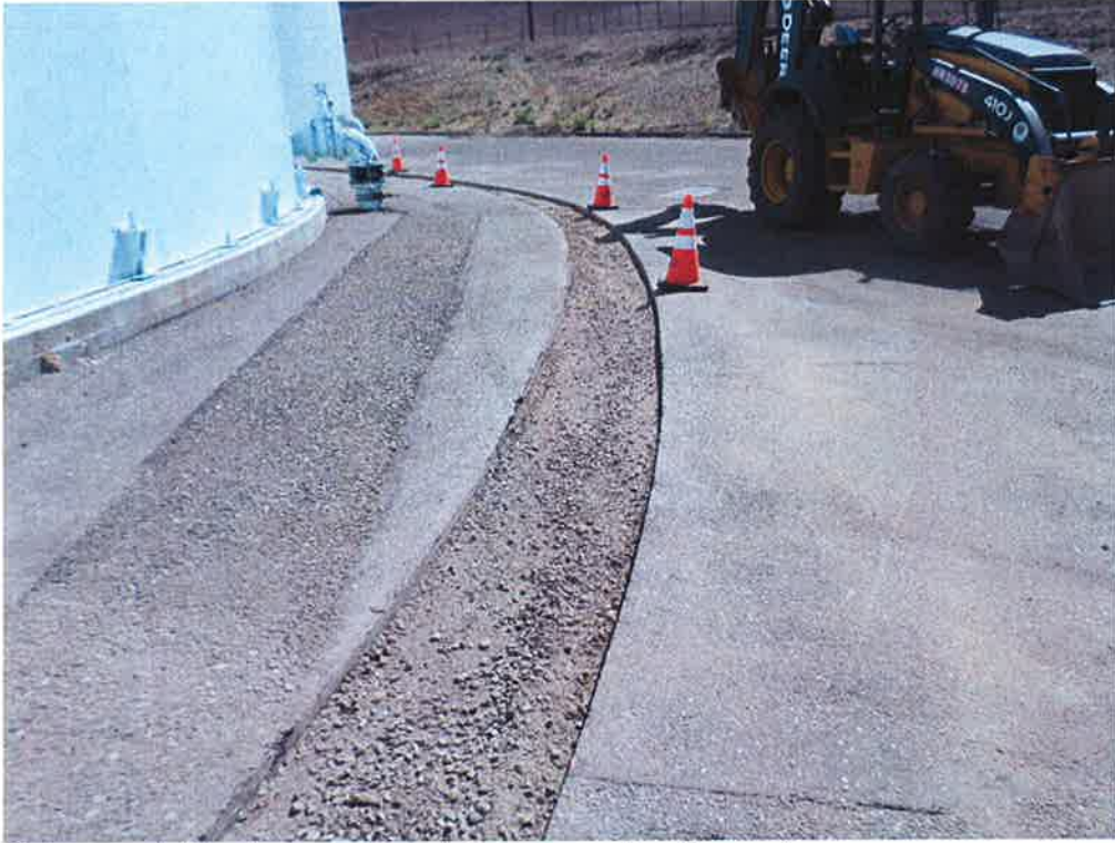
Spies installing base in trench in preparation for paving.
