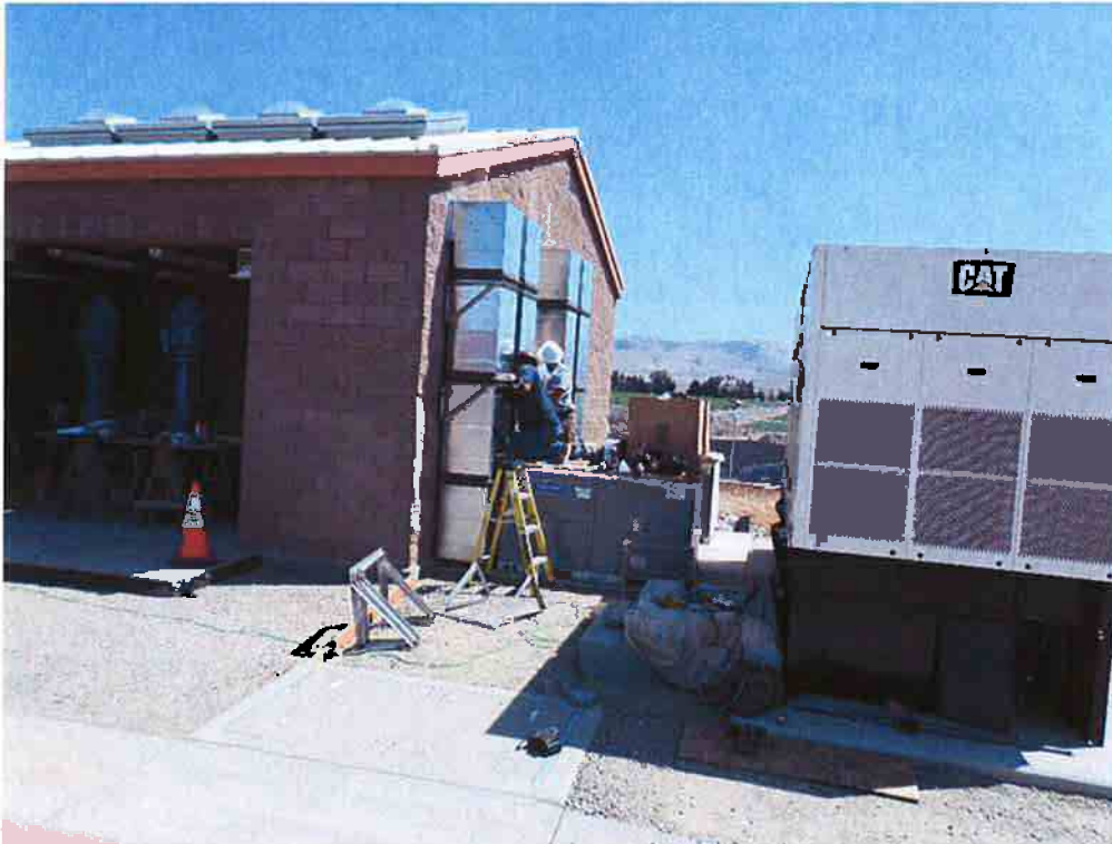
DAHL Air Conditioning installing AC duct supports.
