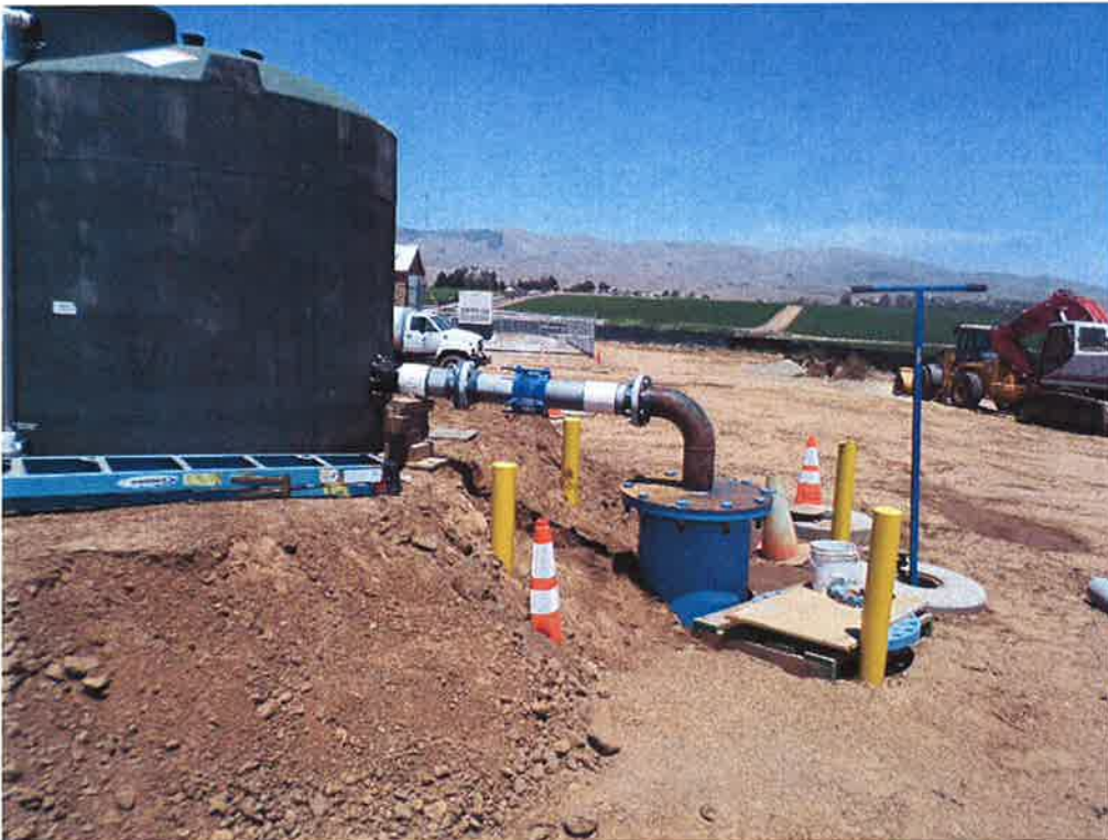
Temporary tank and piping for testing the pump station prior to taking water from the City of Santa Maria.
