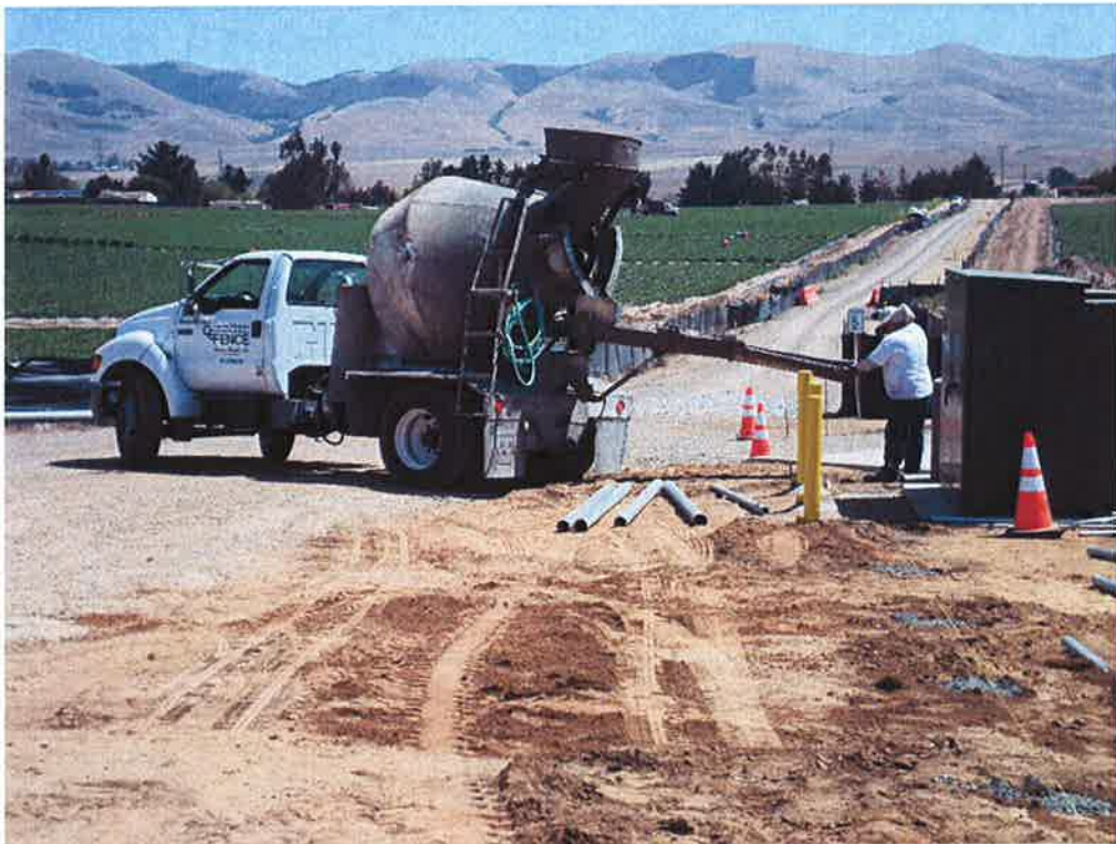
Central Coast Fencing pouring concrete to set fence posts.
