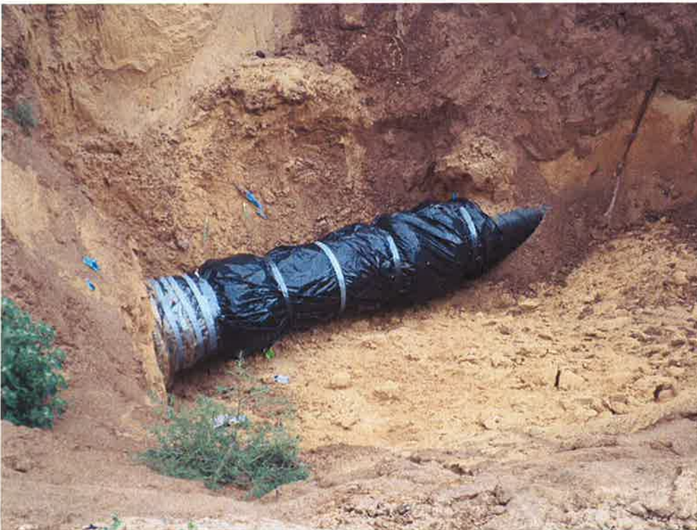
Connection wrapped in plastic and ready for backfill.
