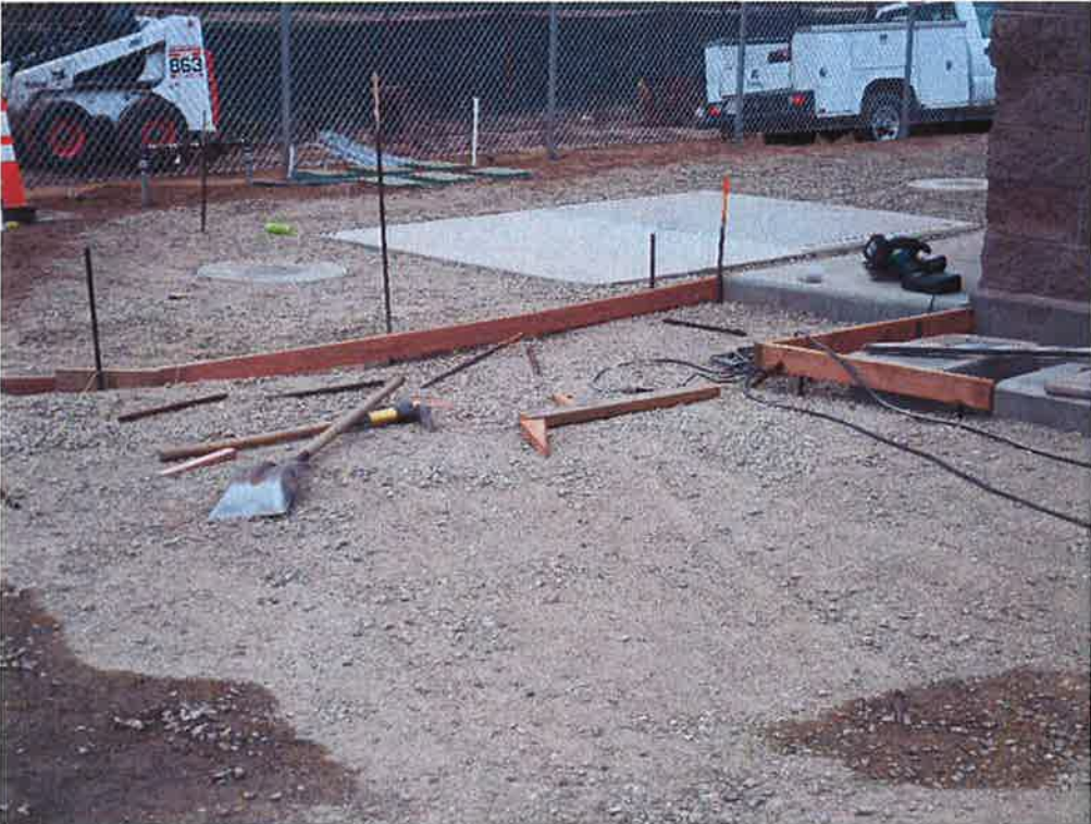
Spiess installing border for pavement for pump station driveway.
