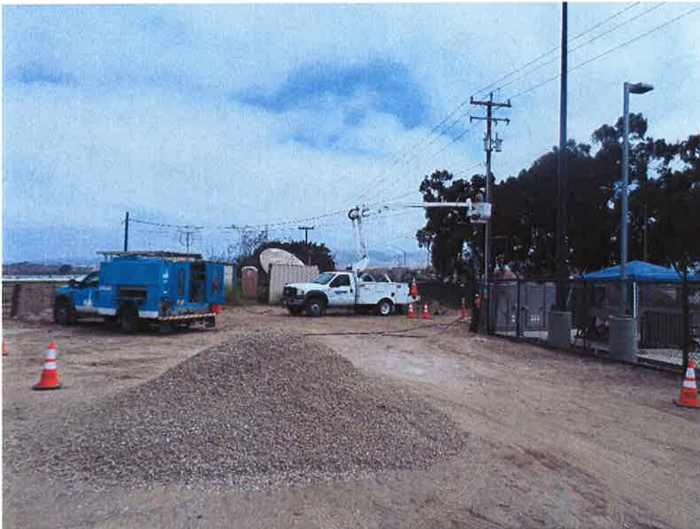
PG&E on site to provide power service to the site.
