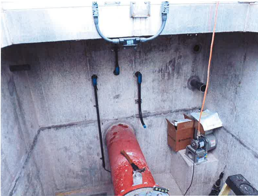
Installing electrical conduit in the vaults.
