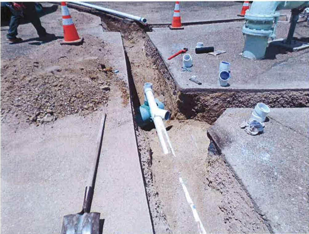
Installing the 4-inch drain line at the Quad Tanks.
