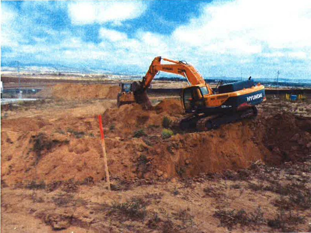
PHC excavating for new reservoir.
