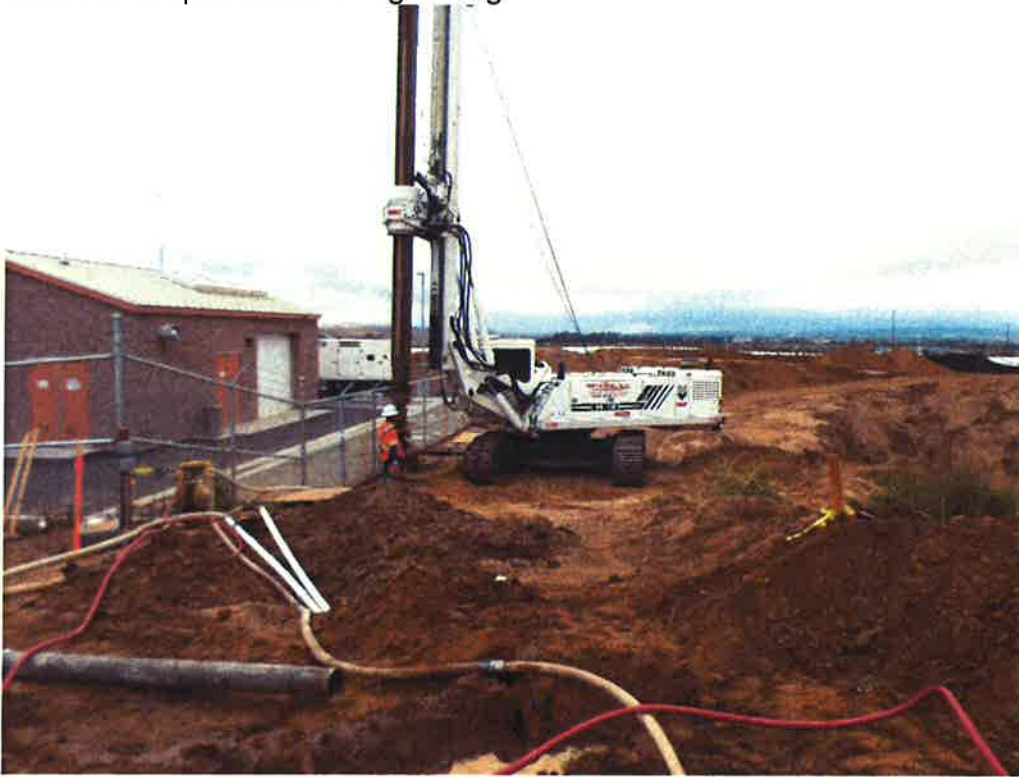
Curtis Drilling starting drilling again using drilling mud to stabilize holes.
