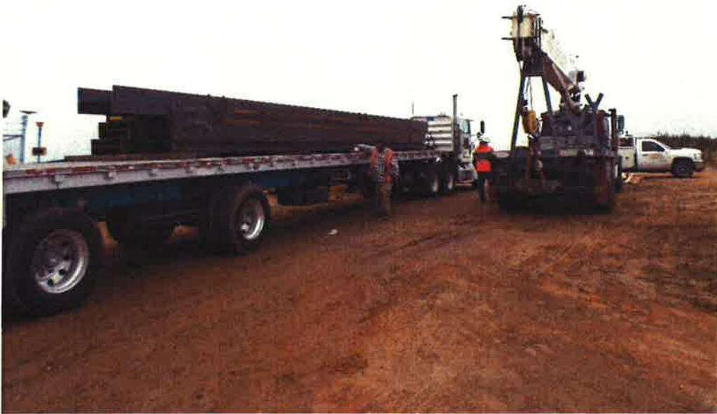
Delivery of I-beam piles for shoring.
