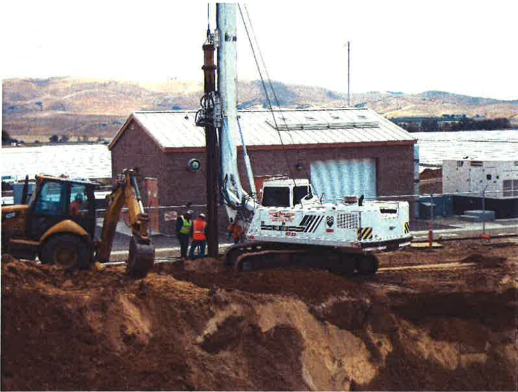
Curtis Drilling continuing drilling hole for pile installation.
