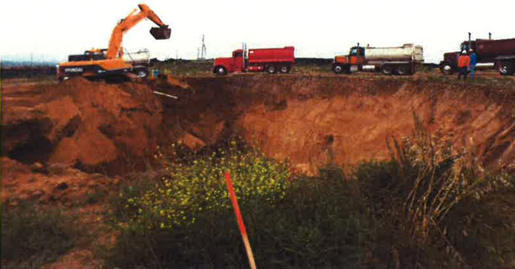
PHC excavating for new reservoir and hauling export material off site.
