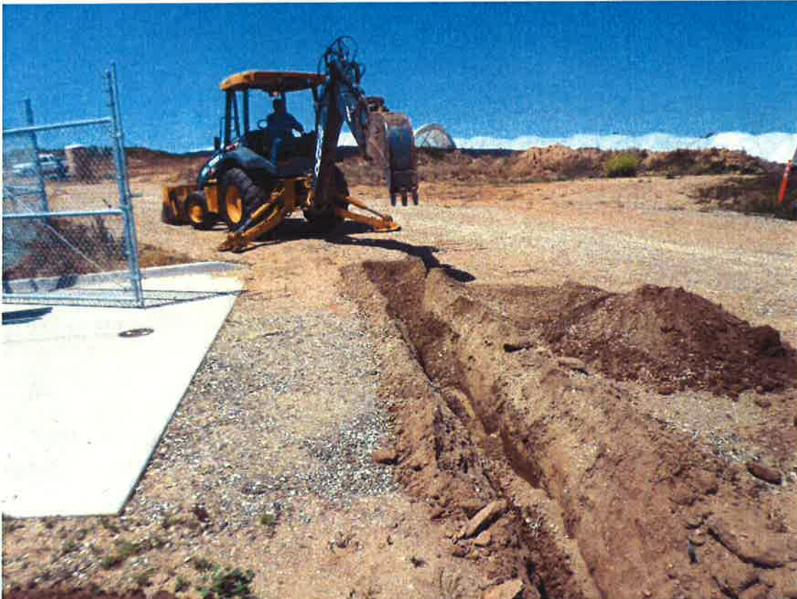
PHC trenching for temporary power for field office trailer.
