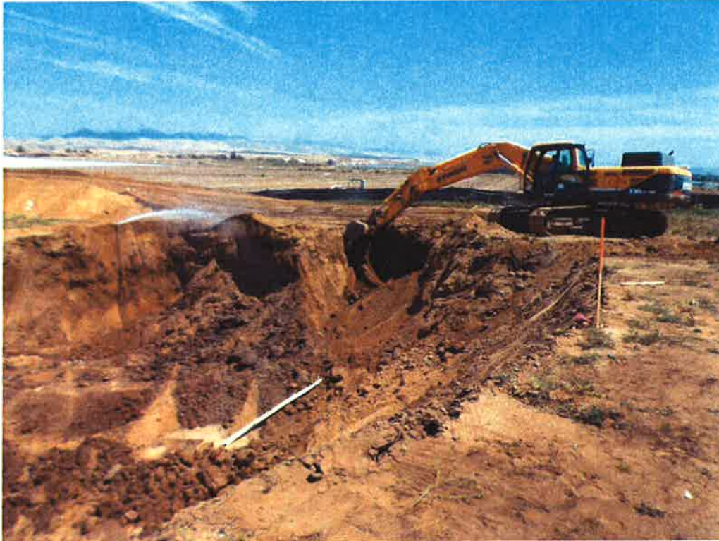
PHC excavating for new reservoir.
