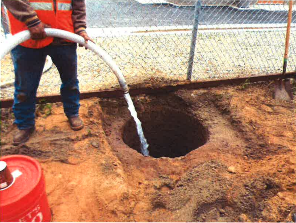
Curtis Drilling adding polymer and water to drill hole.
