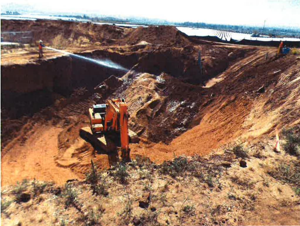
PHC excavating for new reservoir.
