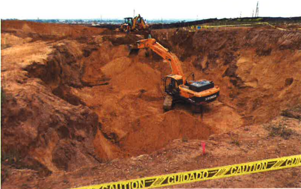
PHC excavating for new reservoir.
