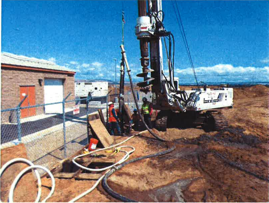
Pumping concrete into hole with I-beam pile installed.
