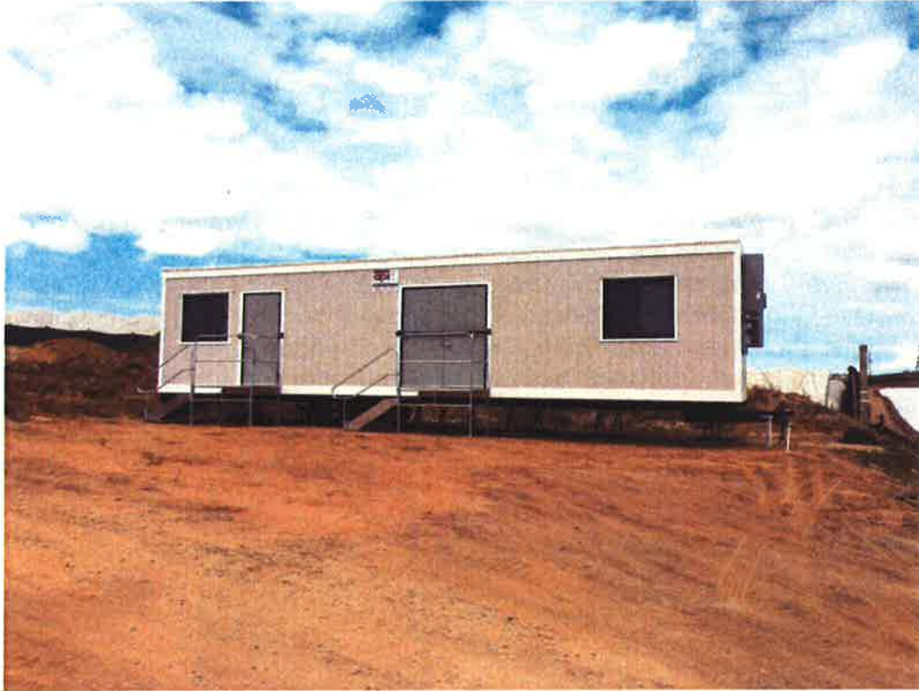
Temporary field office.
