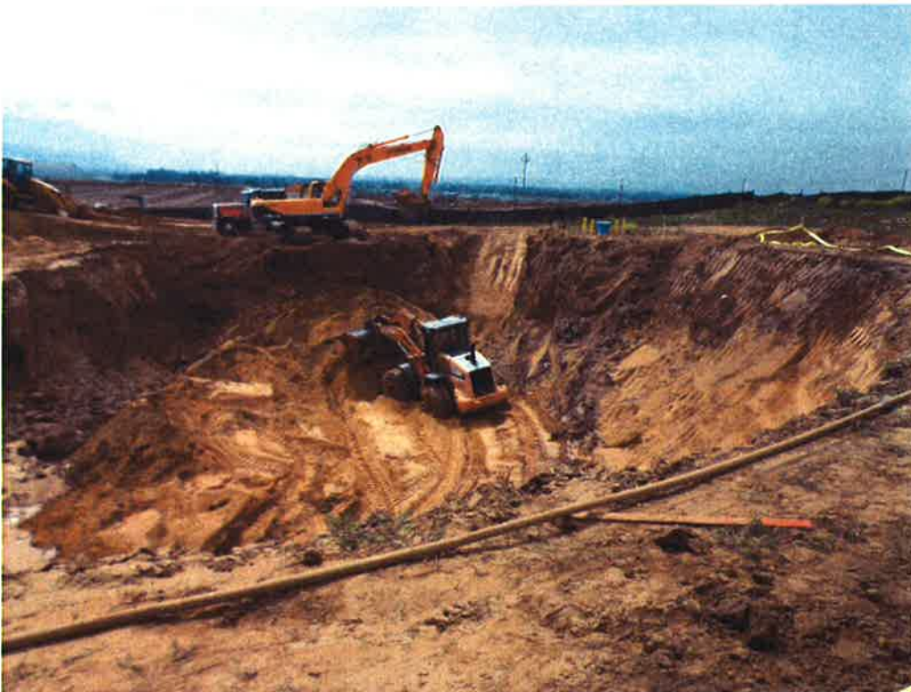
PHC continuing excavation for the new reservoir.
