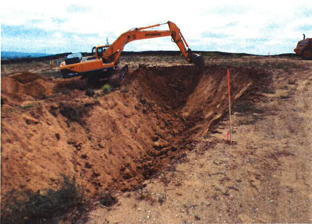
PHC starting excavation for the new reservoir.
