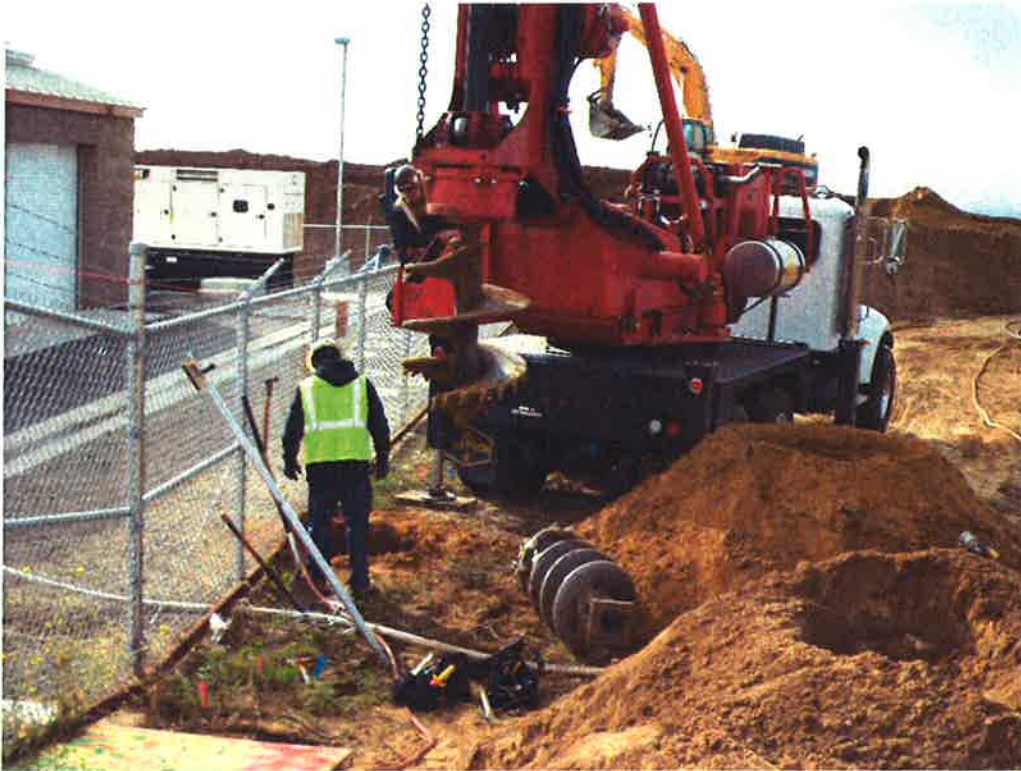
Curtis Drilling coring for installation of I-beam piles.
