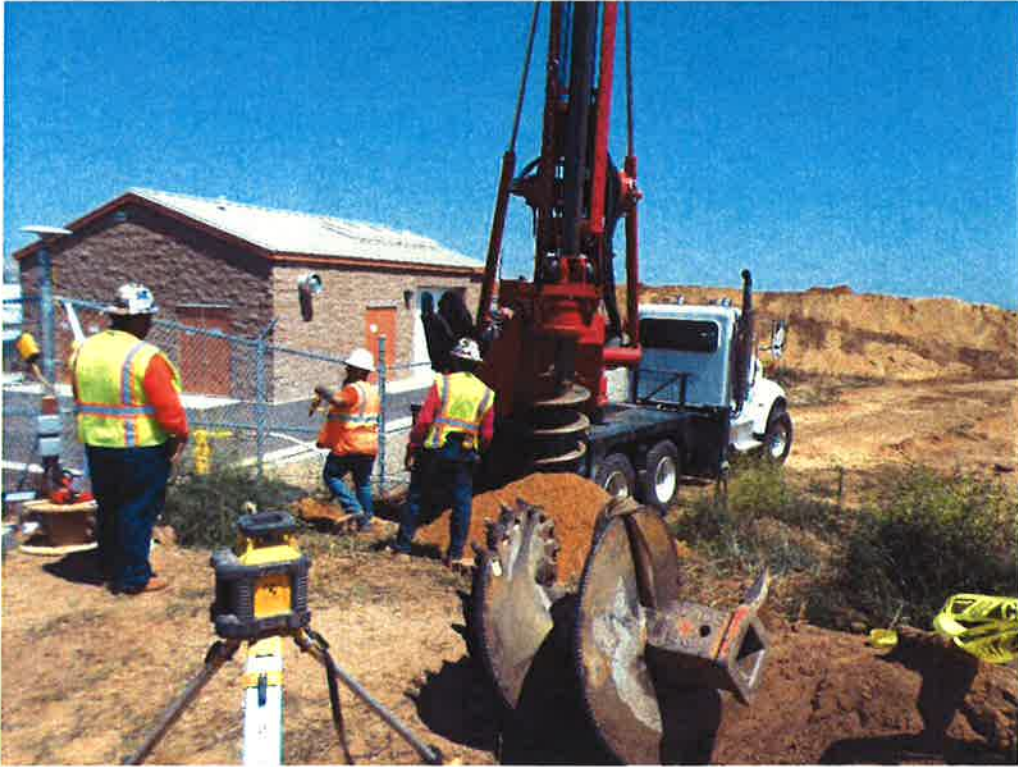
Curtis Drilling on site beginning drilling for shoring piles.
