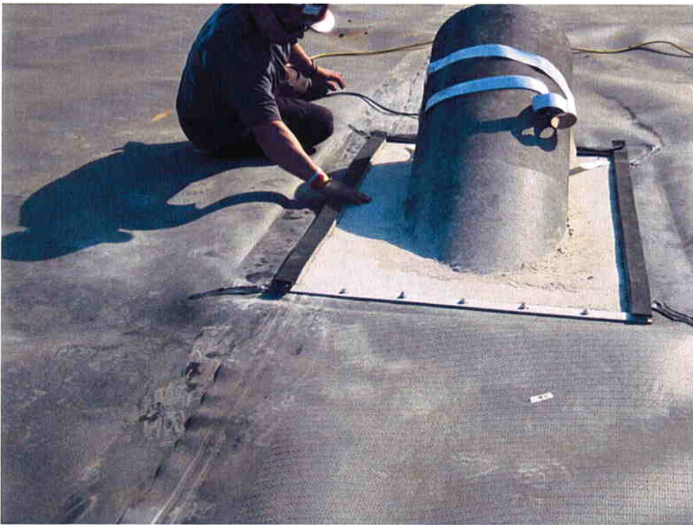
Installing the baton and boot at the inlet pipe penetration in Aeration Basin #1.
