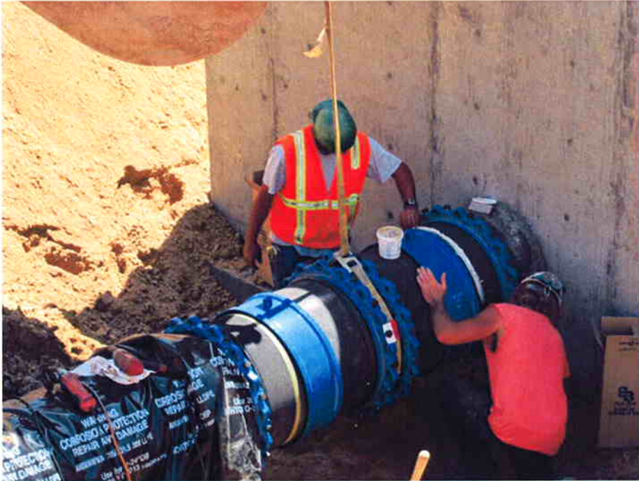
Cushman installing 24" ML pipe connection into Distribution Box #2.
