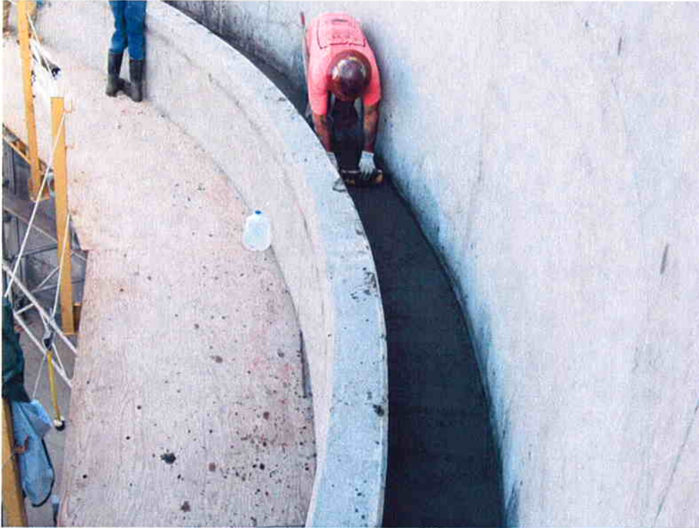
Finishing concrete floor of launder in Clarifier #2.
