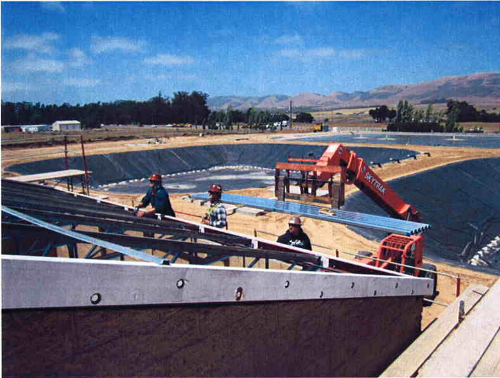
Cushman installing metal decking on truss system.
