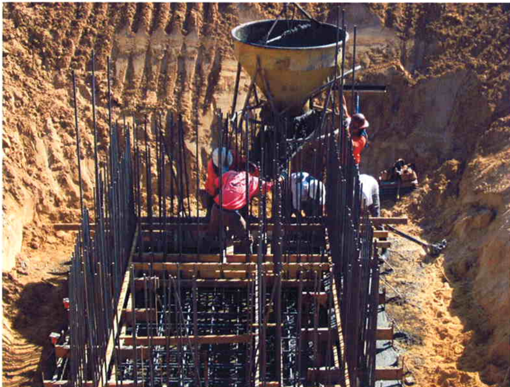
Cushman pouring foundation of Processed Water Pump Station.
