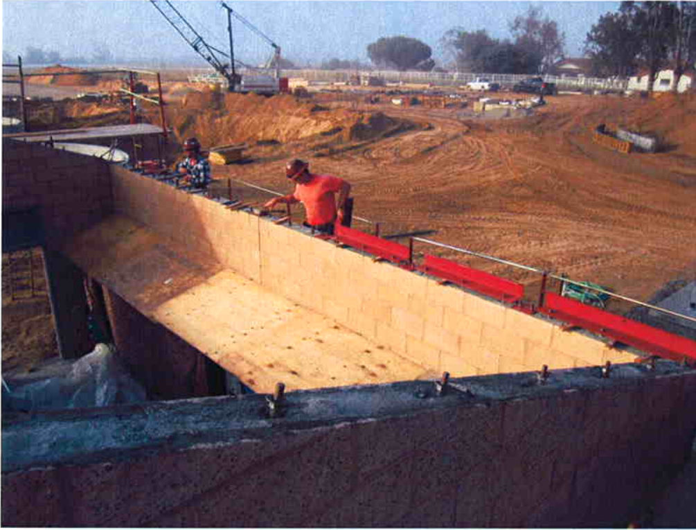
Cushman installing roof plate at Electrical/Blower Building.
