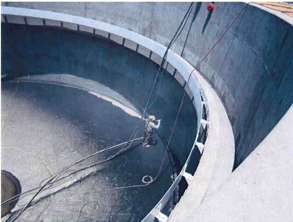
Subcontractor KNK Coating sandblasting the surface of Clarifier #2 in preparation for applying Xypex coating.
