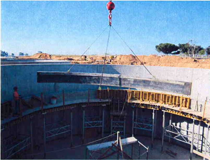
Setting forms in Clarifier #2 for last launder pour.
