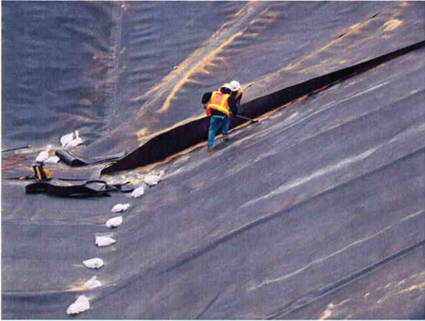
Barber-Webb clearing the liner in preparation for double fusion welding.
