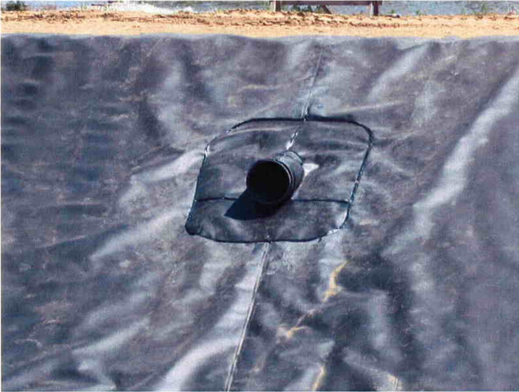
Final liner installation with extrusion weld around the pipe inlet of Aeration Basin #1.
