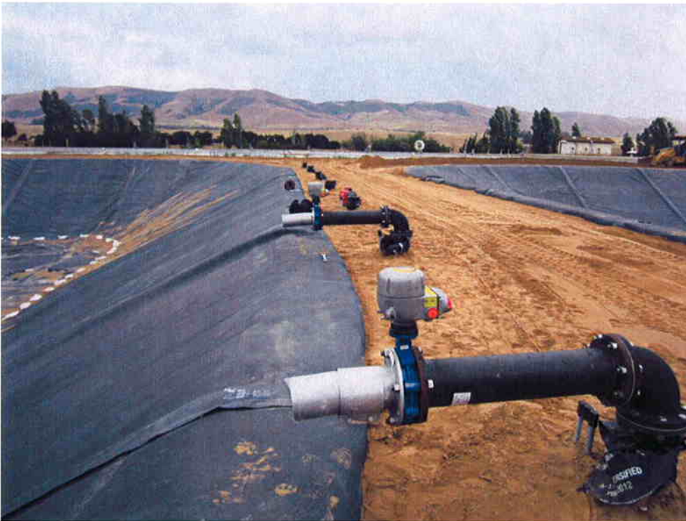
Above ground AR pipe risers and motorized butterfly valves being installed.
