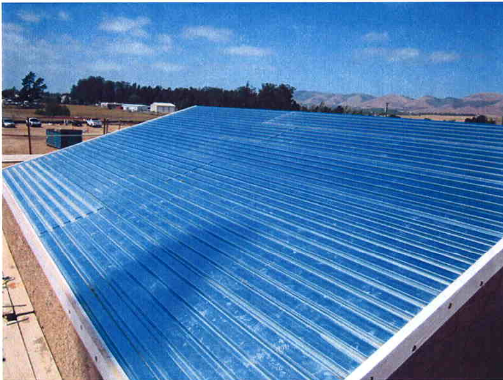
Metal decking installed before crimping.
