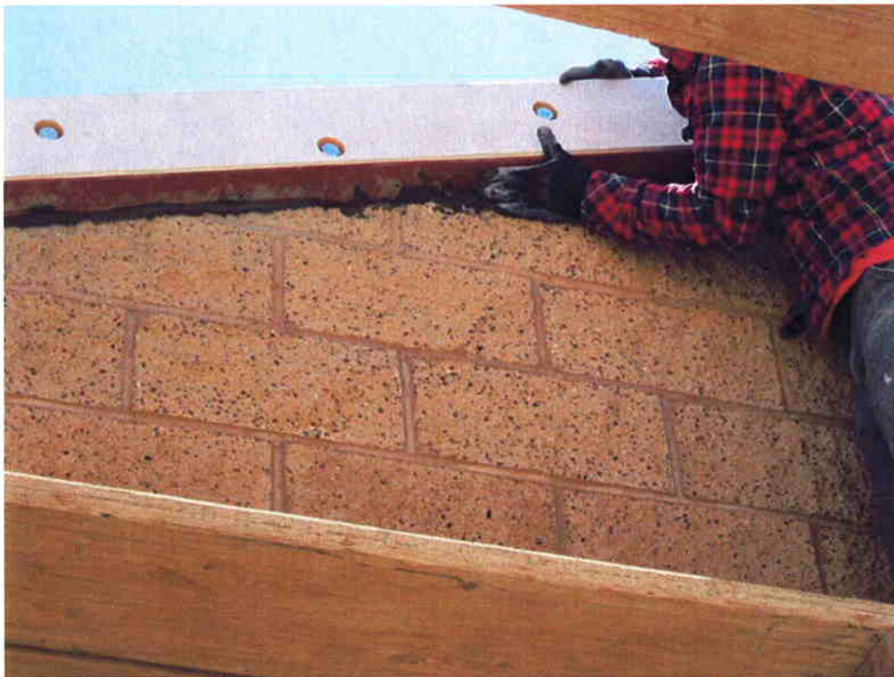
Cushman dry packing space between masonry and roof plate.
