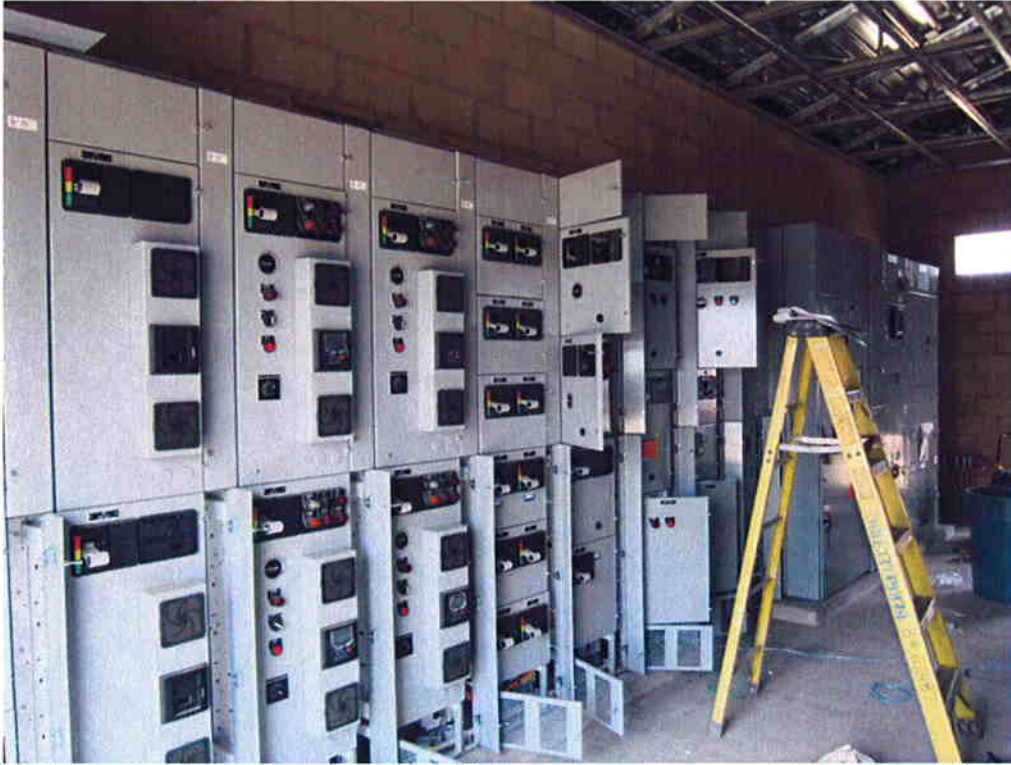
Motor control center equipment installed.
