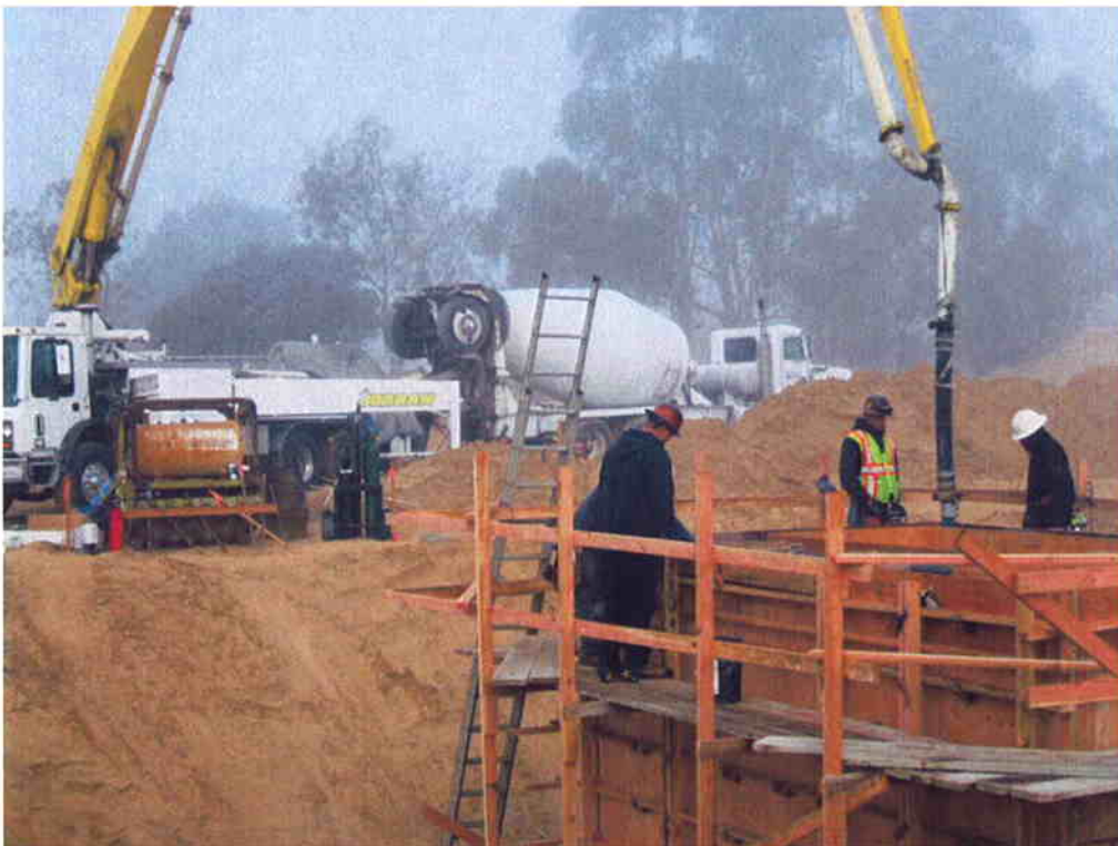
Cushman pouring walls of the Processed Water Pump Station.
