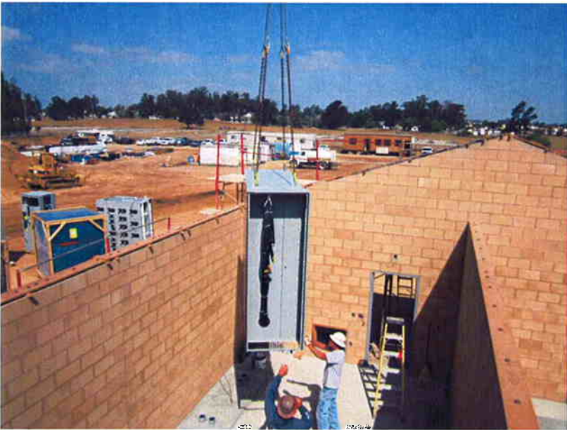
Hoisting electrical equipment into building before installing the roof.
