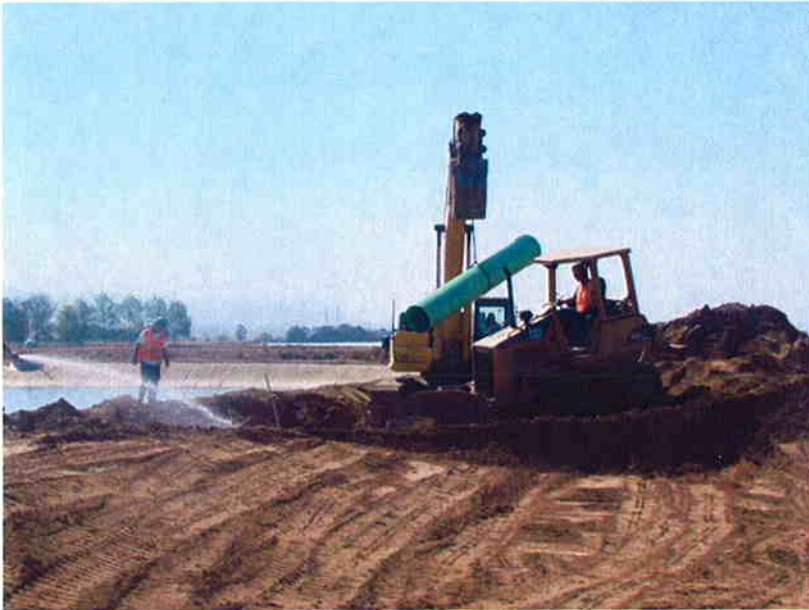
Installing 24" SE2 pipe at north end near existing Pond #4.
