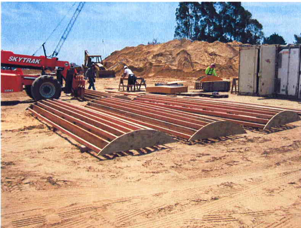
Cushman building forms for the circular interior of the Scum Well.
