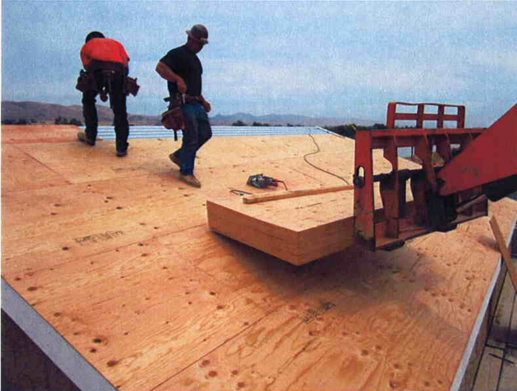
Cushman installing plywood sheeting over metal decking.
