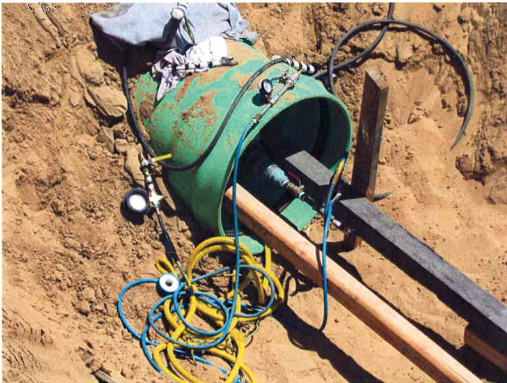
Pressure testing the 24" SE2 pipe.
