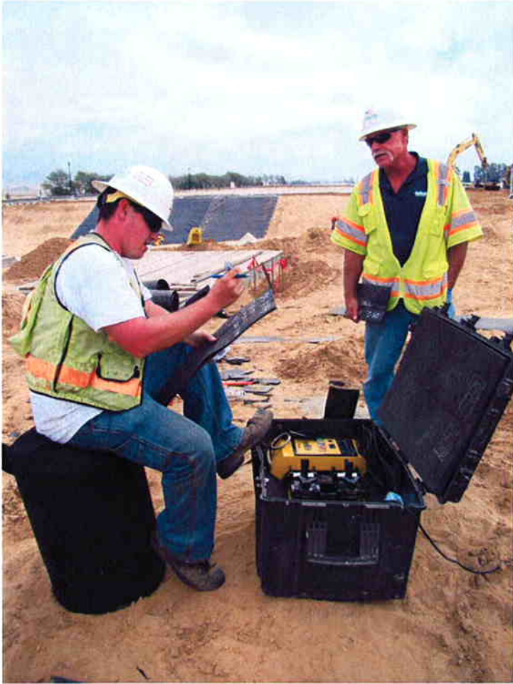
Field testing and inspection of destructive double fusion weld samples.
