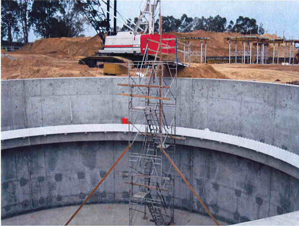
Cushman building scaffolding for access into Clarifier #2.
