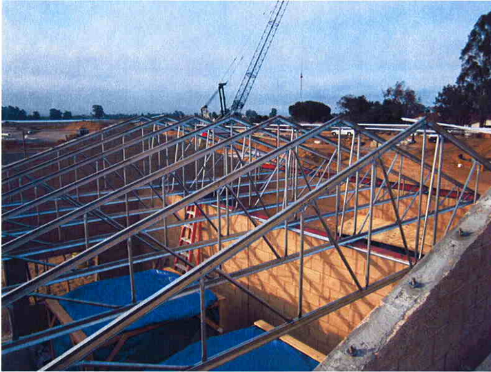
Metal roof trusses installed.
