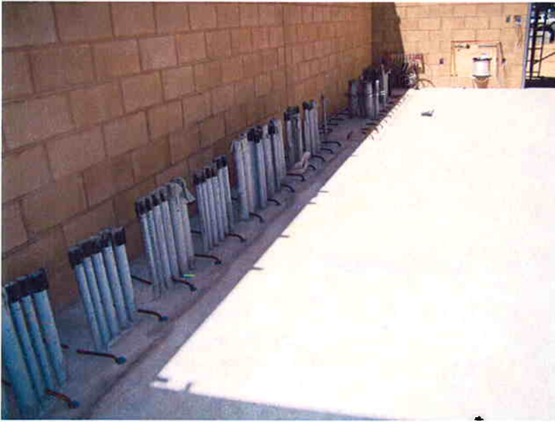
Conduit and epoxy dowels set for pouring electrical equipment pad.
