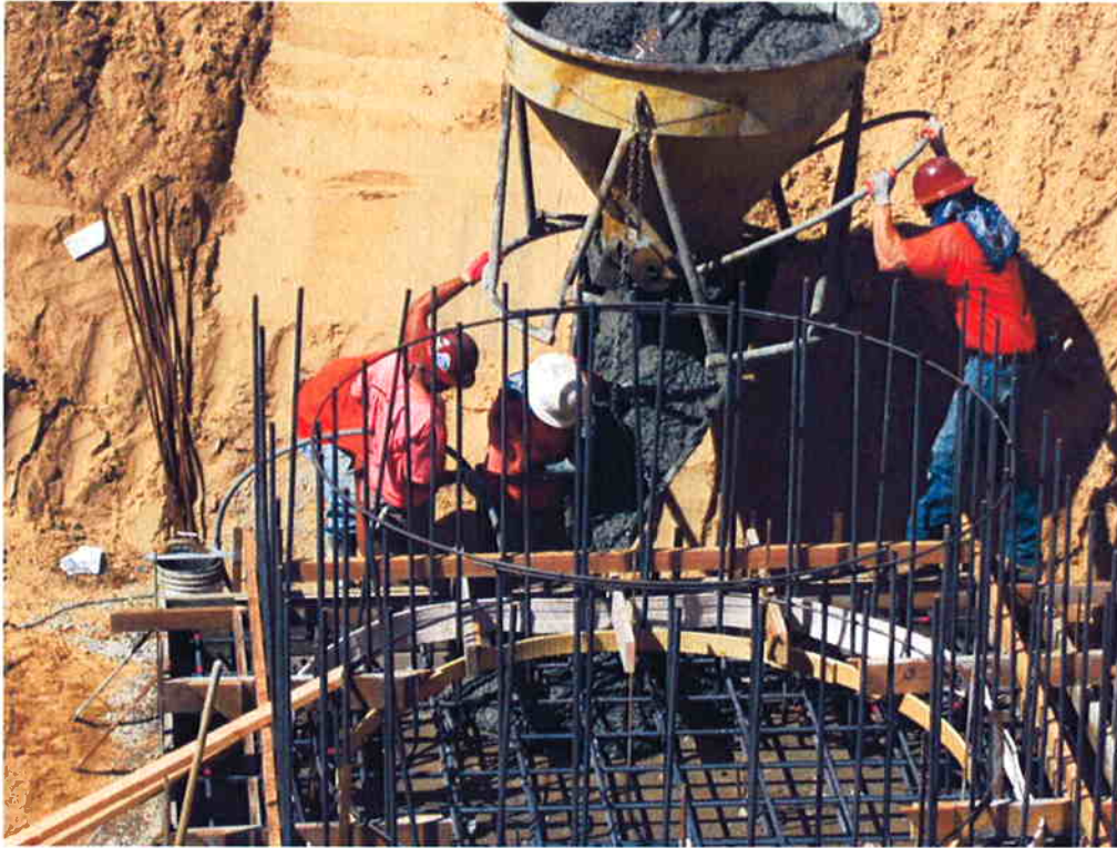
Pouring foundation of the Scum Well.
