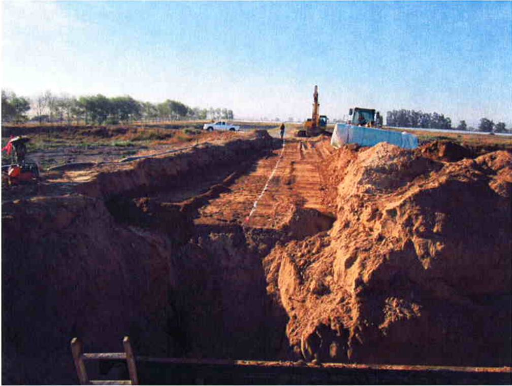
Laying out 24" SE2 pipe toward DWR easement crossing.
