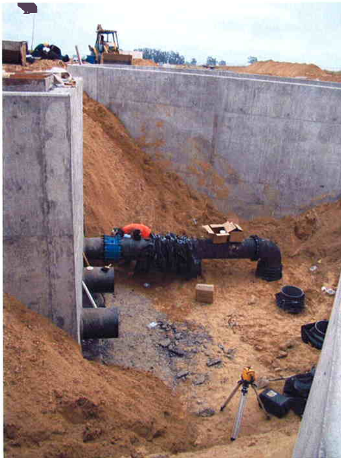
18" ML piping being installed out of Distribution Box #2.
