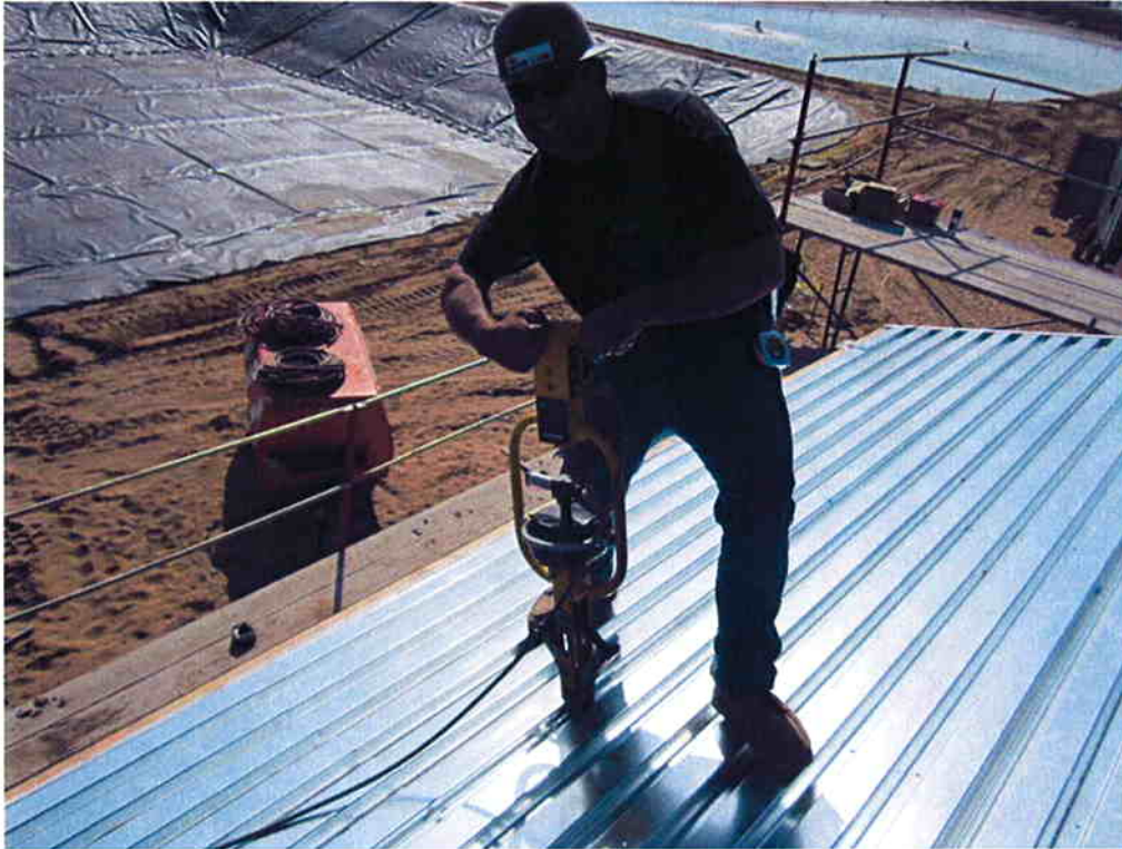
Cushman crimping metal decking with pneumatic crimper followed by puddle welding.
