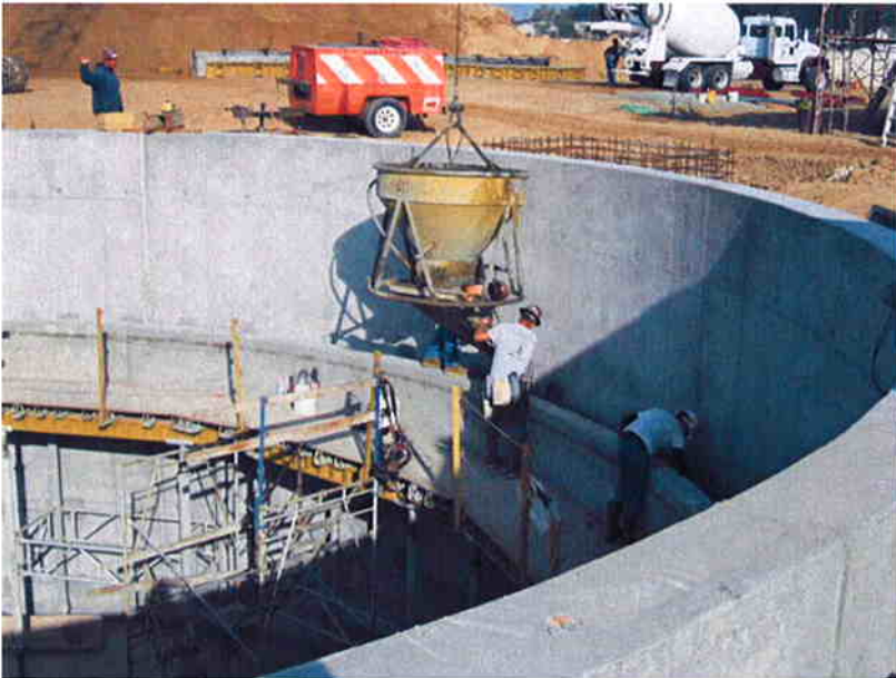
Cushman pouring concrete for launder floor in Clarifier #2.
