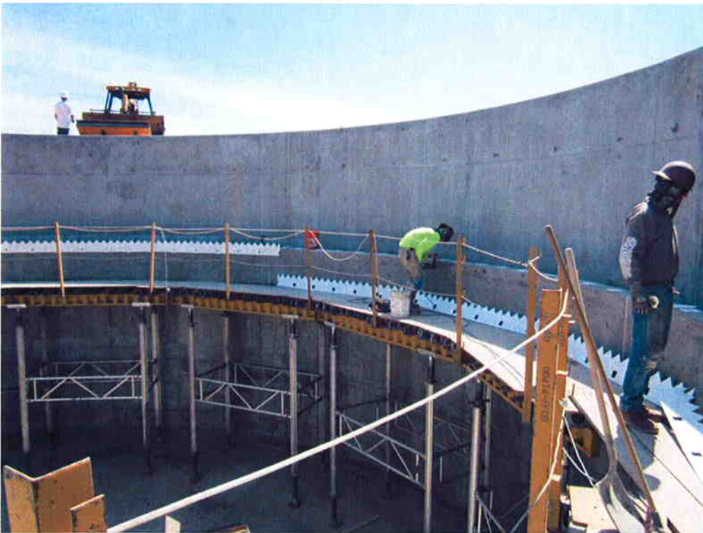
Installing toothed weir plate in Clarifier #2.
