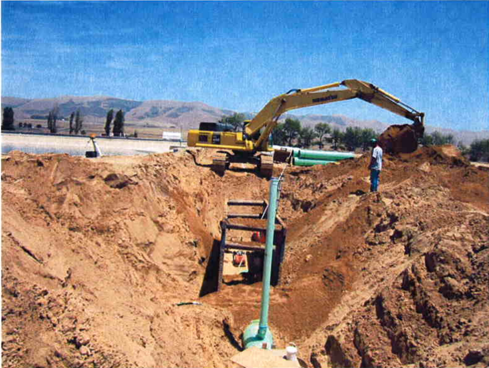
Cushman installing 24" SE2 pipe going east along the south end of Pond #4. Pipe riser is for pressure cleanout.
