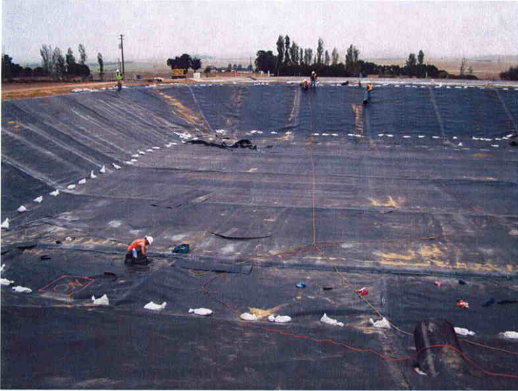
Liner installation and testing at Aeration Basin #1.
