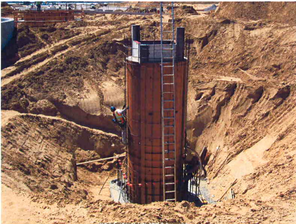
CMC Rebar installing rebar for Scum Well walls.
