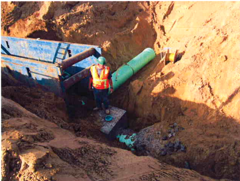
Thrust block installed on 24" SE2 pipe.
