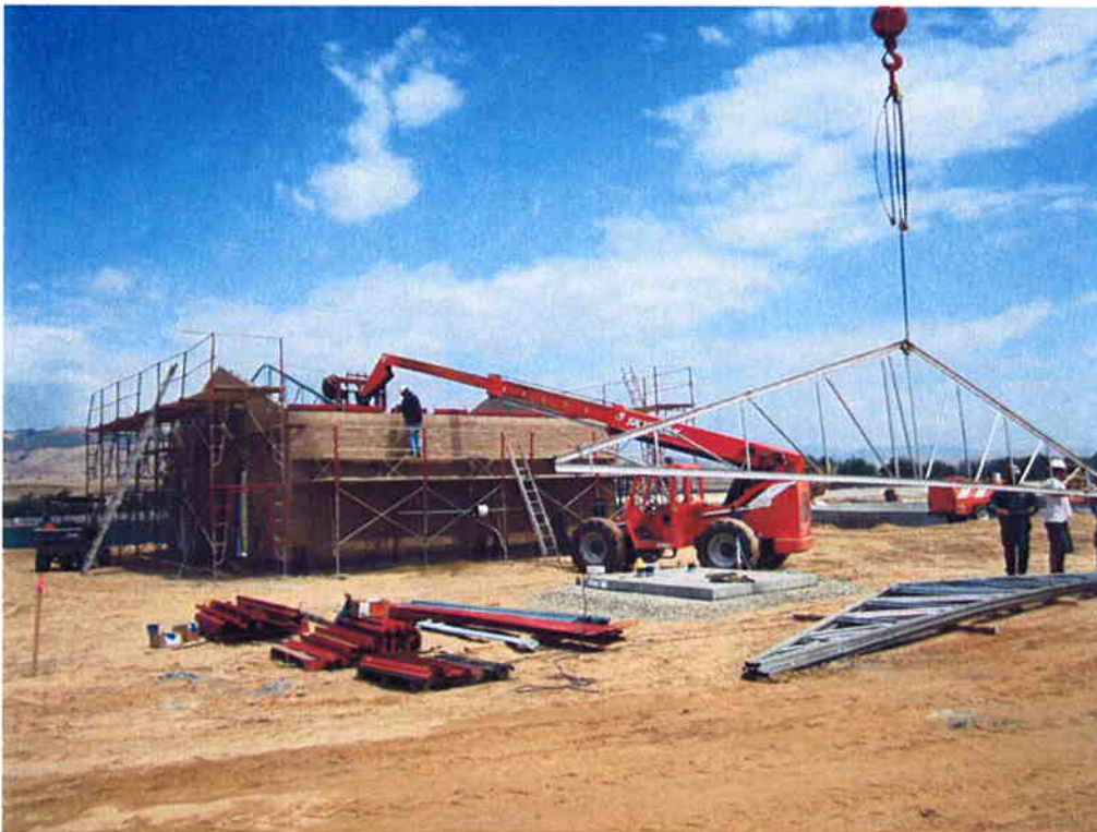
Cushman installing metal roof trusses.
